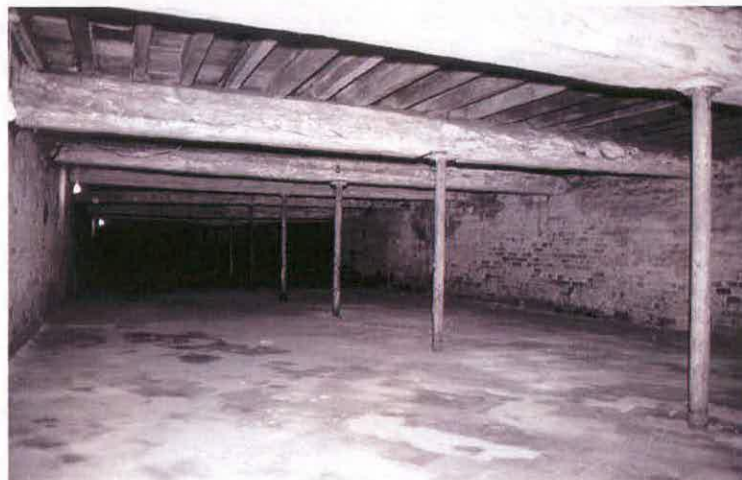
Figure 34 Range 8. View of ground floor
