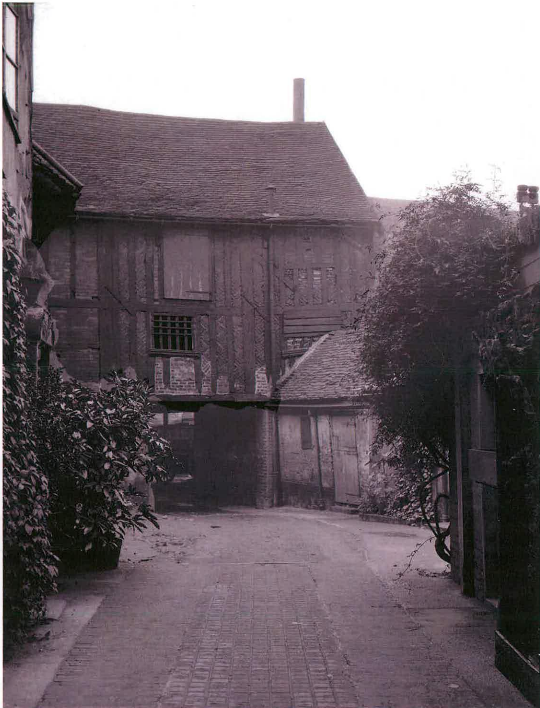
Figure 26 Pre-war photograph of Crossway, showing single-storey outhouse destroyed by enemy bombing
