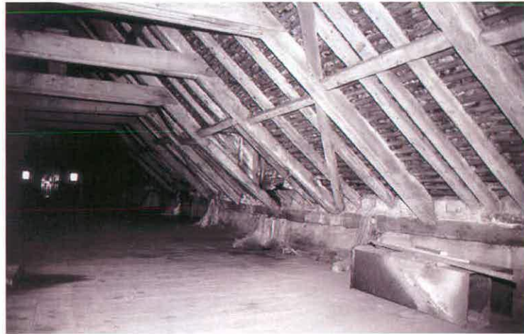
Figure 32 Range 8. Interior of attic showing roof construction
