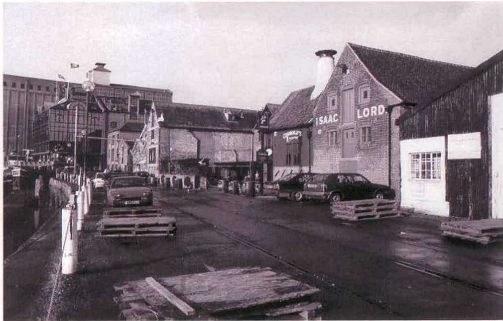
Figure 35 General view of quayside showing part of ranges 7, 8 and 11
