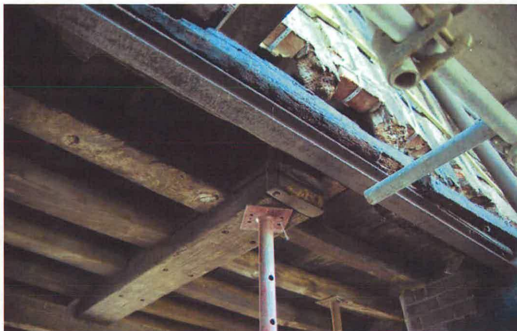
Figure 28 Detail of underside of carriageway through the Crossway
