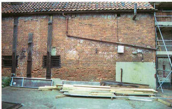
Figure 24 South wall of range 5, showing change in brickwork
