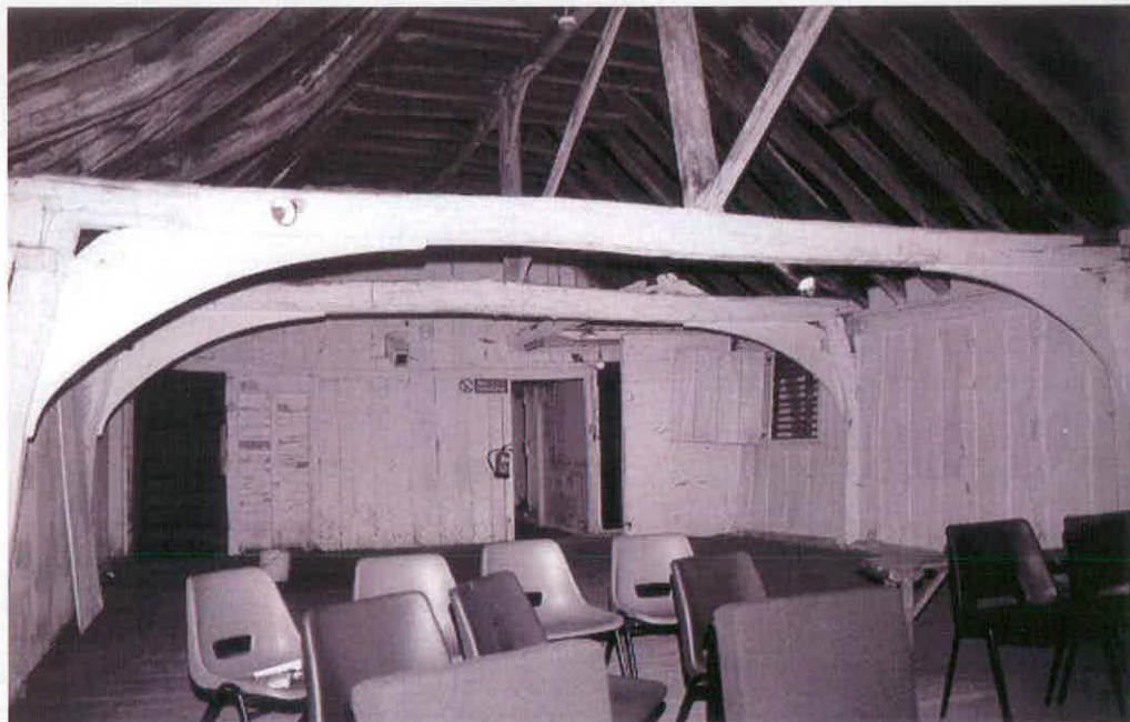
Figure 22 Range 3 (Sale Room). View of first floor looking south
