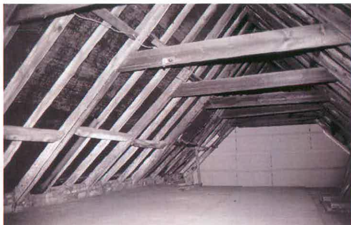
Figure 25 Range 5. View of roof construction
