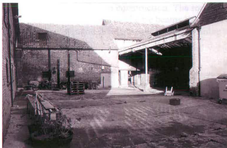
Figure 26 View of south courtyard, looking northwards towards range 5.
