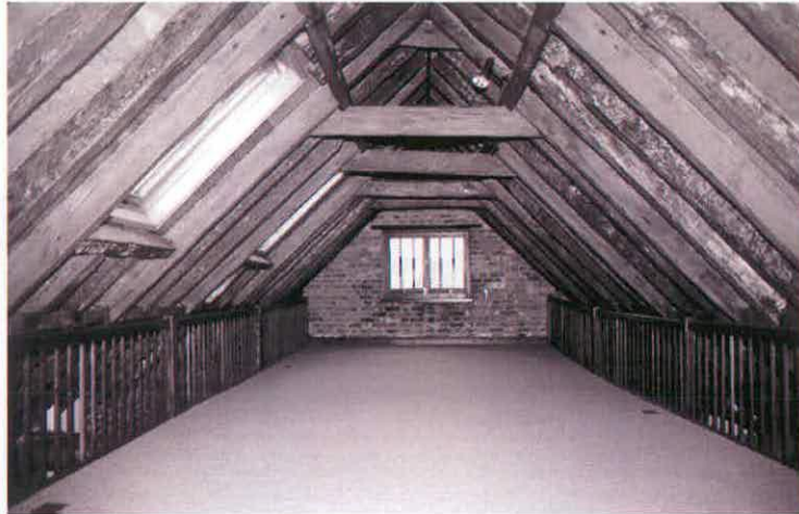
Figure 28 Range 6. View of attic showing construction of roof
