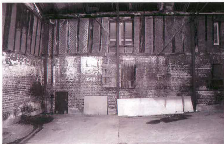
Figure 31 West elevation of range 8 showing exposed timber-framing at first floor
