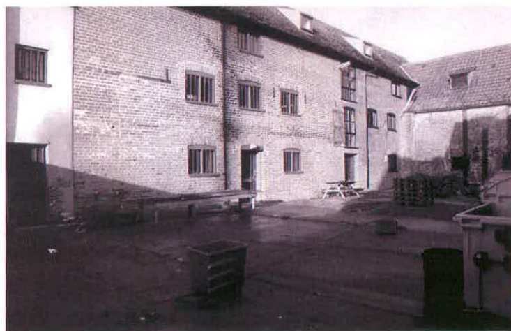
Figure 27 East elevation of Range 6, viewed from south courtyard
