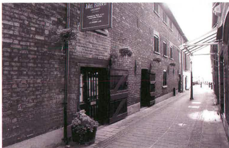
Figure 30 West elevation of range 7, looking southwards towards Common Quay
