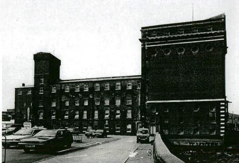
Fig. 10 – The east elevation of the East Mill, truncated to the north by the 1897 Silo, and raised to the south to create a water tower (EH,BB99/09872).
