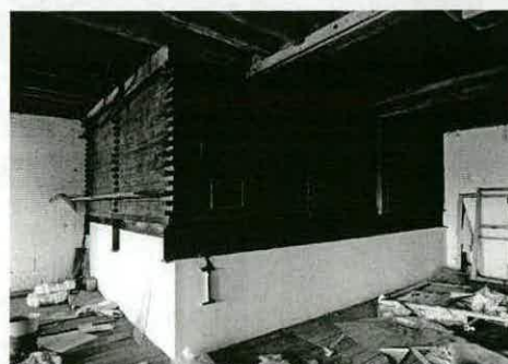
Fig. 19 – Lower portion of wood-wall silo visible on second floor (EH, BB/09893).
