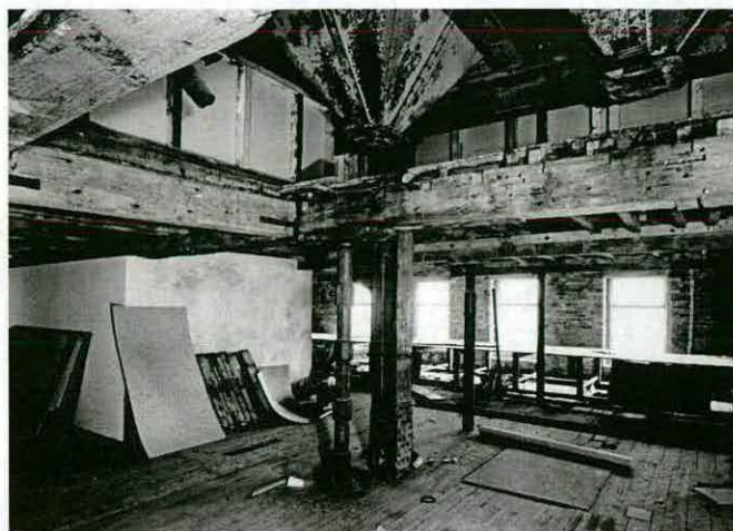
Fig. 17 – First floor of West Mill, looking south, showing reused props and steel hopper-bottoms (EH, BB99/09896).
