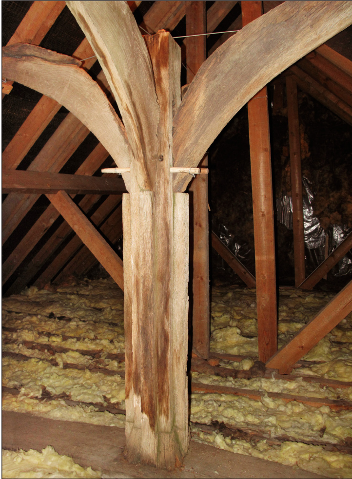
Figure 150 The surviving crown post at Waterloo House, West Fen Road (DP196872).
