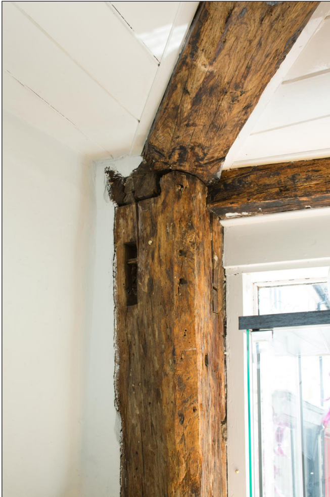
Figure 121 3a High Street Passage, corner post showing redundant mortice for head of shop window (DP173791).
