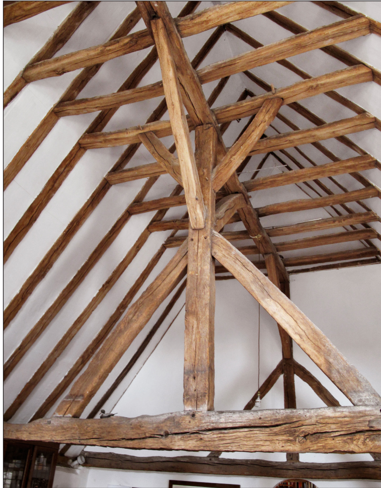
Figure 149 The crown-post roof at 41 Broad Street; The Three Blackbirds (Photograph Rebecca Lane © Historic England).
