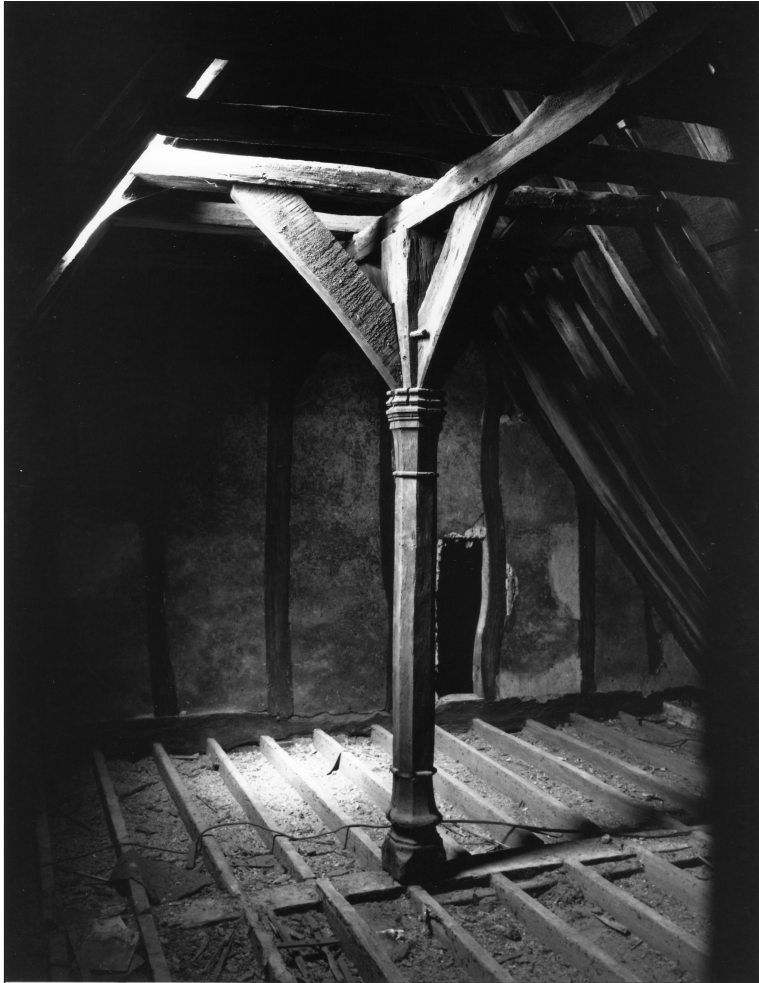
Figure 148 The crown post at 7-11 Silver Street (BB91/1889).
