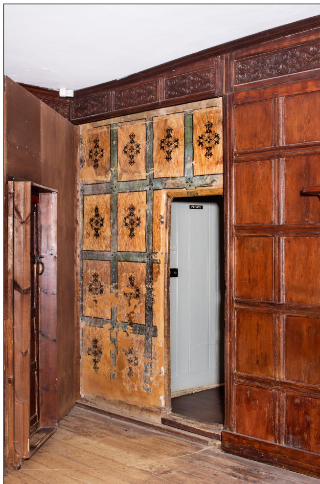
Figure 106 Oliver Cromwell's House, front range, detail of wall paintings in the eastern room, uncovered behind later panelling during restoration (DP195558).
