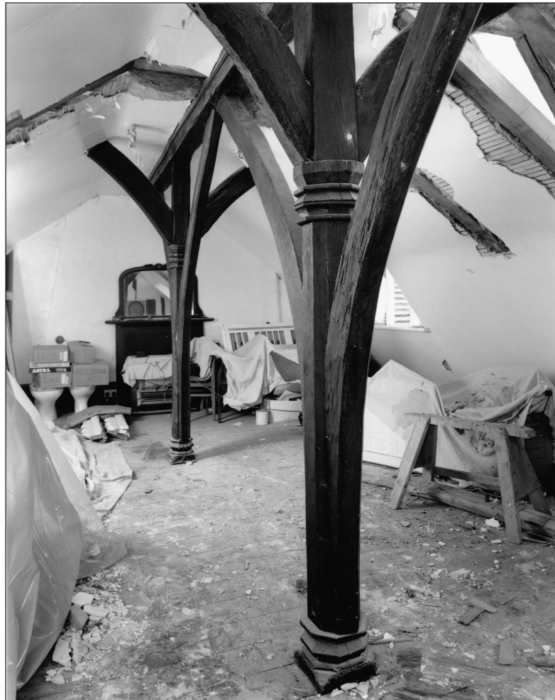
Figure 147 The crown-post roof of the Black Hostelry, within the monastic precinct (BB91/15528).
