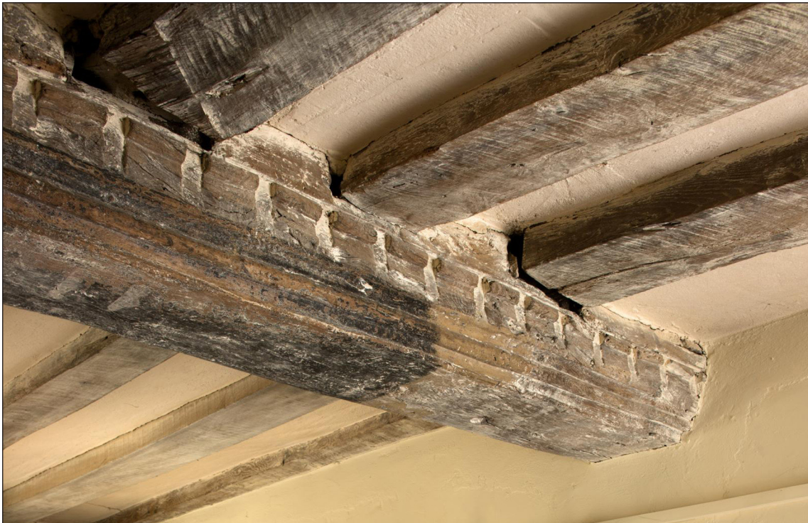
Figure 137 The crenellated spine beam at 48 St Mary's Street (DP187930).
