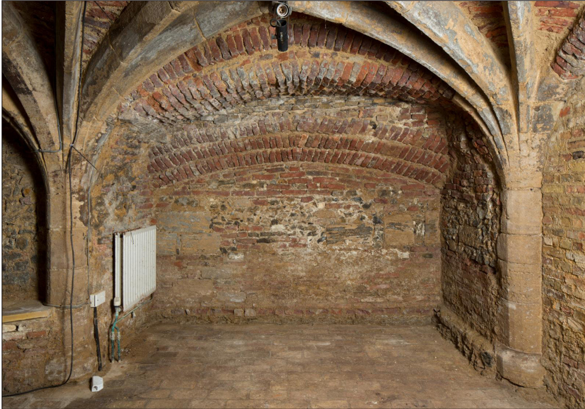
Figure 127 Undercroft under 16-18 High Street, stone recess in the south wall showing the use of early moulded brick (DP173483).
