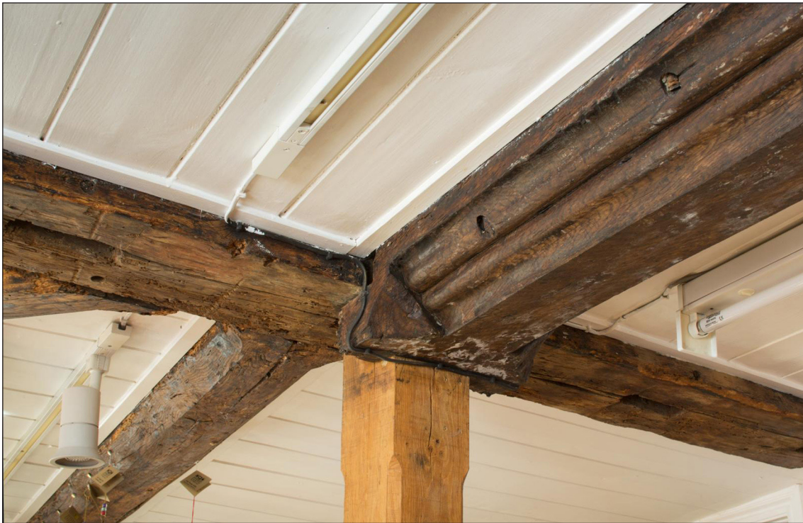
Figure 83 3a High Street Passage, detail of 16th century beam lapped onto the earlier cross beam (DP173792).
