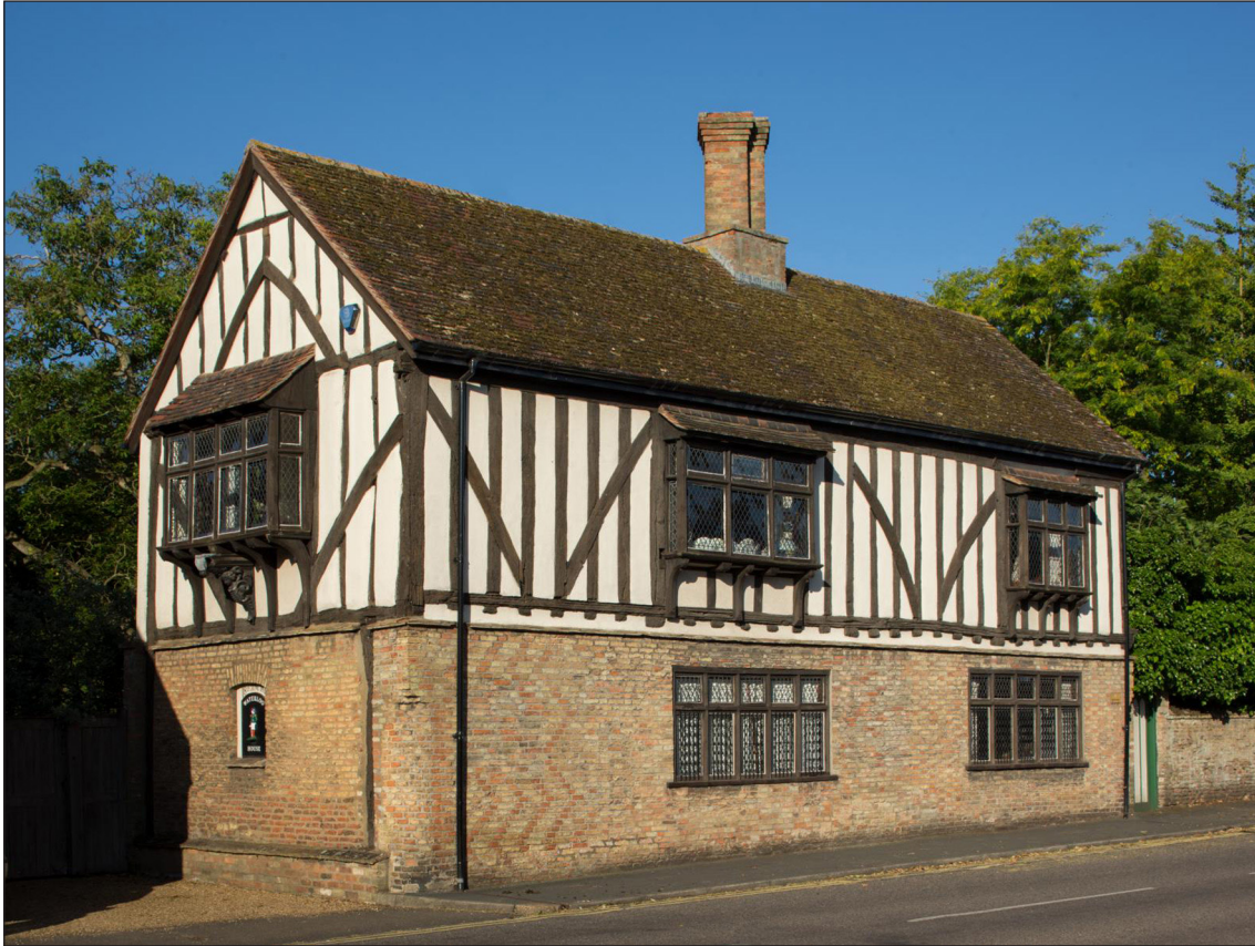
Figure 135 Waterloo House, West Fen Road showing the close studding that originally typified many of the 15th and 16th century buildings in Ely (DP173855).
