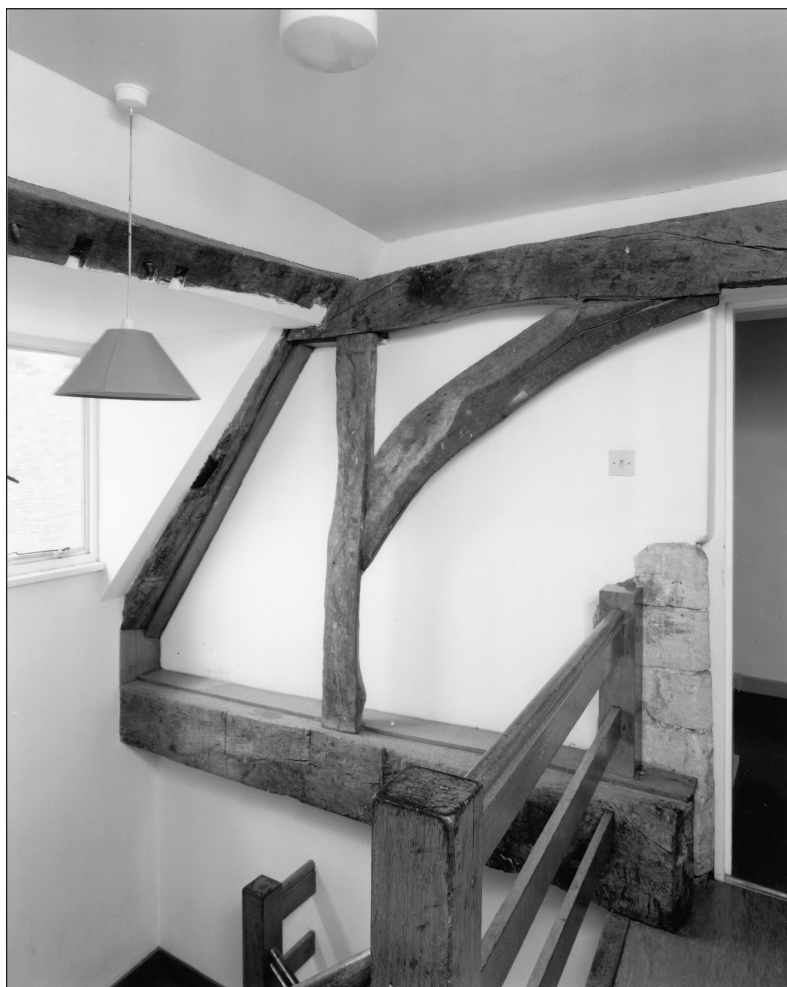
Figure 151 Part of the queen-post roof over the south section of the west range of the monastic precinct (BB98/20033).
