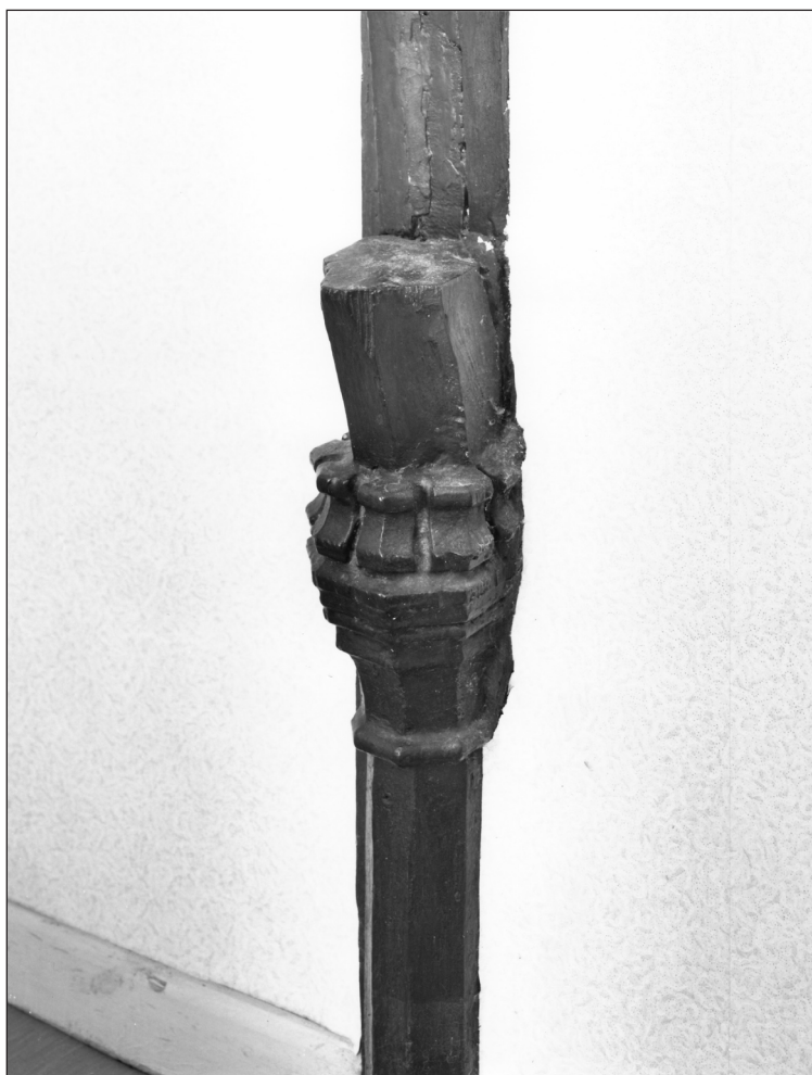
Figure 138 7-11 Silver Street, detail of the decorative treatment of the post supporting the central open truss (BB91/1887).
