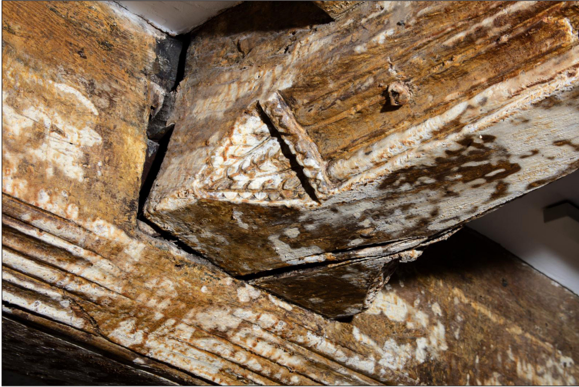
Figure 141 33 High Street, detail of the foliate design on the chamfer stops (DP187931).
