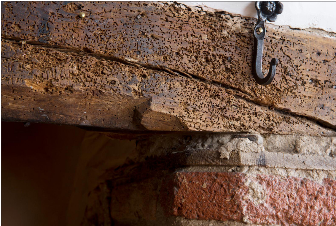
Figure 97 2 Waterside, detail of chamfer stop to fireplace bressumer in the west bay (DP173823).
