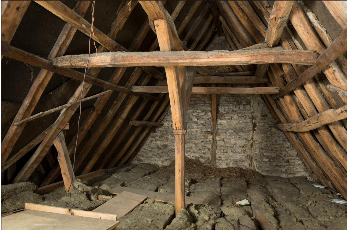
Figure 133 The 14th century roof at 23 Broad Street which incorporates some original pine rafters (DP173787).
