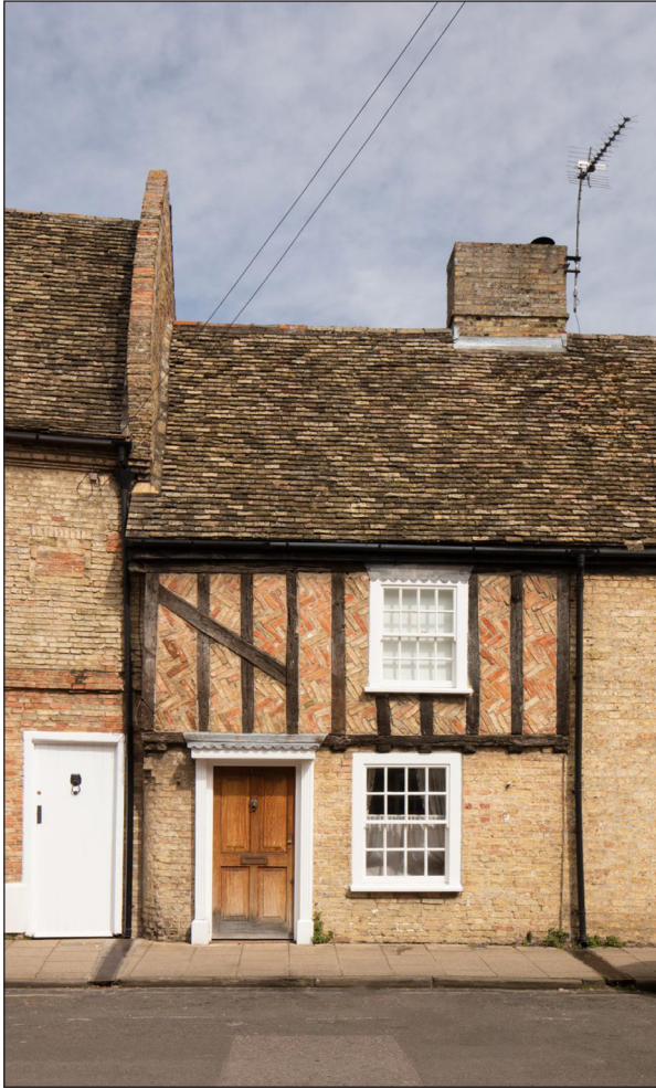
Figure 136 15 Waterside showing the use of close studding a building of the 16th century (DP187981).
