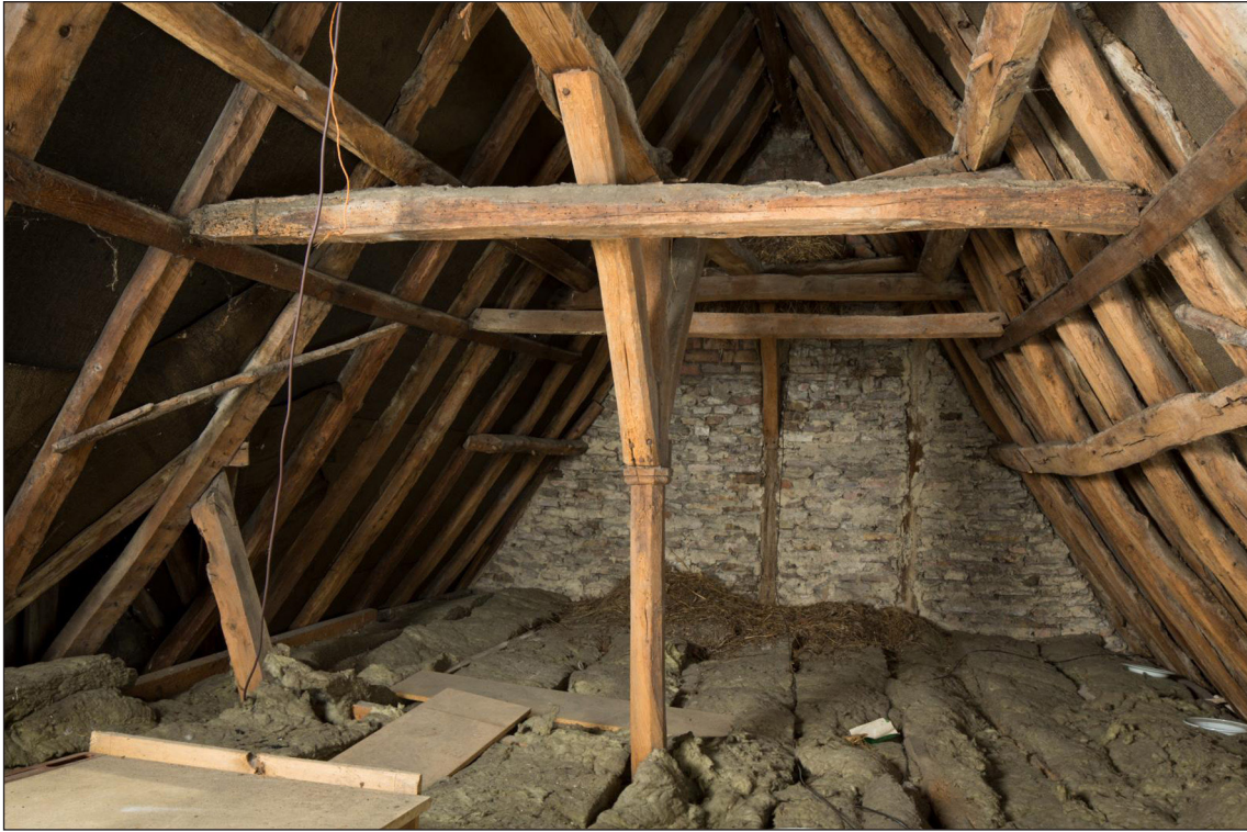
Figure 146 The 14th-century crown-post roof at 23 Broad Street (DP173787).
