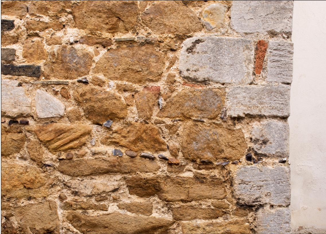
Figure 123 Detail of wall using clunch, Oliver Cromwell's House (DP195556).
