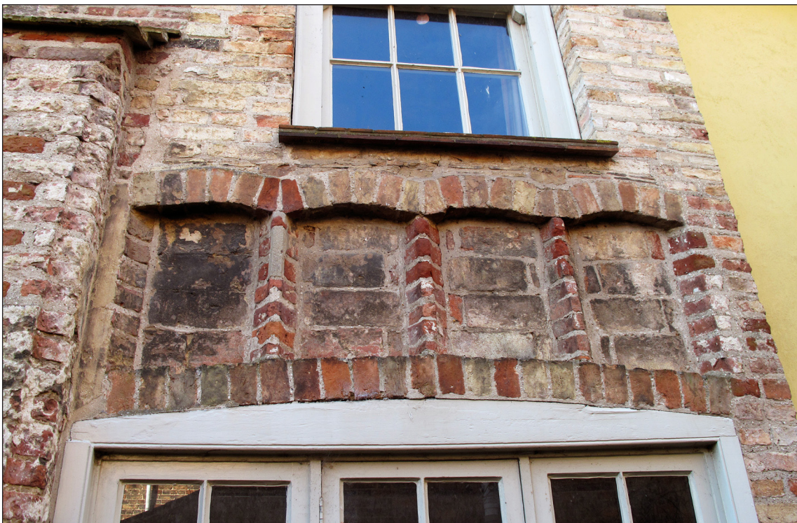
Figure 128 41 Broad Street, The Three Blackbirds, detail of 15th century brickwork forming the hall window (Photograph Rebecca Lane © Historic England).
