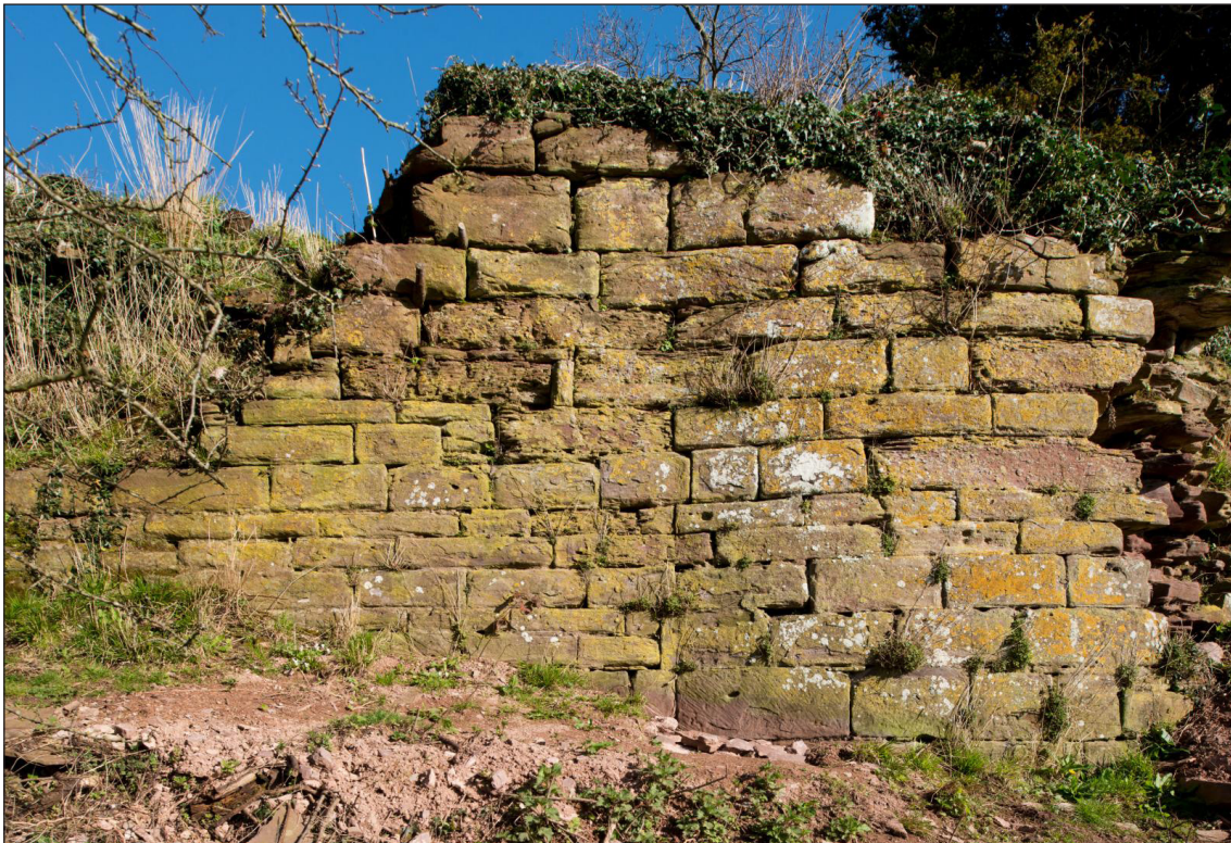
Figure 23 Part of the east section of the south curtain wall and the south east tower, view from south (DP195785).
