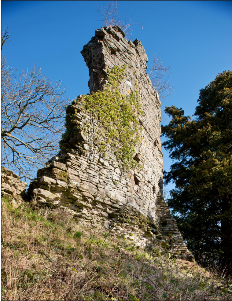
Figure 5 Southeast corner of the tower showing the remains of the plinth at ground floor level (DP195780).
