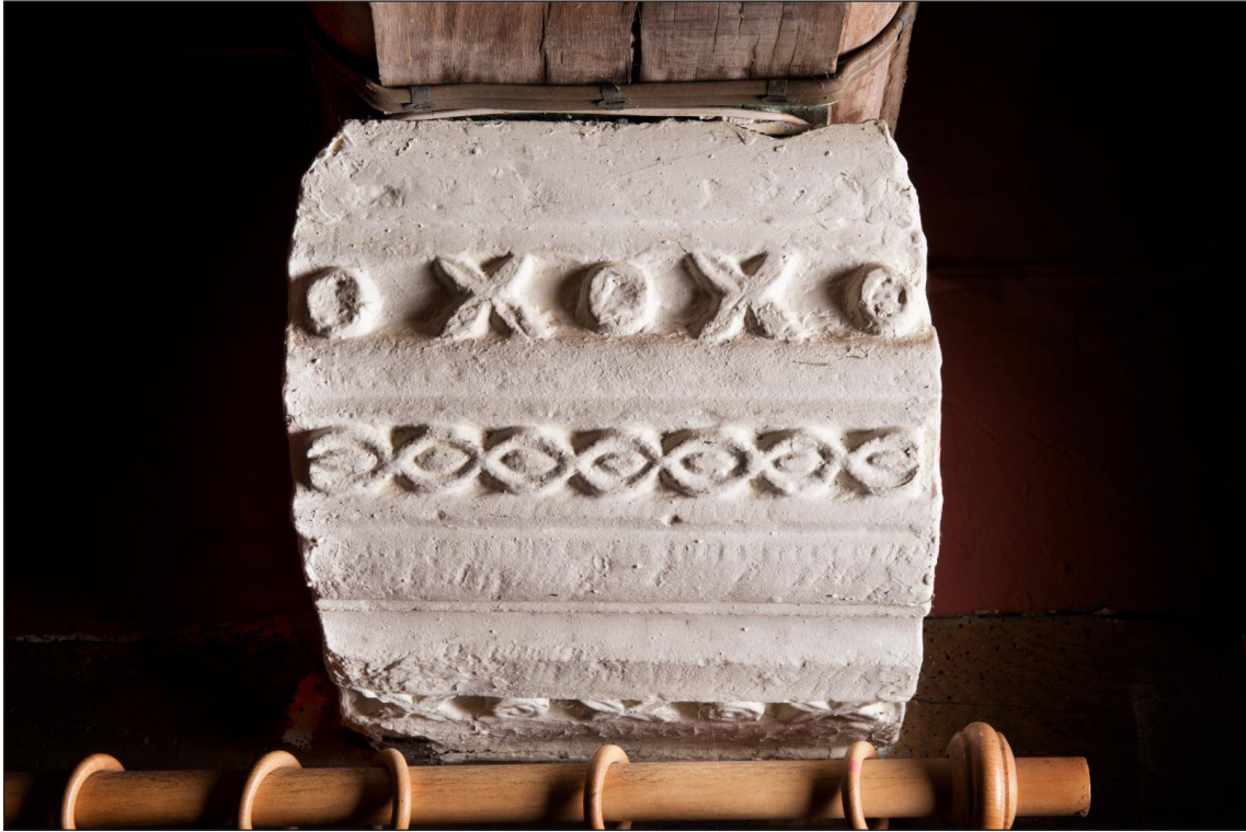
Figure 27 Snodhill Court, one of the corbels supporting the eastern end of the cross beams in the hall (DP195435).
