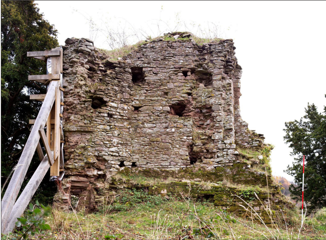
Figure 8 Internal elevation of the south-eastern corner of the tower, showing the offset between ground- and first-floor level (DP195363).
