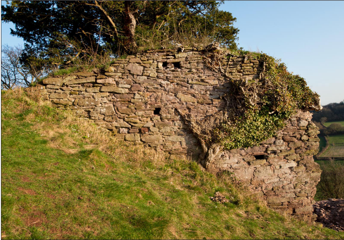
Figure 20 South wing wall, view from the north (DP195800).
