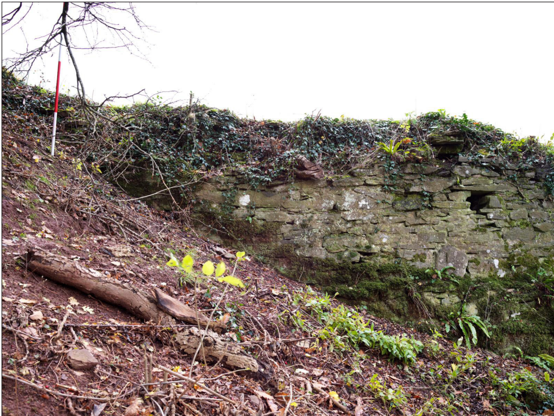
Figure 21 North wing wall, view from south (DP195360).
