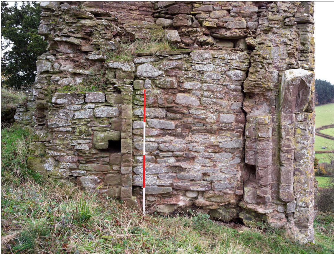
Figure 6 Ground floor entrance passage showing remains of door jamb (DP195368).
