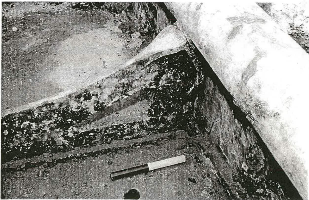
Main span crossbeam SE end
