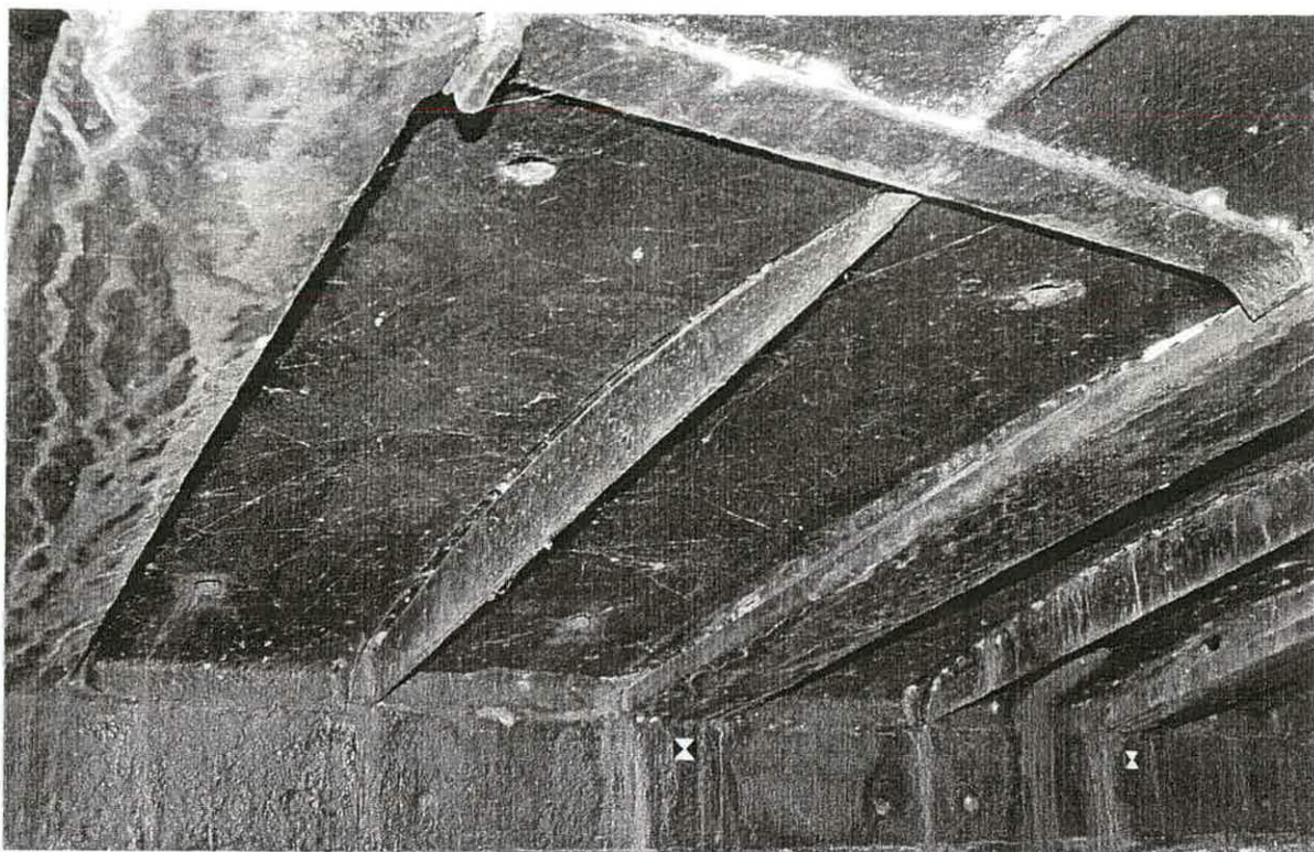
Main span, soffit adjoining seating on SW side
