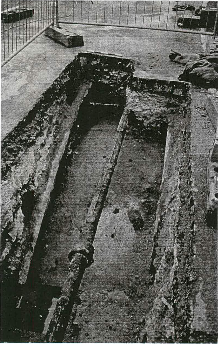
Side span, TP2 from SW
