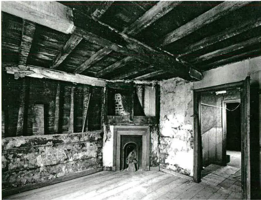
*Fig. 30 – Timber-framed construction visible in the front room, second floor, No. 76 Bermondsey Street (English Heritage, BB000118).*
