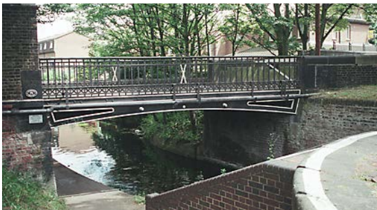
Grade II* Parnell Road Bridge and Three Colts Bridge 1830, cast iron girder and plate deck. (IoE 206529, 206526 Patricia Philpott)
