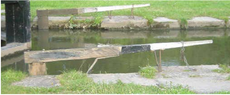
Rufford Branch – unusual paddle mechanisms: wooden levers lifted into a vertical position to open the paddle and horizontal rotating handles. ( www.penninewaterways.co.uk )
