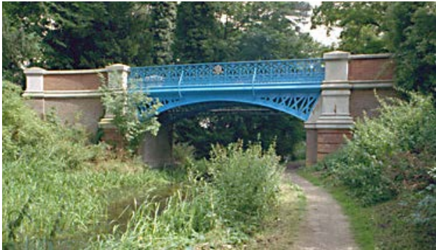
Bridge over Wendover Arm of Grand Union Canal in grounds of Halton House, c.1880 cast iron (IoE 42654 Alistair F Nisbet)
