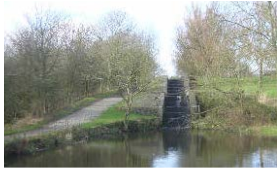
(Left) Waterhouses Aqueduct over River Medlock on Hollingwood Branch (IoE 212440, Pamela Jackson): (Right) Hollingwood Branch The second and third locks formed an unusual lock staircase, with three gates. On the hillside to the right was a pumping station, where a James Watt beam engine pumped water back up to the higher level. ( www.penninewaterways.co.uk )
