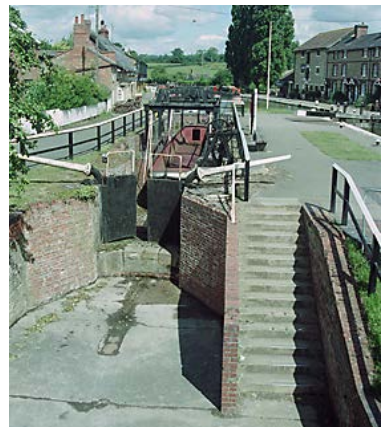
(Right) Marsworth Canal lock of c.1800, with dry dock, built as a narrow duplicate lock 1838-9, altered later C19. (IoE 42089 Nick Jarvis)
