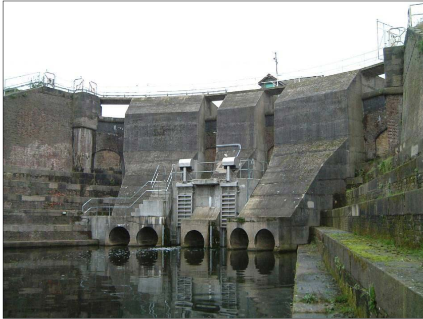
Photograph 5: Siphons at Brent Reservoir
