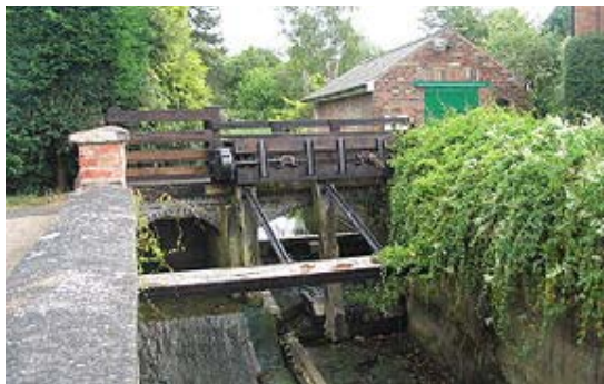
Old sluice gate, Asfordby (Wikipedia Tim Heaton)
