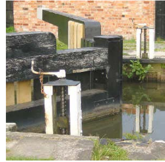
Rufford Branch – unusual paddle mechanisms: wooden levers lifted into a vertical position to open the paddle and horizontal rotating handles. ( www.penninewaterways.co.uk )
