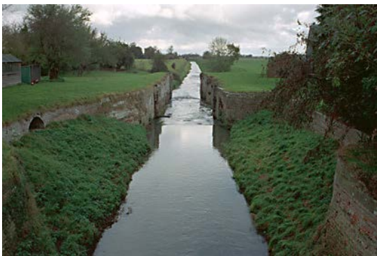
(Left) Alvingham Lock and basin (1767). The river Ludd, is culverted and passes under the lock by means of an inverted syphon (IoE 195450 Trevor Sowray)
