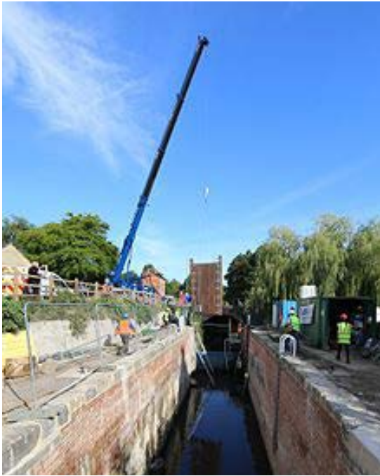
Gates being fitted to Bowbridge Lock as part of restoration phase 1a (Wikipedia Geni)
