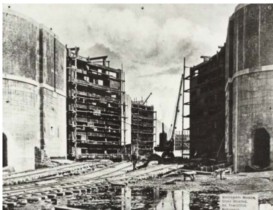
Manchester Ship Canal Eastham Locks under construction (Waterways Archive BW192/3/2/1/1 5/4BW192/3/2/1/15/4)
