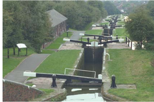
(Left) Lock No 9 lock formed a staircase with lock 10, although addition of a top gate to lock 10 has formed two locks separated by a short pound. Still effectively operates as a staircase. (IoE 442662 Colin Cundy)
