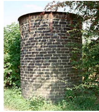
(Right) Airshafts above Barnton Tunnel (IoE 449370 R.G. Noxon) and Preston Brook Tunnel (IoE 429730 Keith Walker)
