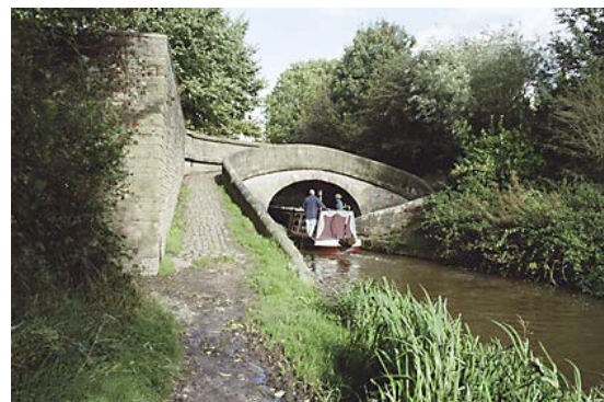
(Left) A skew bridge with segmental archway, Black Road, Macclesfield, (IoE 391032 Patricia Layhe)
