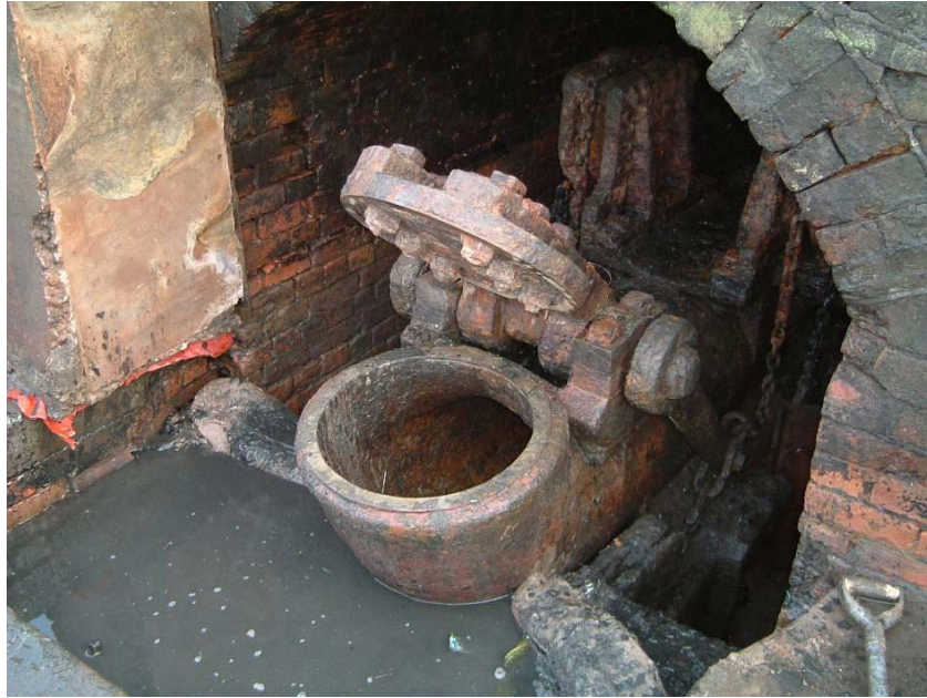
Photograph 7: Tea pot lid valve exposed for works at Rotton Park Reservoir
