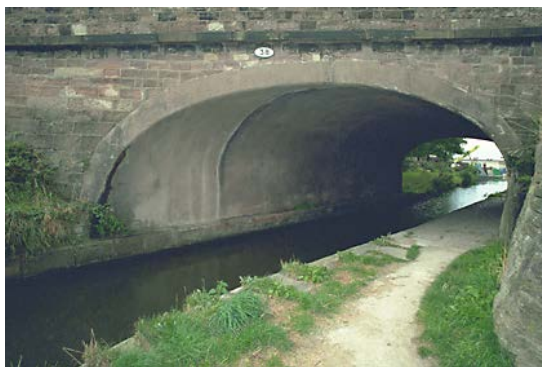
(Left) A skew bridge with segmental archway, Black Road, Macclesfield, (IoE 391032 Patricia Layhe)
