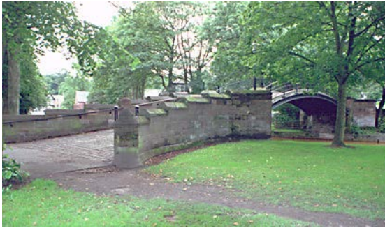
Footbridge between Barton Road and The Green, Worsley 1901. Built for the 1st Earl of Ellesmere. Wrought iron with dressed stone abutments. (IoE 211988 Patrick Norris)
