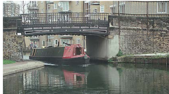
Grade II* Parnell Road Bridge and Three Colts Bridge 1830, cast iron girder and plate deck. (IoE 206529, 206526 Patricia Philpott)
