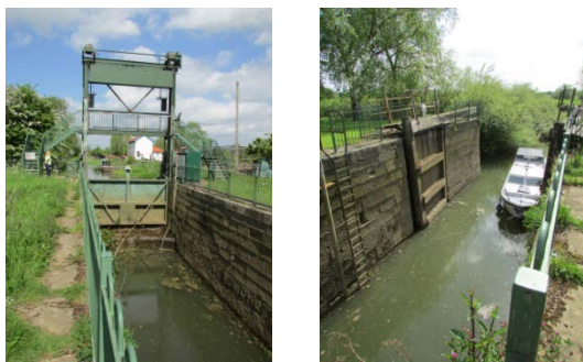
Elvington Lock 2015 Upper and lower gates (Keith Falconer)
