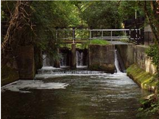
The disused Stoke lock, which now functions as a weir and sluice (Wikipedia Pedro)
