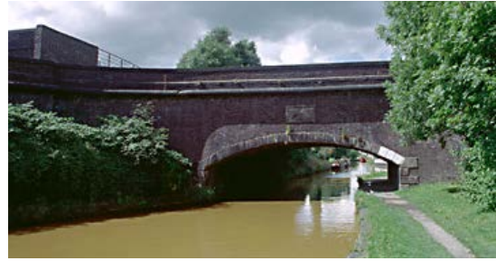
(Right) Pool Lock Aqueduct carrying the Macclesfield Canal over the Trent and Mersey Canal. Dated 1829. (IoE 56499 J M Pickering)
