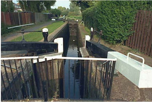
(Left) Lock No 9 lock formed a staircase with lock 10, although addition of a top gate to lock 10 has formed two locks separated by a short pound. Still effectively operates as a staircase. (IoE 442662 Colin Cundy)
