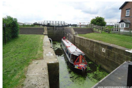
West Haddlesey Flood Lock. The far gates are tall to protect the canal from flooding when river levels are high. ( www.penninewaterways.co.uk )
