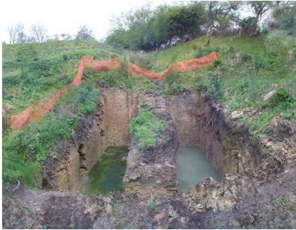
Excavation of Fussell's Trial Balance Lock (Dorset & Somerset Canal Society)
