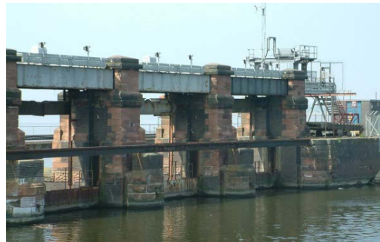
(Right) Sluices discharging water from the River Weaver into the Mersey (Wikipedia Peter Hodge)
