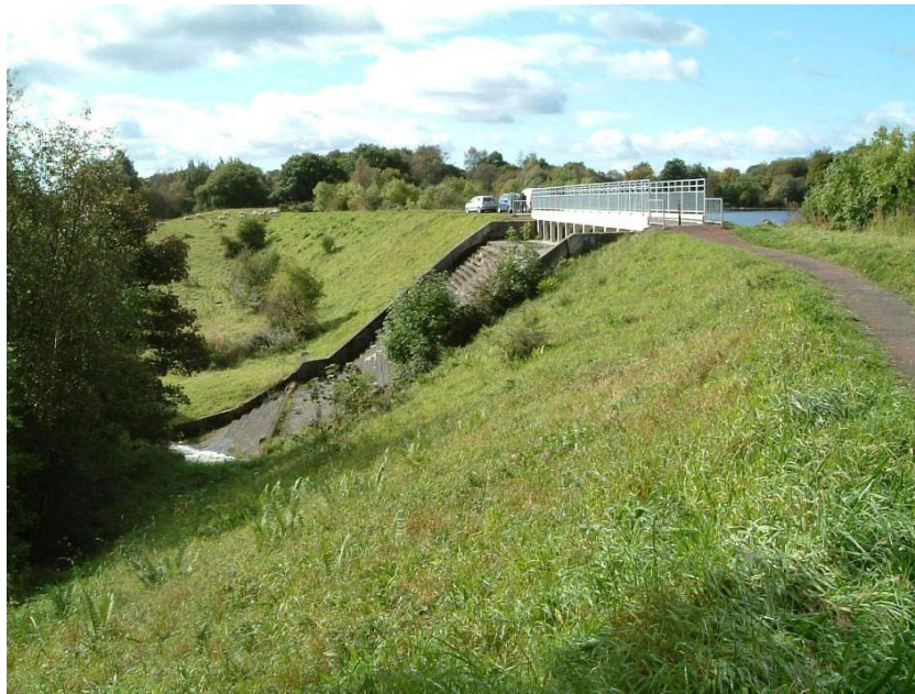
Photograph 1: Townhead Reservoir, showing the auxiliary spillway of 1934
