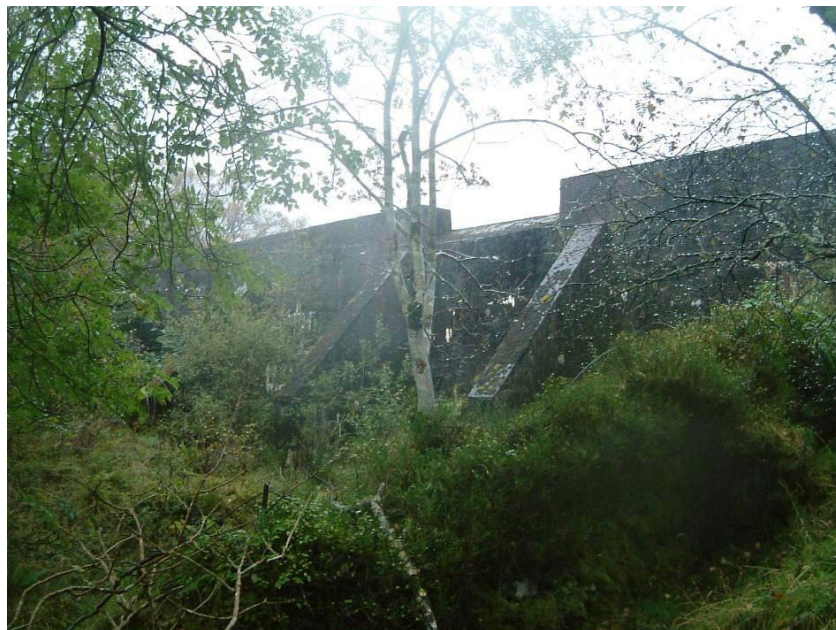
Photograph 2: Loch na Bric – concrete buttress dam
