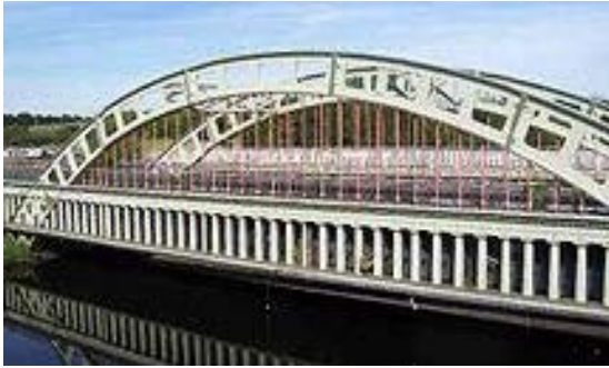
Stanley Ferry Aqueduct (Wikipedia Chris55)
