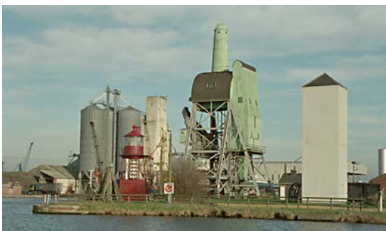
Hoist and Accumulator Tower, South Dock Goole (IoE 165281 Les Waby)
