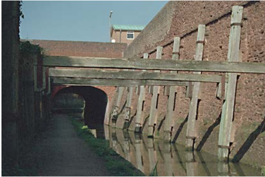
Albert Street Cutting, Bridgwater (IoE 374026 Michael Bass)
