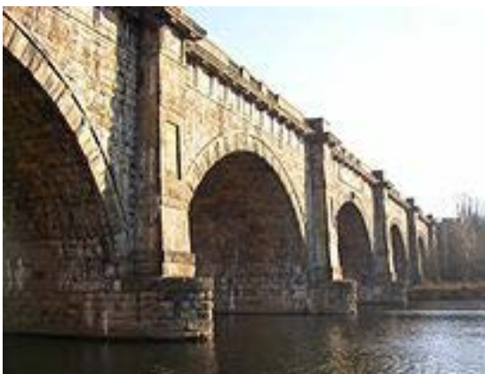
Lune Aqueduct (Wikipedia Humphrey Bolton)
