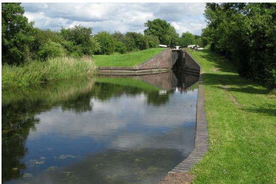
Droitwich Junction canal, rebuilt Hanbury Locks (Wikipedia, geni)
