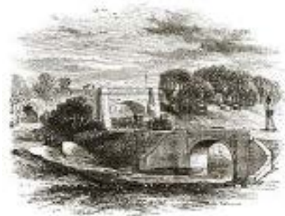
Bullbridge Aqueduct over the North Midland railway
