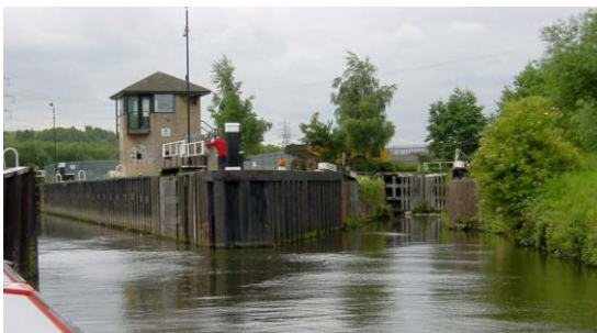
Kilnhurst Lock, with the older, disused lock to the right. ( www.penninewaterways.co.uk )
