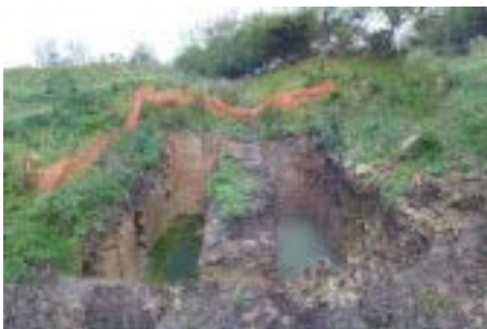
Excavation of Fussell's Trial Balance Lock (Dorset & Somerset Canal Society)
