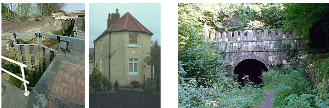
(Left) Northgate Locks Chester (IoE 469913 Michael J Tuck); (Centre) Tollhouse of original Delph flight 1779 (IoE 403768 Colin Cundy); (Right) Sapperton Tunnel North Portal (IoE 128352 E. Currier)
