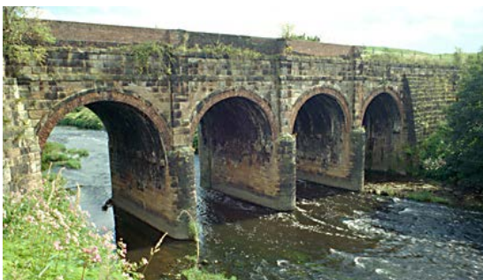
Prestolee Aqueduct over River Irwell (IoE 210525 David H Swain)
