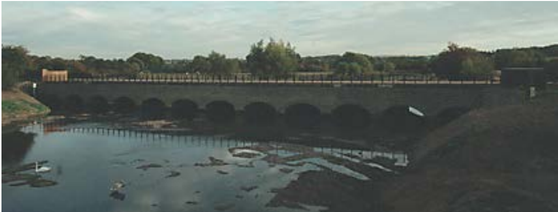
Trent & Mersey Canal Aqueduct at Egginton (IoE 82704 Geoffrey R Hood)
