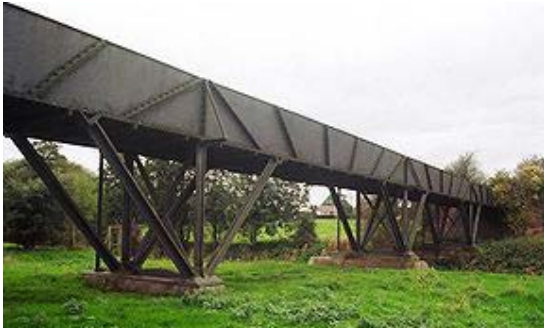
Longdon-on-Tern Aqueduct (Wikipedia Priewis)
