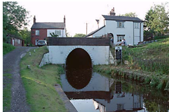
South portal, Preston Brook Tunnel (IoE 436331 Keith Walker)
