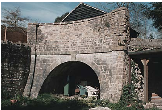
(Left) South west entrance to Wellow Tunnel (IoE 32365 John Peters)
