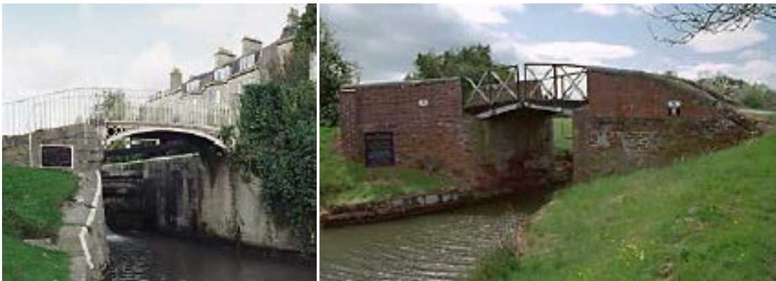
K & A Canal Widcombe Bath (IoE 442752 Micaela Basford) Canal Bridge Wootton Wawen Stratford Canal (IoE 482584 William S. Thorne)
