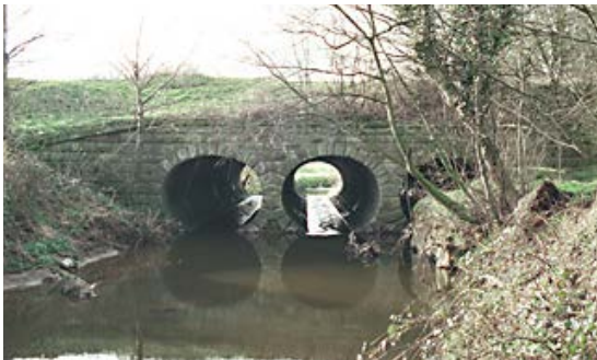
Hollowforth Aqueduct, Barton (IoE 185849 Peter Sargeant)
