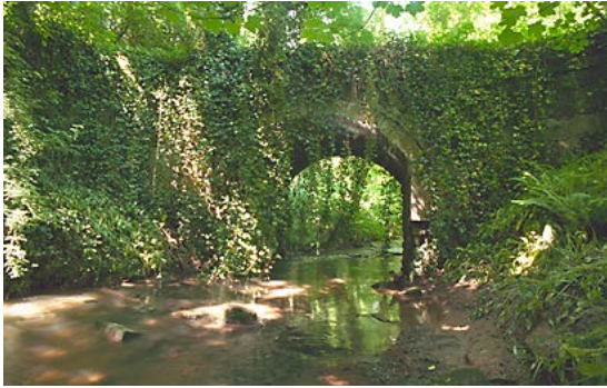
Dick Brook Bridge Astley (IoE 152272 Philip Williamson)
