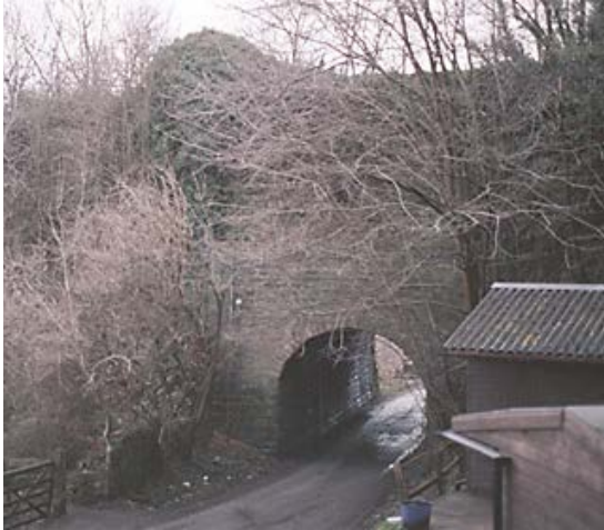
Ripley embankment, Cromford Canal (loE Steve Watson)
