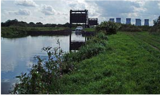
River Don Aqueduct (Wikipedia Bob1960evens)
