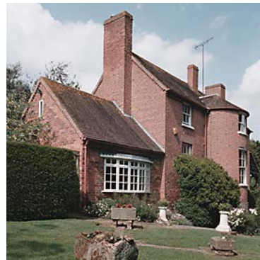
(Right) Wharf House Marlbrook, the headquarters of the Kington and Leominster Canal Company (IoE 484020 John Burrows)
