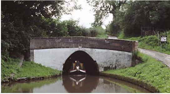
Trent & Mersey Barton Tunnel (IoE 435806 R G Noxon)
