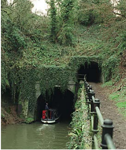
Shrewley Tunnel North Portal with horse tunnel alongside. ( IoE 436126 Helmut Schulenburg)
