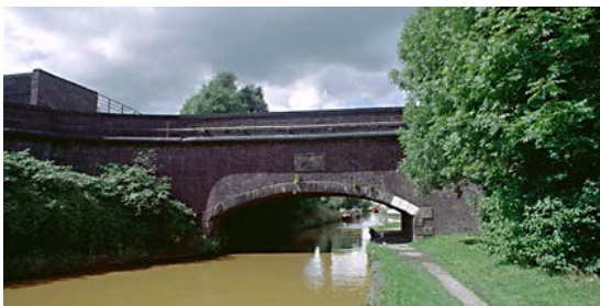
(Left) Pool Lock Aqueduct carrying the Macclesfield Canal over the Trent and Mersey Canal. Dated 1829. (IoE 56499 J M Pickering):
