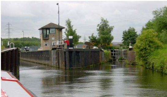
Kilnhurst Lock, with the older, disused lock to the right. ( www.penninewaterways.co.uk )
