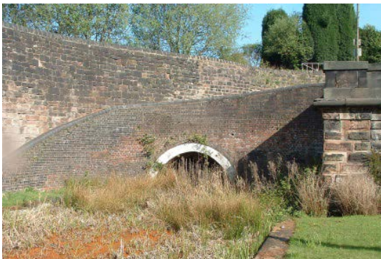
Brindley's south portal Harecastle Tunnel (Wikipedia Akke Monasso)
