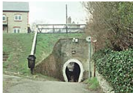
(Right) Grand Union Canal Horse tunnel below canal embankment, Cosgrove (IoE 235243 Alistair F Nisbet)
