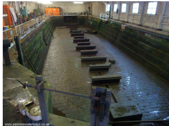
(Right) Aire & Calder Dry Dock Stanley Ferry workshops ( www.penninewaterways.co.uk )
