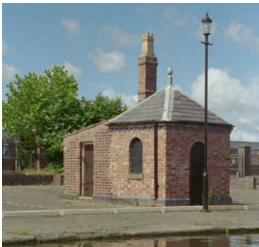
Two room hut, Tollhouse Ellesmere Port (IoE 56296 K Truman)
