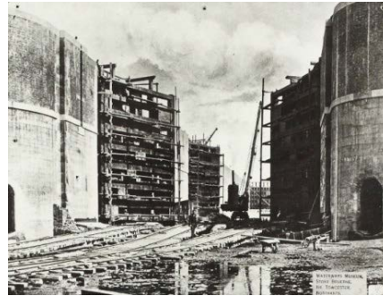
(Right) Manchester Ship Canal Eastham Locks under construction (Waterways Archive)
