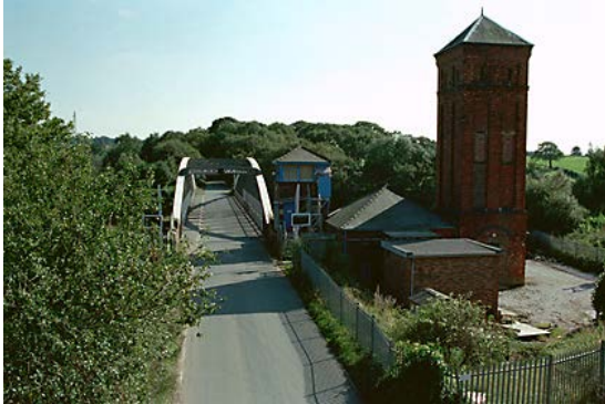
Moore Lane Bridge Manchester Ship Canal (IoE 58966 Keith Walker)
