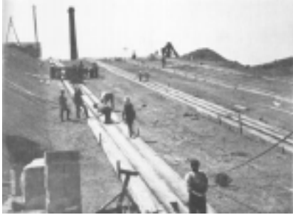
Leicester Line, Foxton Inclined Plane under construction 1900 and in use c.1905 (Wikipedia and Waterways Archive)
