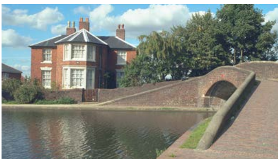
BCN Junction House at the junction of the Fradley to Fazeley and the Minworth to Fazeley branches (IoE 272795 David R. Grounds)
