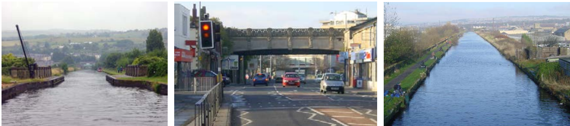
Leeds & Liverpool Canal Burnley Embankment (www.penninewaterways.co.uk)
