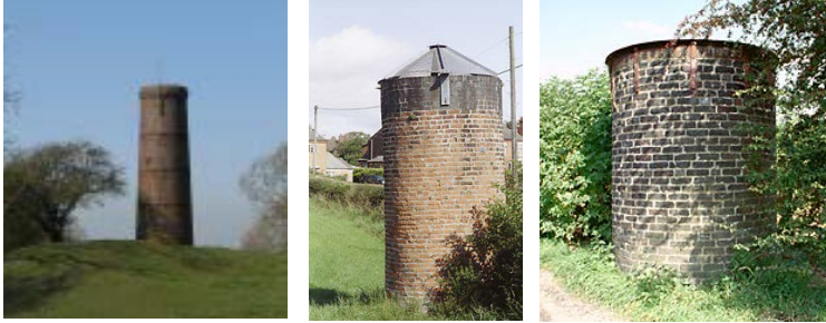
(Left) Blisworth Tunnel Ventilation Shaft, (Grand Union Canal) (Centre, Right) Trent & Mersey, Airshafts above Barnton Tunnel (IoE 449370 R.G. Noxon) and Preston Book Tunnel (IoE 429730 Keith Walker)
