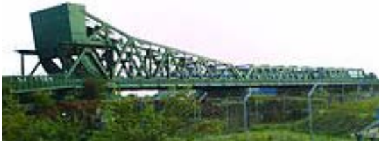
(Left) Keadby Bridge, River Trent (Wikipedia Asterion)
