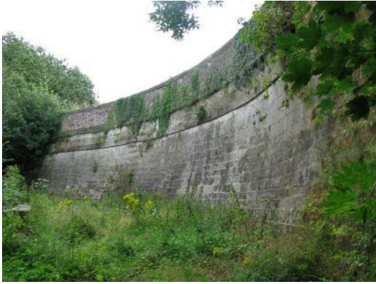
(Left) The north-western curved retaining wall for the Bollin aqueduct (copyright MRIAS)
