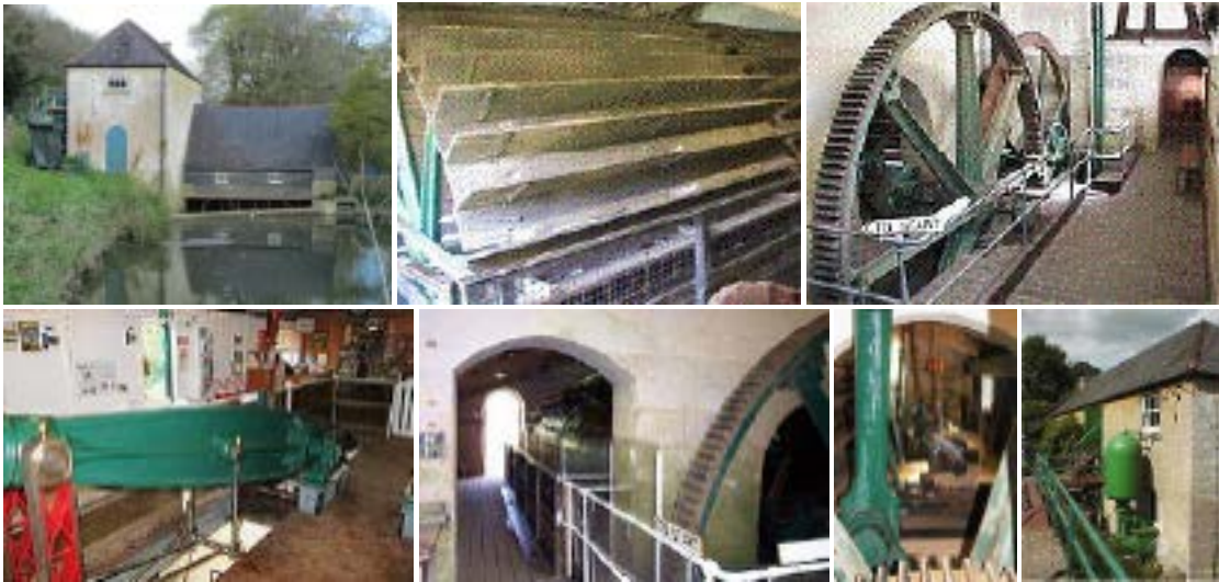
Claverton Pump House (Keith Falconer and Claverton Pumping Station Trust)
