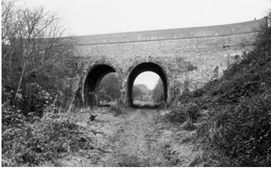
Grand Western Canal Halberton Aqueduct (Engineering Timelines)
