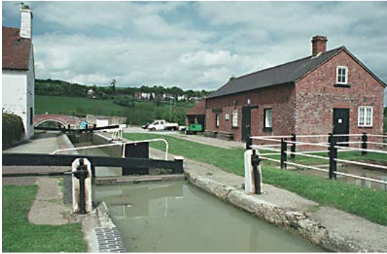
Oxford Canal Napton lock and workshops. (IoE 305642 Helmut Schulenburg)
