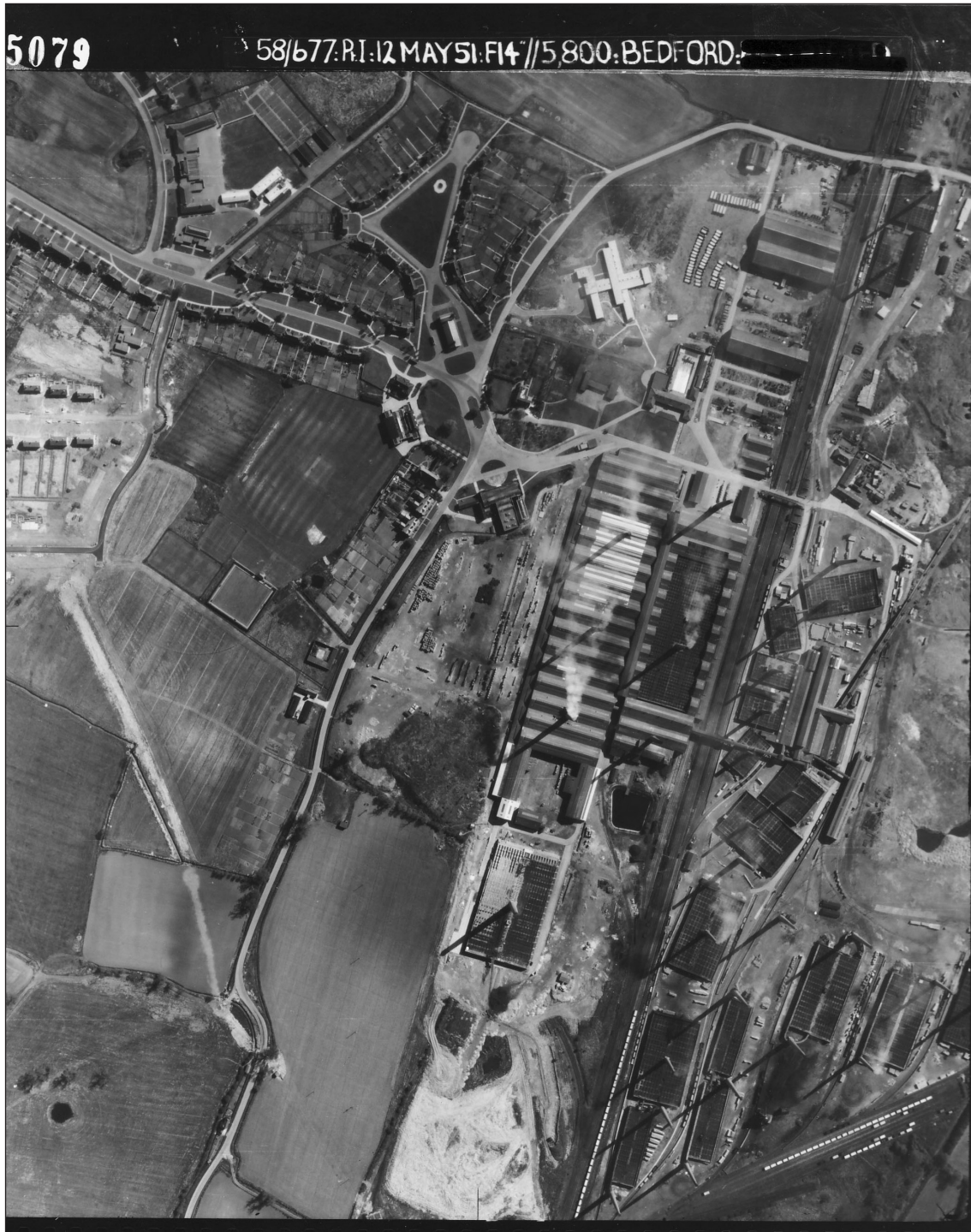
Figure 7 Aerial Photograph, 12 May 1951 Historic England Archive (RAF photography)
