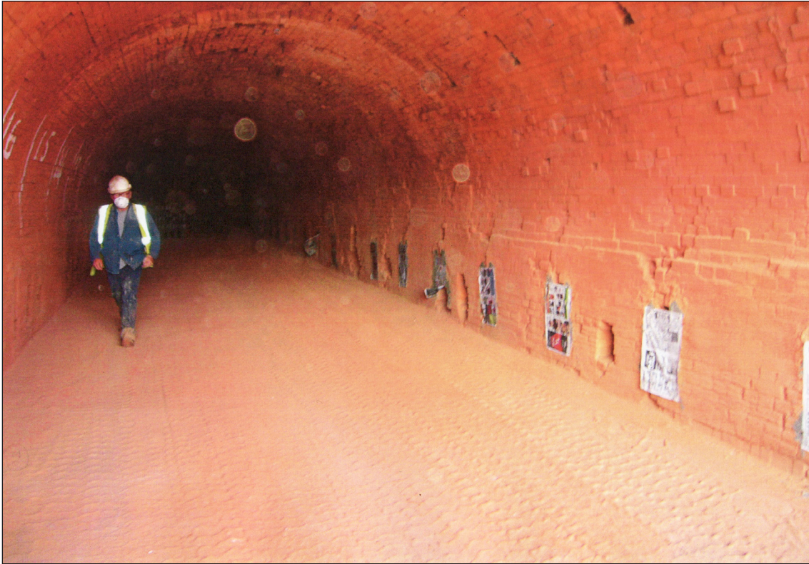
Figure 16 CK3, kiln chamber © Historic England
