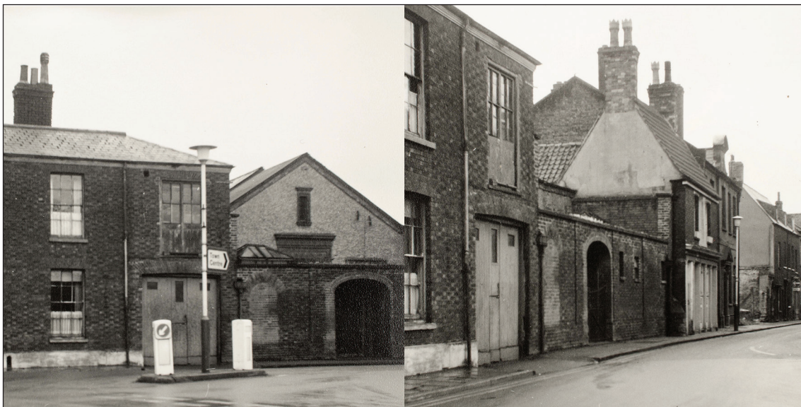
Figure 36: Details from two photographs showing the north elevation of the parish/drill hall on St Nicholas Street. Note: The Ordnance Survey map of 1976 (Fig 33) suggests the catalogued date of 1977 for the photograph on the right-hand side is incorrect. [Source: Norfolk Museums Service (Lynn Museum) KILLM 2007.64.1 nd, KILLM 2007.65.1 1977; Images: HEA DP219388, DP219389]
