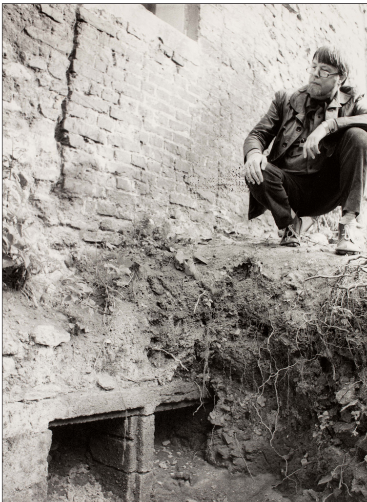
Figure 47: Colin Shewring, Borough Conservation Officer, pictured in 1977 during the excavation of a medieval stone wall with two rectangular openings, or cupboards, immediately beneath the south side of Fells Warehouse. [Source: King's Lynn Norfolk Studies Collection; Image: HEA DP219426].
