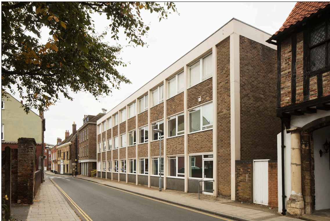
Figure 46: View north-east to Lovell House on the north side of St Nicholas Street. [HEA DP217377 Patricia Payne 20-SEP-2017 ©Historic England]
