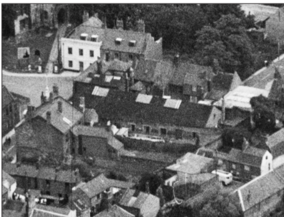
Figure 35: An aerial photograph looking north-east from July 1963 shows the western and southern elevations of the parish/drill hall on St Nicholas Street [Source: Historic England Archive (Aerofilms Collection) ALF62883/EAW116074 8-JUL-1963]
