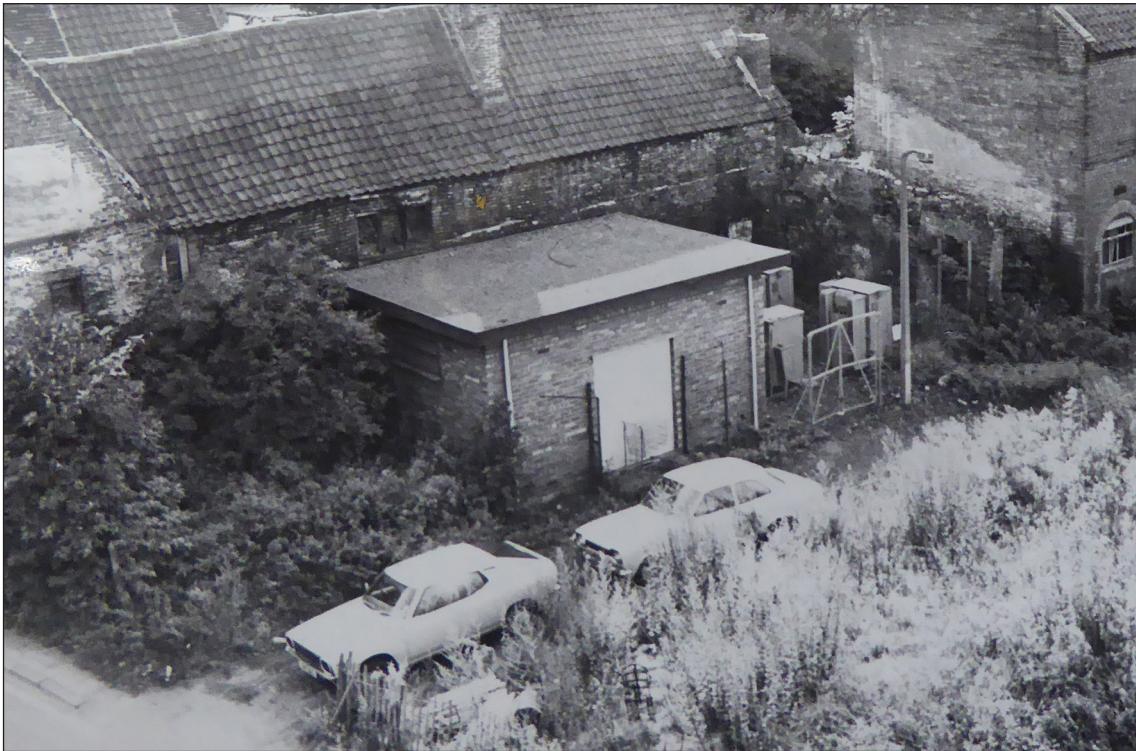
Figure 37: View, looking south-west, of the northern elevation of the electricity sub-station built on the site of the Chapel Buildings. [King's Lynn Norfolk Studies Collection (Chapel Street photograph file, nd)].
