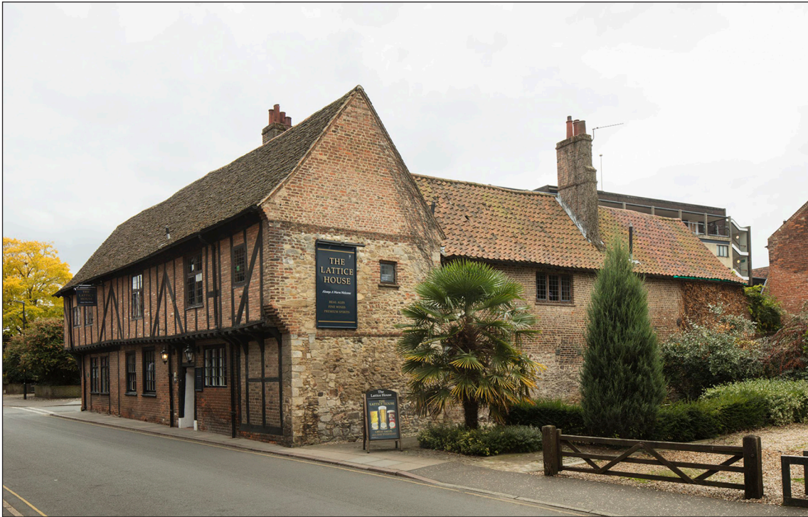
Figure 43: Lattice House, Chapel Street, looking south-west. [HEA DP217395 Patricia Payne 20-SEP-2017 ©Historic England]
