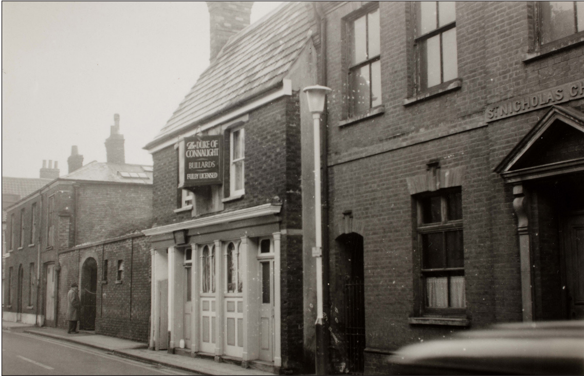
Figure 16: The Duke of Connaught public house, probably photographed in the 1960s. The building is potentially late 18th century in date, though a new ground-floor front was inserted around the early 20th century. [Source: King's Lynn Norfolk Studies Collection. Image: HEA DP219468]
