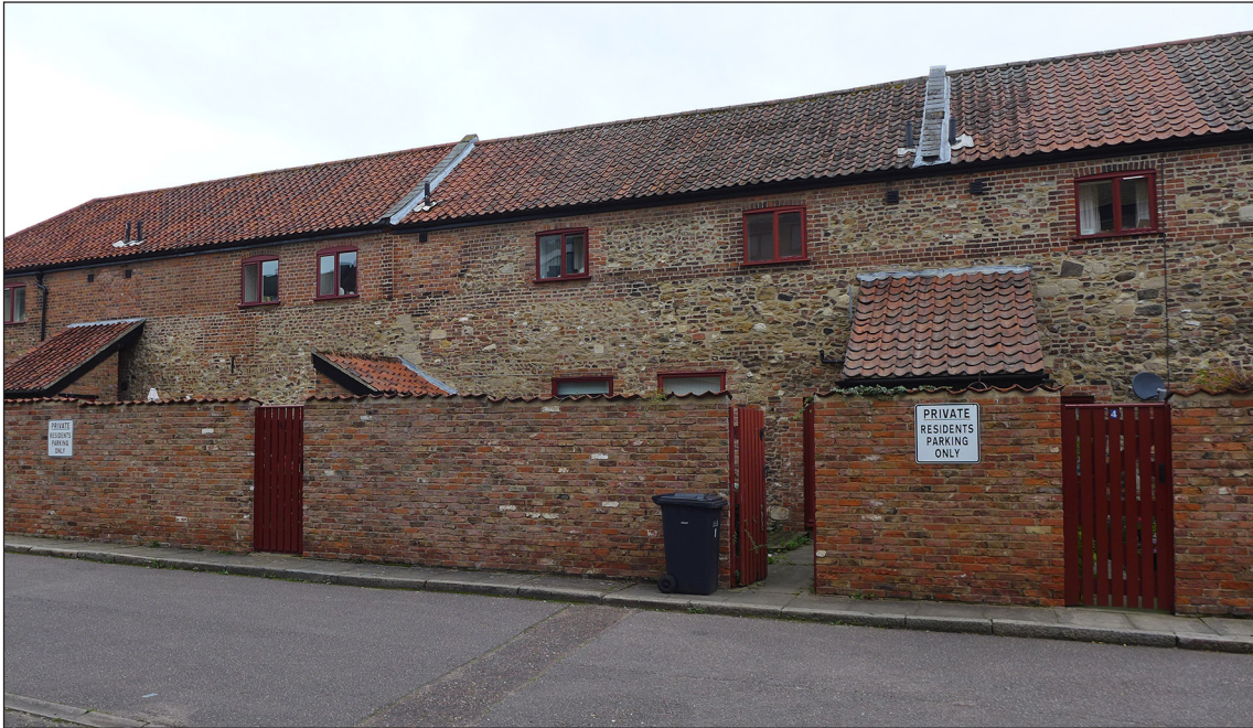
Figure 48: The south elevation of Fells Warehouse. A large quantity of stone rubble and some dressed stone blocks are visible in the rear elevation, which was clearly not intended to be seen. The variation in colour suggests that some stones were internal and some were external to their original building. (Photo: Wayne Cocroft 04-OCT-2017 Historic England)
