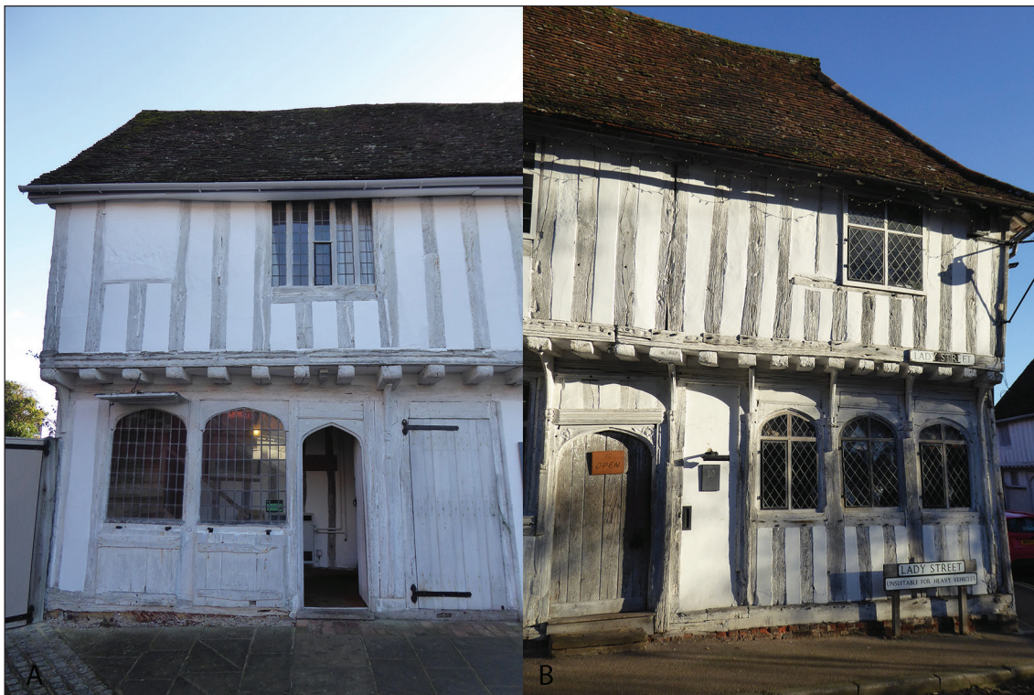
Figure 11: Two medieval shop fronts in Lavenham, Suffolk, both Grade I Listed: A) The 15th-century shop front at the eastern end of the Guildhall Range (NHLE 1181069) B) The 15/16th-century shop front on the building at the corner of Water Lane and Lady Street (NHLE 1351532). Images: Sarah Newsome 7-JAN-2018
