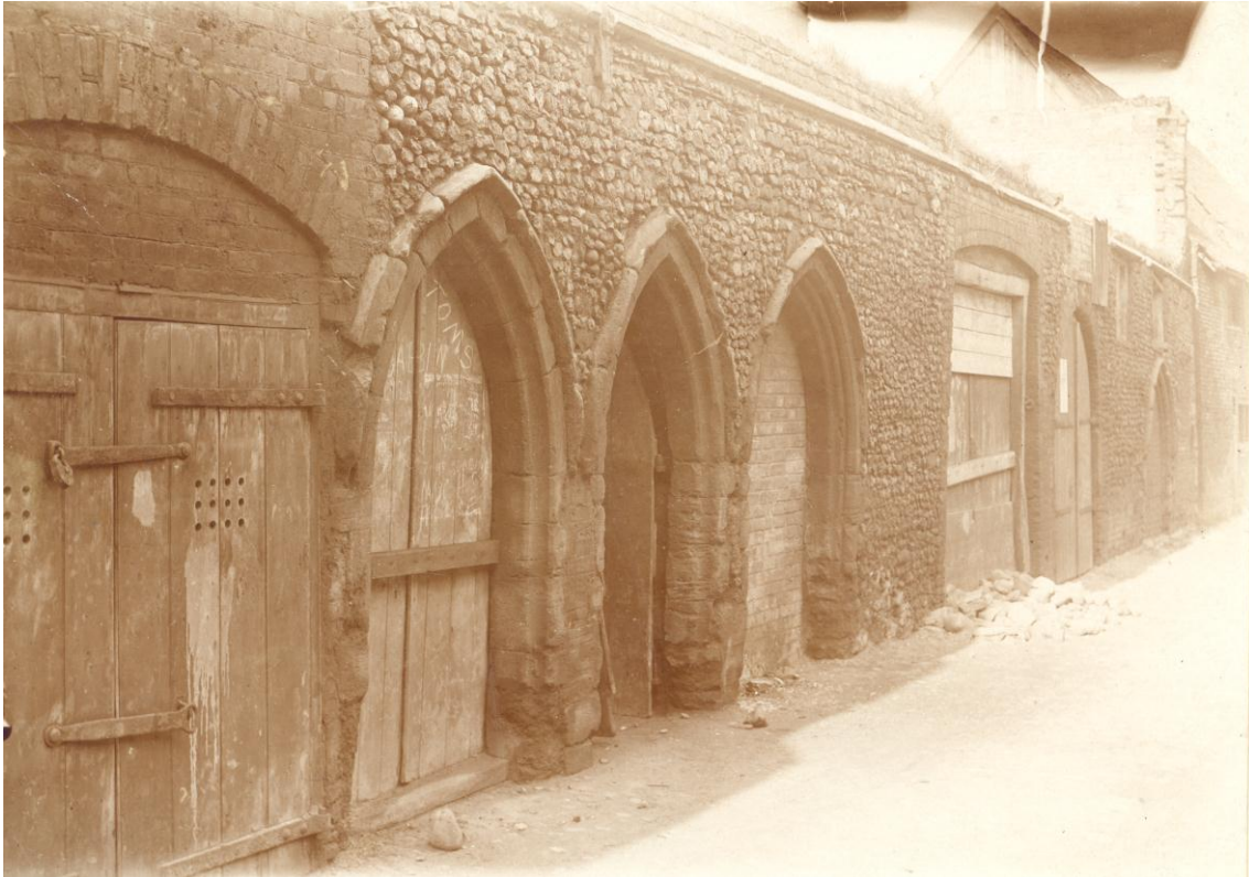
Fig. 39 The north side of the range shown on Fig. 38. Note the building on the very far right with a steep gable and mullioned windows with dripmoulds. True's Yard Fisherfolk Museum TY6136
