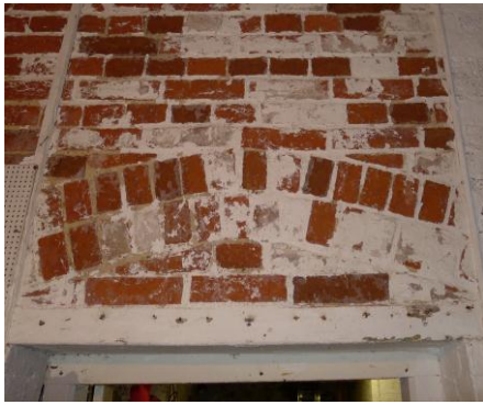
Fig. 68 ( above left ) Two relieving arches above the door from the Buoy Store into the Inner Store. Photograph: Jonathan Kewley 6-JUN-2017 ©Historic England
