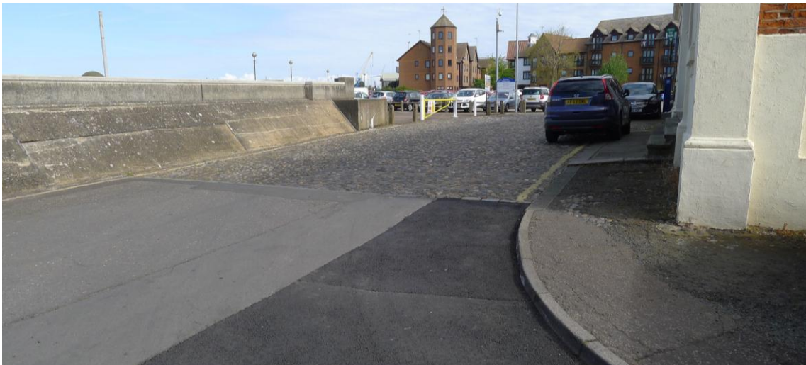
Fig. 128 The cobbled carriageway on the west side of the Public Baths. Note the cobbles visible under the tarmac on the pavement on the right. Photograph: Jonathan Kewley 2-MAY-2017 ©Historic England
