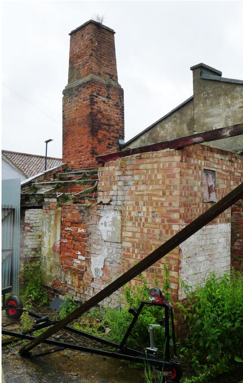
Fig. 101 The Chimney Store, looking south-west. Photograph: Jonathan Kewley 6-JUN-2017 ©Historic England
