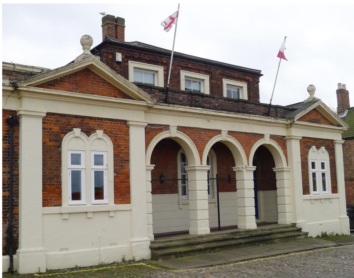
Fig. 43 The principal (west) front of King's Lynn Public Baths. Photograph: Jonathan Kewley 27-FEB-2017 ©Historic England
