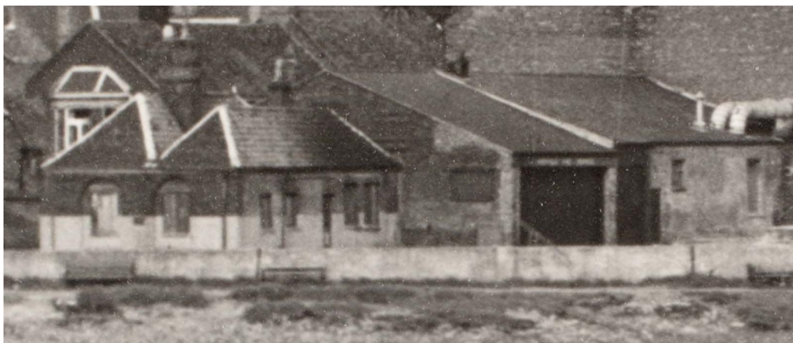
Fig. 34 The Fish Cross, later the Meter's Office, the one part of the old north range of the Common Staithe which survived the demolitions of the late 1820s, finally pulled down in 1967; it is the pantiled building behind the firemen in Fig. 32. Photograph by George King, 1963. Norfolk Library and Information Service (King's Lynn Library Archives)
