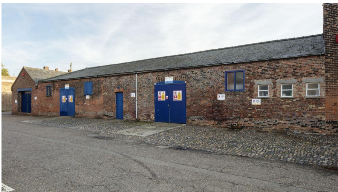
Fig. 35 The warehouses on the Common Staithe, built in 1829 (the right-hand section, up to just left of the foot door) and 1834 (the rest of the range under the same roof; the gabled building beyond is 20 th century). Detail of DP 219084 28-SEP-2017 Patricia Payne ©Historic England
