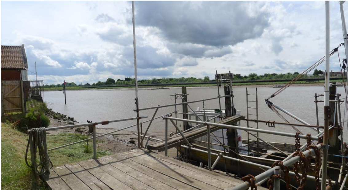
Fig. 126 The scaffolding jetty by the Crown and Mitre. Photograph: Jonathan Kewley 3-JUL-2017 ©Historic England
