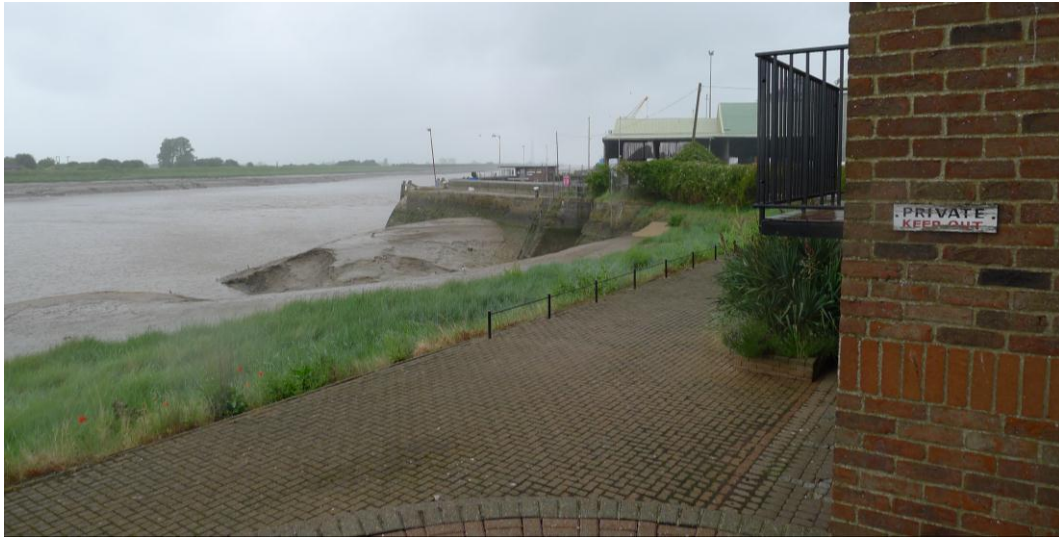
Fig. 122 The river frontage at Trinity Quay, looking north towards the Wash. Photograph: Jonathan Kewley 6-JUN-2017 ©Historic England
