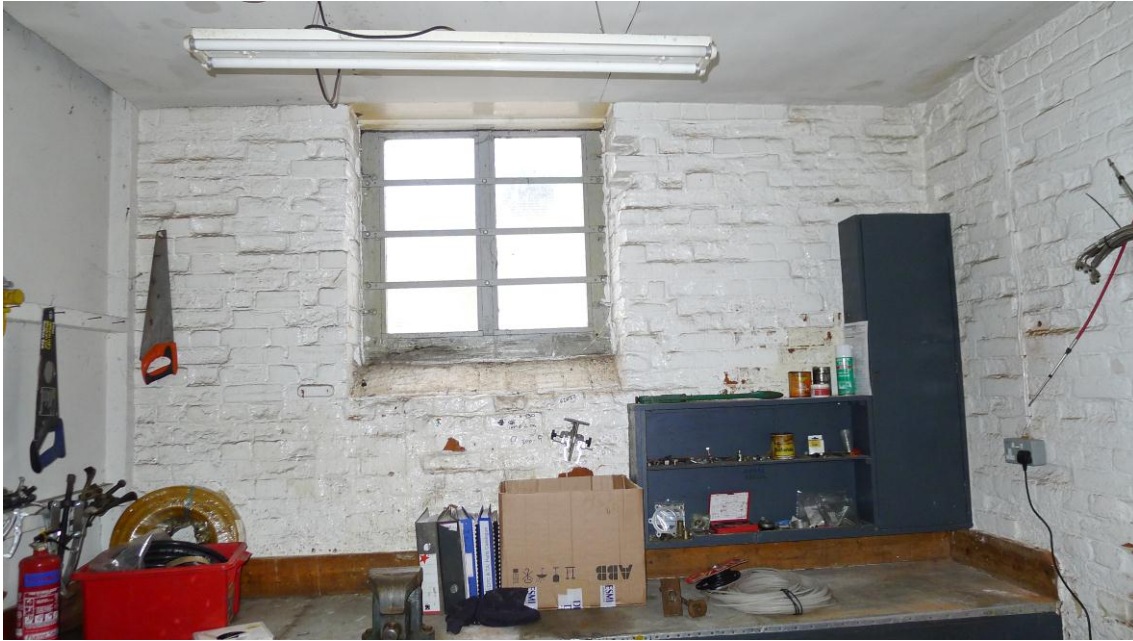
Fig. 71 The eastern section of the Engineers' Store, looking north. Photograph: Jonathan Kewley 6-JUN-2017 ©Historic England
