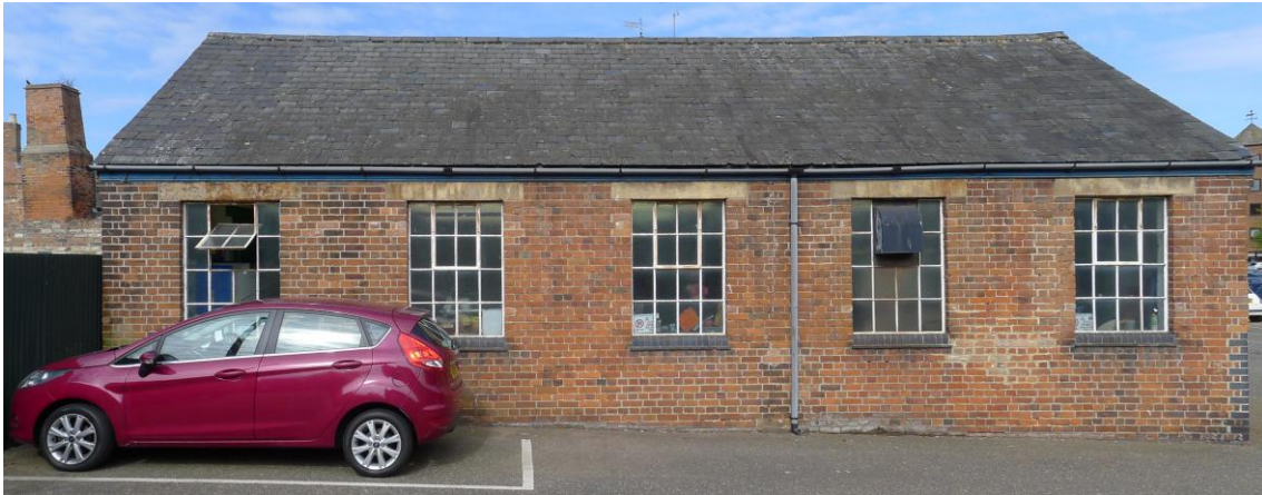
Fig. 47 The Carpenters' Workshop from the east. Photograph: Jonathan Kewley 2-MAY-2017 ©Historic England.
