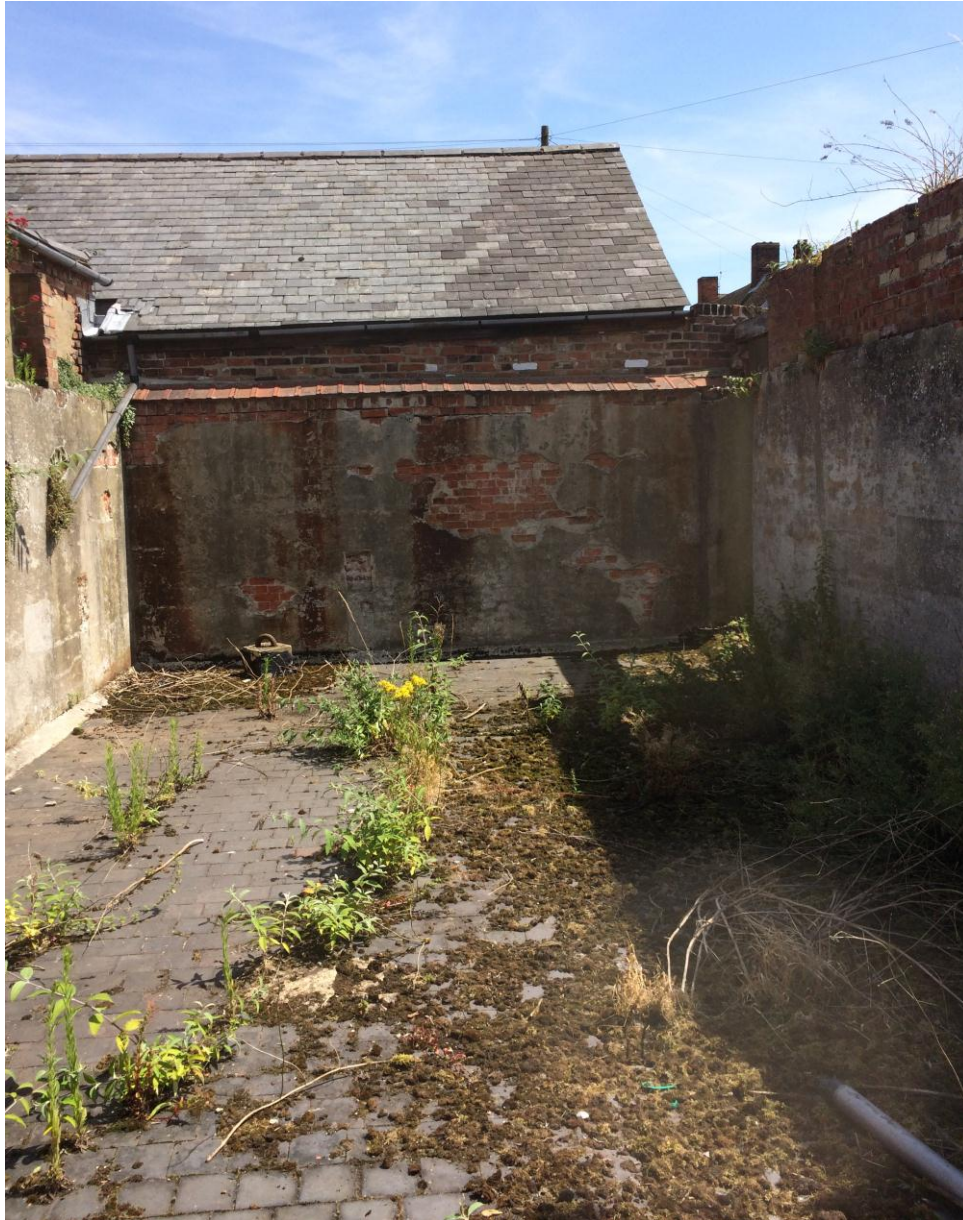
Fig. 98 The Settling Tank looking east. Photograph: Jonathan Kewley 17-JUL-2017 ©Historic England
