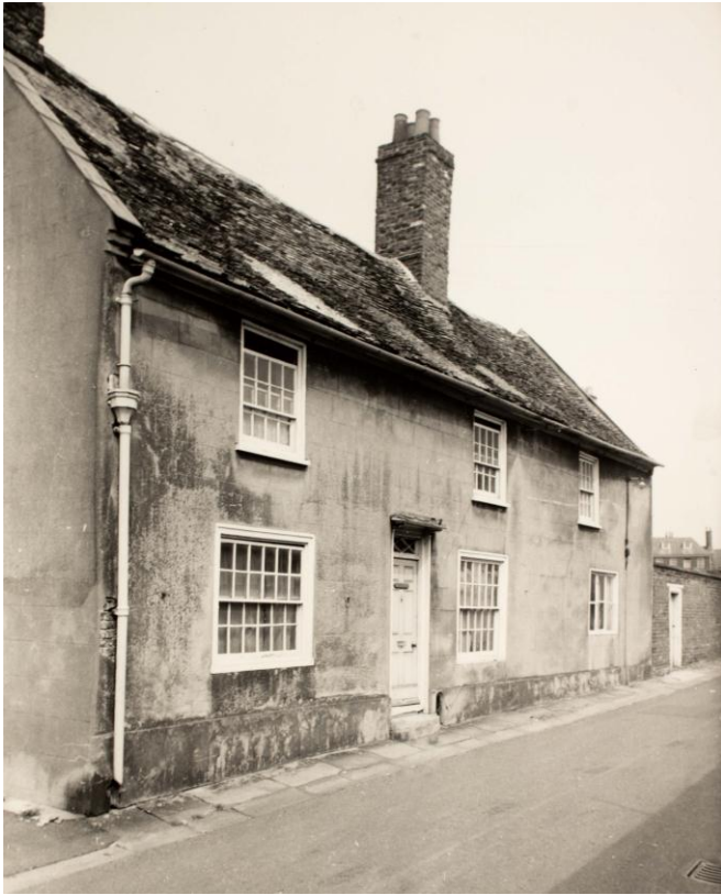
Fig. 41 The last surviving building from the south range of the Common Staithe, prior to its demolition: Birtledene, Ferry Street, from the south-west, early 1960s. Norfolk Museums Service (Lynn Museum)
