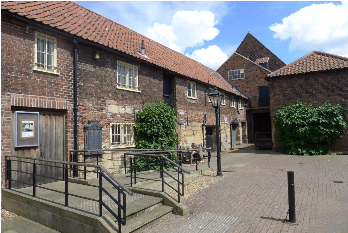
Fig. 16 St George's Guildhall, between King Street and the river; note the use of stone at lower level in the buildings. Photograph: Jonathan Kewley 5-JUL-2017 ©Historic England
