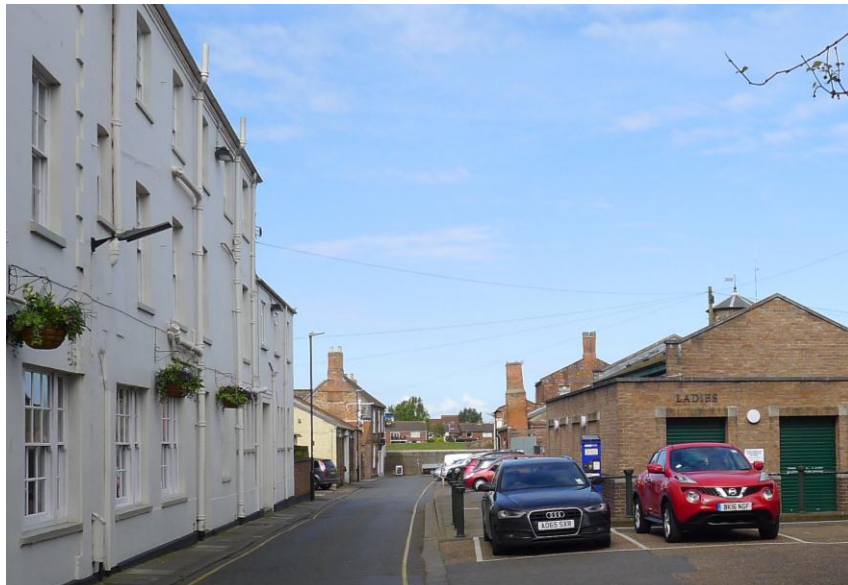
Fig. 59 Looking west along Ferry Street, the southern boundary of the site. On the left is the Globe Hotel. Photograph: Jonathan Kewley 2-MAY-2017 ©Historic England
