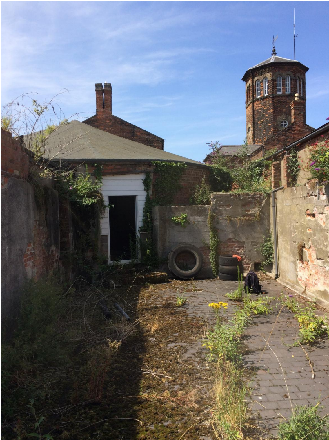
Fig. 99 The Settling Tank looking west. Photograph: Jonathan Kewley 17-JUL-2017 ©Historic England
