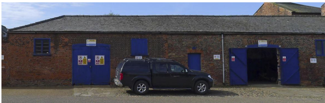
Fig. 62 The warehouses from the north. Photograph: Jonathan Kewley 2-MAY-2017 ©Historic England
