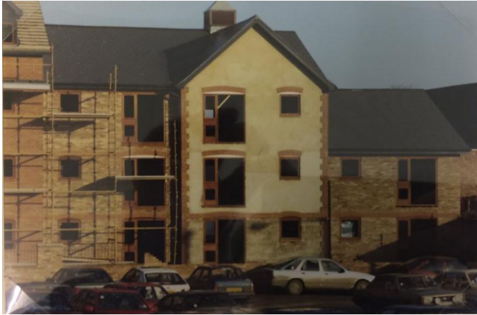
Fig. 57 Trinity Quay under construction in 1990. Norfolk Museums Service (Lynn Museum)
