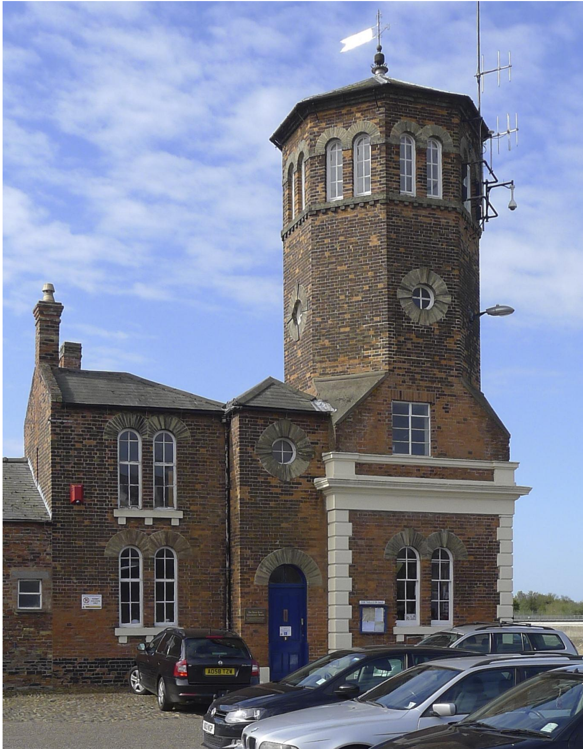
Fig. 102 The north front of the Pilot Office. Photograph Jonathan Kewley 2-MAY-2017 ©Historic England
