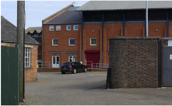
Fig. 26 Looking north from Ferry Street, showing the rounded corner of the wall enclosing the former Gurney's premises, later Barclays Bank; note the cannon, which is on the NHLE Photograph: Jonathan Kewley 2-MAY-2017 ©Historic England
