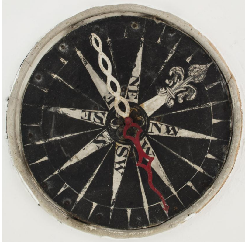
Fig. 109 The dial of the wind-gauge on the ceiling of the Tower Room. Detail of DP217318 20-SEP-2017 Patricia Payne ©Historic England
