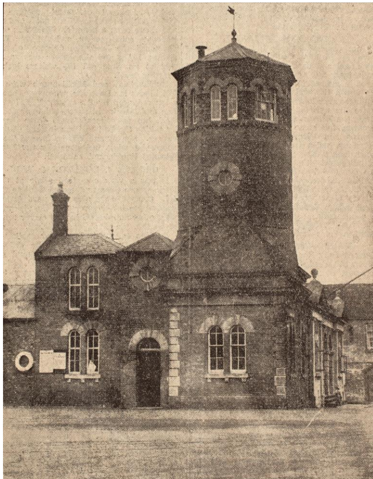
Fig. 104 The Pilot Office from the north-west in 1937. Norfolk Library and Information Service (King's Lynn Library Archives)
