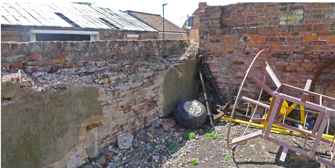
Fig. 115 The double-skinned wall running east-west parallel with Ferry Street, and seen here from the north. The further skin was the back wall of Birtledene and the nearer seems to have been the back wall of one of the warehouses on the Common Staithe.
