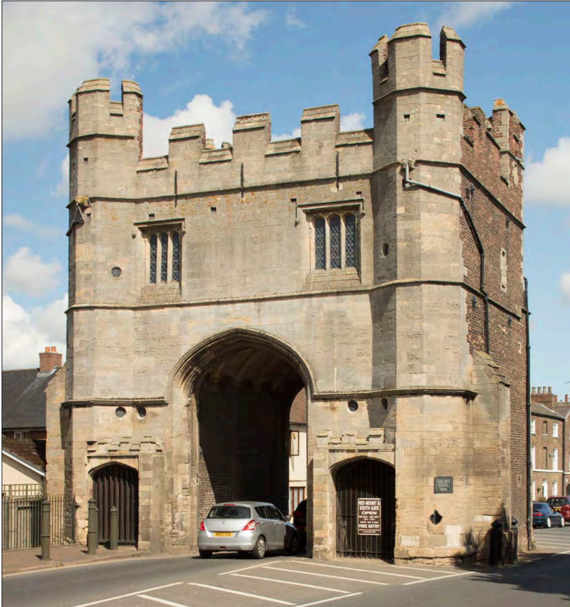
The South Gate from the south-east, showing the stone south and brick east elevations. HEA DP219059 Patricia Payne 15-AUG-2017 © Historic England
