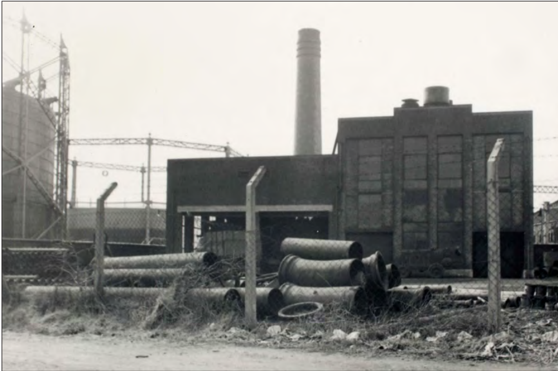
Fig 191. The Gas Works in 1964 showing on the right the carburetted water gas plant. Norfolk Museums Service (Lynn Museum) 1992.217.49; image HEA DP219380
