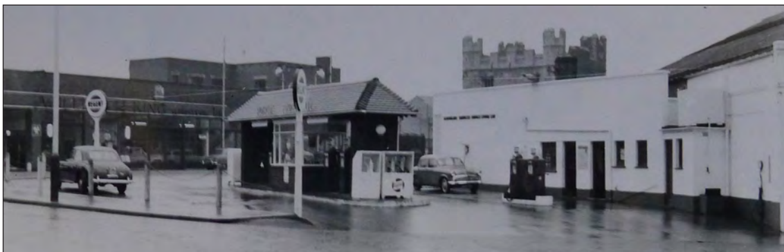
Fig 234 The filling station from the south-east in 1960. In the background are the Ford Garage and the South Gate. Norfolk Library and Information Service (King's Lynn Library)
