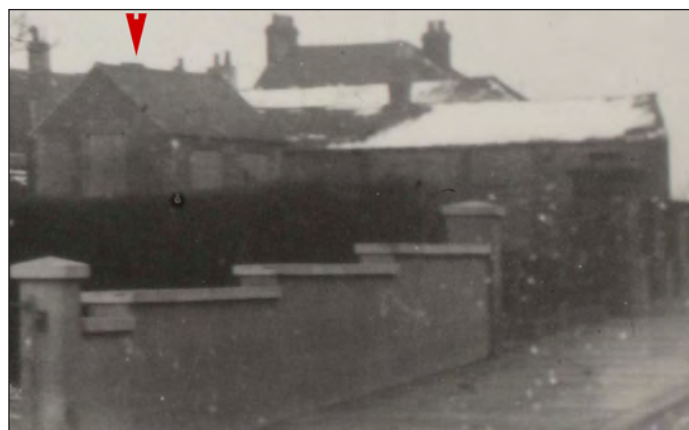
Fig 171 (below) Building L (marked) from the south-west in c 1960. Norfolk Library and Information Service (King's Lynn Library). Image: detail of HEA DP219465
