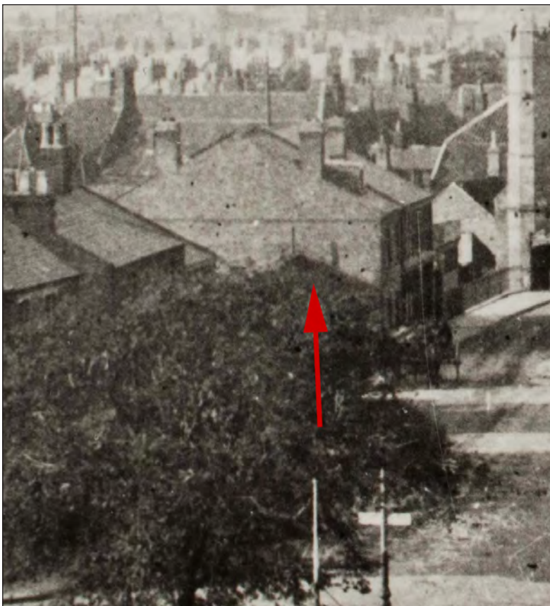
Fig 141 The buildings at the top of Out South Gates on the west, in a detail from a late 19 th or early 20 th century photograph. Norfolk Library and Information Service (King's Lynn Library Archives)
