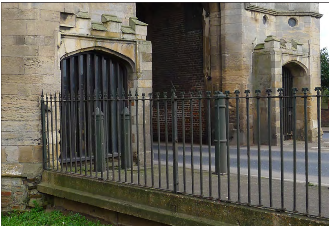
Fig 62 The southern entrances to the former pedestrian passages through the South Gate inserted to the east (right) in 1817 and the west (left) in 1841. The iron railings in the foreground probably date from 1841. Photograph Jonathan Kewley 27-FEB-2017 © Historic England
