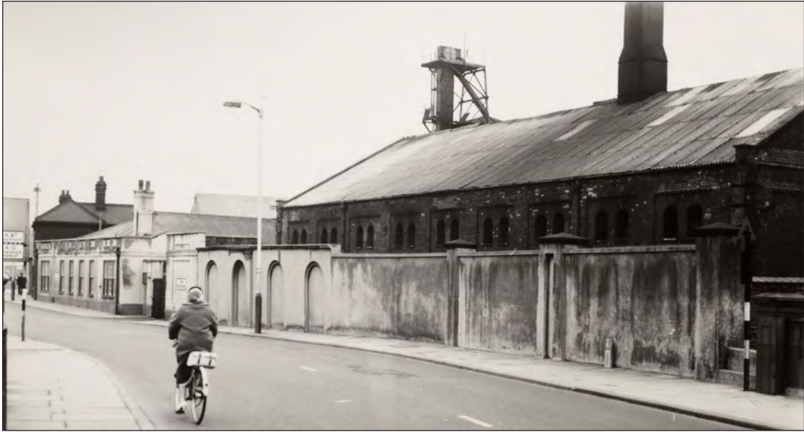
Fig 187 The Gas Works looking west along the Wisbech Road c 1960, showing the retort house on the right. Note that the domed entrance has been demolished. Norfolk Library and Information Service (King's Lynn Library); image detail of HEA DP219462
