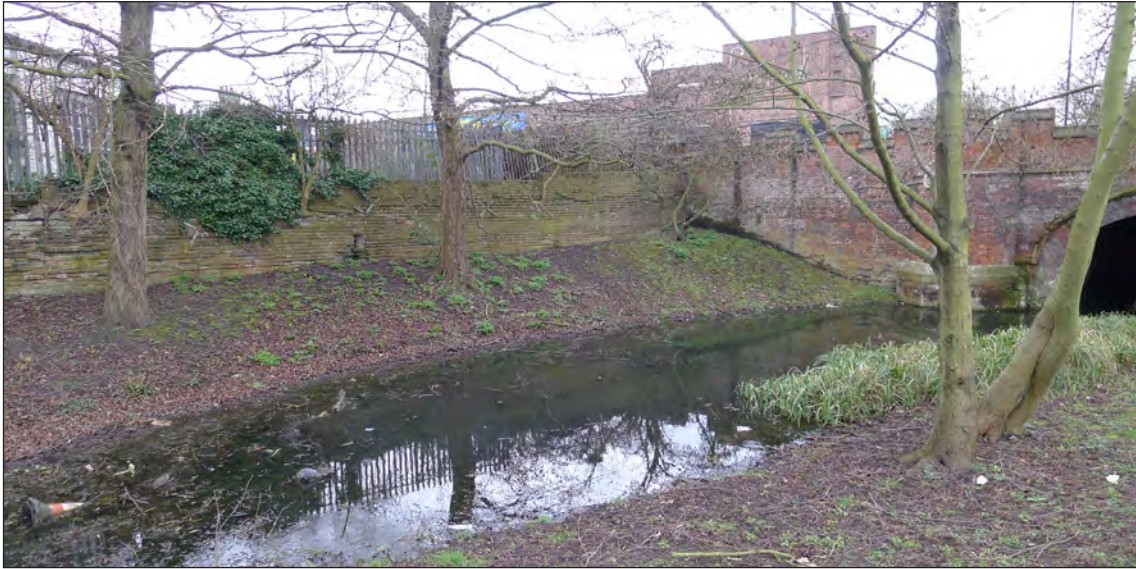
Fig 25 The short section of the Middleton Stop Drain immediately east of Southgates Bridge which still contains water, looking west. Photograph Jonathan Kewley 27-FEB-2017 © Historic England
