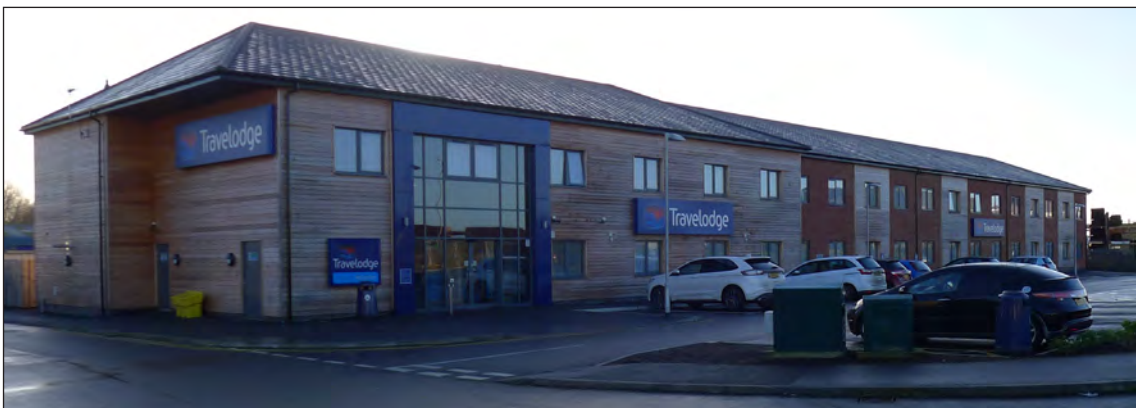
Fig 218 The King's Lynn Travelodge on Kellard Place from the north-west. Photograph Jonathan Kewley 16-JAN-2018 © Historic England
