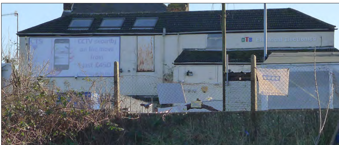
Fig 160 The former Highland Laddie from the west. Photograph Jonathan Kewley 16-JAN-2018 © Historic England
