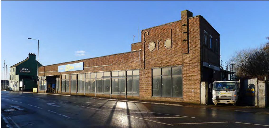
The former Ford garage on Out South Gates from the north-east. Photograph Jonathan Kewley 16-JAN-2018 © Historic England
