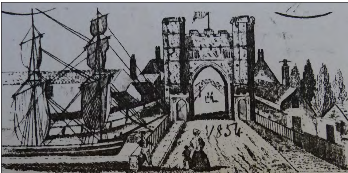
Fig 63 An anonymous drawing of the South Gate from the south, dated 1854, showing its appearance in the period between the insertion of the pedestrian passages and the cutting-through of the new carriageway. Norfolk Library and Information Service (King's Lynn Library Archives)
