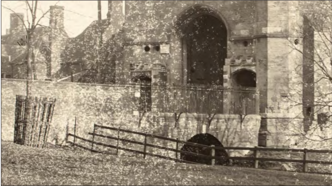
Fig 69 A pre-1899 photograph of the South Gate from the south-east, showing the eastward extension of the bridge constructed in 1817 to carry the new pedestrian footway. Norfolk Museums Service (Lynn Museum) MB05451. Image: HEA DP219374
