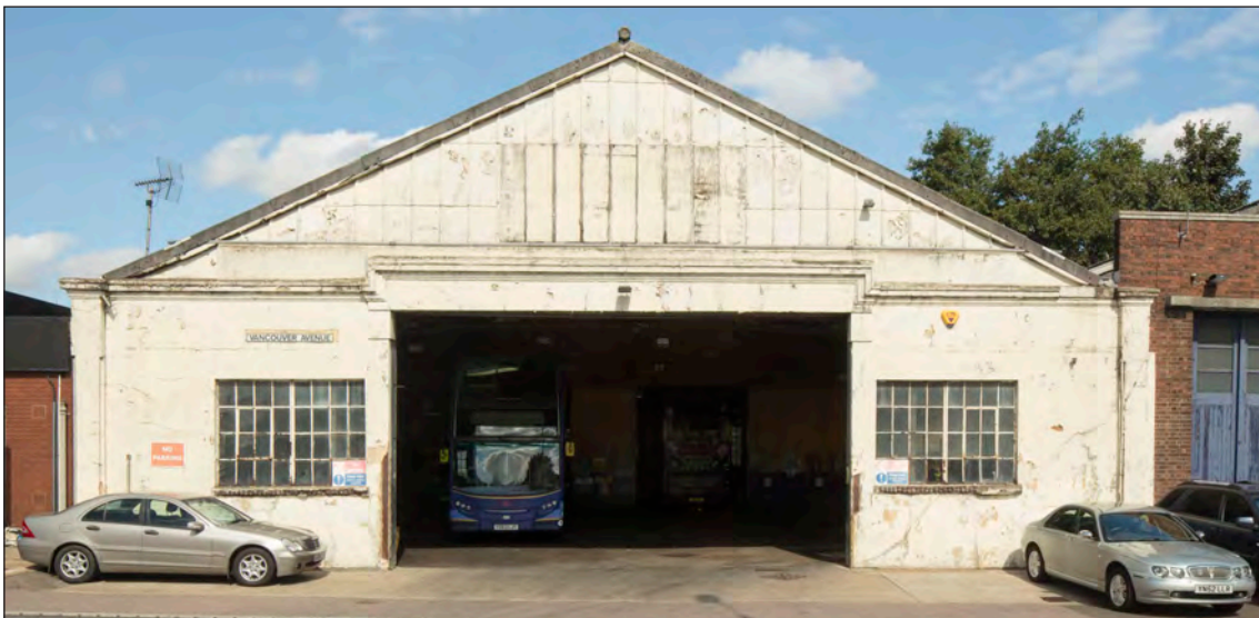
Fig 226 The principal, south front of the earlier half of the Bus Garage. Detail of HEA DP219056 15-AUG-2017 Patricia Payne © Historic England
