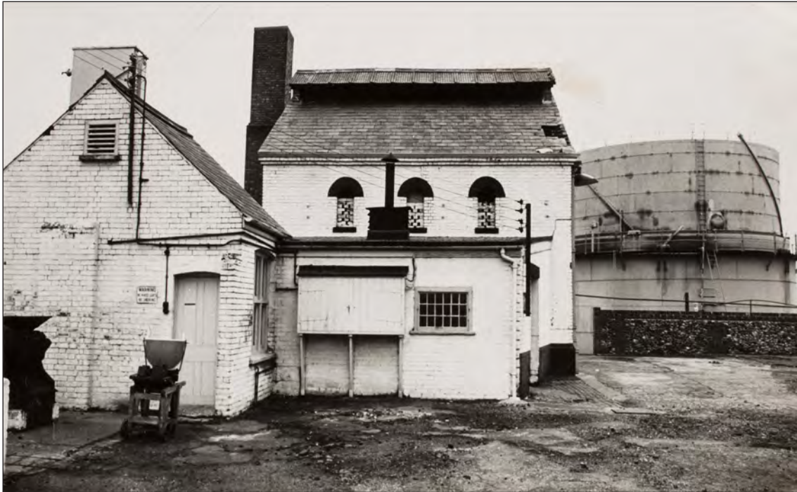
Fig 189 The new purifying house near the riverbank, and gasometer behind, both built in or shortly after 1897. Norfolk Library and Information Service (King's Lynn Library); image: HEA DP219439
