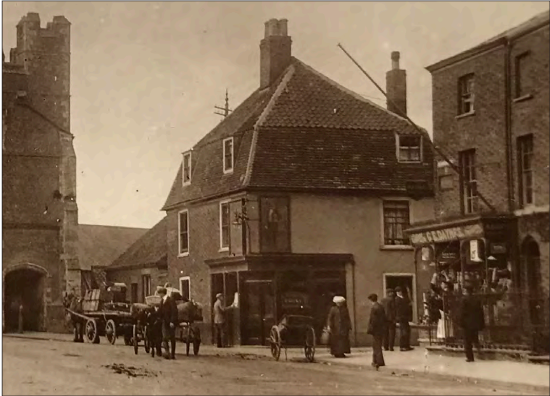
Fig 109 Detail of a photograph probably from the decade before the Great War showing the Honest Lawyer from the north-east. HEA © Historic England
