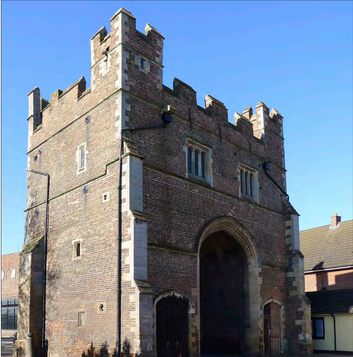
Fig 56 The east elevation of the South Gate. Photograph Jonathan Kewley 5-APR-2018 © Historic England
