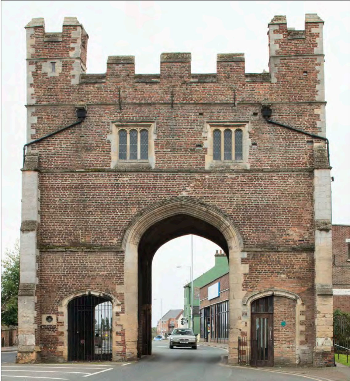
Fig 54 The north front of the South Gate. HEA DP219073 Patricia Payne 20-SEPT-2017 © Historic England
