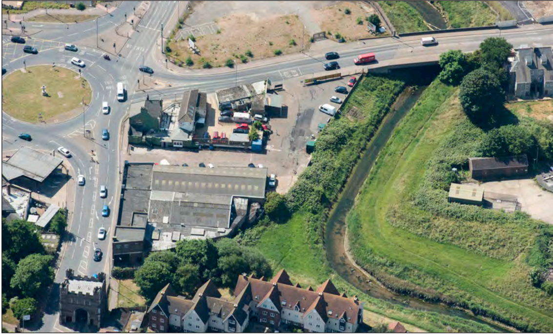
Fig127 An aerial view of area 4 from the north. Detail of HEA 33197/021 Damian Grady 19-JUN-2017 © Historic England
