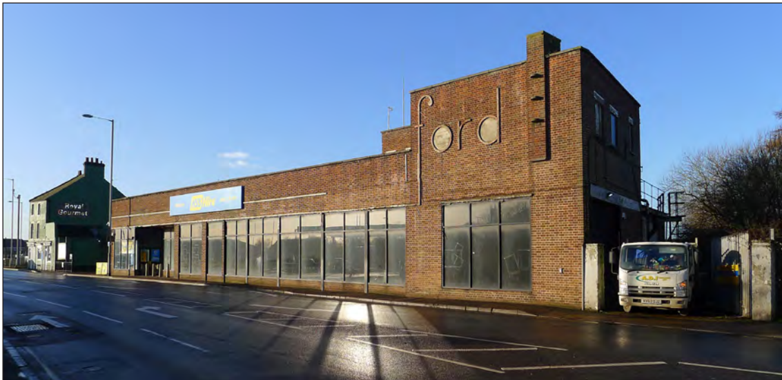
Fig 147 The former Ford garage on Out South Gates from the north-east. Photograph Jonathan Kewley 16-JAN-2018 © Historic England
