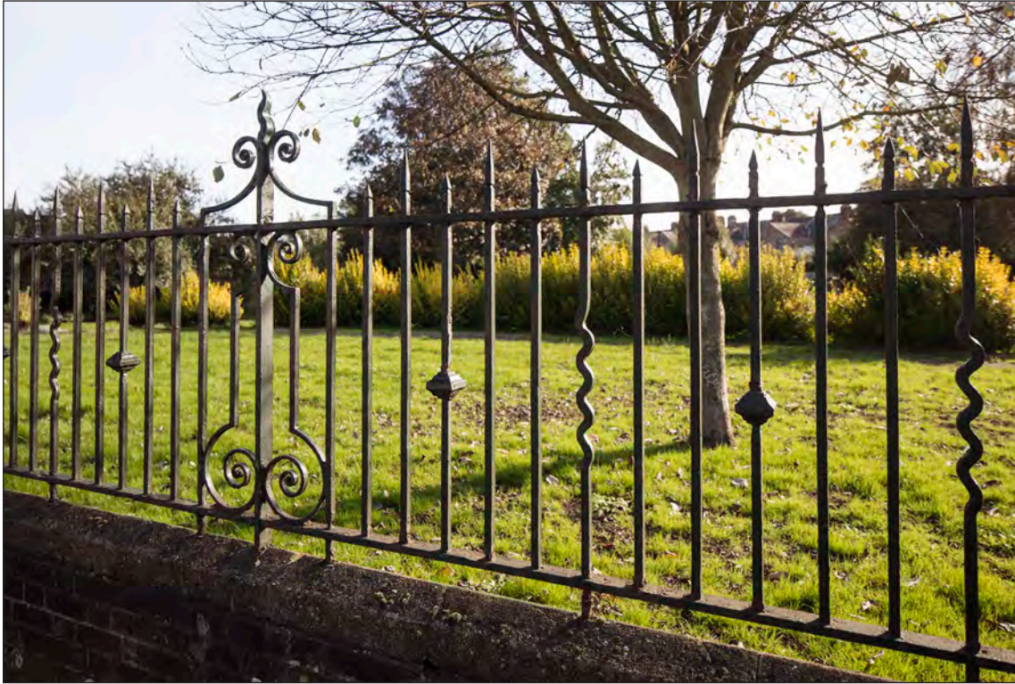
Fig 93: The railings on the park's western boundary wall, looking north-east. (HEA DP219103 Patricia Payne 17-OCT-2017 © Historic England)
