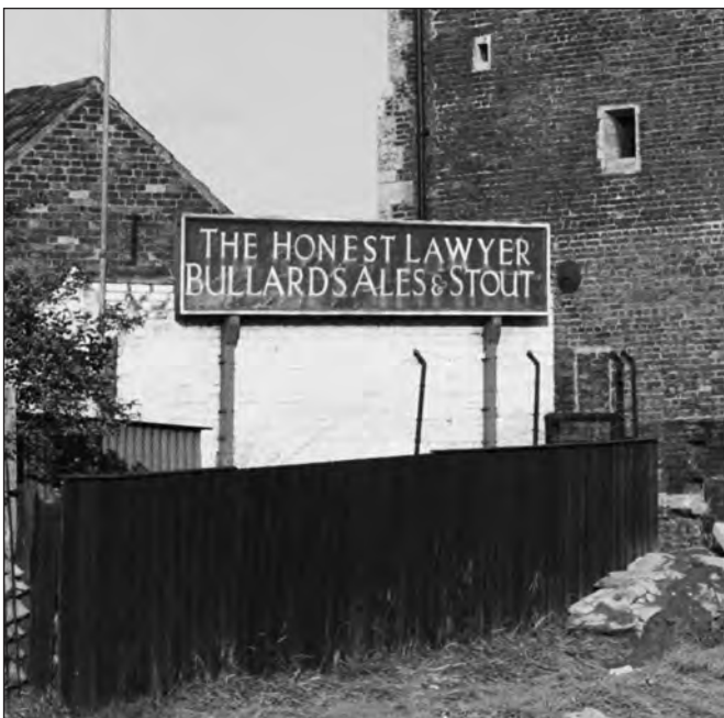
Fig 114 The south end of the Honest Lawyer in 1957 showing the brick gable behind and, in front, an outbuilding with a monopitch roof and a sign advertising the hostelry.
