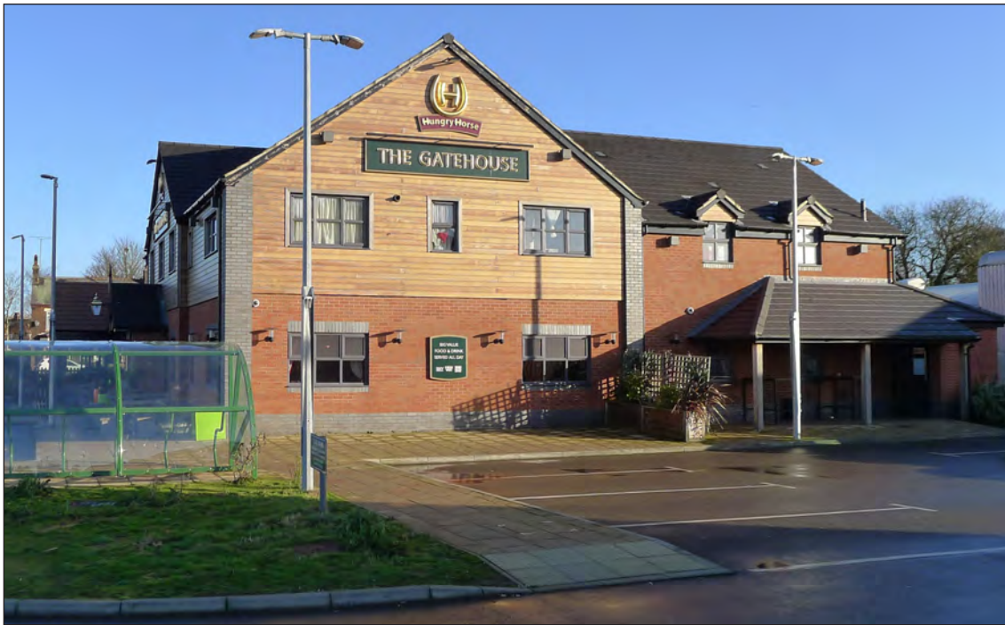
Fig 215 The south elevation of the Gatehouse ‘pub restaurant’ on Kellard Place. Photograph Jonathan Kewley 16-JAN-2018 © Historic England
