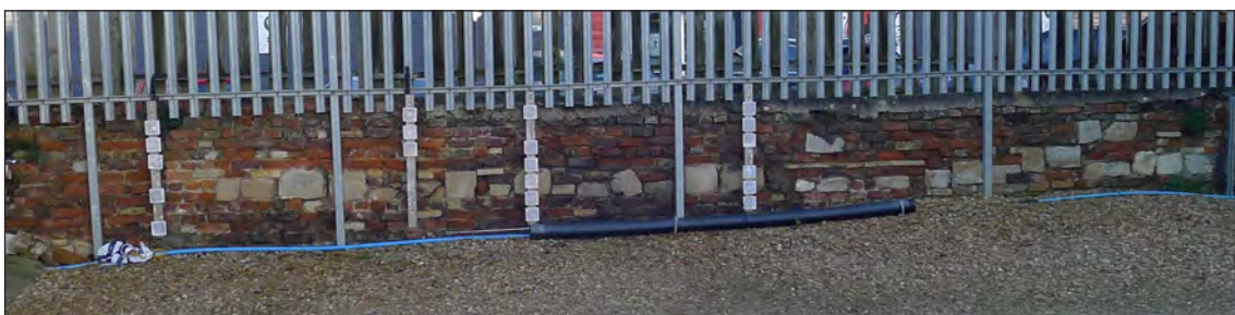
Fig 164 The wall at the back (north) of what is now the yard or car park for the former Highland Laddie, looking from the south. It appears to be the remains of an otherwise-demolished building (see Fig 163). Note the stone amongst the brickwork. Photograph Jonathan Kewley 16-JAN-2016 © Historic England
