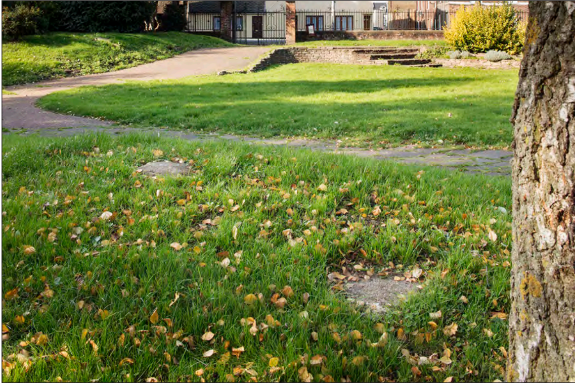
Fig 99: Exposed concrete on top of the northern end of the air raid shelter mound, looking south-west (HEA DP219125 Patricia Payne 17-OCT-2017 © Historic England)
