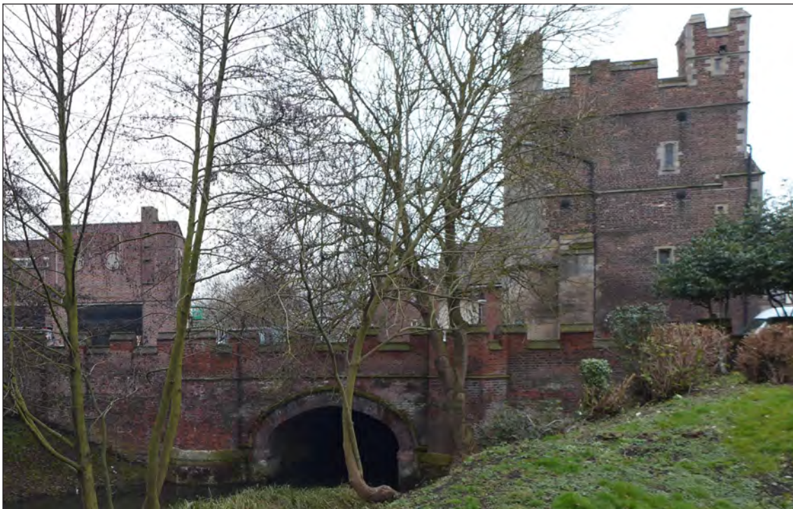
Fig 73 The view west from Southgate Park showing the battlemented wall created in 1899-1900 and combining an eastward extension of Southgate Bridge with a retaining wall to support the road running over it. Photograph Wayne Cocroft 8-FEB-2017 © Historic England
