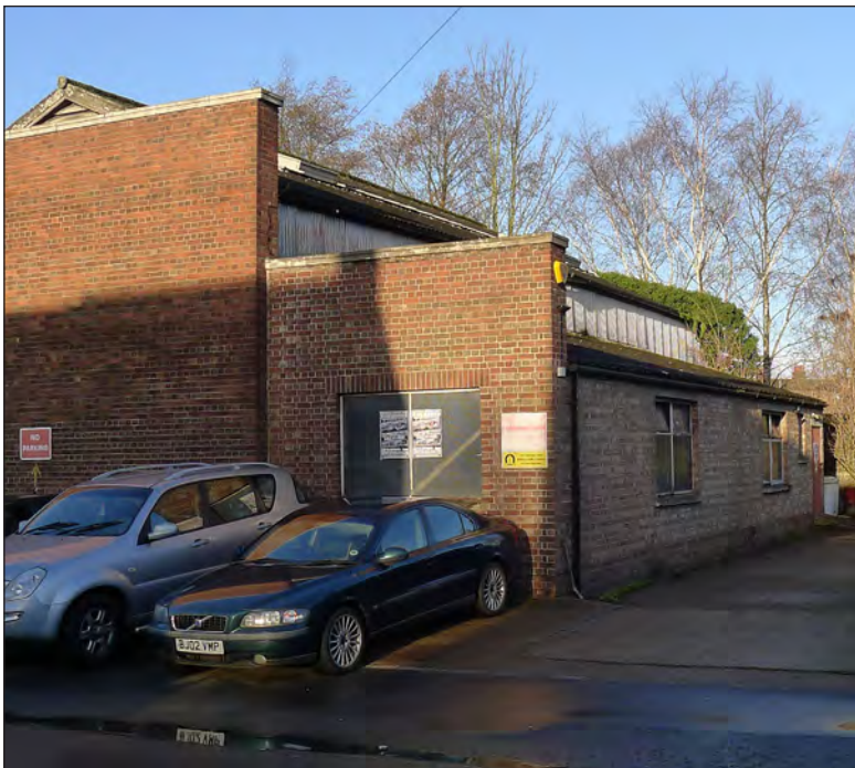
Fig 230 The small lean-to extension on the east of the Bus Garage, probably from 1950. Photograph Jonathan Kewley 16-JAN-2018 © Historic England
