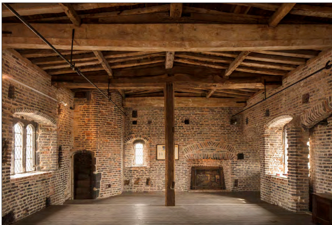
Fig 60 The interior of the second floor of the South Gate, now one room. HEA DP217365 Patricia Payne 13-JUL-2017 © Historic England
