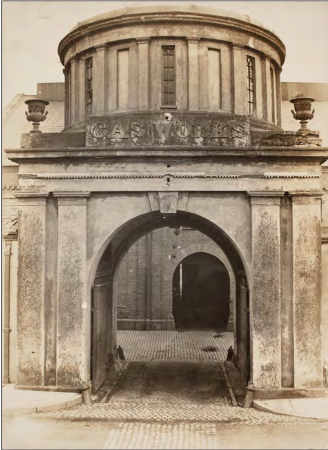
Fig 182 (left) The entrance to the Gas Works, probably in the second half of the 19 th century. Norfolk Library and Information Service (King's Lynn Library); image: detail of HEA DP219417
