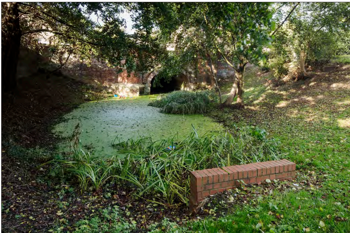
Fig 89 The water-filled western end of the Middleton Stop Drain as it disappears under the bridge. The brick wall in the foreground probably marks some form of sluice at the end of a storm drain (HEA DP219116 Patricia Payne 17-OCT-2017 © Historic England)
