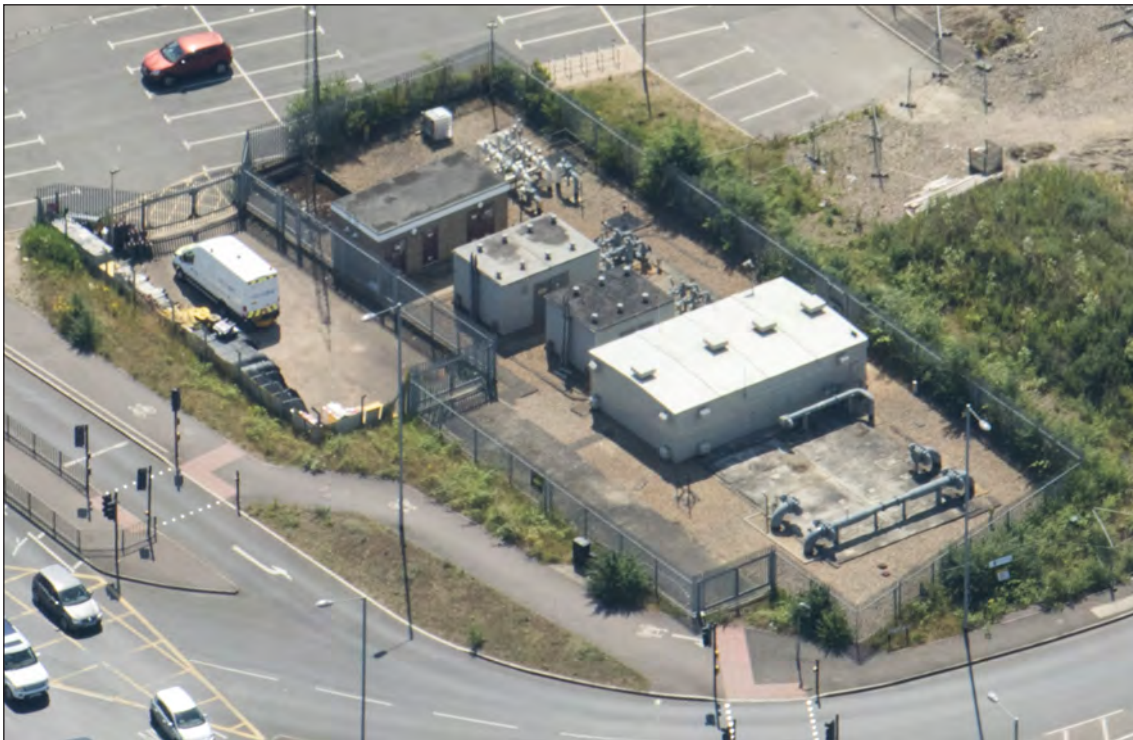
The National Grid Gas Pressure Reduction Station and Depot from the air. Detail of HEA 33197/025 Damian Grady 19-JUN-2017 © Historic England
