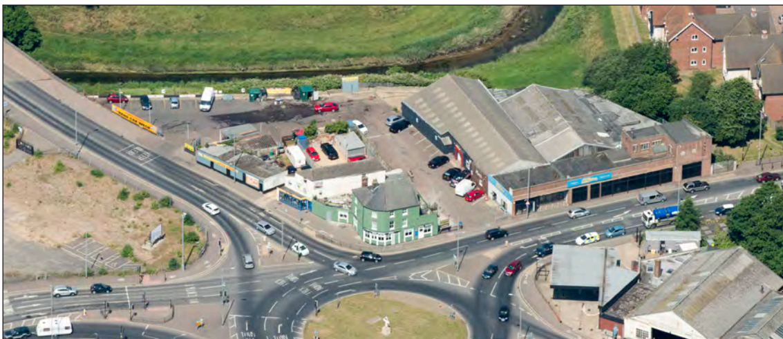
Fig126 An aerial view of area 4 from the south-east. Detail of HEA 33197/031 Damian Grady 19-JUN-2017 © Historic England
