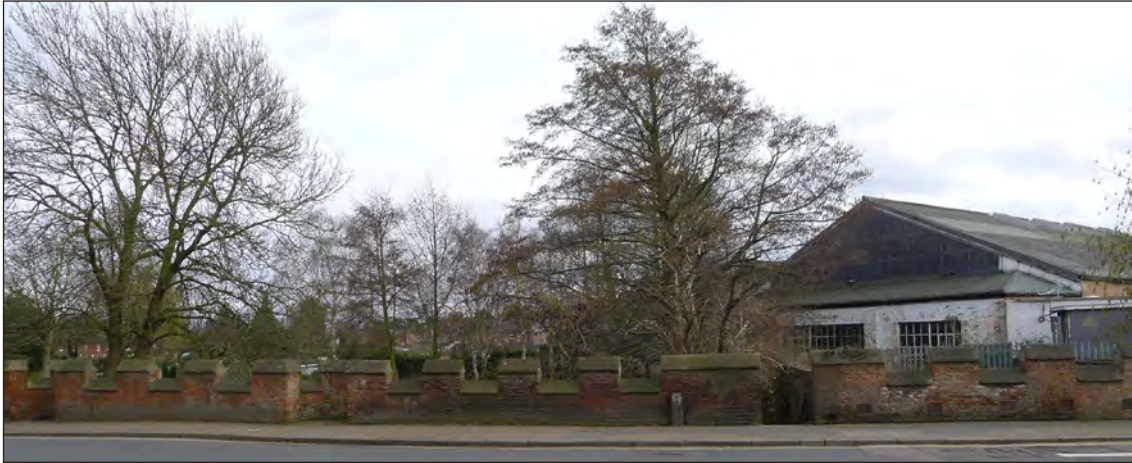
Fig 237 The battlemented dwarf wall which retains the carriageway added east of the South Gate in 1899-1900. Photograph Jonathan Kewley 27-FEB-2017 © Historic England
