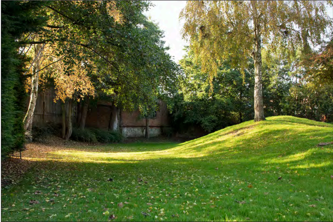
Fig 88 The former Middleton Stop Drain looking south-east (HEA DP219113 Patricia Payne 17-OCT-2017 © Historic England)
