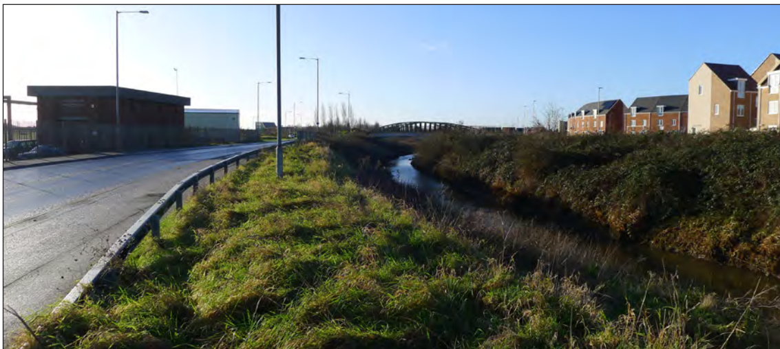
Fig 214 Looking south along Nar Ouse Way and the River Nar from just south of the HAA boundary. On the left is the Gaywood Internal Drainage Board Pierrepoint Pumping Station, on the right new housing on the former manure works site. Photograph Jonathan Kewley 16-JAN-2018 © Historic England
