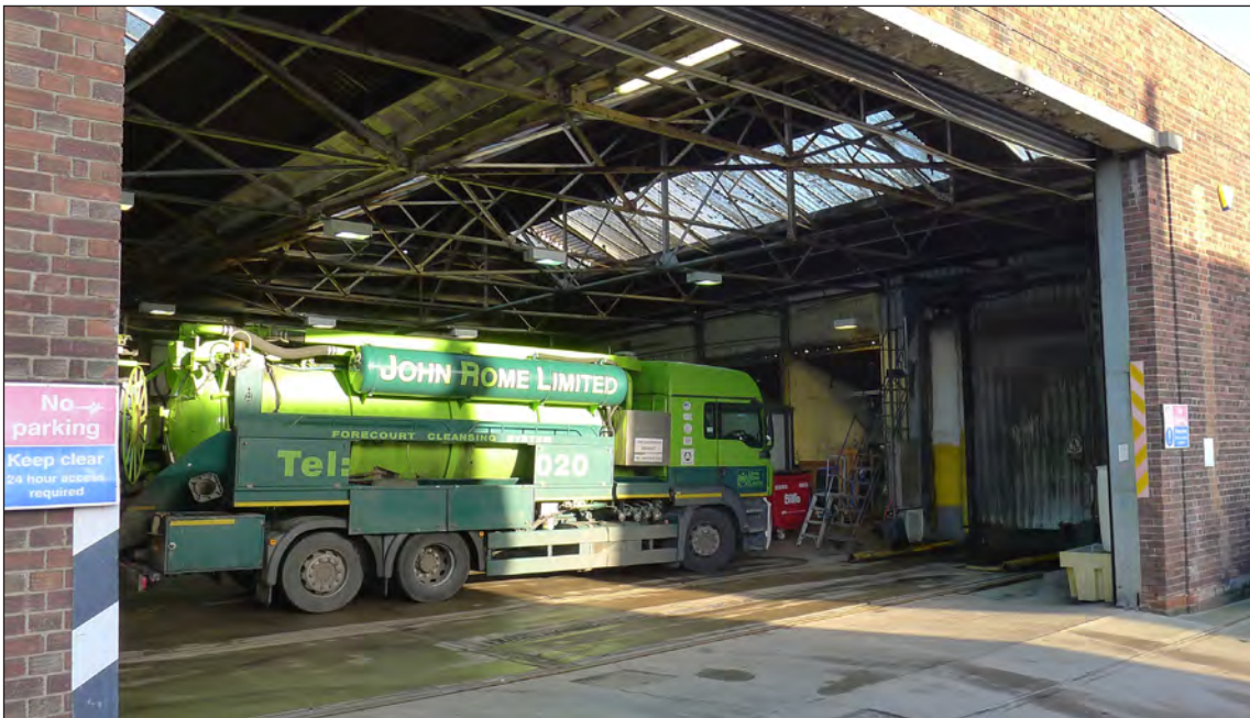
Fig 232 The interior of the eastern section of the Bus Garage, looking from Vancouver Avenue. Photograph Jonathan Kewley 16-JAN-2018 © Historic England
