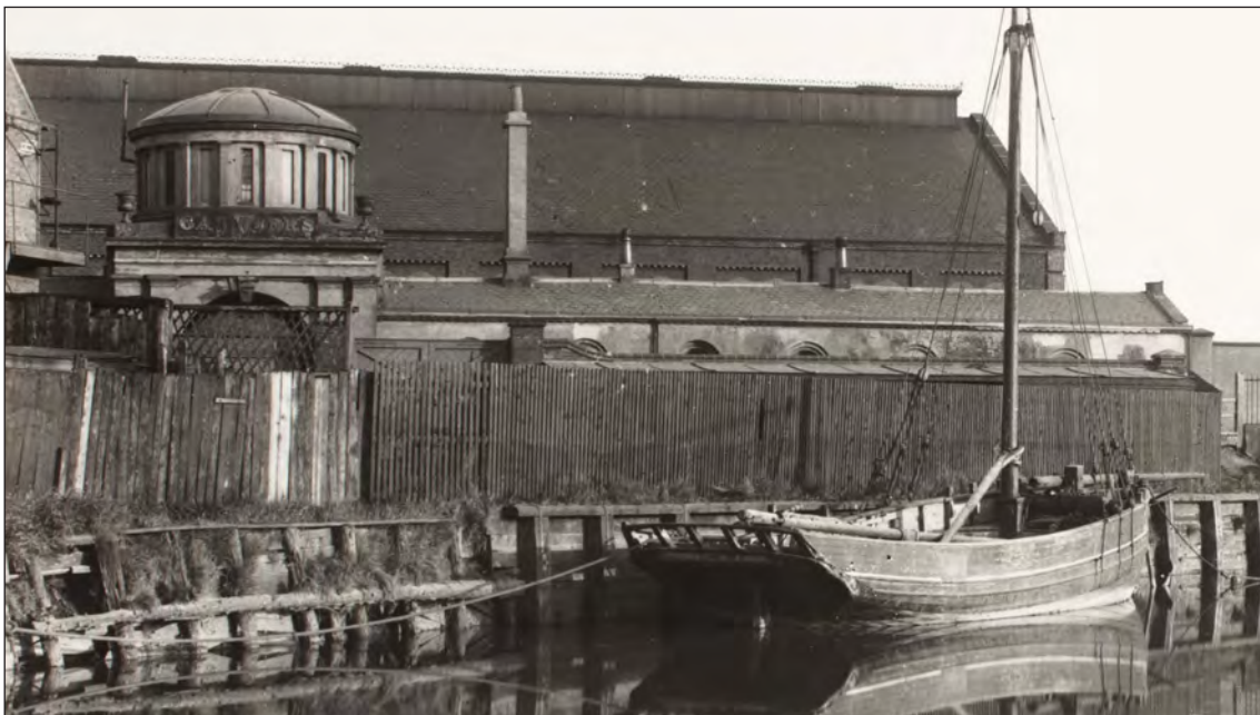
Fig 181 The Gas Works at some time in the late 19th or very early 20th century. The view is from the north, with the Nar in the foreground. Between the wooden fence and the handsome entrance building runs the Wisbech Road. Norfolk Library and Information Service (King's Lynn Library); image: detail of HEA DP219451
