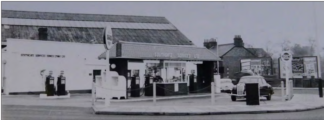
Fig 233 The filling station from the west c 1959-60, with the roof of the Bus Garage behind. Norfolk Library and Information Service (King's Lynn Library)
