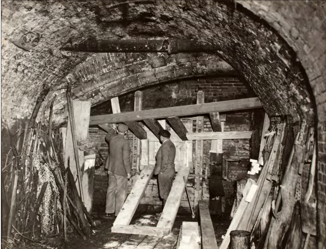
Underneath Southgates Bridge when the Middleton Stop Drain had temporarily been drained, probably in the 1950s. Note the stone arch immediately above the wooden beam. Norfolk Museums Service (Lynn Museum) MB03282. Image: HEA DP219363
