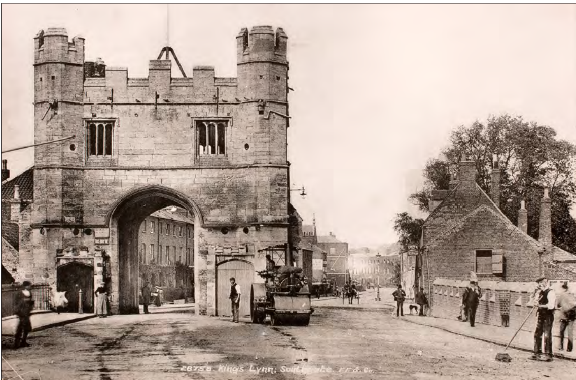
Fig 65 The South Gate from the south after the widening of the road in 1899-1900. Norfolk Museums Service (Lynn Museum) MB01086. Image: HEA DP219364
