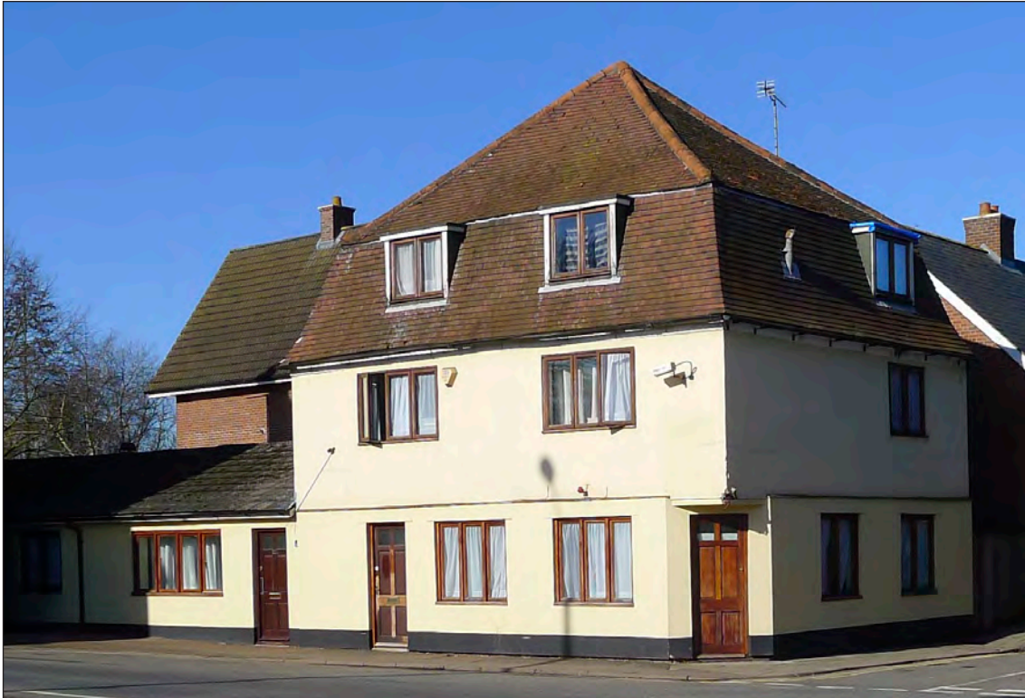
The former Honest Lawyer public house from the north-east. Photograph Jonathan Kewley 05-APR-2018 © Historic England
