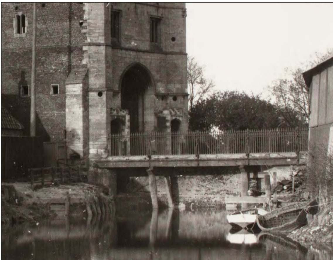
Fig 70 Southgate Bridge from the west, 1891, showing the footway cantilevered out for the 1841 pedestrian passage. Norfolk Library and Information Service (King's Lynn Library Archives). Image: HEA DP219448
