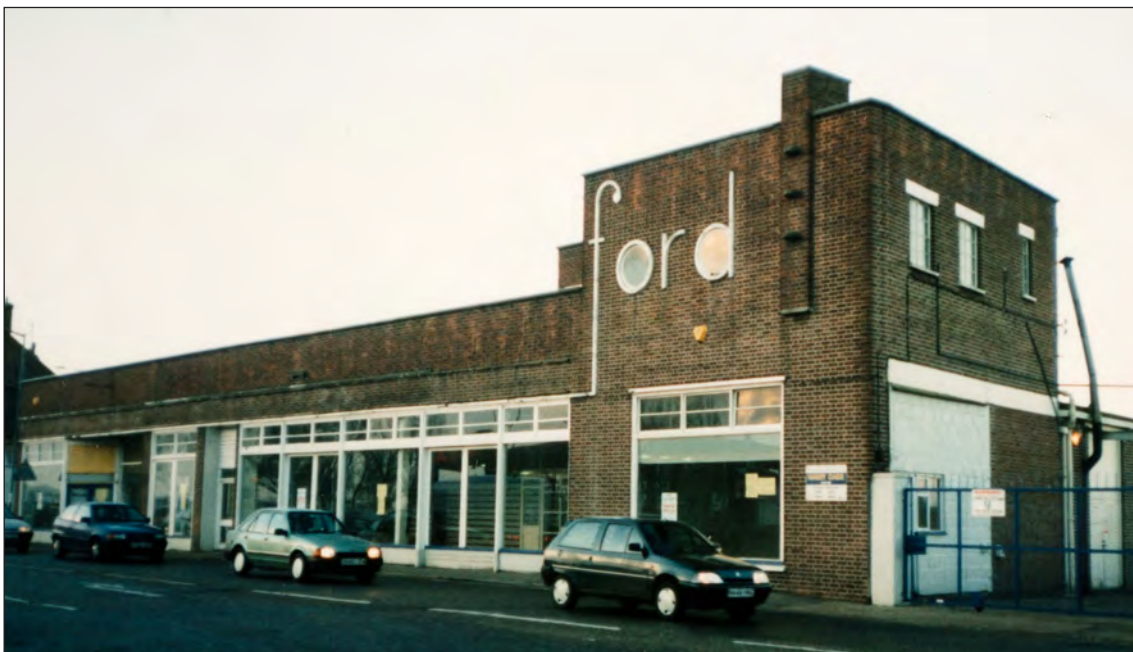
Fig 148 The former Ford garage from the north-east in 1996, showing the original windows. Norfolk Library and Information Service (King's Lynn Library Archives). Image: HEA DP219456
