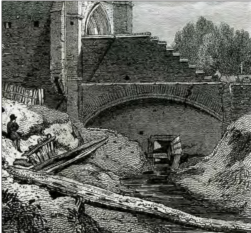
Fig 72 Southgate Bridge from the west by John Sell Cotman, 1818, showing the sluice in the blocked-up arch. Norfolk Museums Service (Lynn Museum NWHCM 1954.138.Todd18.Freebridge.145c.)
