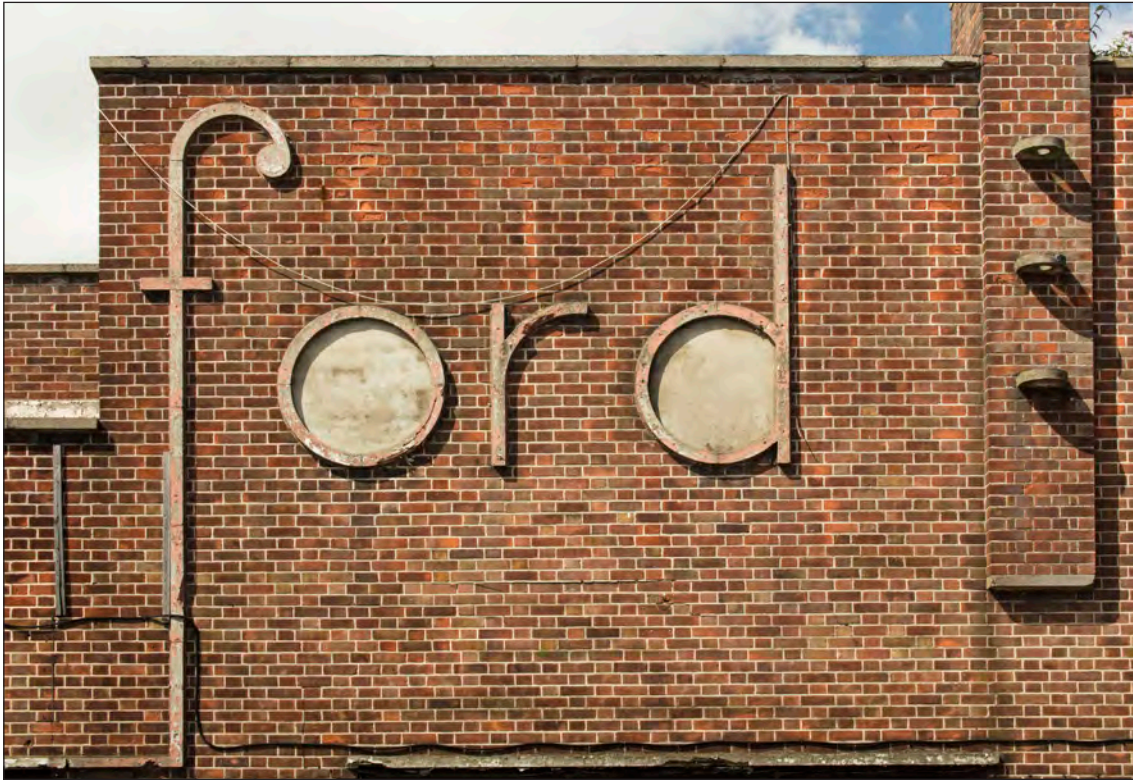
Fig 149 The 'ford' sign on the former garage. HEA DP219060 15-AUG-2017 Patricia Payne © Historic England
