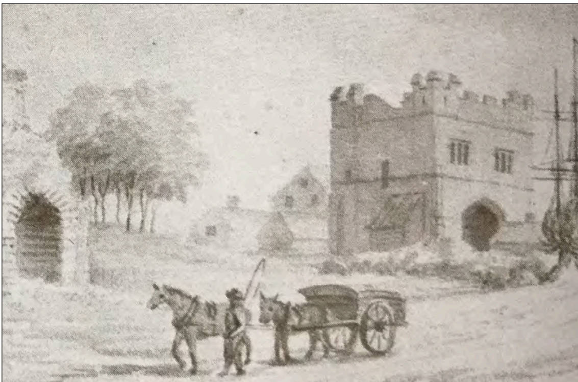
Fig 132 Detail of The Old Gannock Gates and South Gate (LA19) by the Rev Edward Edwards, showing, in the centre, buildings south of the South Gate. Norfolk Museums Service (Lynn Museum)
