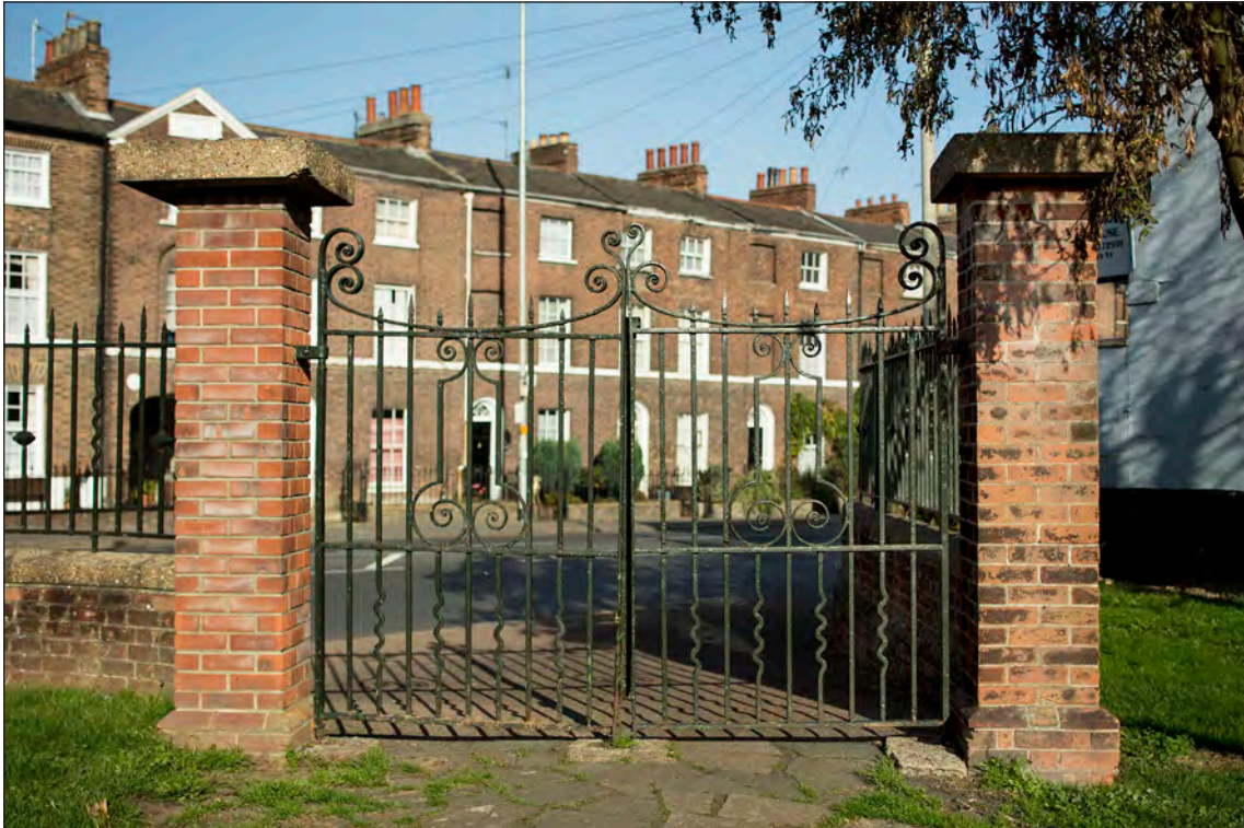
Fig 92. The gates at the northern end of the park's western boundary wall, looking north-west. (HEA DP219101 Patricia Payne 17-OCT-2017 © Historic England)
