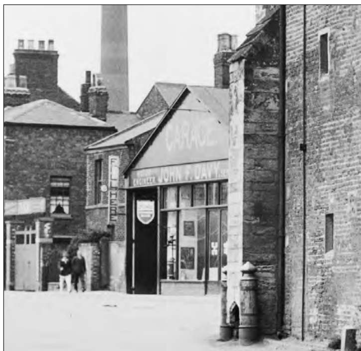
Fig 144 Looking south past the South Gate in 1928, showing John F Davy's garage. Detail of HEA op35020
