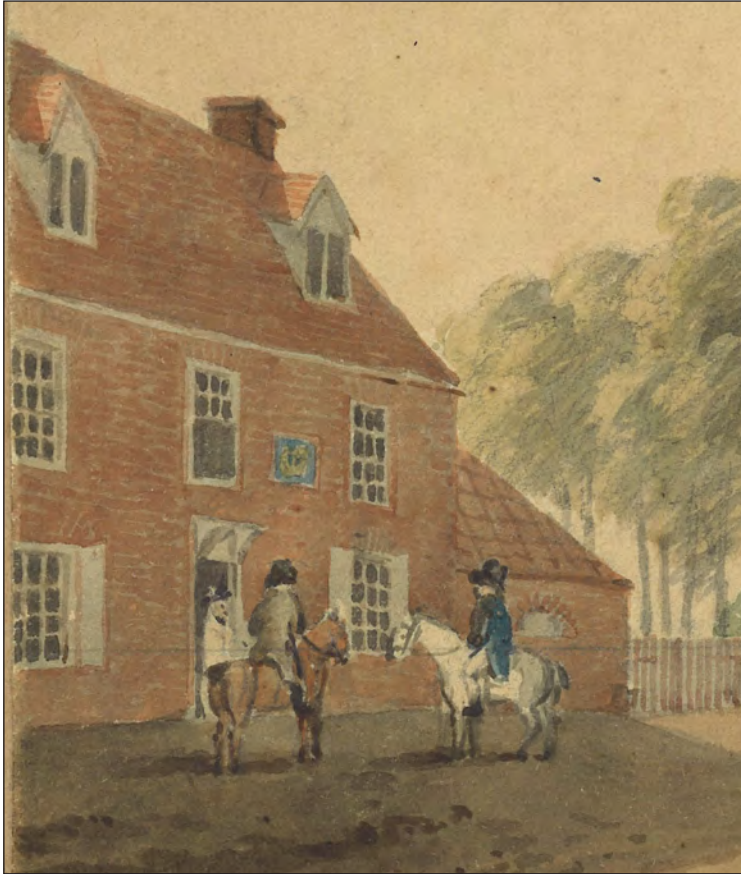
Fig 80 Detail of another watercolour by James Sillett showing the new Crown Inn from the north-west. The clump of trees to the right is somewhere near the south end of Out South Gates. Norfolk Museums Service (Lynn Museum) KILLM 1991.741
