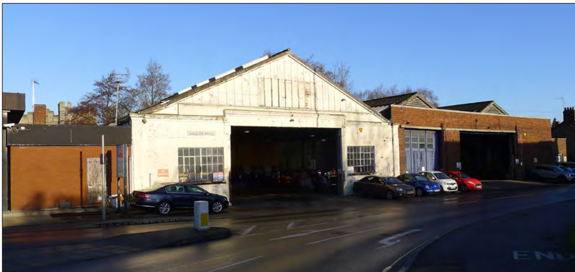
Fig 240 The Bus Garage from the south. Photograph Jonathan Kewley 16-JAN-2018 © Historic England
