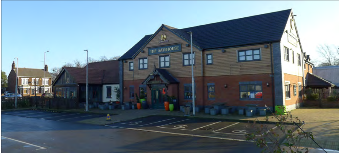
The west front of the Gatehouse 'pub restaurant' from Kellard Place. Photograph Jonathan Kewley 16-JAN-2018 © Historic England
