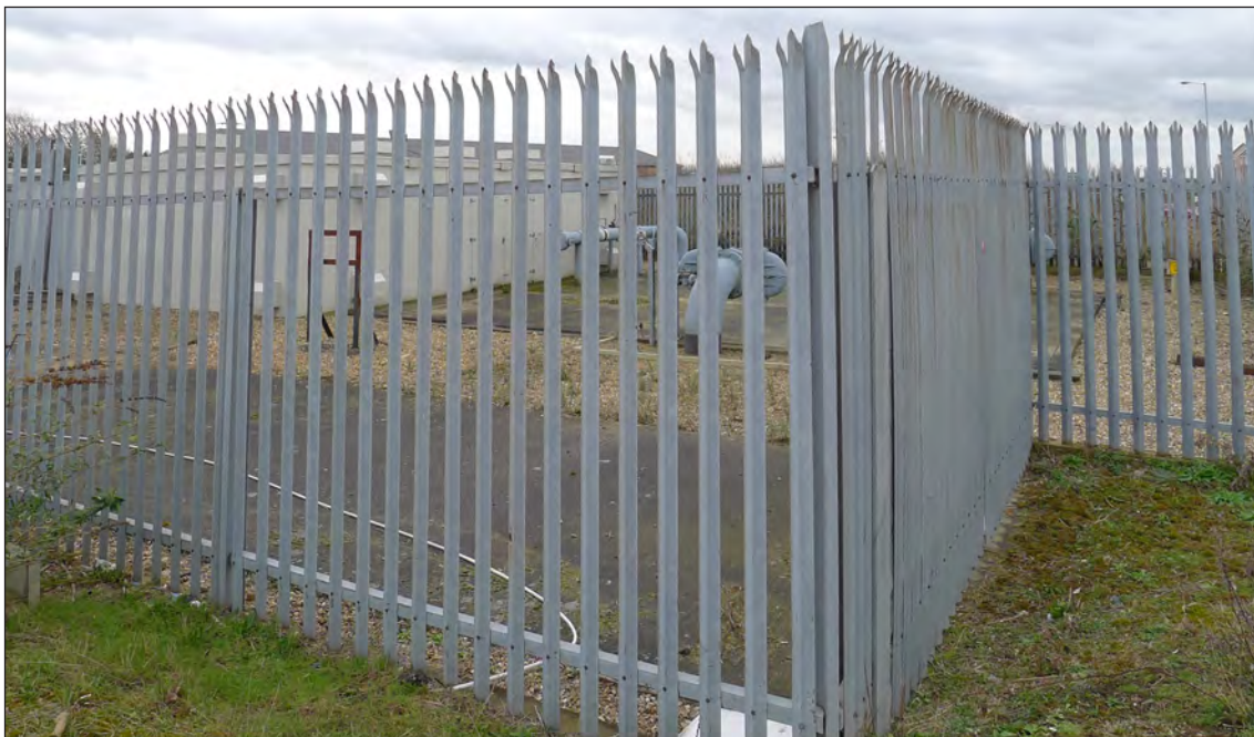
Fig 207 The National Grid Gas Pressure Reduction Station and Depot which lies between the Hardwick Road and Kellard Place; this view is from the north. Photograph Jonathan Kewley 27-FEB-2017 © Historic England
