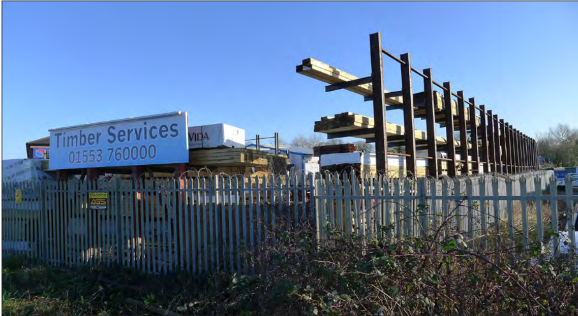
Fig 210 The yard of Timber Services Ltd on Horsley Field Industrial Estate; this view is from Nar Ouse Way, immediately south of the HAA boundary. Photograph Jonathan Kewley 16-JAN-2018 © Historic England
