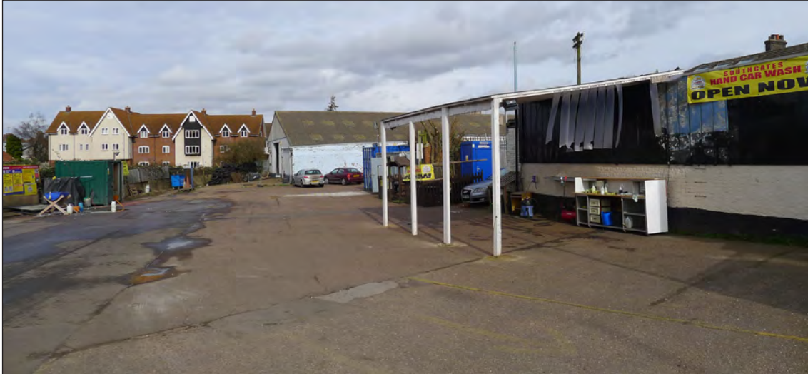
The hand car wash on the site of the demolished buildings west of the parade of shops on the Wisbech Road. Photograph Jonathan Kewley 27-FEB-2017 © Historic England
