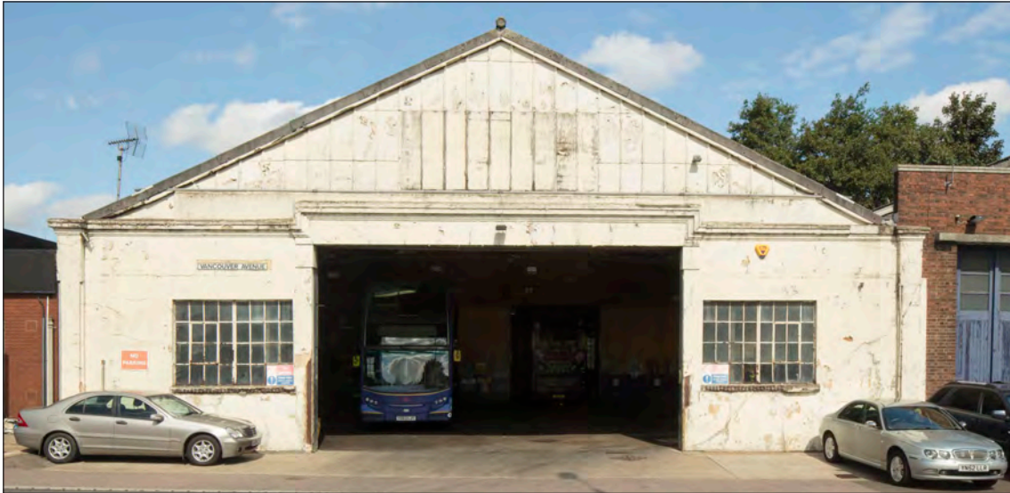
The principal, south front of the earlier half of the Bus Garage. Detail of HEA DP219056 15-AUG-2017 Patricia Payne © Historic England
