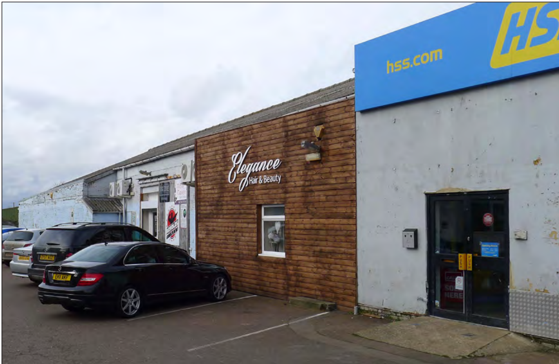
Fig 150 The south elevation of the former Ford garage. Photograph Jonathan Kewley 27-FEB-2017 © Historic England
