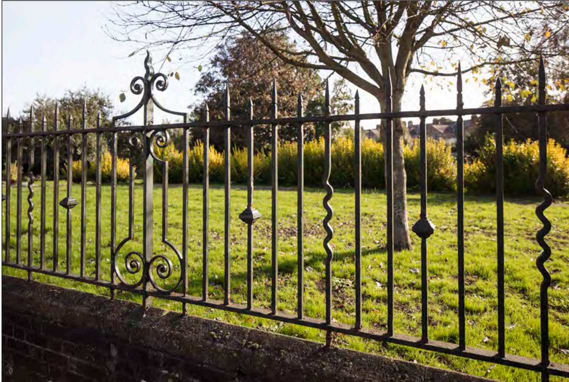
The railings on the park's western boundary wall, looking north-east. (HEA DP219103 Patricia Payne 17-OCT-2017 © Historic England)
