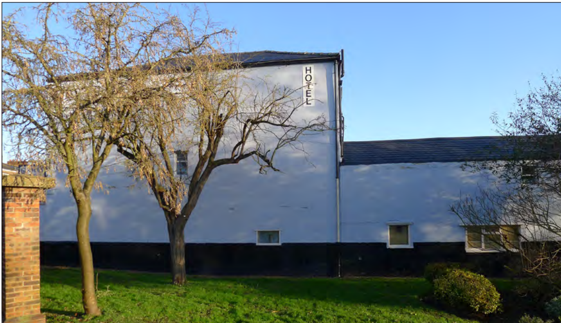
Fig 85 The Guanock Hotel (the most southerly building on Guanock Terrace) from Southgates Park. Photograph Jonathan Kewley 16-JAN-2018 © Historic England
