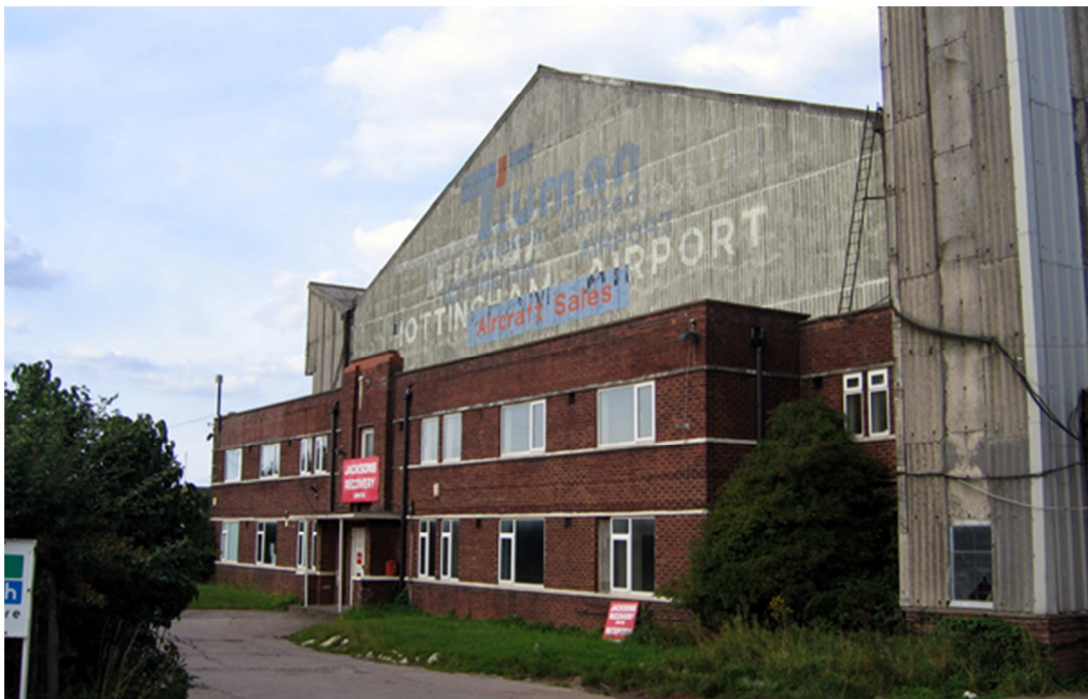
Figure 6: There are two ladders, one at either end of the roof truss, allowing access to the pair of roof gullies. [Milan Petrovic 07-08-2009]
