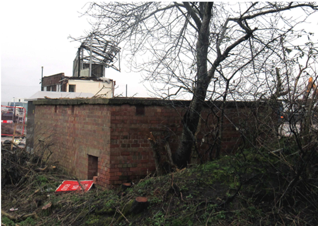
Figure 19: Air-raid shelter (Bldg.47) rear elevation showing two emergency escape apertures. [Milan Petrovic February 2017]
