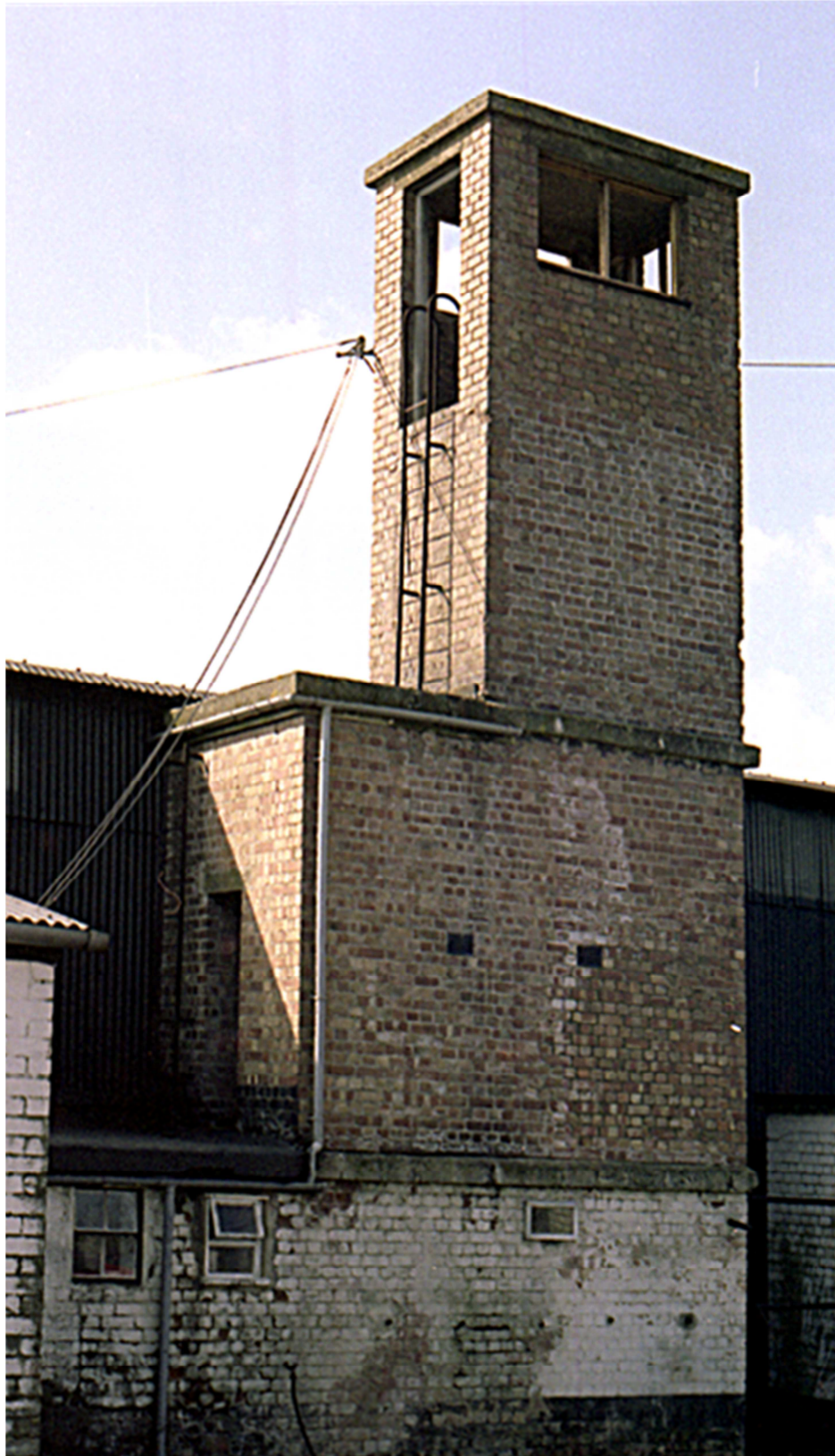
Figure 22: Built above the toilet annexe is this external example - NGR: SP 33466 61235, at Bishop's Tachbrook - a Stirling aircraft repair factory. The extra height enabled good views over two Bellman hangars. [Paul Francis 1993]
