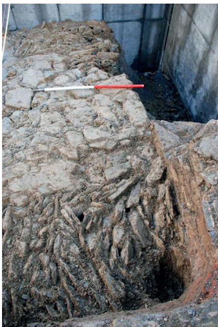
Fig.97. Cobbled flooring of a late medieval livestock building at Buckfast Abbey. The soft clay ground was first consolidated with a sub-base of tightly packed pitched stones (local slate stone) then another similar layer was set on top, and finally a stone rubble floor. There were two post-medieval floors on top, the last probably 19th century. Stewart Brown.
