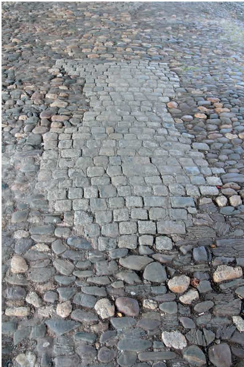
Fig.16. Exeter transit shed, the Quay. Cobbles patched with small granite setts.
