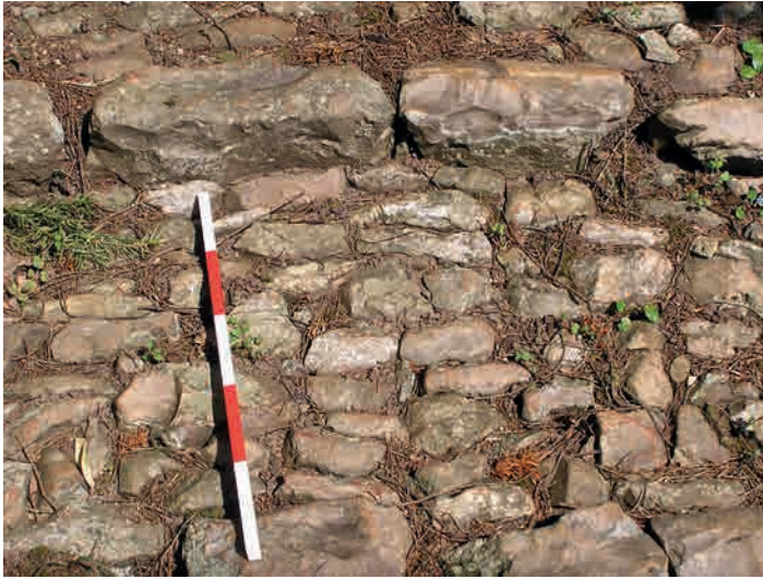
Fig.28. (Above) Chert cobbles at Offwell, St Mary on the S path to the lychgate. The 19th century porch (right) is surfaced with quartzite pebbles.
