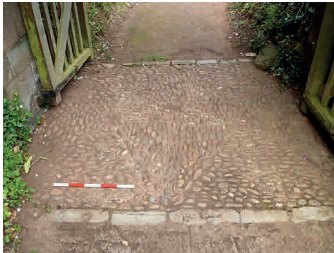
Fig.47. Variations on the lozenge pattern. Clockwise from top left. Hatherleigh, St John the Baptist, has very large lozenges; at Inwardleigh, St Petrock, the lozenges are contained by tramlines of internal kerbs. The lychgate at Clyst Hydon, St Andrew has a lozenge pattern contrived in pebbles. These are always less striking than those designed using flattish-topped cobbles.
