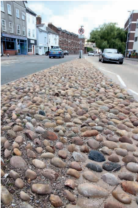
Fig.93. 'Keep off' 20th century pebble cobbles on a traffic island in Blackboy Road, Exeter, part of a hard landscaping scheme to control pedestrian movement. Large pebbles/small boulders are laid in cement, their irregular domed tops presenting a surface that no-one would choose to walk on.
