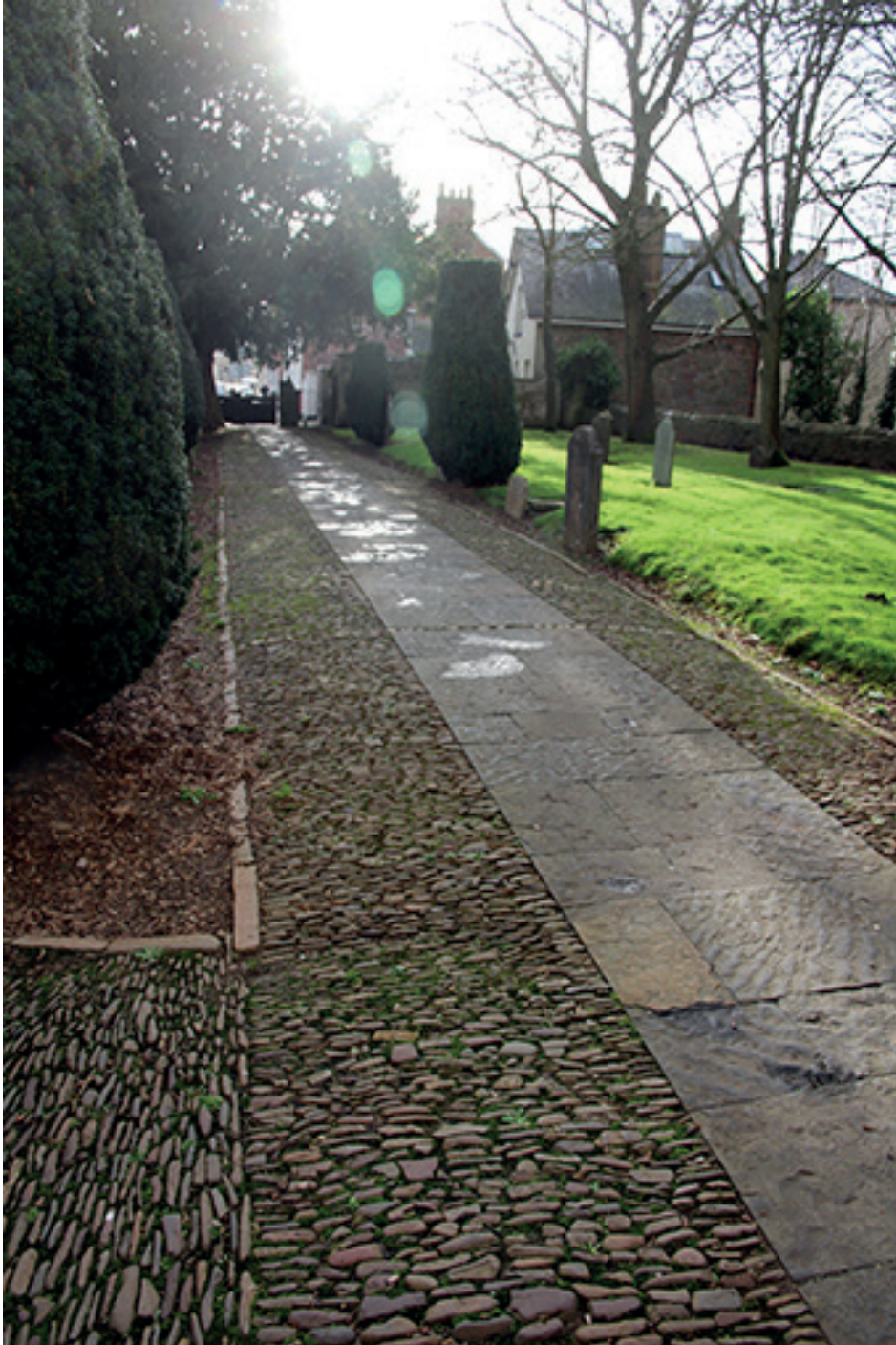
Fig.165. The riven surface of the new path at Tiverton St Peter collects water in wet weather, which is not ideal for access if it freezes, but was chosen as a better fit with context than Pennant with a smooth finish.
