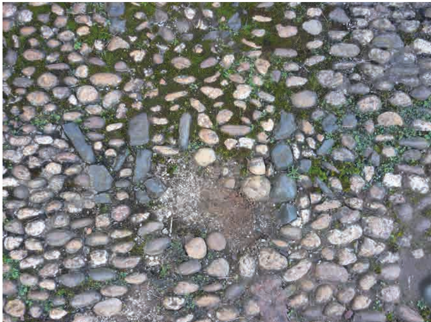
Fig.63. Some types of cobblestone may be able to withstand jointing loss better than others. Very small pebble-shaped cobbles at Poltimore are easily dislodged if only a small loss of jointing occurs.
