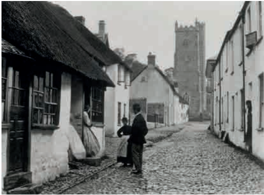
Fig.90. Moretonhampstead in a photograph of the 1870s showing a cobbled street, roadway and footway, in a Dartmoor town. The footway is on one side of the street only. Where buildings have been extended by front outshuts, presumably for shops, this is only a narrow strip. Moretonhampstead History Society, reproduced with permission.
