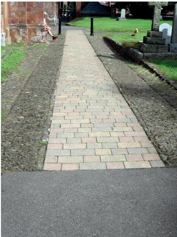
Fig.152. Examples of new paths through cobbles. Paved path of riven Pennant stone at Tiverton (top left). This has undulations greater than those recommended in Part M but considered to provide a more natural-looking finish. A path of paviours at Poltimore (top right). These provide a good surface for access but do not extend to the principal entrance, which is the one most-used. Concrete paviours inserted into a cobbled path at Crediton. These are visually assertive in the setting and it is disappointing that they lead to a very steep ramp into the church in the south porch.
