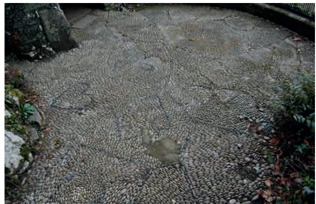
Fig. 103. A range of cobbled surfaces at Endsleigh, Milton Abbott, designed 1810. These employ flat-topped cobbles, including patterns (top); pebble cobbles with coloured patterns for the shell house (bottom right) as well as sheep's knuckles in a highly self-conscious Picturesque context (bottom left) Photographs by Oliver Bosence and Peter Marlow.
