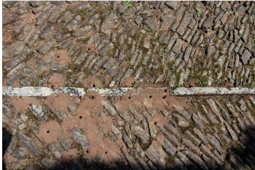
Fig.62. Insects at work at Sowton. Bees or wasps are nesting in the jointing material, throwing up casts onto the cobbled surface. As with earthworm activity this will affect the density and composition of jointing material and may make the cobblestones shift.
