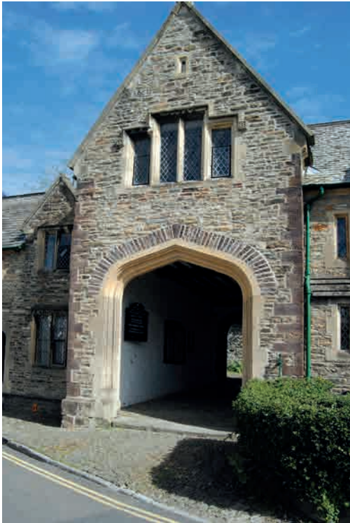
Fig.13. A cobbled footway outside the entrance to Pilton, St Mary, connects with cobbles under the 1849 entrance to the churchyard between almshouses and continues as a path through the churchyard to the porch.
