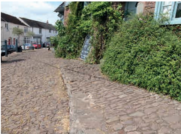
Fig.144. A cobbled 'doormat' outside the porch of Trusham St Michael (top left) has been relaid in cement losing the visual liveliness of traditionally-laid cobbles. This can be seen in more extreme form in a cobbled secular footway relaid in cement with cement kerbs at Sandford (right) which can be compared with other surviving Sandford footways (left), which have had some cement repair but are largely traditional.
