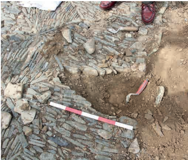
Fig.59. Left, excavation of the 2-phase Merton path revealed a sub-base incorporating small stones above formation level for the cambered, patterned section only. Below, sketch of the Merton camber by John Alexander. The section of plain path had gritty sand only in the bedding.
