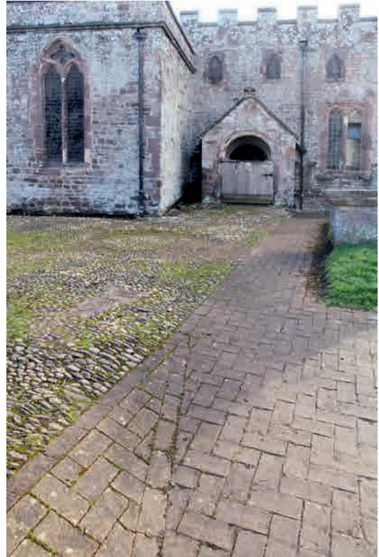
Fig.152. Examples of new paths through cobbles. Paved path of riven Pennant stone at Tiverton (top left). This has undulations greater than those recommended in Part M but considered to provide a more natural-looking finish. A path of paviours at Poltimore (top right). These provide a good surface for access but do not extend to the principal entrance, which is the one most-used. Concrete paviours inserted into a cobbled path at Crediton. These are visually assertive in the setting and it is disappointing that they lead to a very steep ramp into the church in the south porch.
