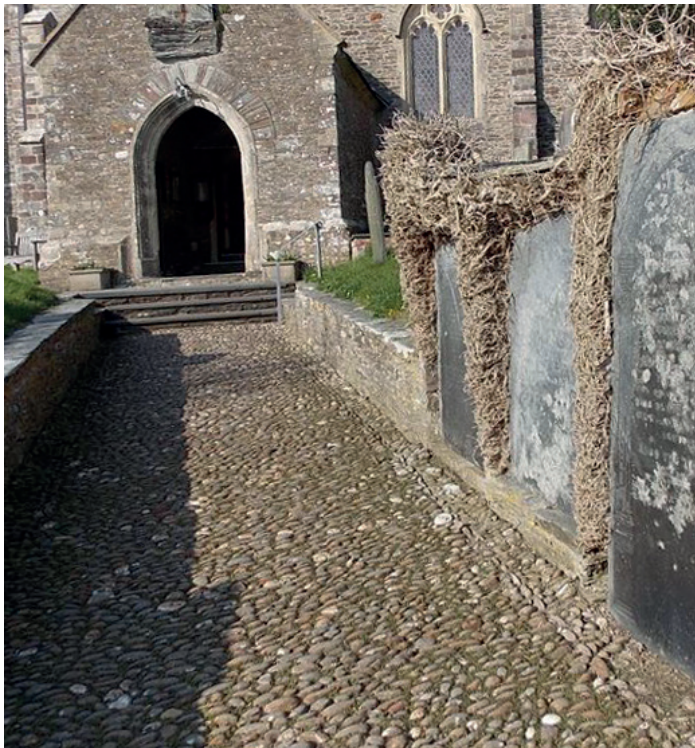
Fig.73. Paths between revetment walls that provide stable edge restraint are generally in better condition than paths with various types of small dressed or undressed stone kerbs.
