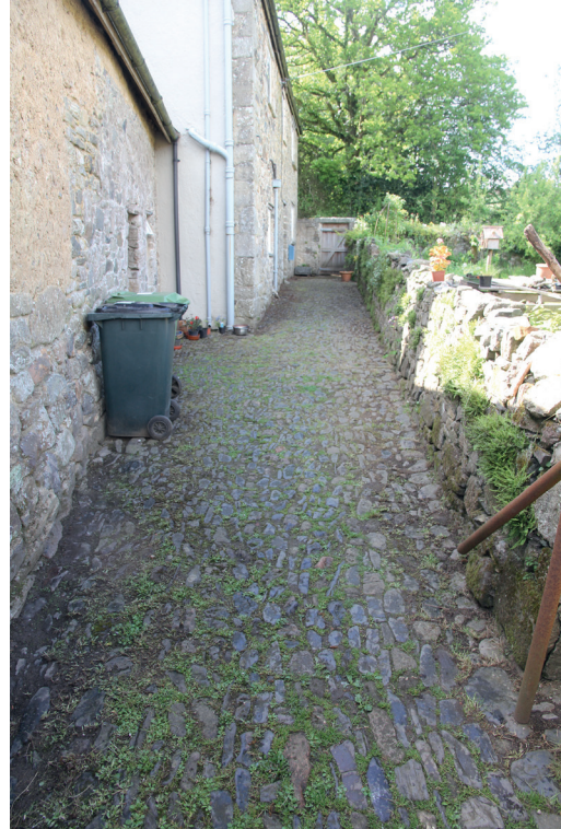
Fig.104. Left, a herringbone garden path to 19th century estate cottages at Upton Pyne and, right, a path to a farmhouse, Sweet Sigford where the cobbles are, unusually, laid along the long axis of the path.
