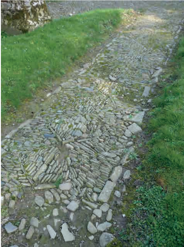
Fig.78. Path destabilisation at Huish inside the churchyard (left). Curiously, the large cobbled court outside the churchyard boundary, used for car parking, appeared to be in very good order (above), perhaps benefiting from the weight of vehicles.
