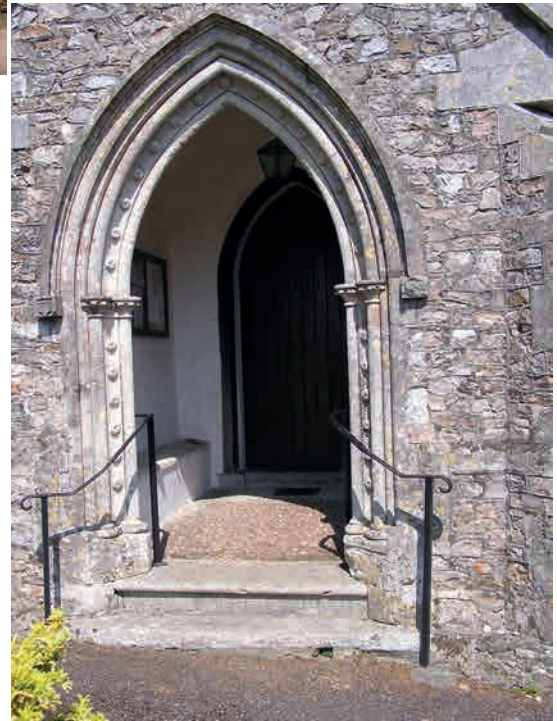
Fig.28. (Above) Chert cobbles at Offwell, St Mary on the S path to the lychgate. The 19th century porch (right) is surfaced with quartzite pebbles.
