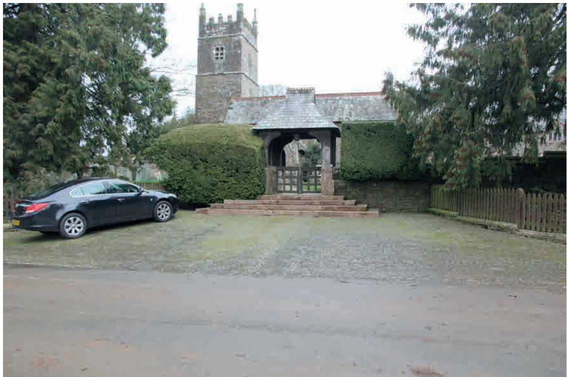
Fig.159. A large area of cobbles just outside the lychgate of Upton Pyne church has been completely relaid (probably in the 1980s). This is used for vehicles, which do not seem to have damaged the surface. The court at Huish is also used for parking. The cobbled surface appears to be in very good condition, although the paths inside the churchyard boundary are not.
