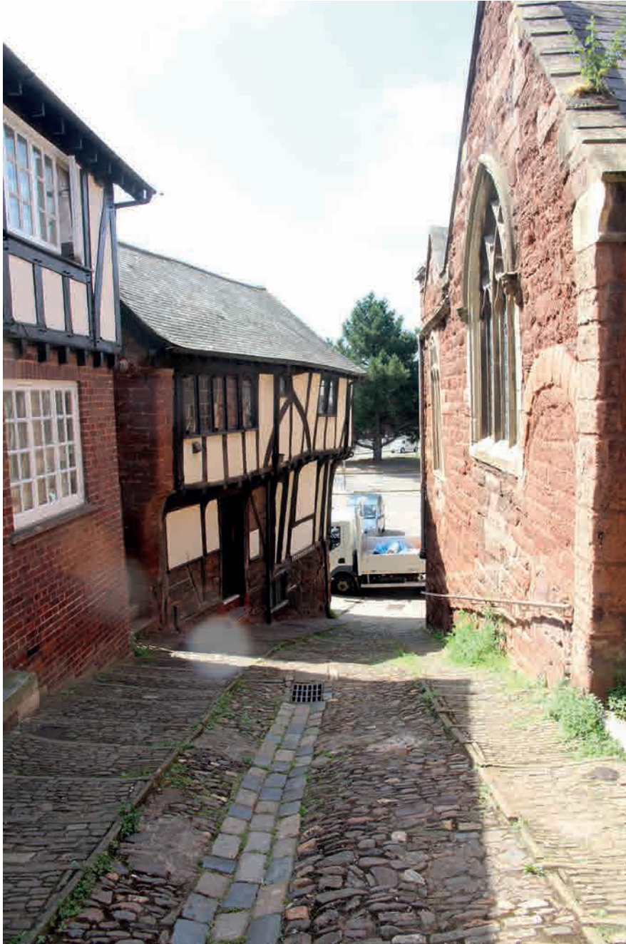
Fig.91. Stepcote Hill. A survival, somewhat altered, of a commonplace type of urban street surface with large roadway cobbles either side of an open drain and smaller footway cobbles. It is probably 19th century. The drain has been partly underground and the risers of the steps of the cobbled footways, now stone, were timber at one time.
