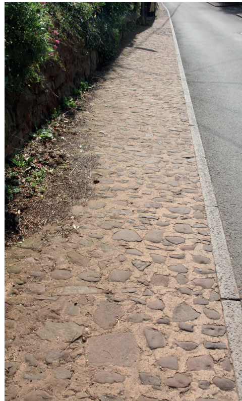
Fig.144. A cobbled 'doormat' outside the porch of Trusham St Michael (top left) has been relaid in cement losing the visual liveliness of traditionally-laid cobbles. This can be seen in more extreme form in a cobbled secular footway relaid in cement with cement kerbs at Sandford (right) which can be compared with other surviving Sandford footways (left), which have had some cement repair but are largely traditional.
