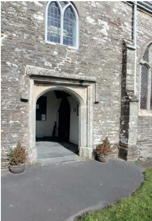
Fig.37. Loddiswell, St Michael, in the largely cobble-free zone of the South Hams, has both a slate-floored porch and the body of the church is flagged with slates. Is the tarmac path a replacement of slate flags?
