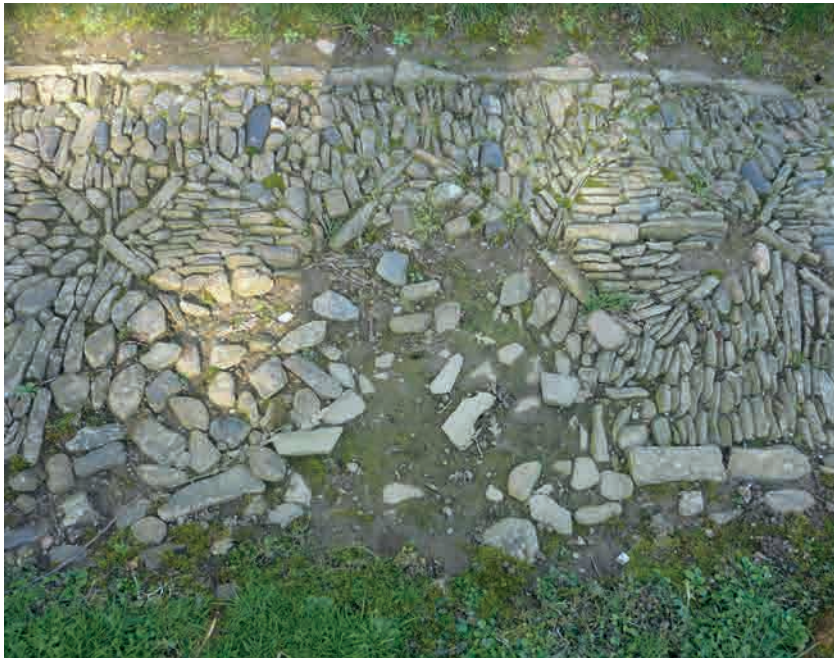
Fig.72. The curious 'floating apart' of one of the paths at Huish may relate to poor churchyard drainage. When visited all the Huish paths had fleshy weeds growing out of the jointing.
