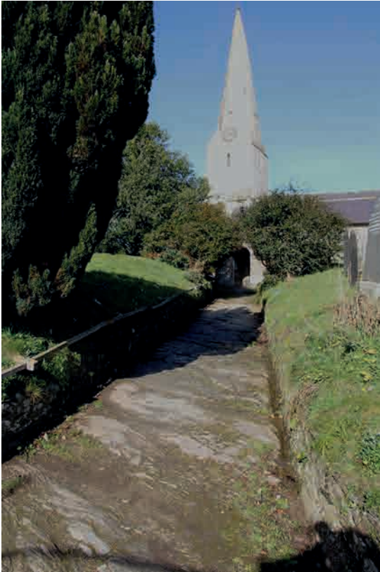
Fig.35. Diptford, St Mary, has a lop-sided bedrock path. There have been attempts to level parts of it up with cement.
