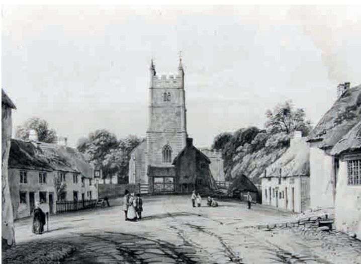
Fig.113. Examples of Spreat's 1842 engravings of selected Devon churches. The only churchyard where cobbles are definitely shown is Whitestone, just outside Exeter (top), with detail. These have disappeared. His engraving of Chudleigh (left) shows cobbled footways and an uneven road surface. The churchyard has a stile and a thatched building, perhaps a church house, built partly inside the boundary, which is part masonry wall and part wooden fencing.
