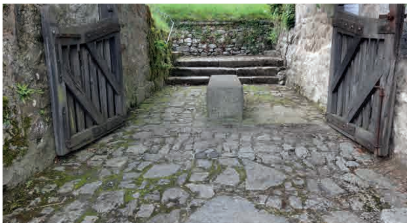
Fig.15. The range of cobblestone sizes illustrated in the contrast between the tiny cobbles at Petrockstow, St Petrock, above, and the large cobbles? or should they be called random stones? at Throwleigh, St Mary, below.
