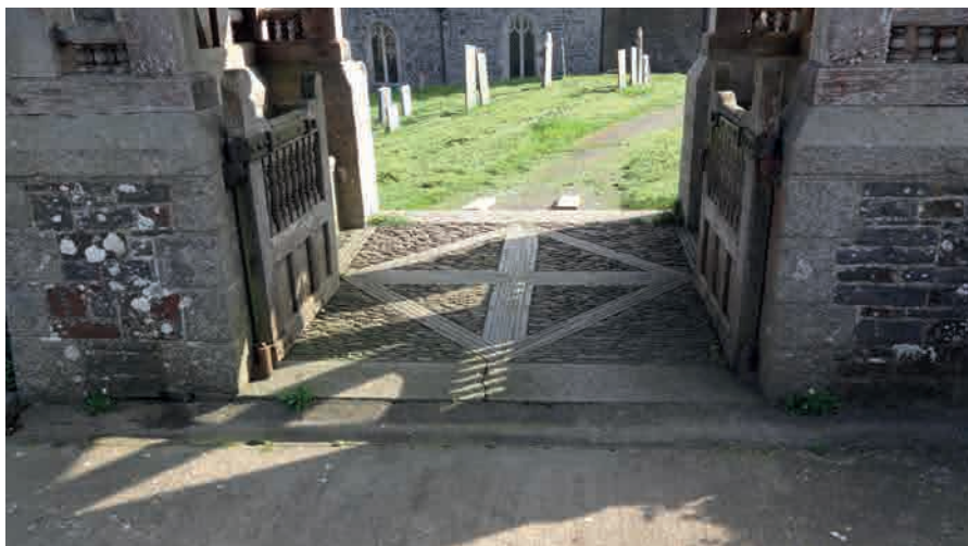
Fig.34. The 1908 patterned cobbles of the lychgate at Warkleigh, St John the Evangelist. Cobbled lychgates appear usually to have been built independently of work on church paths.
