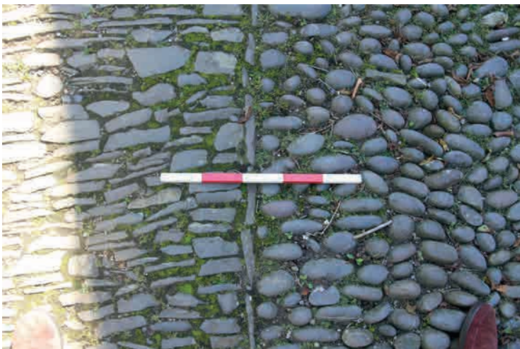
Fig.25. Pilton, St Mary. A unique example of flat-topped and slightly domed Carboniferous sandstone cobbles used side-by-side, presumably two different phases.
