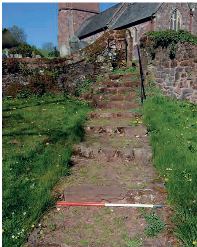
Fig.52. Various flights of cobbled steps. This page. Offwell, St Mary (left), closed for safety reasons; Dunchideock, St Michael and All Angels (right). Nest page (top), Sandford, St Swithun, showing a cobbled village pavement and the steep rise of cobbled steps to the S porch and (below) South Tawton, St Andrew, cobbled steps as part of a very fine Arts and Crafts lychgate of 1903. These examples of cobbled steps show how cobbles can morph from the vernacular into the polite, satisfying the principles of Picturesque as well as Arts and Crafts architecture.
