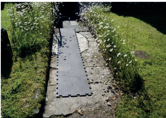
Fig.169. Temporary rubber matting over uneven slabs at Marwood.
