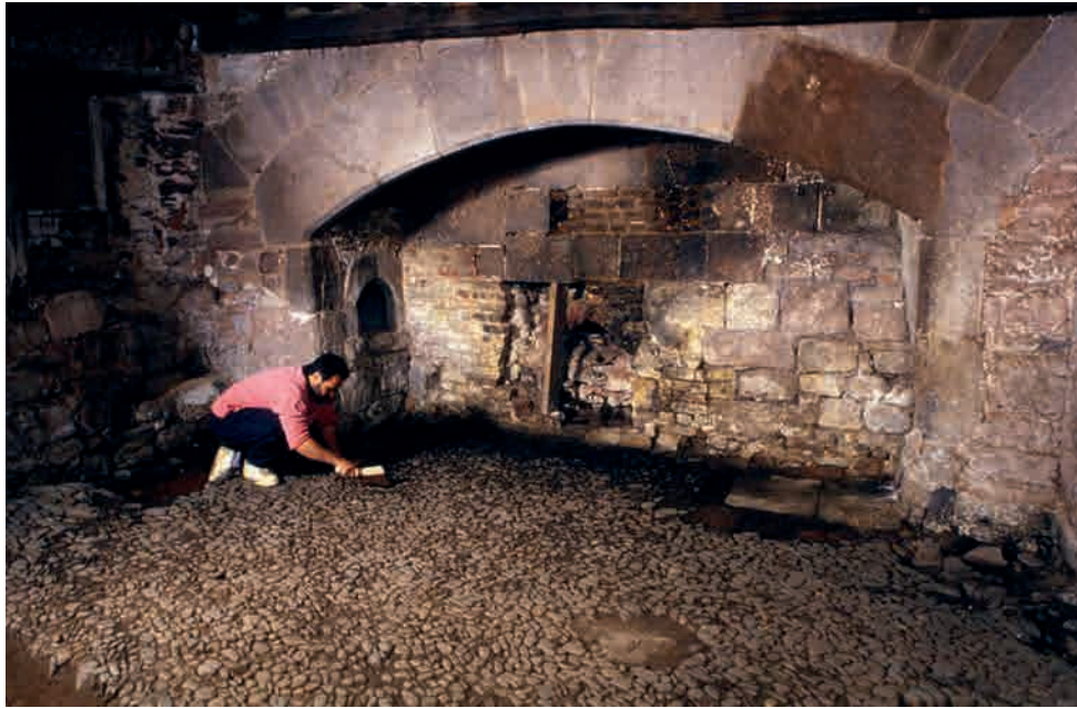
Fig.102. Bowhill, Exeter, kitchen cobbles, probably early 18th century. David Garner for Historic England.
