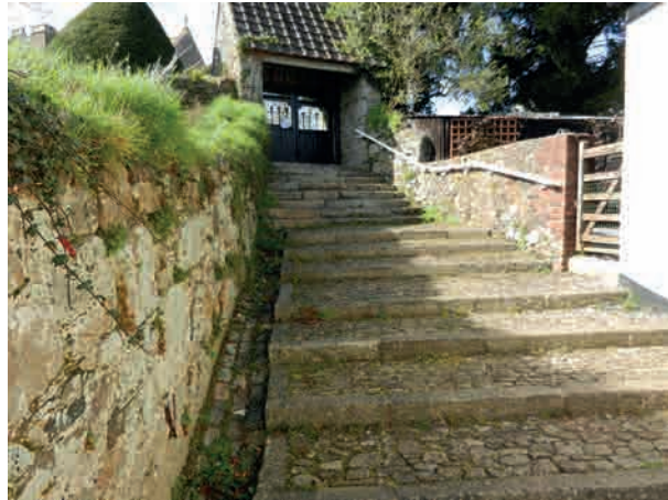
Fig.148. Examples of handrails to steps: (left) Sandford, cantilevered, on the left side, (right) Ilington on the right (avoiding the drainage channel). Handrails on both sides of a path, if possible, are helpful to both right-handed and left-handed people, travelling up or down a flight of steps.
