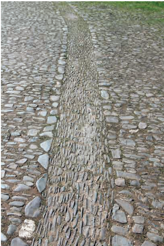
Fig.42. Small cobbles selected for a surface drainage channel in 'the Causeway' outside the lychgate of Upton Pyne, St Mary.
