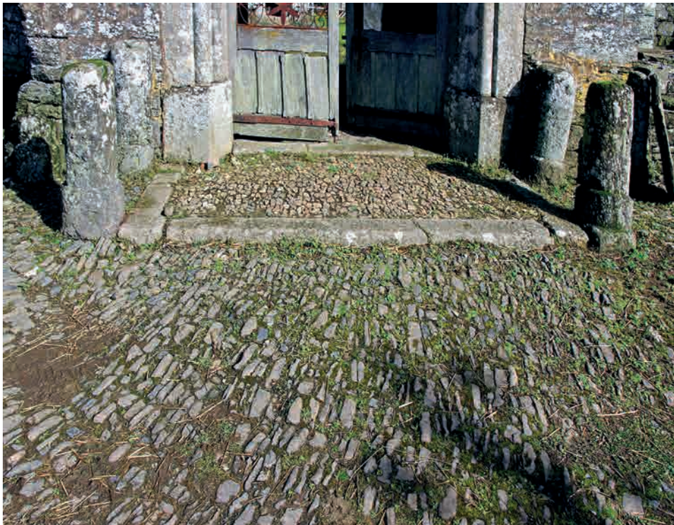
Fig.106. Bradstone Manor. Judging from context the sandstone cobbles in the foreground may be 17th century. The more dainty quartzite cobbles of the step are thought to be 19th. JRL Thorp.
