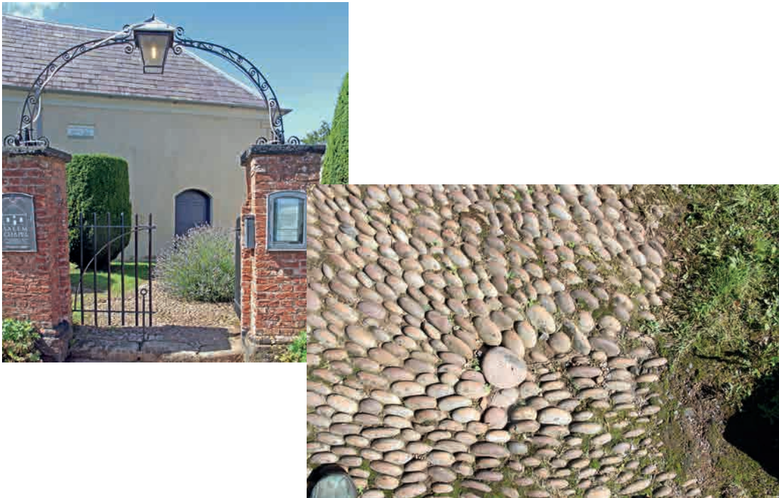
Fig.22. Quartzite pebble cobbles from the E Devon pebblebeds used for a court outside Salem Chapel, E Budleigh. The domed shape of the stones, rising above the bedding, make these uncomfortable to walk on and they do not provide a secure purchase for a walking stick.
