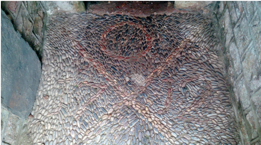
Fig.17. (Above) Kingskerwell, St Mary, dated 1712. Located close to the 'Devon marble' limestone area of South Devon, this is interpreted here as masons' offcuts used for the patterned area in grey and pink.
