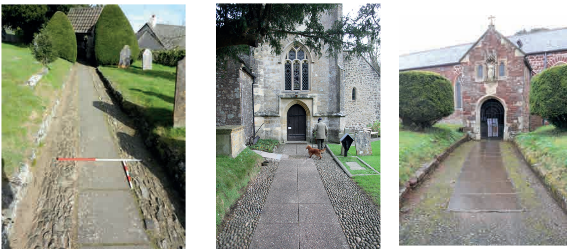
Fig.162. Concrete slabs driven through cobbled paths at Ilington (c.1970s); Salcombe Regis, driven through a pebble path and Alphington, the slabs discontinuous, presumably to retain a patterned area in the cobbles.
