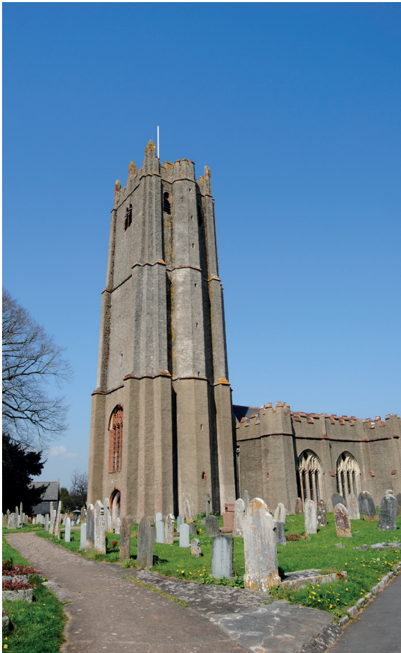
Fig.145. Examples of cement and tarmac path surfacing leave a church 'high and dry' in its setting and, unlike cobbles, do not provide a pleasing link with the churchyard landscape. Clockwise from top left: Alwington; Iddesleigh; Ipplepen.
