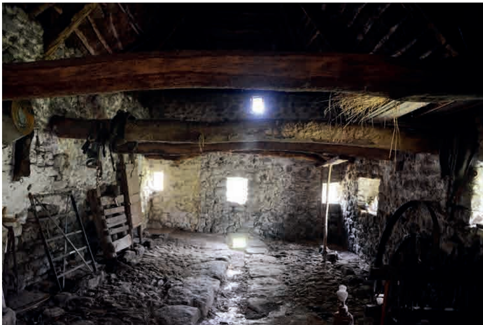
Fig.6. Random-laid granite cobbles of probable late medieval date provide functional rough-surfaced platforms for cattle on either side of a central drain in the shippon end of a Dartmoor longhouse, Higher Uppacott, Poundsgate. The flooring may be as early as the 14th century, the date of the primary phase of the longhouse. J R L Thorp.
