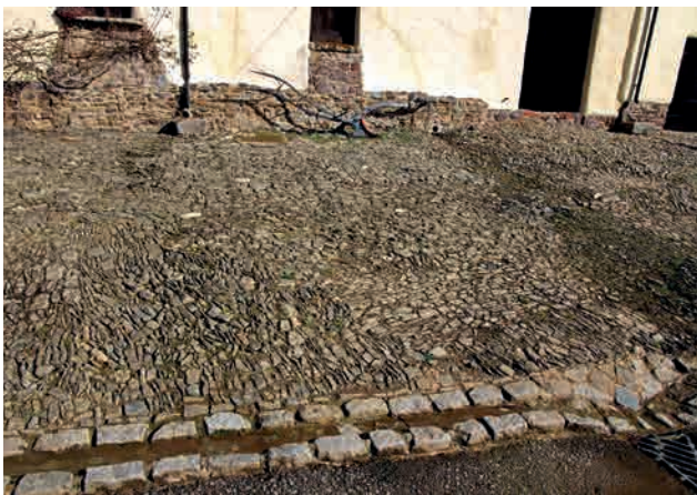
Fig.95. Cobbled farmyards: Gotham, Tiverton (top left) on a steeply sloping site; a mid Devon farmstead with cobbled footways and cobbled interiors to the buildings (two right-hand photos); cobbles in the farmyard at Great Heale, Colebrooke (below). Great Heale by JRL Thorp.
