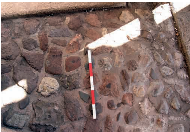
Fig.83. The relaid cobblestones from a Roman Road surface in Exeter are large, some more than 20cms on the surface and include irregularly-shaped pieces of the distinctive red conglomerate found at Heavitree on the eastern outskirts of Exeter, some purplish volcanic stone, found on the south west side of the city (Poccombe stone) and one or two water-worn stones probably pulled out of the River Exe. Poccombe stone was used in the Roman City walls.
