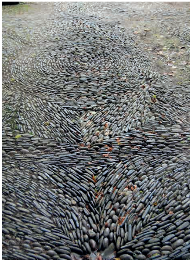
Fig.48. Meeth, St Michael (top). A unique example of whorls, used here in the porch (cobbles dated 1818). A more elaborate version of whorls was used in a secular context at the Picturesque Swiss Cottage at Endsleigh, designed 1810 by Sir Jeffry Wyattville for the Duke of Bedford, with grounds laid out by Repton. Endsleigh cobbles photograph by Peter Marlow.
