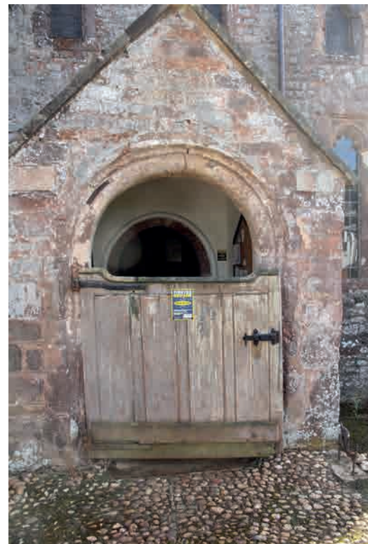
Fig.125. The jambs of outer porch doorway of many churches preserve fittings for gates or doors. Few survive: the example at Poltimore St Mary is probably early 19th century. Documentary references sometimes distinguish between the 'churchyard' gate and the 'church' (presumably porch) gate. These gates may have designed to keep livestock out of the porch.
