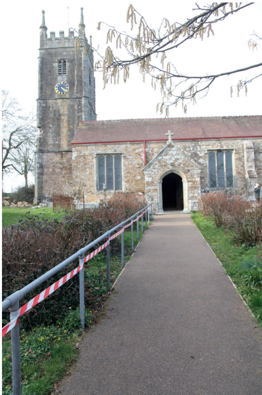
Fig.168. 'Playtop' laid over the Black Torrington cobbles, which are protected by a membrane. The detailing is utilitarian.
