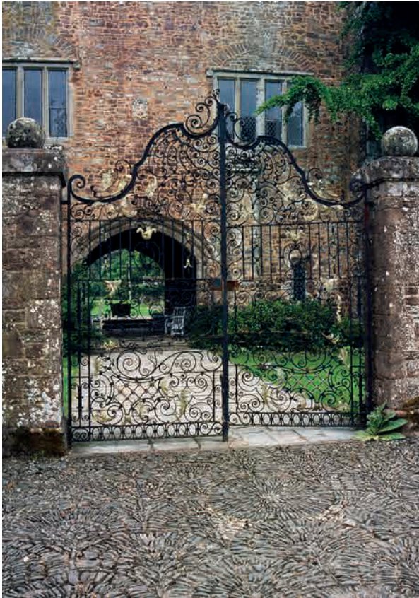
Fig.5. Cobbles laid in fans in front of the 18th century Italian gates at the entrance to Bickleigh Castle: the castle (really a fortified house) was restored by successive owners after 1925. Nothing as elaborate as these fan patterns, a continental European tradition, is found in churchyard paths. Dr Stuart Blaylock.
