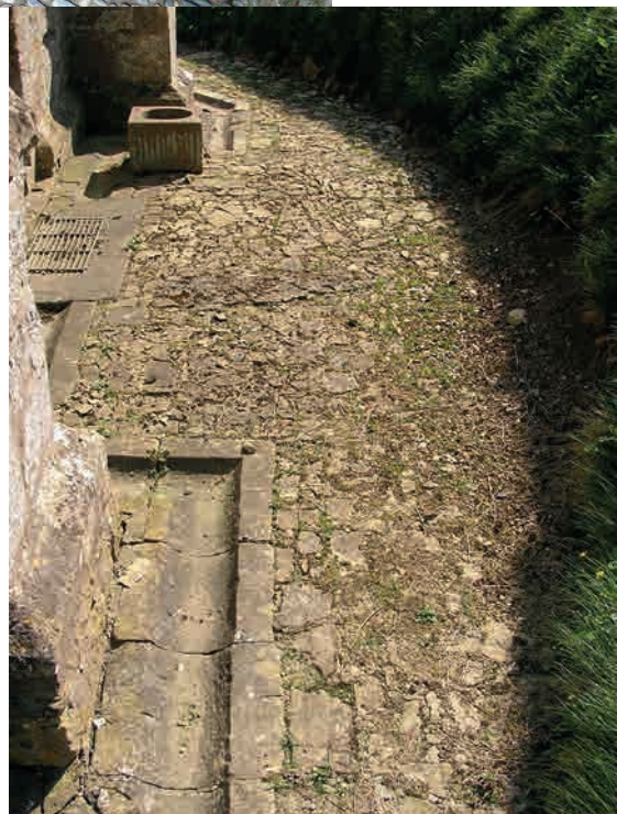
Fig.18. (Right) Membury, St John. This cobbling may use quarry waste from the nearby Tolcis quarry that produced white lias.
