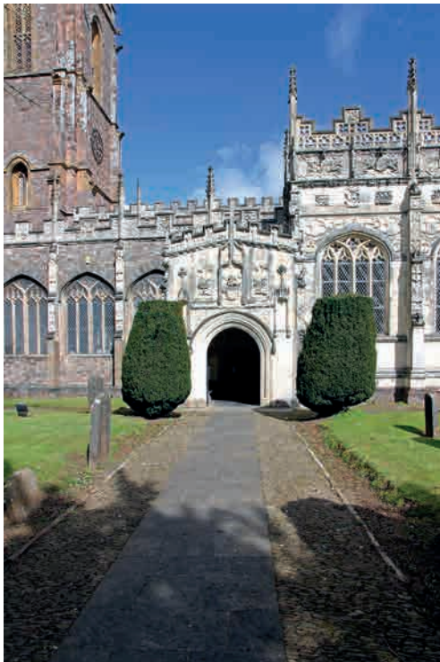
Fig.164. A path of riven Pennant stone driven through cobbles at Tiverton St Peter. It was possible to preserve white quartzite initials in one of the cobbled borders. Level access from the footway outside the church and into the S porch made this a less complicated amendment for improved access than might be the case on another site.
