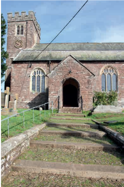
Fig.148. Examples of handrails to steps: (left) Sandford, cantilevered, on the left side, (right) Ilington on the right (avoiding the drainage channel). Handrails on both sides of a path, if possible, are helpful to both right-handed and left-handed people, travelling up or down a flight of steps.
