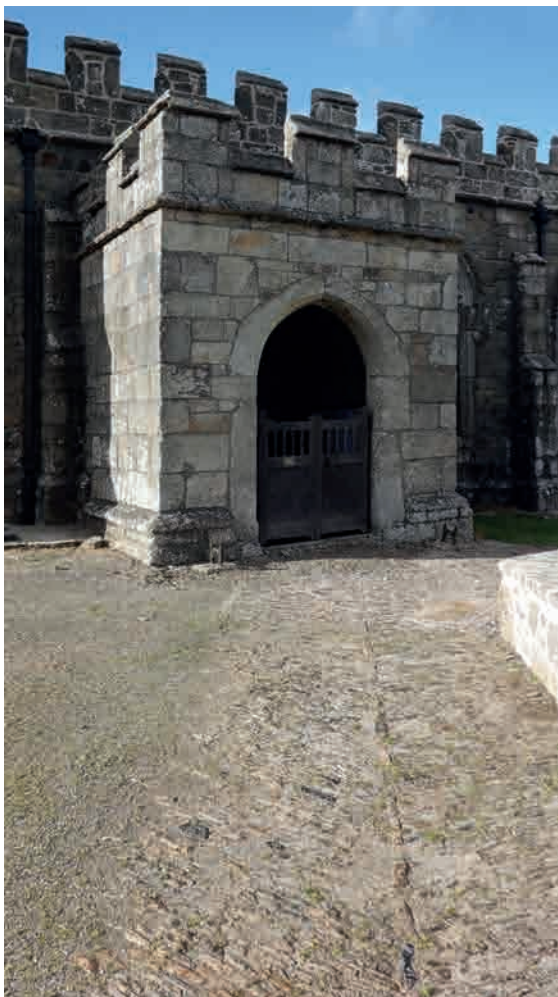
Fig.29. (Left) South Tawton, St Andrew. Abundant use of granite for the building, for revetment walls to the path and for an apron round the church, but sandstone cobbles used for the path.
