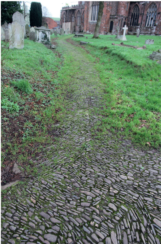
Fig.80. A sub-path at Crediton disappearing as grass invades from the sides. Next page (top), a highly-Romantic route to Buckland Brewer church beneath coppiced trees. The cambered path is carpeted with moss and most church-goers prefer to use an alternative route. Below. A fleshy weed growing out of the jointing of one of the Huish paths.
