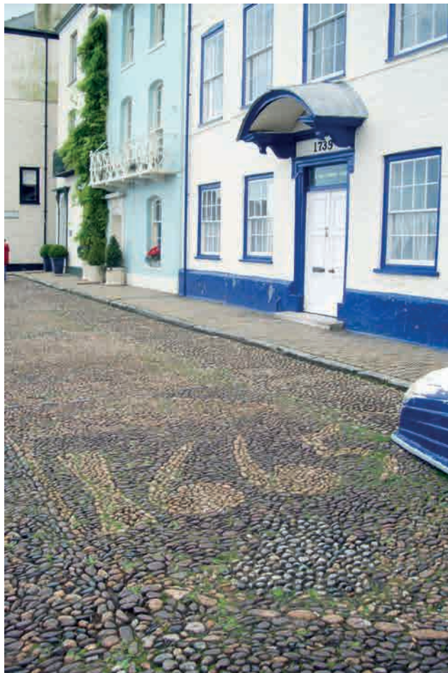
Fig.86. Dated cobbles at Bayard's Cove, Dartmouth. The form of the numbers making up the date is convincing, even if there has clearly been much re-laying over time. These are the earliest internally-dated cobbles in Devon known to the authors of this report. Dr Stuart Blaylock.
