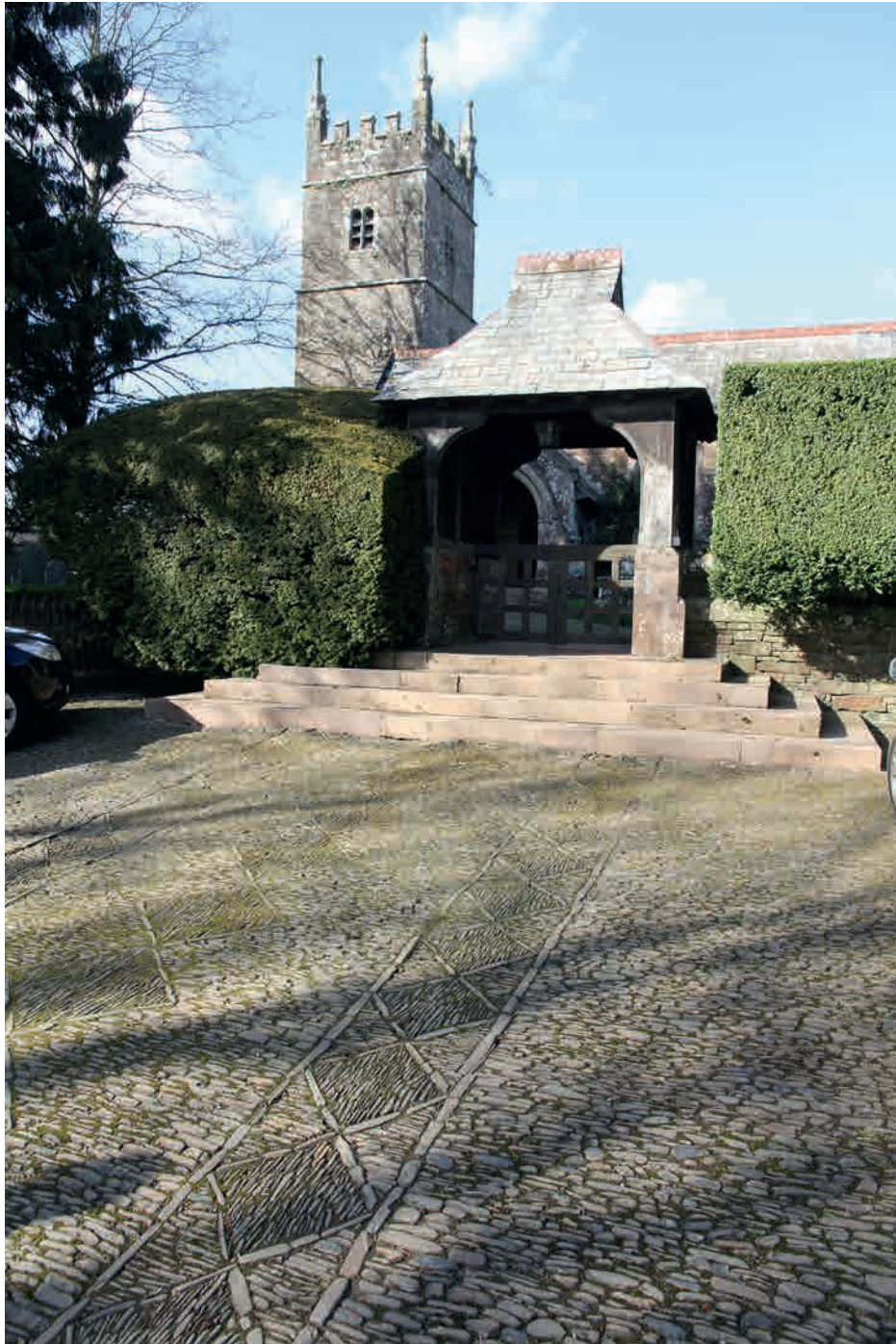
Fig.8. The court that lies outside the boundary walls of the church of St James the Less, Huish, rebuilt (apart from the tower) by G E Street, is part of a sophisticated Victorian and perhaps Edwardian church landscape. This provided, inside the churchyard, several patterned cobbled paths leading to the church porch, vestry and rectory, but also provided a patterned cobbled court between the lychgate and road beyond which is a World War 1 memorial. The court may have had a ceremonial function as well as providing an area for parking vehicles.
