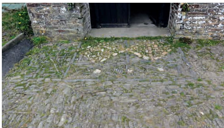
Fig.49, High Bickington, St Mary. A rectangular cobbled 'doormat' incorporating lozenges and white quartzite cobbles. This mat is unusually elaborate. Semi-circular patterns are also often found.
