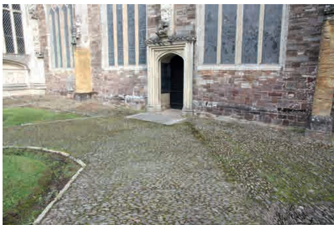
Fig.128-130. Tiverton, St Peter. Clockwise from top left. The lychgate; a view across the S side of the churchyard, looking NE; one of the cobbled paths (forked) in the early 20th century; the large cobbled apron where paths meet outside the SE doorway.
