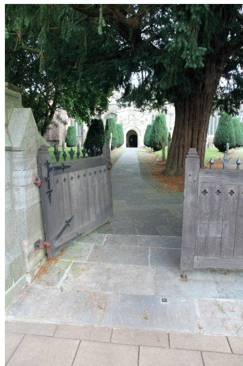
Fig.164. A path of riven Pennant stone driven through cobbles at Tiverton St Peter. It was possible to preserve white quartzite initials in one of the cobbled borders. Level access from the footway outside the church and into the S porch made this a less complicated amendment for improved access than might be the case on another site.
