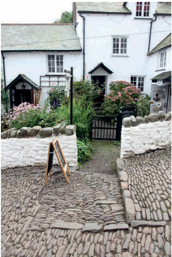
Fig.26. Carboniferous sandstone cobbles illustrating something of their variety of shape, colour and size. Clockwise from top.
