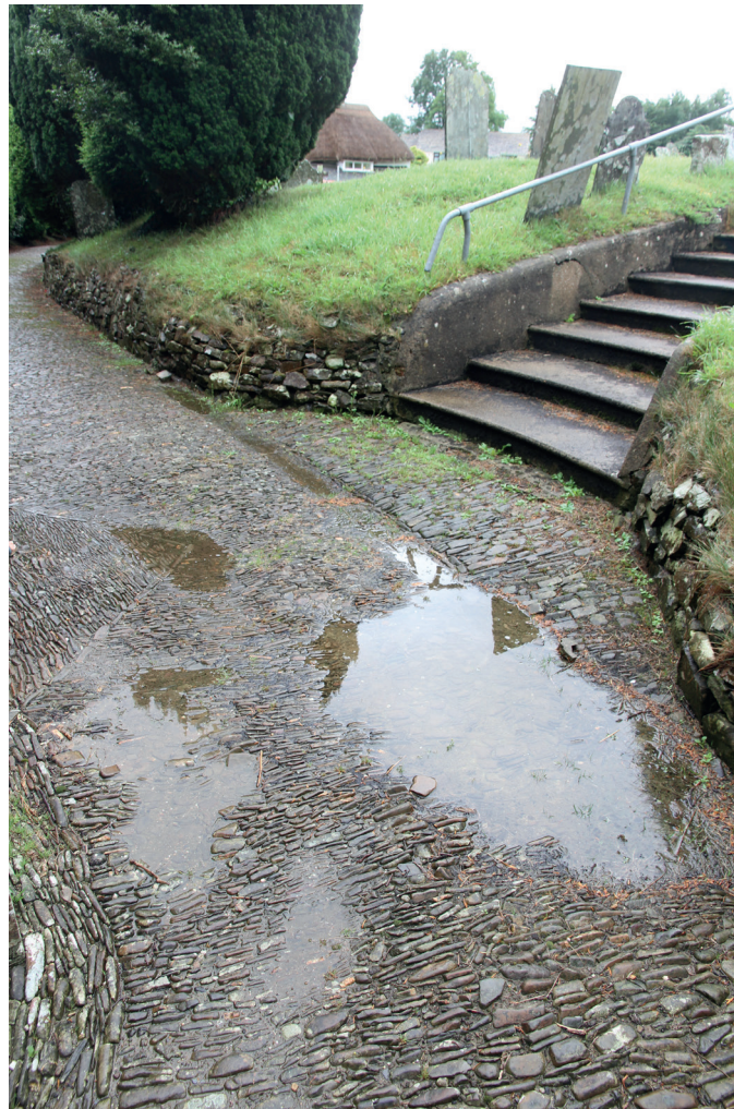
Fig.70. An uncommon example of a group of water-filled sinkings after rainfall at Petrockstow.
