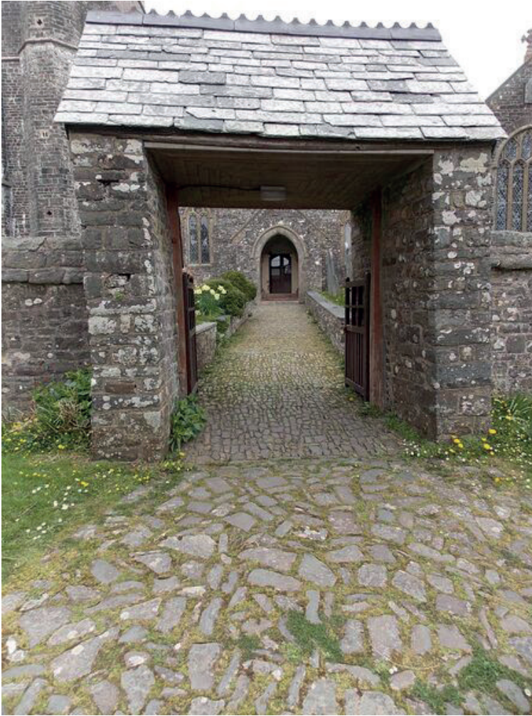
Fig.41. West Woolfardisworthy, Holy Trinity. Smaller cobbles used inside the churchyard boundary compared with large, random-laid cobbles outside reinforce the special character of the churchyard as an enclosed space and the setting of the church building.
