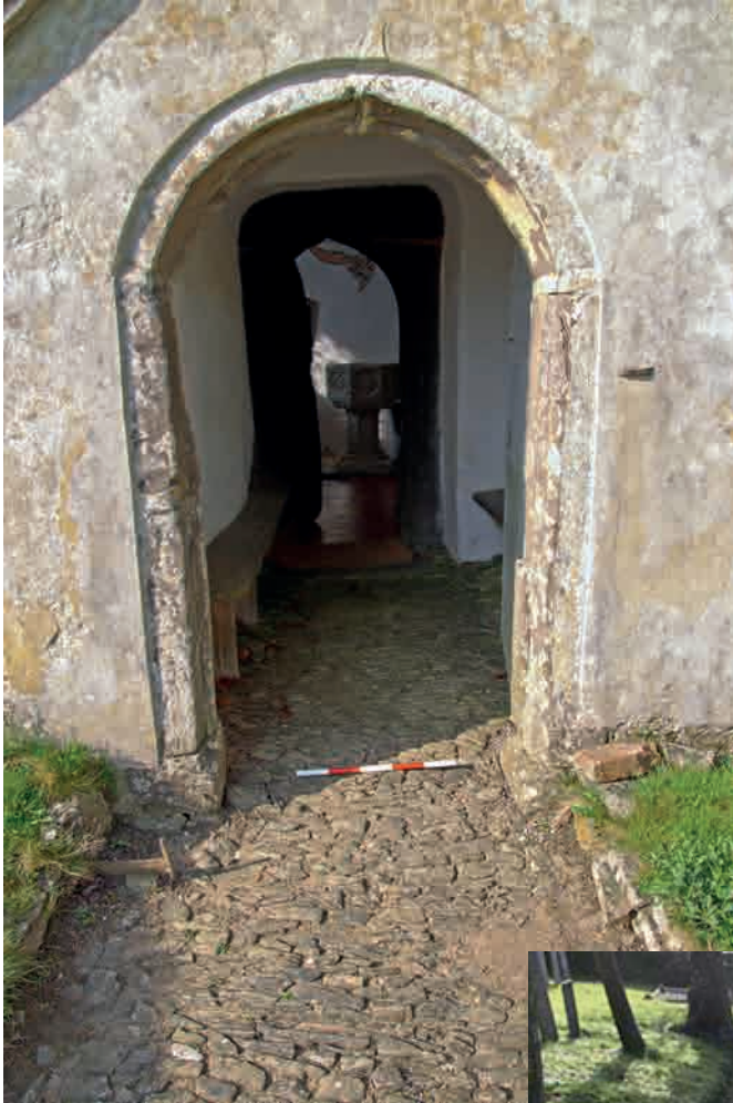
Fig.3. The path to the Church of St Peter, Satterleigh uses large, rustic cobbles similar to those found in farmyards. The cobbled surface is continued into the south porch.
