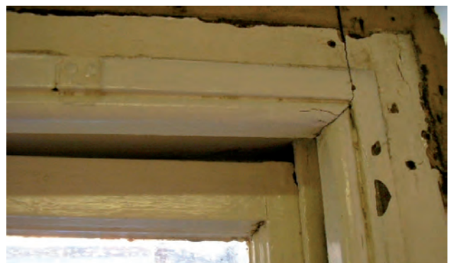
Top: Exterior view of test window as received; left detail showing the decayed sill; right detail showing the gap between the upper sash and the frame
