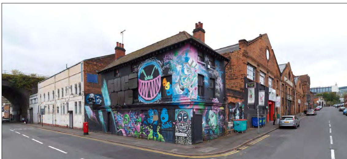
Figure 83: The former Spotted Dog pub, seen from the north-east (DP219838)
