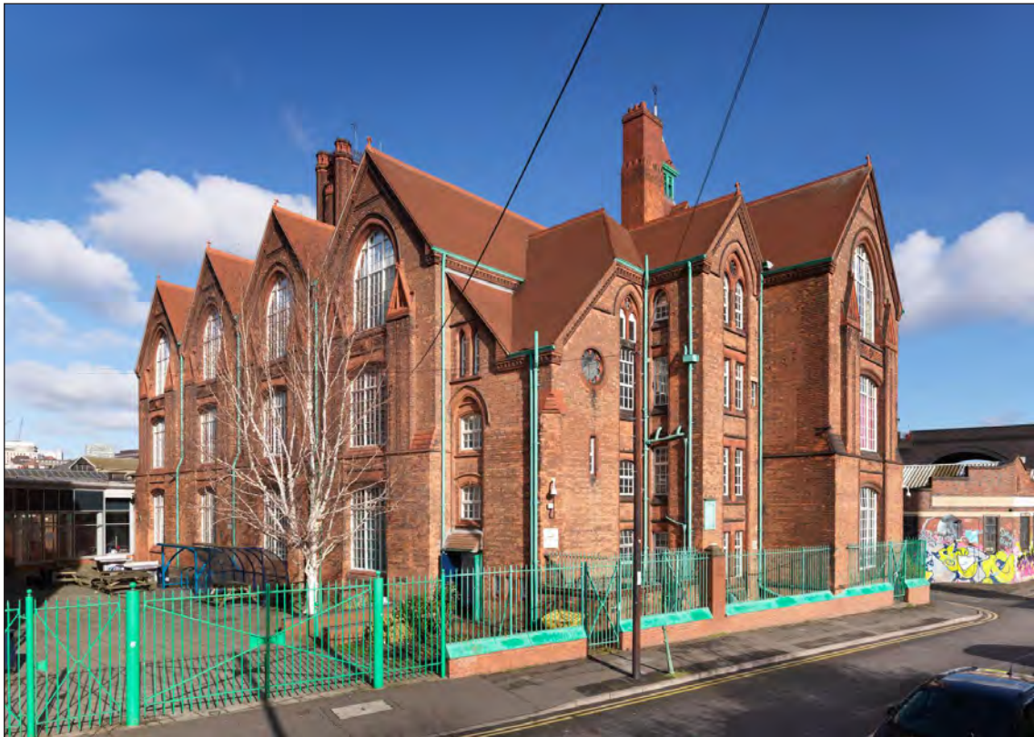
Figure 11: The former board school by Martin and Chamberlain of 1891 on Floodgate Street (DP195928)
