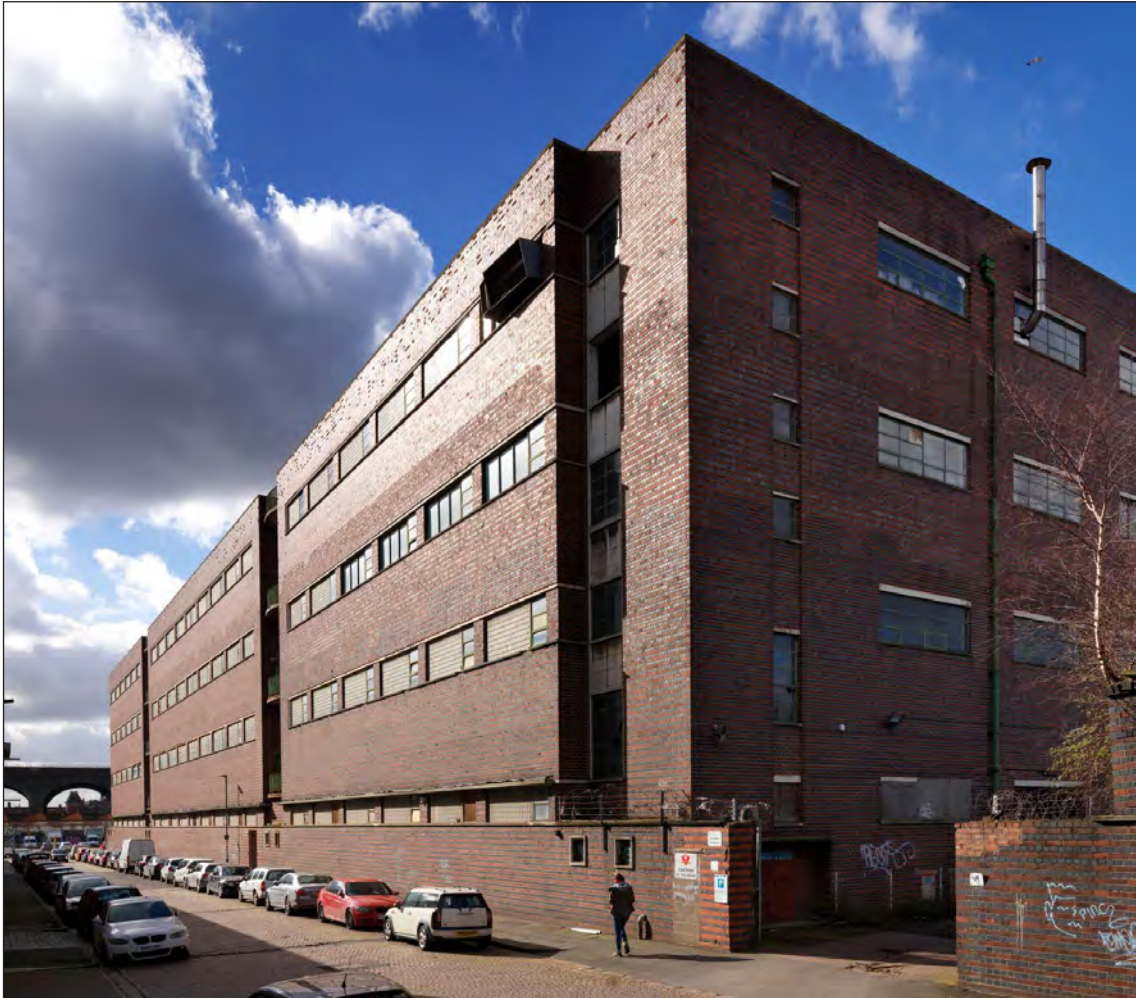
Figure 42: The building of c 1954 from Pickford Street in 2017, looking south-west (DP195875)
