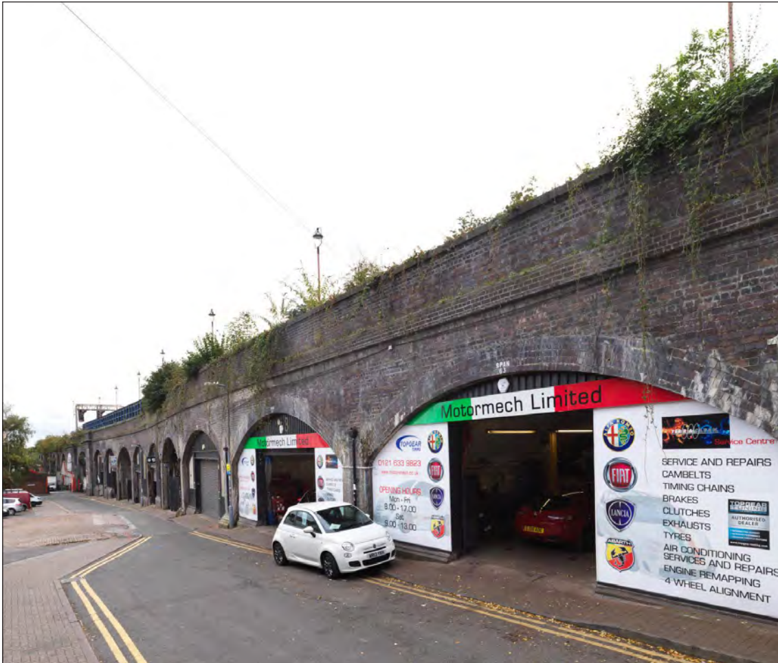
Figure 82: Shaw's Passage and the viaduct arches, seen from Park Street (DP219826)
