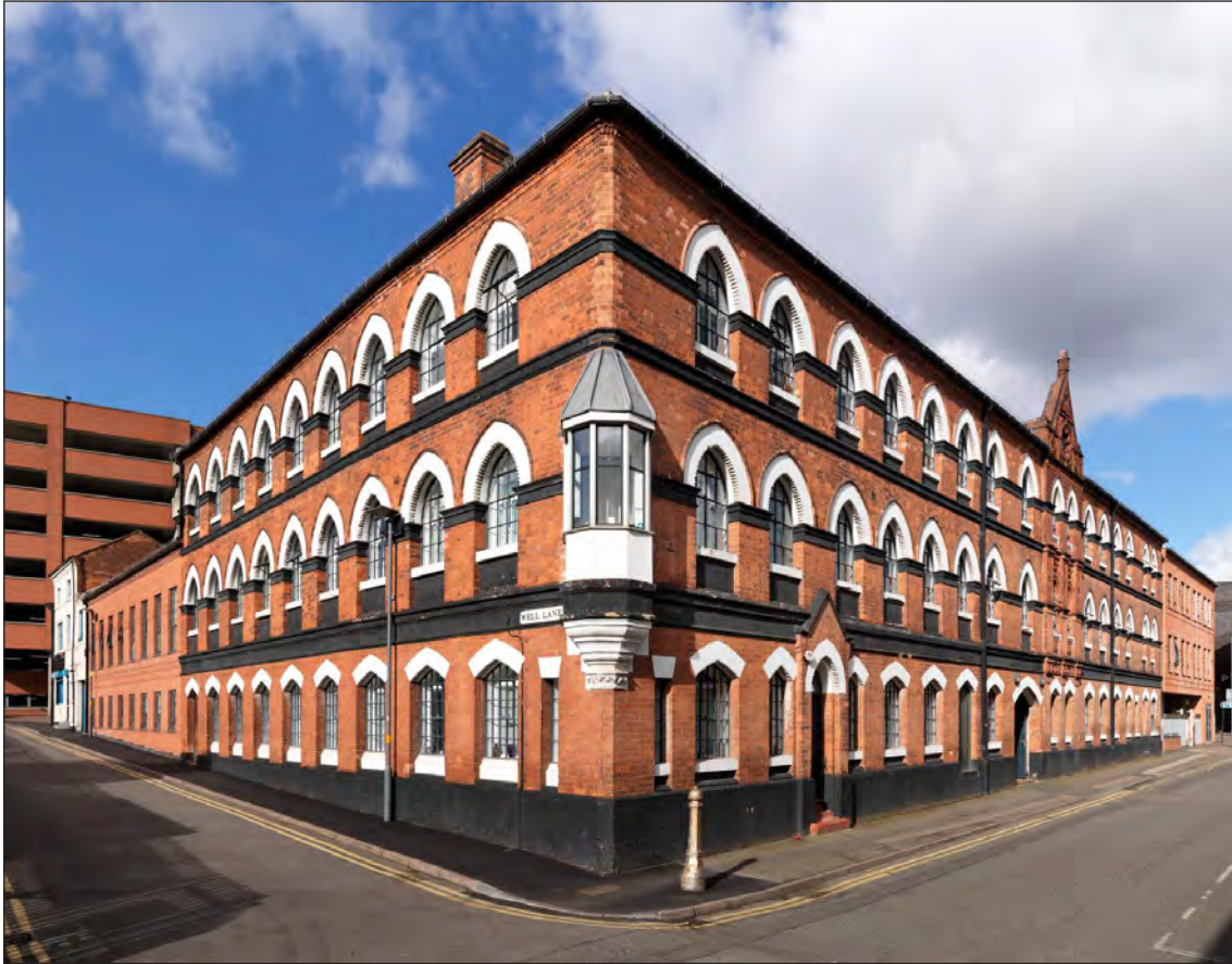
Figure 12: The former umbrella factory at 78 Allison Street, built in 1872 for Corder & Turley, manufacturer of umbrella ribs (DP195878)
