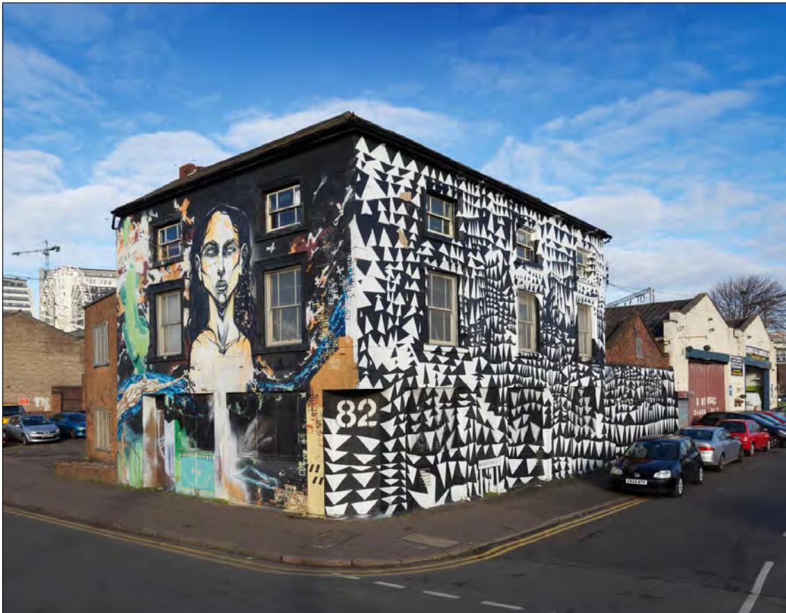
Figure 78: 82 Fazeley Street, the former Royal Oak pub, seen from the south-east (DP219852)
