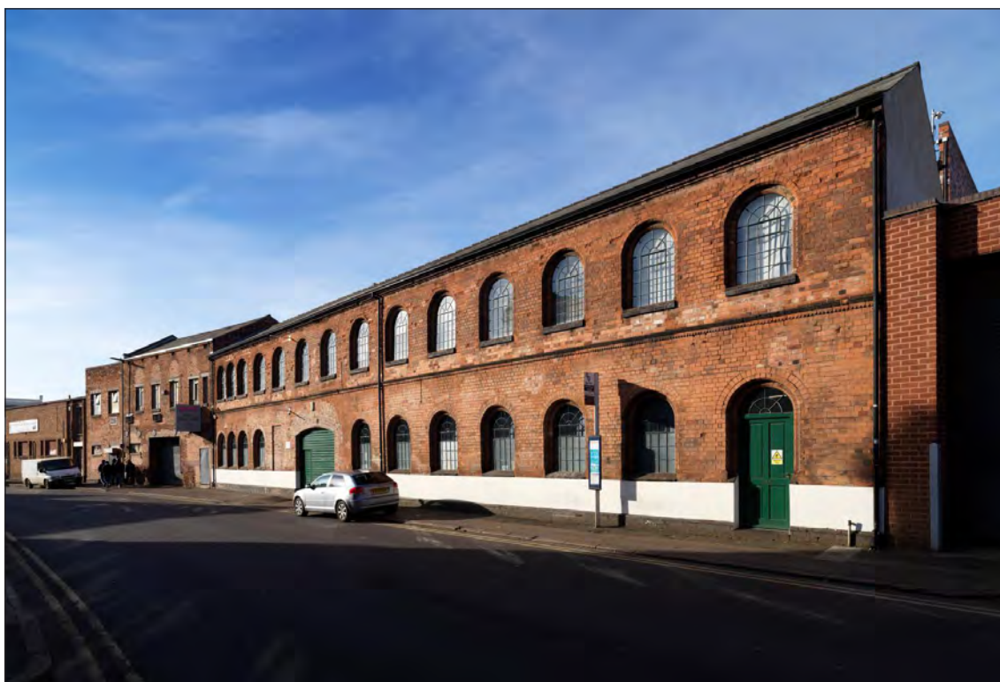
Figure 17: The Arch, Heath Mill Lane (DP219875)
