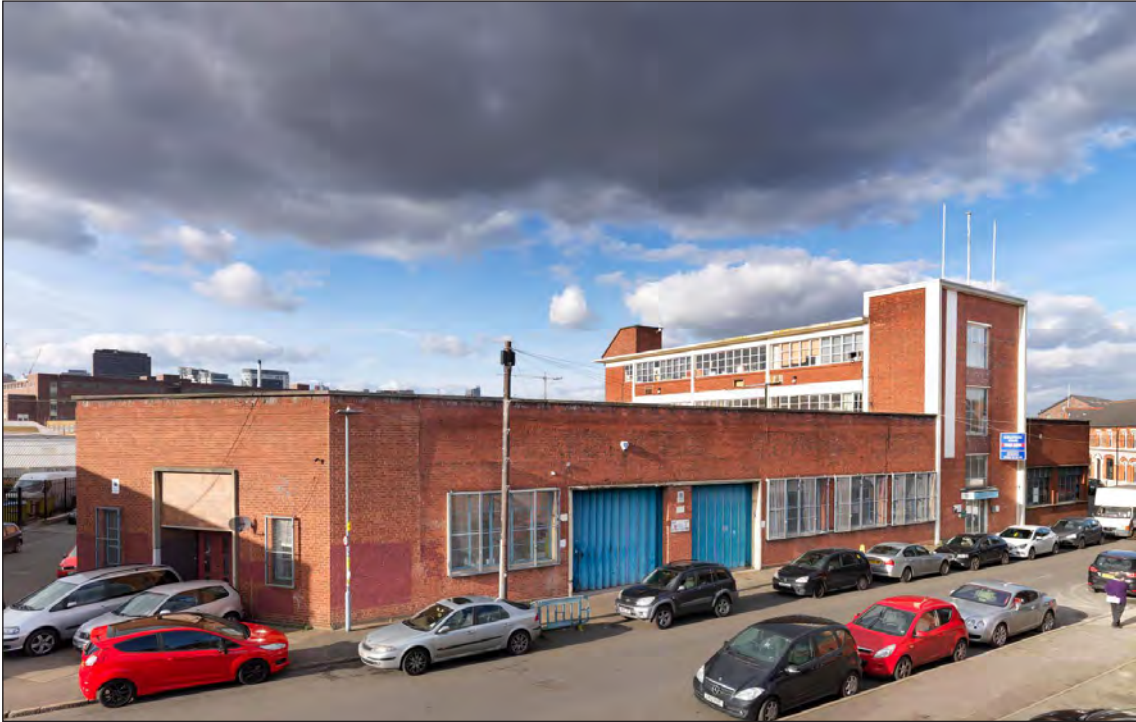
Figure 51: 90 Floodgate Street, seen from the south-west along Floodgate Street, in 2017 (DP195896)
