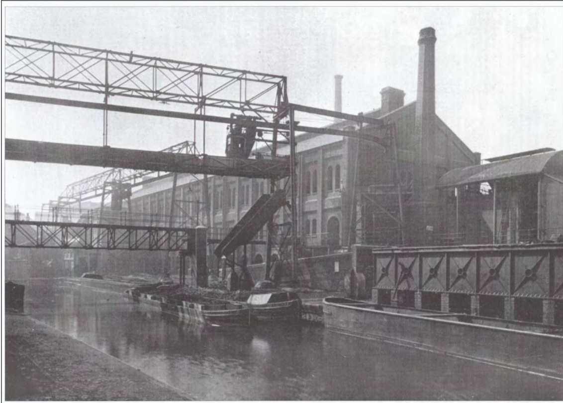
Figure 65: Undated photo from the north-east, showing the telfers and the coke chute about to load a canal boat below (Horne 2009, 2)
