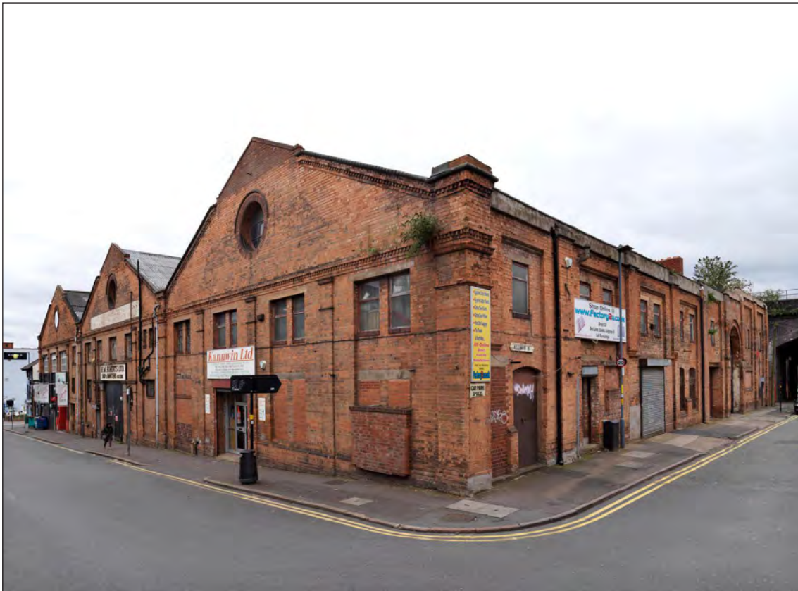
Figure 77: The former pig market of 1891-2, seen from the north-west (DP219836)
