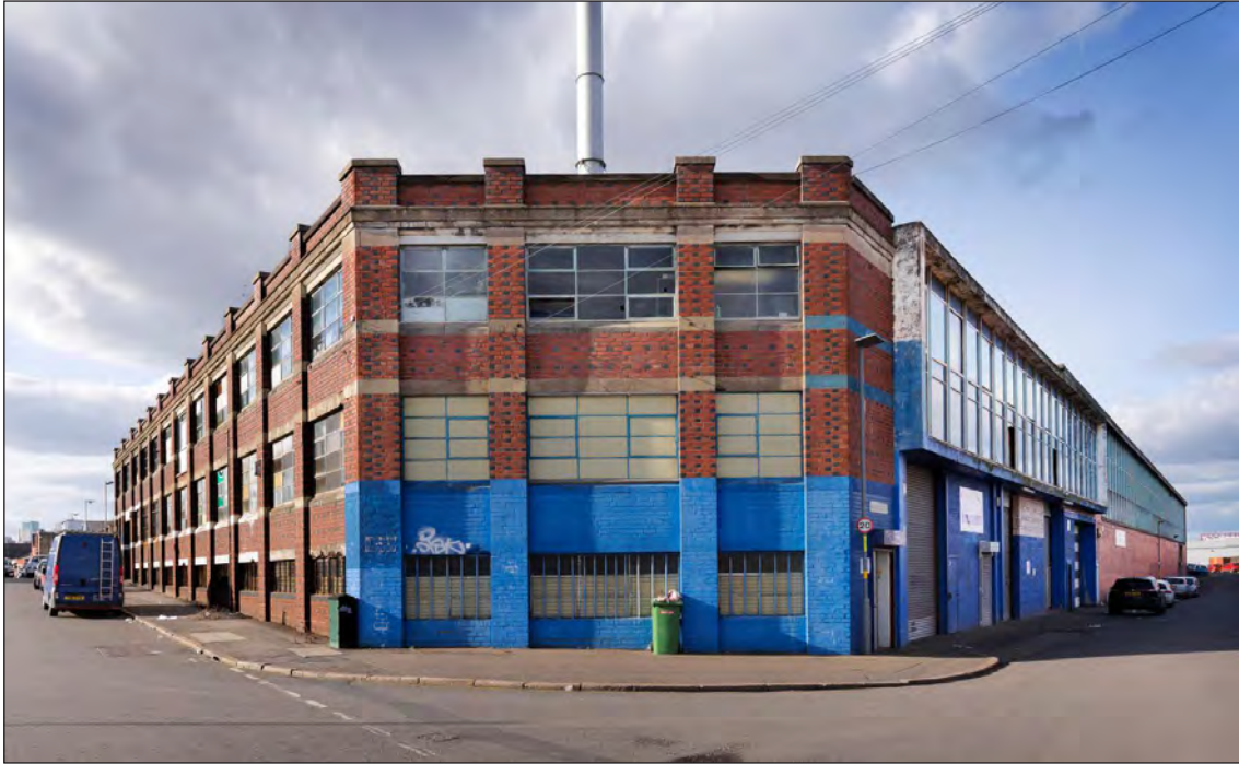
Figure 52: 60-69 Glover Street (DP195885)
