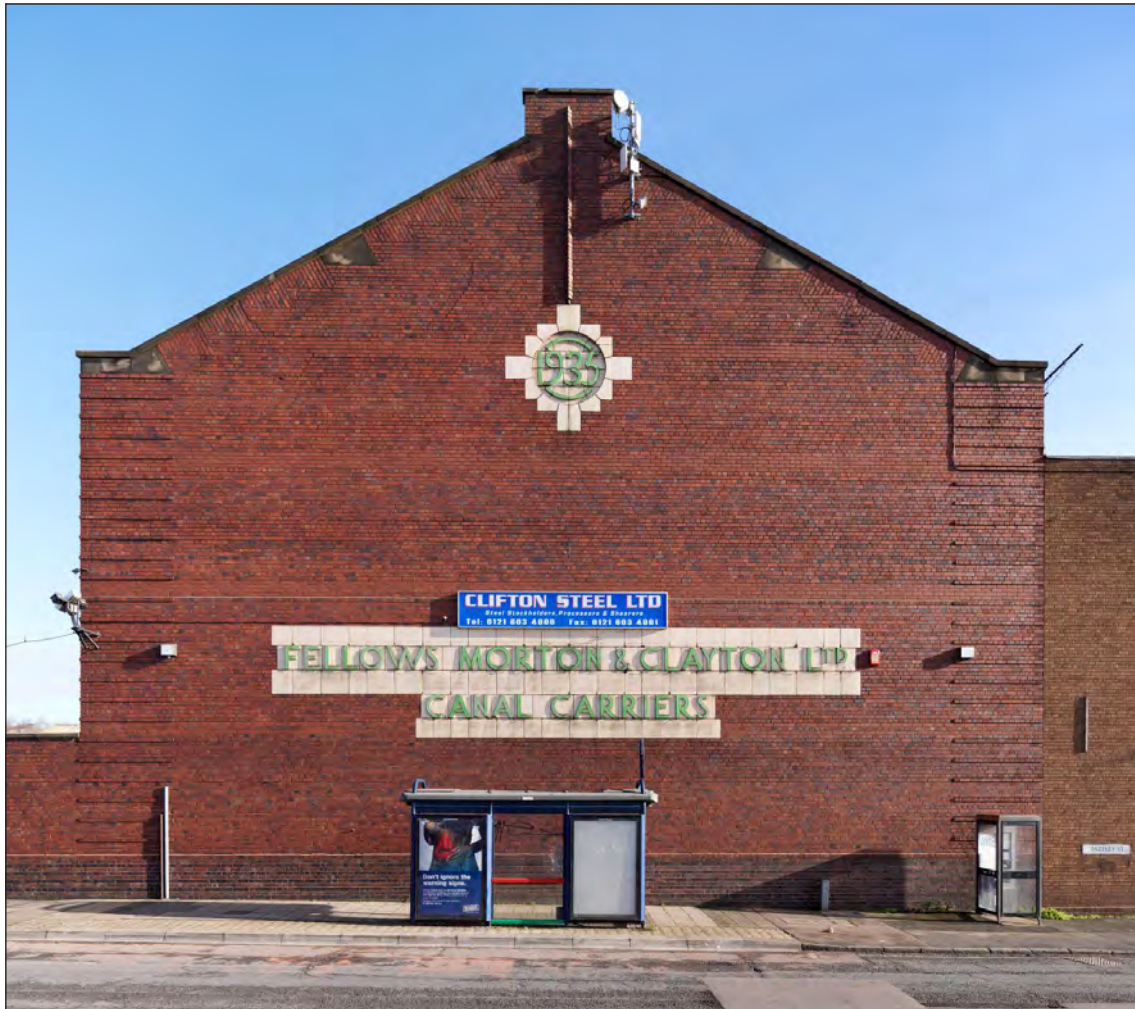
Figure 43: Street elevation to Fazeley Street (DP195911)
