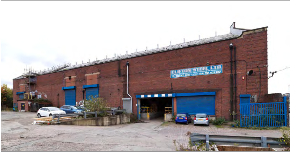
Figure 44: The warehouse, seen from the south-west (DP219841)
