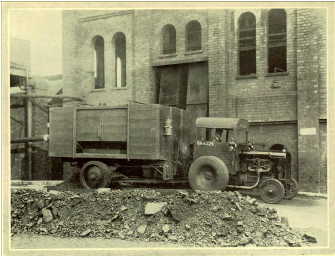
Figure 64: Photo of c 1928 showing a Fordson tractor delivering coal to the hopper at the north-west corner of the retort house (National Grid Gas Archive, G11_BRM_30029, City of Birmingham Gas Department, Adderley Street Works, February 1928, 4)
