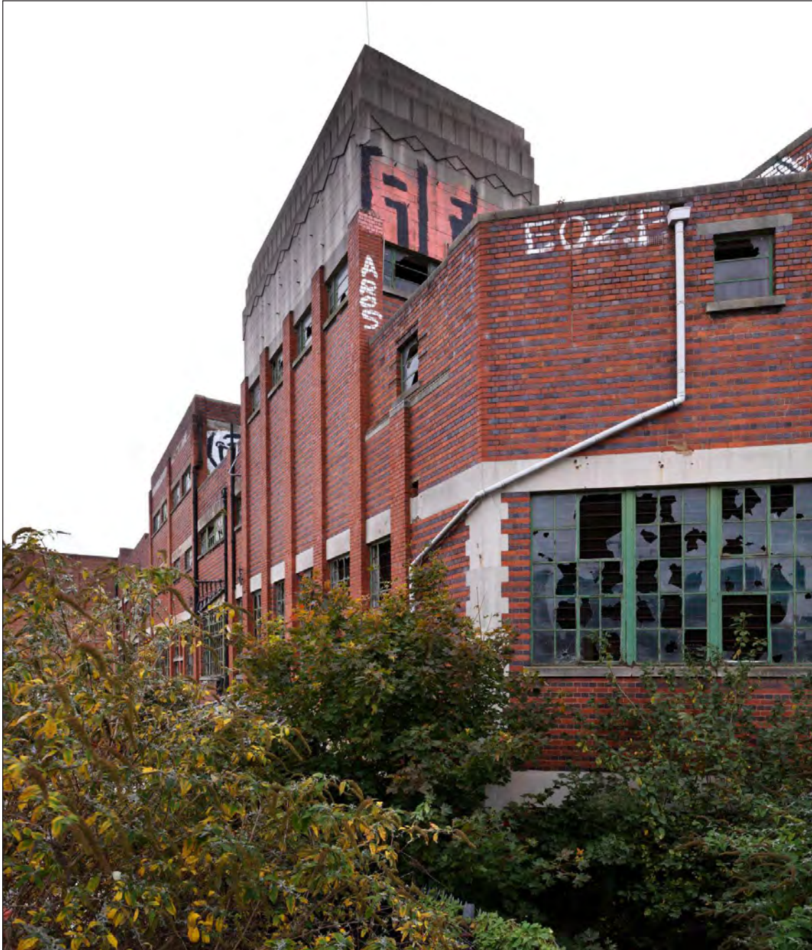
Figure 33: The lift tower of the 1932 extension, seen from Benacre Drive (DP219840)
