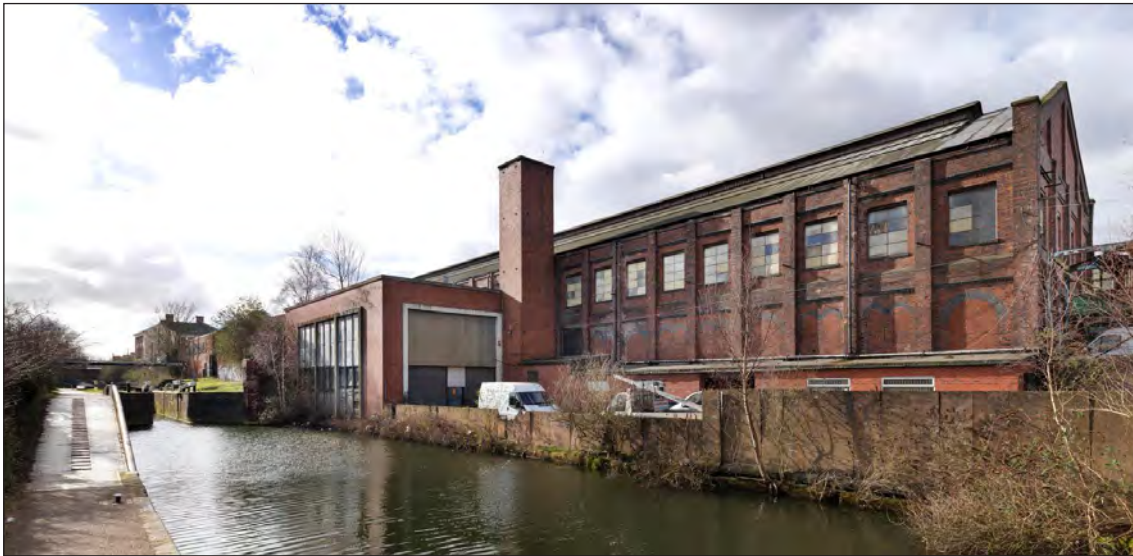
Figure 54: The retort house from the north-east (DP195945)
