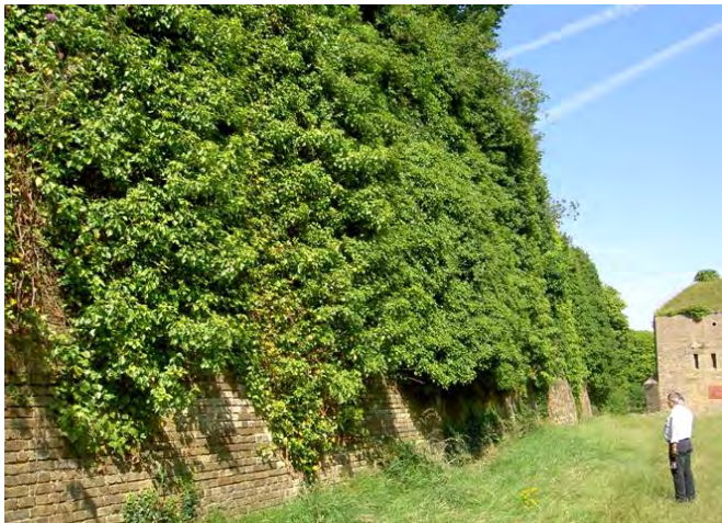
Condition surveys – are they possible with ivy cover?
