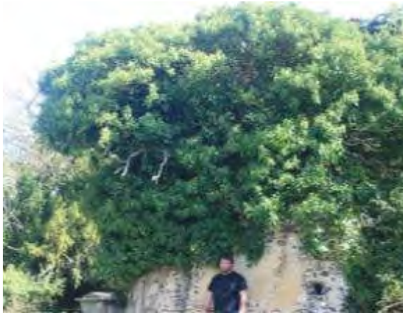
Assessing the condition of structures is difficult
