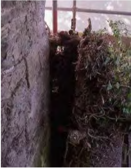
Figure 1.1 Wigmore Castle – decades old ivy being removed from unharmed walls.
