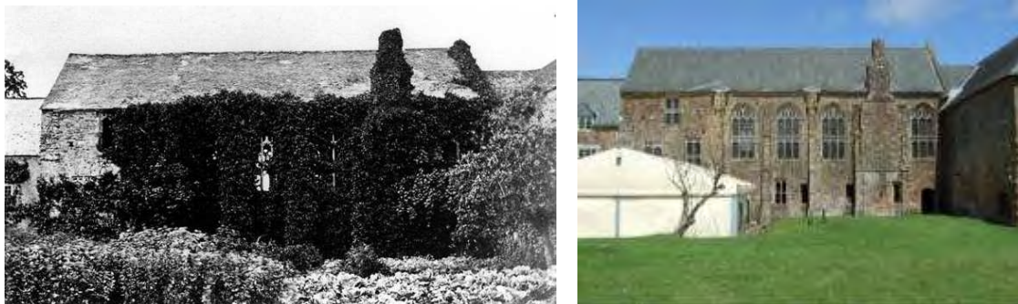
Figure 2.1 Cleeve Abbey refectory with ivy cover (left) and after ivy removal.
