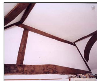
Figure 96. Roof truss and windbraces in 'The Keep'. (AA046067)
