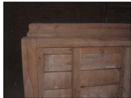
Figure 174. Moulded wooden rim applied to top of water tank. (DP004025)
