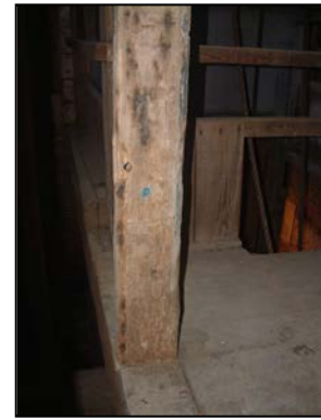
Figure 160. Detail of reused medieval timber on first floor. (DP004019)
