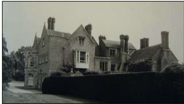
Figure 200. Rear elevation, photographed in 1982. Note the wooden oriel window replacing the stone surround shown in Figure 199. (DP004050) (Reproduced by permission of The National Trust, Hughenden Manor)
