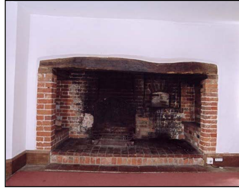
Figure 192. Fireplace in living room (east). (AA046024)
