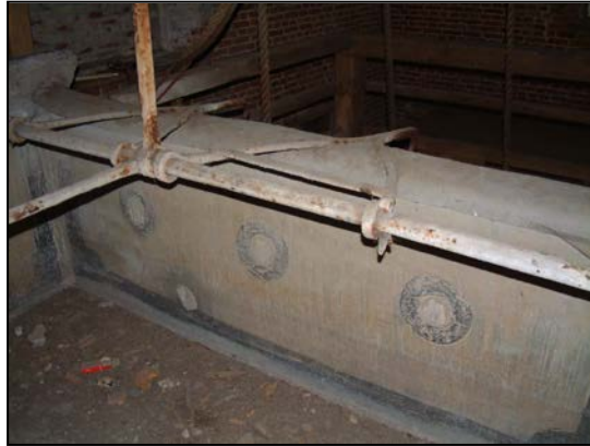
Figure 173. Interior of water tank, showing detail of leadwork. (DP004027)
