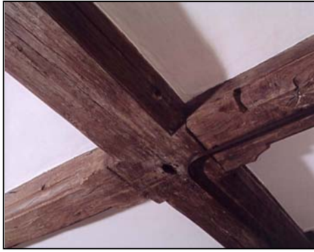
Figure 204. Ovolo-moulded beams on the ground floor of the south-west wing. (AA046071)
