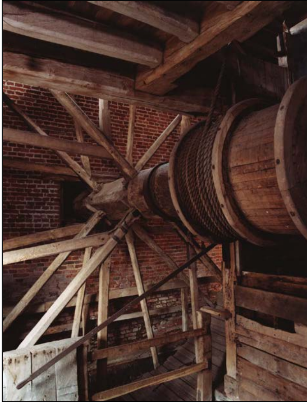
Figure 176. Winding drum and ropes. (AA047437)
