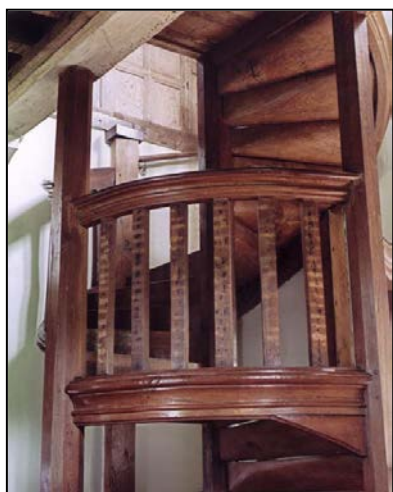
Figure 128. Spiral stair on the ground floor of the 'Cromwellian Stables'. (AA046046)
