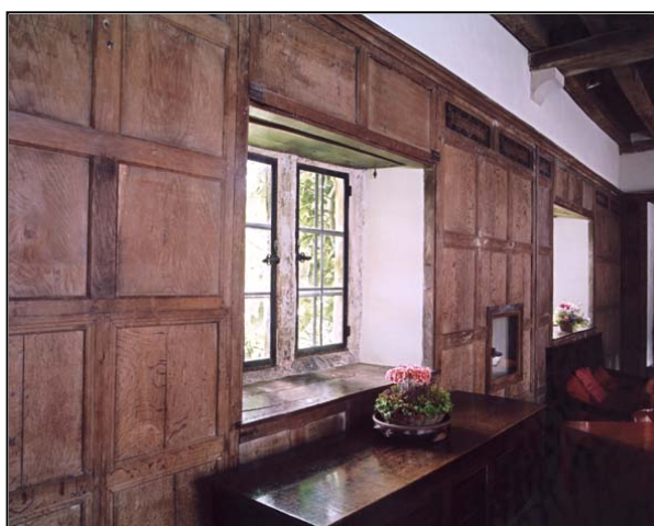
Figure 123. Windows and niche on ground floor of 'Cromwellian Stables'. (AA046038)
