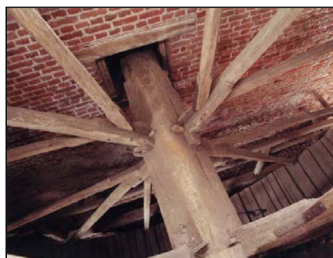
Figure 164. Tread-wheel shaft and wheel spokes, viewed from first floor. (AA047419)
