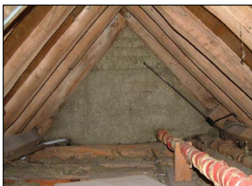
Figure 108. Detail of the roof structure above purlin height. (DP004068)
