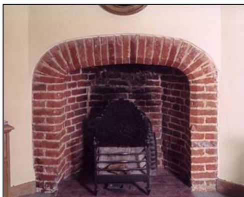
Figure 206. Corner fireplace on first floor of south-west wing. (AA046072)
