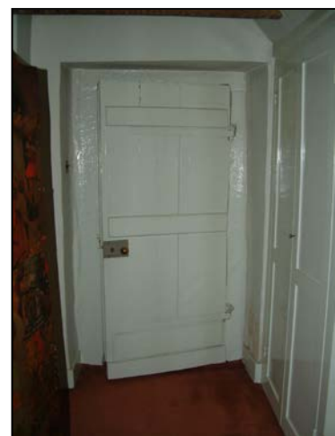
Figure 202. Door to attic bedroom. (DP004058)
