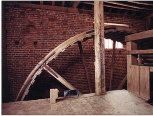
Figure 159. Reused timber and part of tread wheel, first floor. (AA047428)
