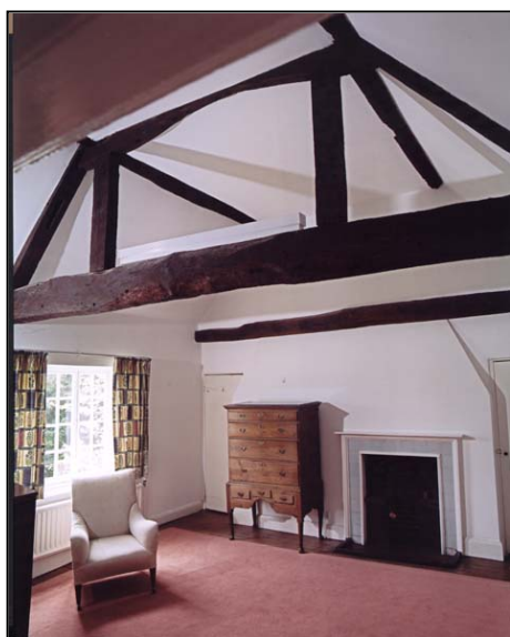
Figure 189. Roof truss visible from western bedroom, front range. (AA046029)
