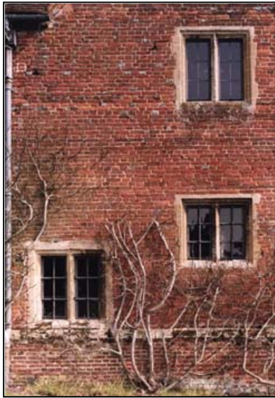
Figure 132. Windows in west wall. (AA045579)
