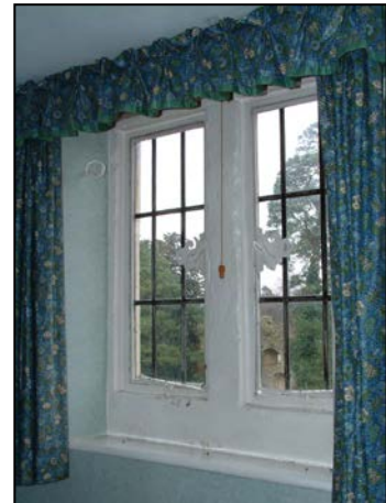
Figure 107. Attic window on the south front. (DP004053)
