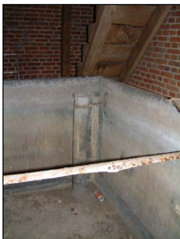
Figure 175. Overflow in north-east corner of water tank. (DP004028)
