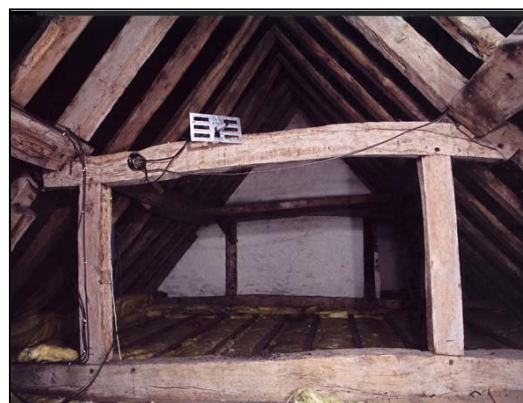
Figure 190. Roof truss over eastern bedroom, front range. (AA046032)
