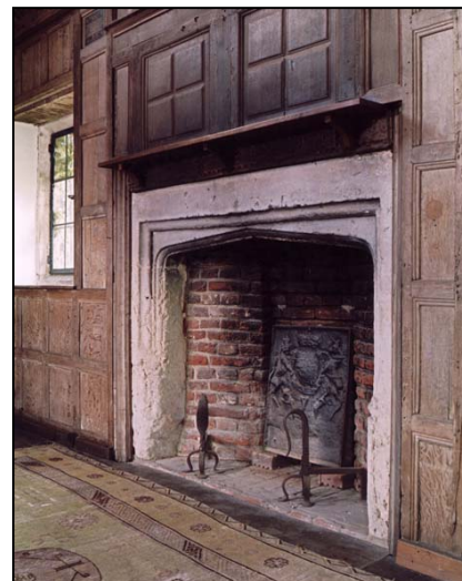
Figure 127. First-floor fireplace. (AA046048)
