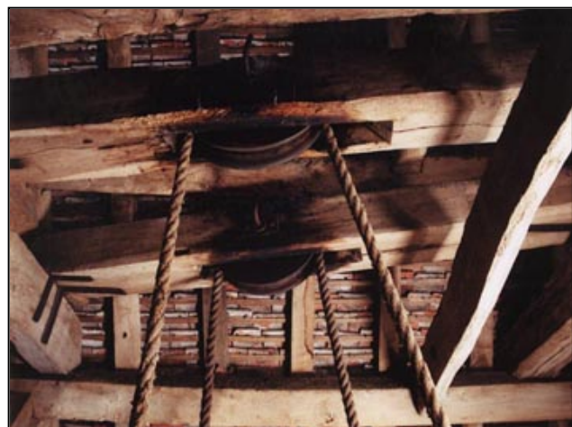
Figure 178. Pulleys in roof. (AA047431)
