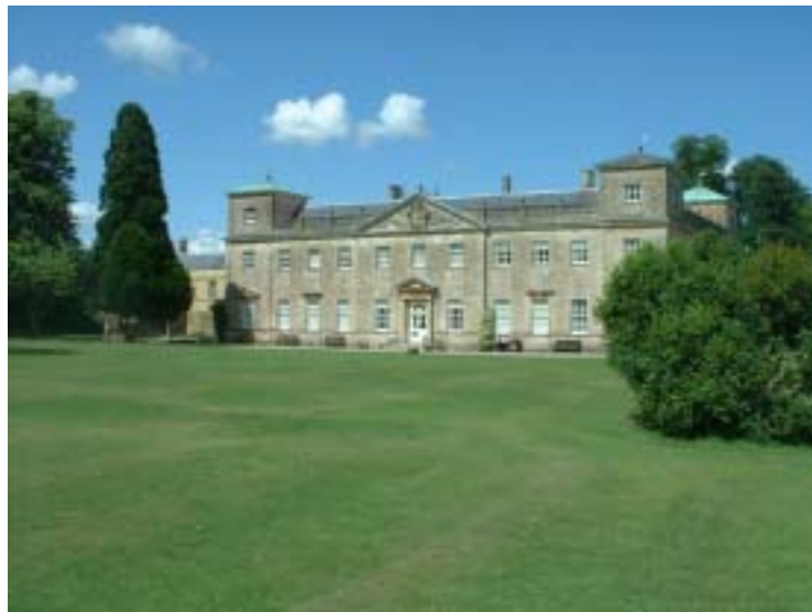
Figure 3 View of Lydiard House
