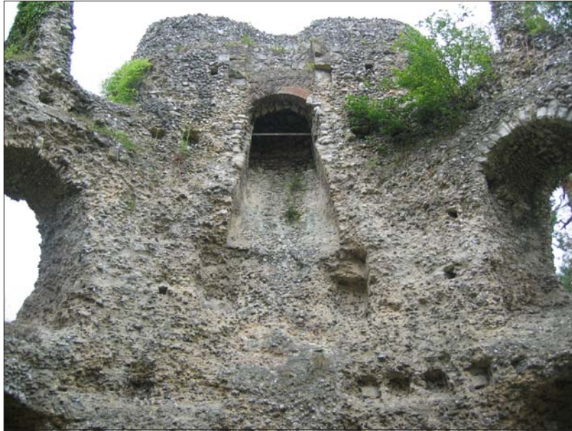
Figure 6. Internal detail of the tower showing chimney
