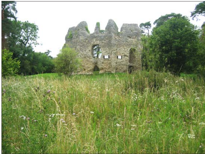
Figure 4. View of tower from the southern platform
