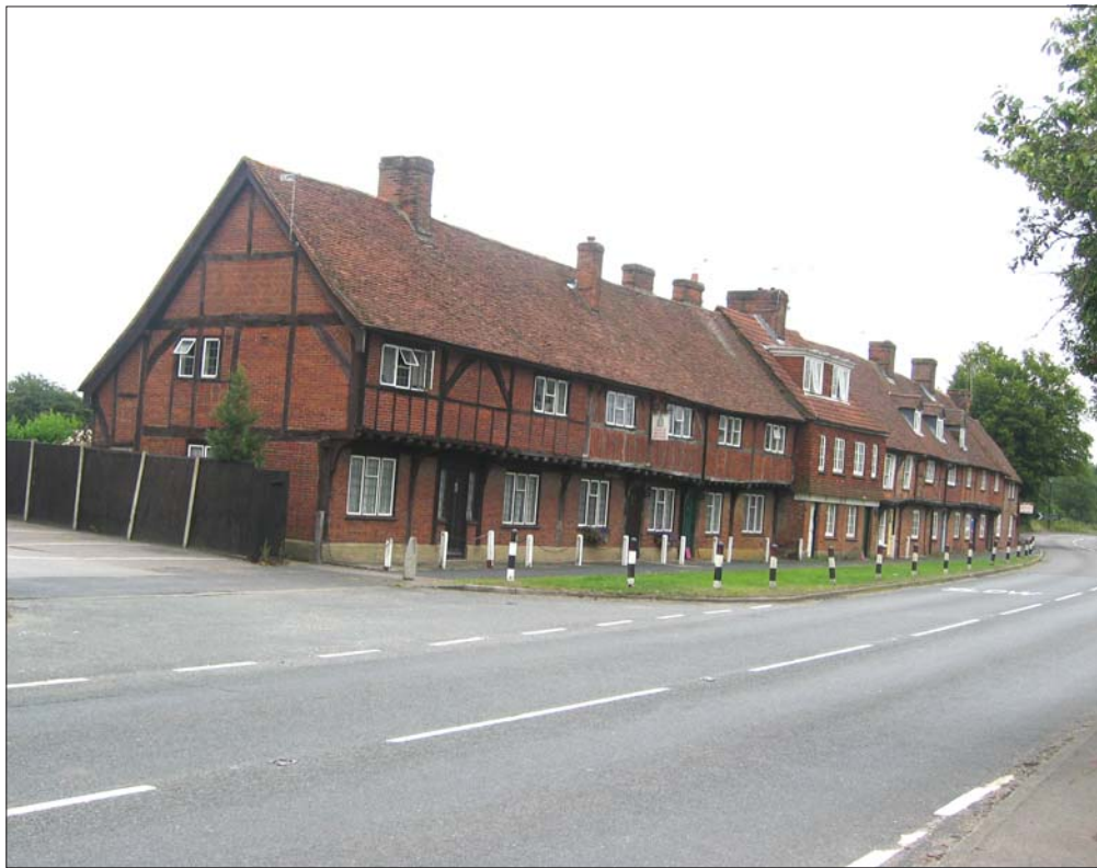
Figure 10. Castle Bridge Cottages form a range of jettied houses facing the street at the northern end of North Warnborough. Nine bays date to 1477/8 while a further seven bays date to 1534/5. Only one bay was heated (Roberts 2003, 238).
