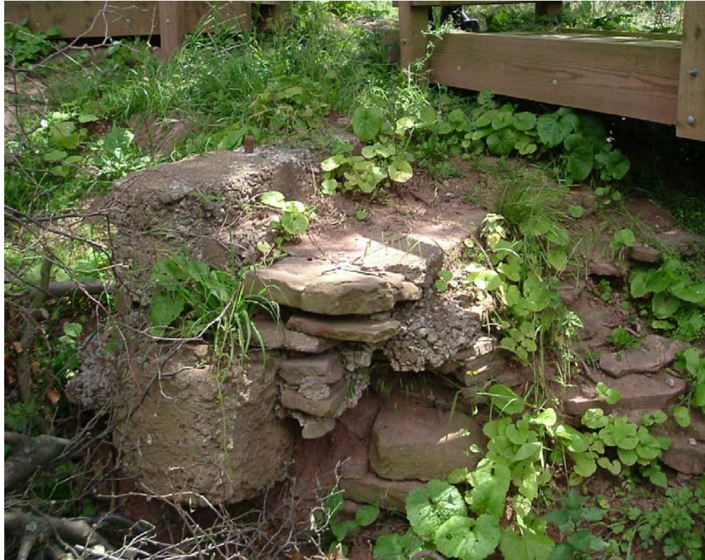
Figure 7: Stonework with concrete repairs at sluice (l).
