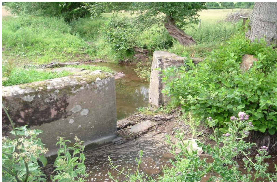
Figure 6: Sluice and weir (1) on the Slough Brook. Rear view.
