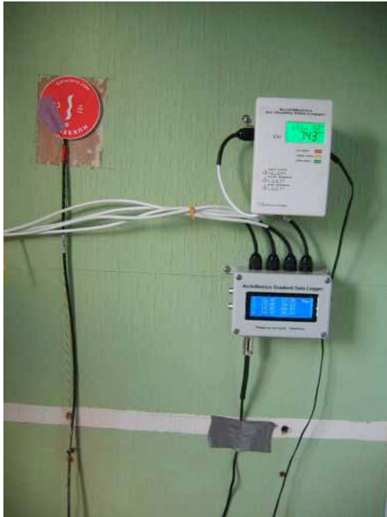
Figure 14. Close up of heat flux sensor and loggers at Abbeyforegate, Shrewsbury 2011.
