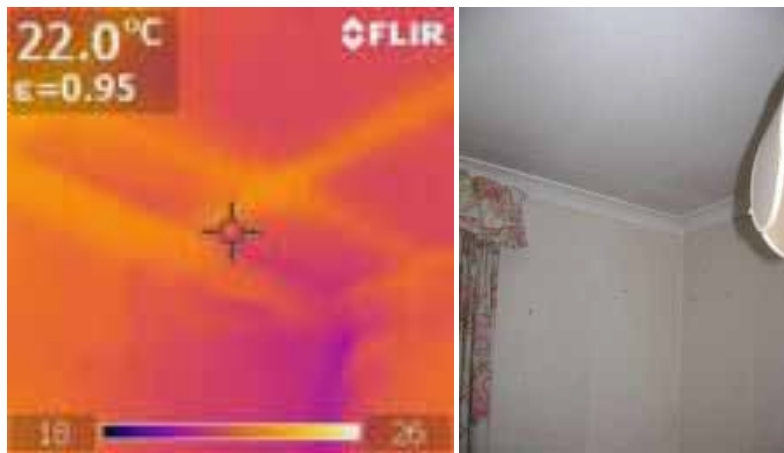
Figure 35. April Cottage, Lower Brailes – first floor bedroom
