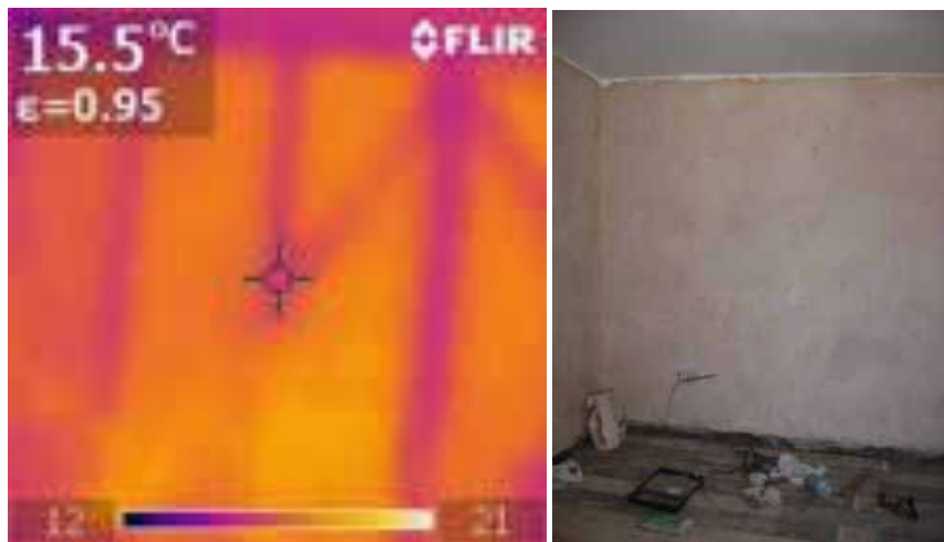
Figure 58. The Old Armoury, Ashburton -second floor: Front SE bedroom – SW wall
