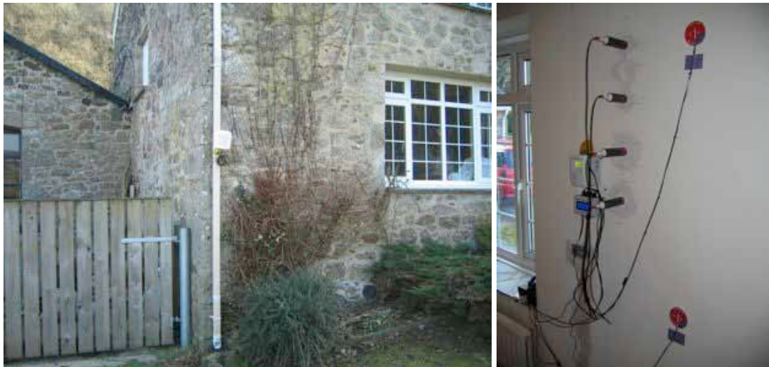
Figure 63. Positions of in situ monitoring equipment at Mill House, Drewsteignton, 2011.
