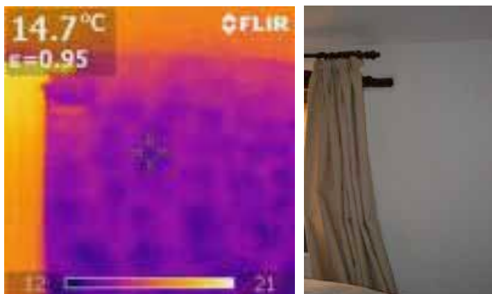
Figure 23. White House Farm, Skipton – Main bedroom, south wall.
