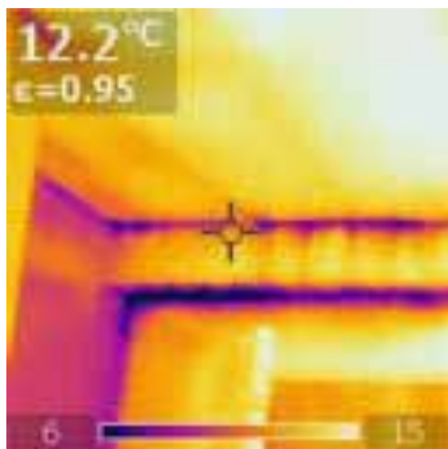
Figure 7. 116 Abbeyforegate, Shrewsbury - first floor south wall.
