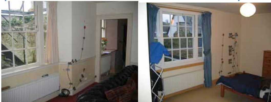
Figure 53. Showing positions of in situ monitoring equipment at The Old Armoury, Ashburton, 2011.
