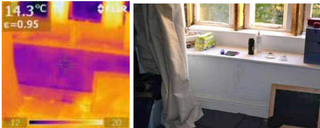
Figure 22. White House Farm, Skipton - main bedroom, south facing window.
