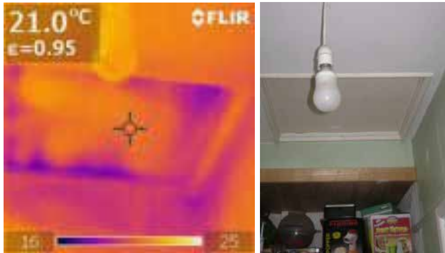
Figure 43. The Firs, Riddlecombe – rear ground floor extension - loft hatch in rear lobby
