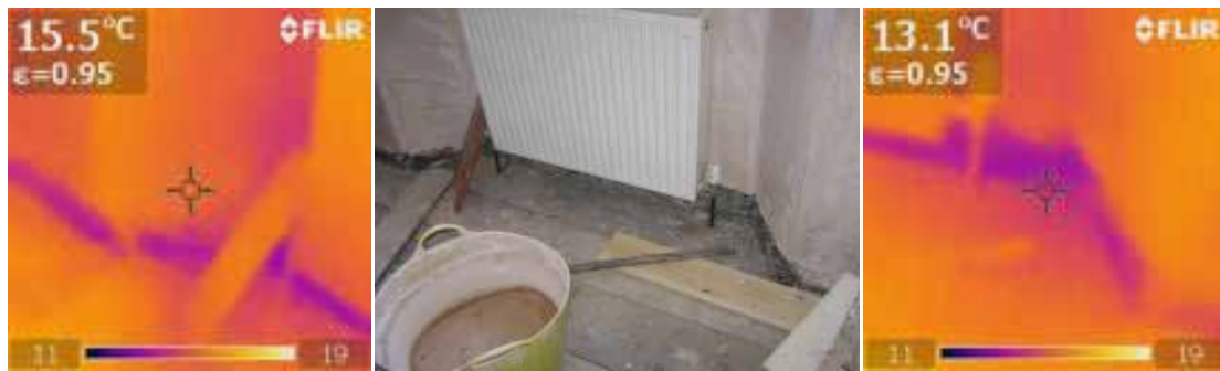
Figure 56. The Old Armoury, Ashburton – second floor: front NW bedroom
