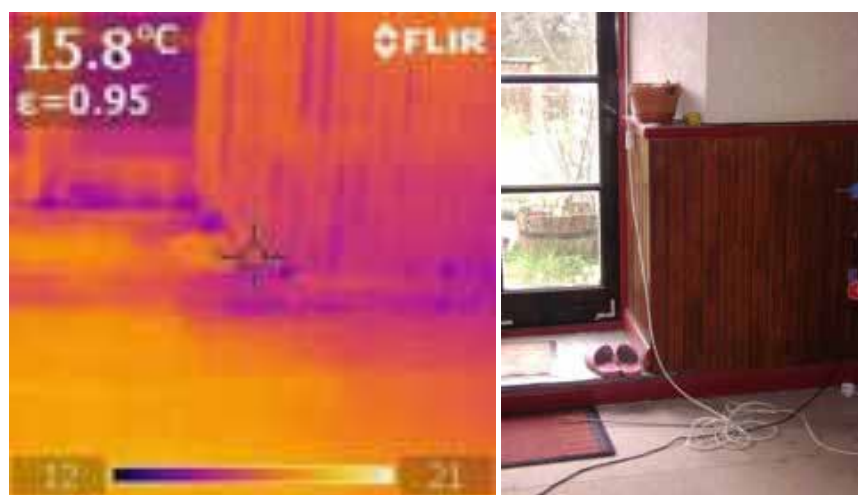
Figure 74. Rock View, Devon Consols - study: external wall
