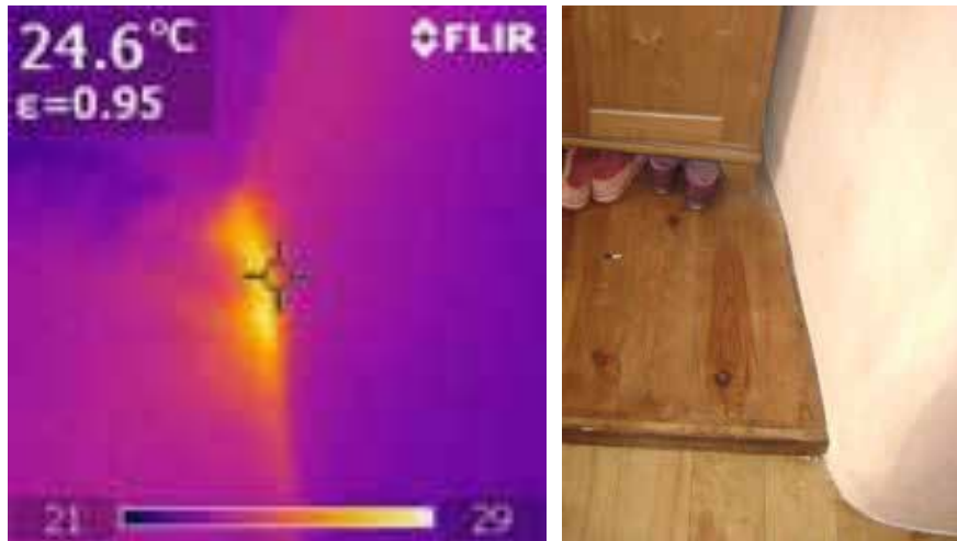
Figure 46. The Firs, Riddlecombe – bedroom 3 - chimney flue gases.
