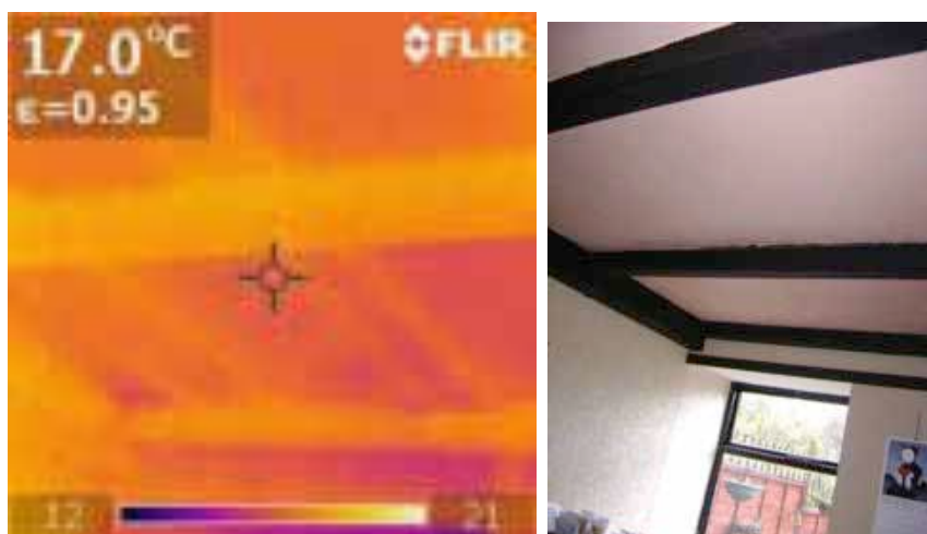
Figure 75. Rock View, Devon Consols - Study ceiling
