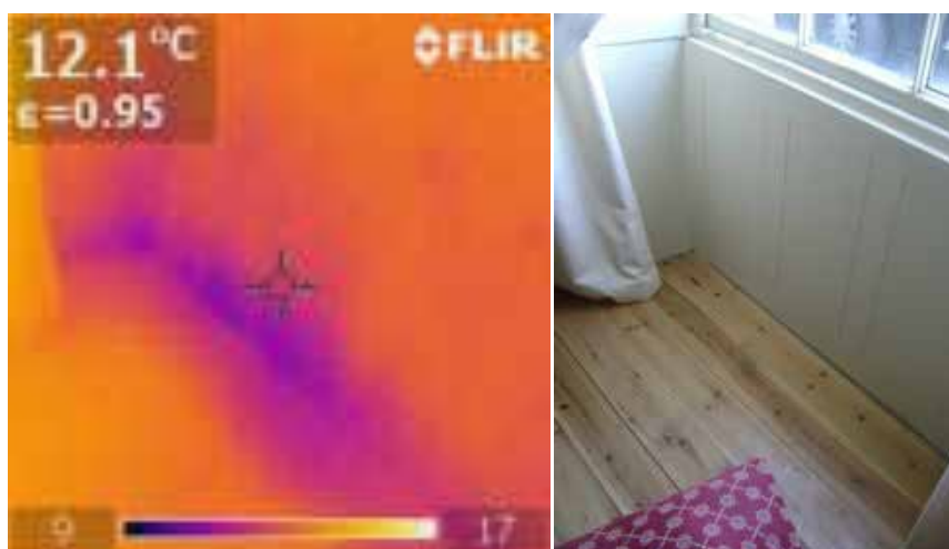
Figure 55. The Old Armoury, Ashburton – ground floor: sitting room
