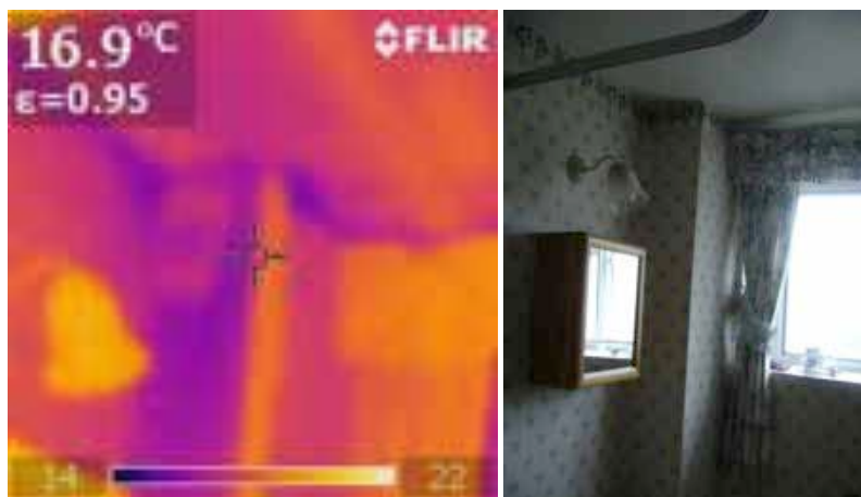
Figure 36. April Cottage, Lower Brailes – bathroom
