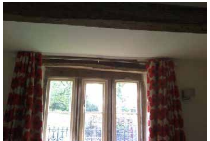
Figure 47. White House Farm, Stirton, Skipton – Thermal bridging on mullion and air ingress around lintel (NB. lower portion of window mullions are subject to solar gain).
