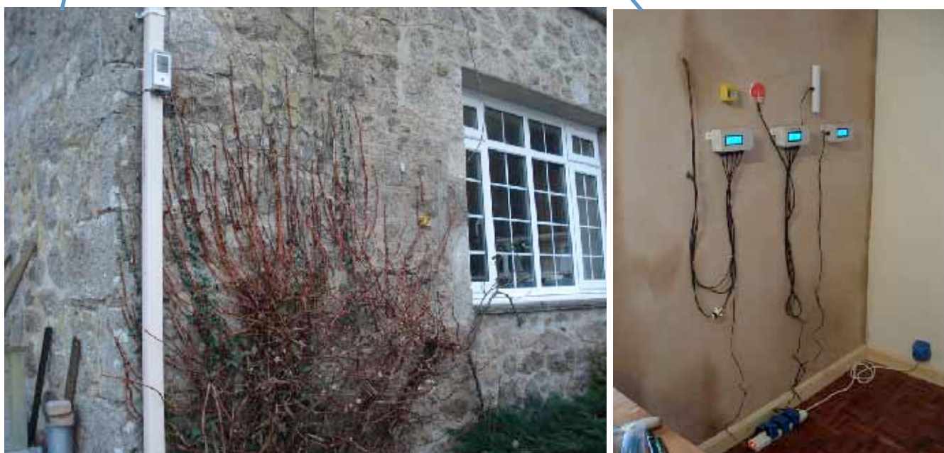
Figure 69. Positions of in situ monitoring equipment at Mill House, Drewsteignton, 2012.
