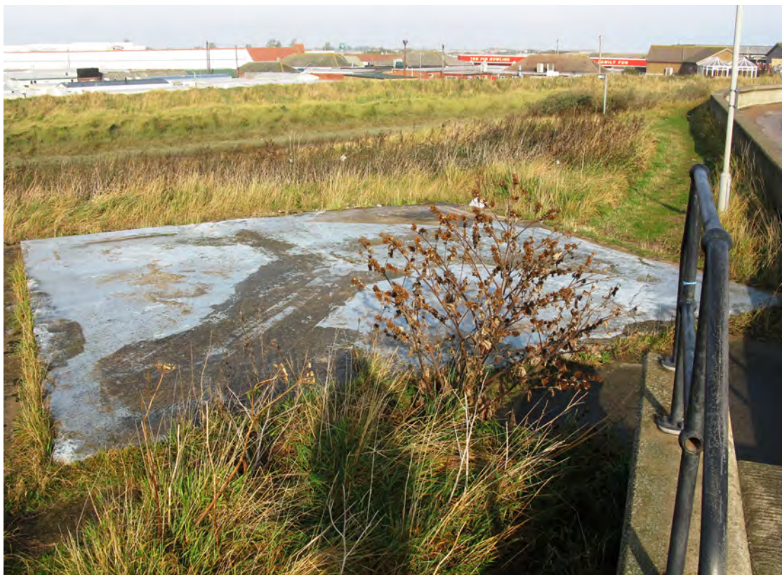
Plate 136 Base of demolished WW2 pillbox IN35, Ingoldmells
