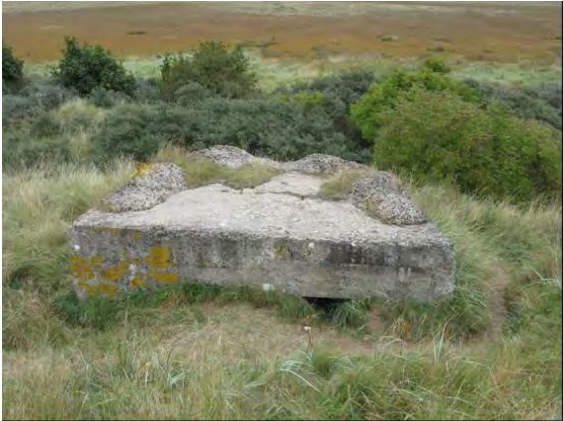
Plate 63 Pillbox SA11 with concrete camouflaging, Saltfleetby
