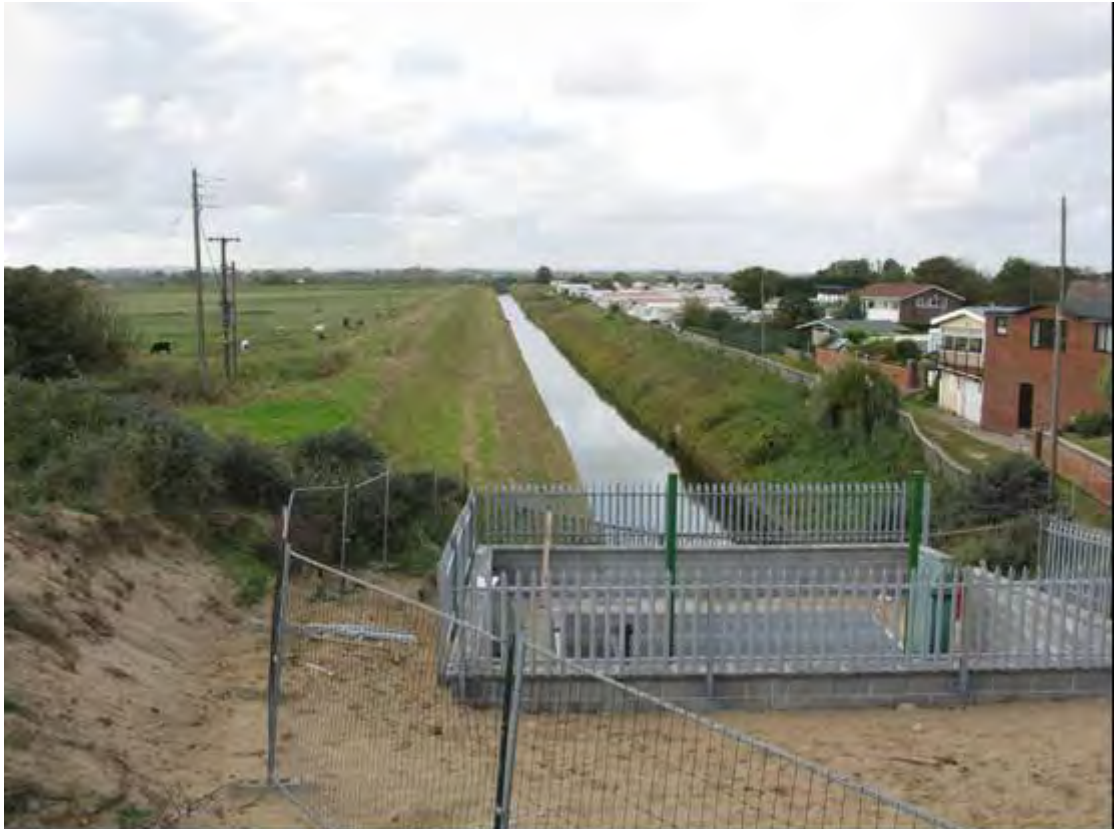
Plate 122 Canalised modern outfall of Anderby Creek
