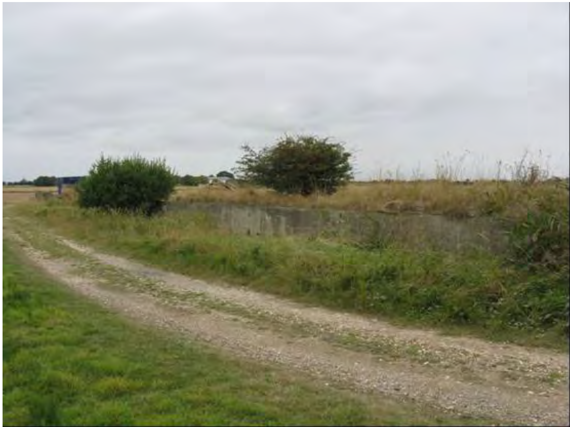
Plate 77 East wall of WW2 enclosure TS9, Theddlethorpe All Saints
