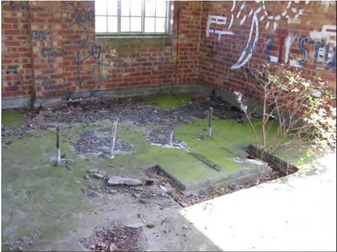
Plate 23 Machine mountings within NS69, North Somercotes
