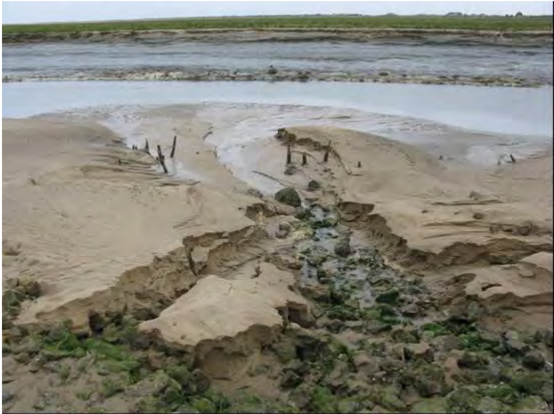
Plate 51 Exposed causeway SH22, Saltfleet Haven
