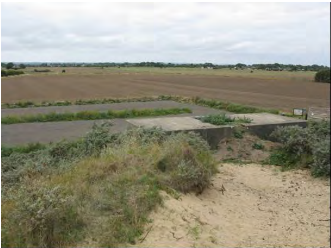
Plate 94 Roof of AA pillbox TH12, Theddlethorpe St Helen
