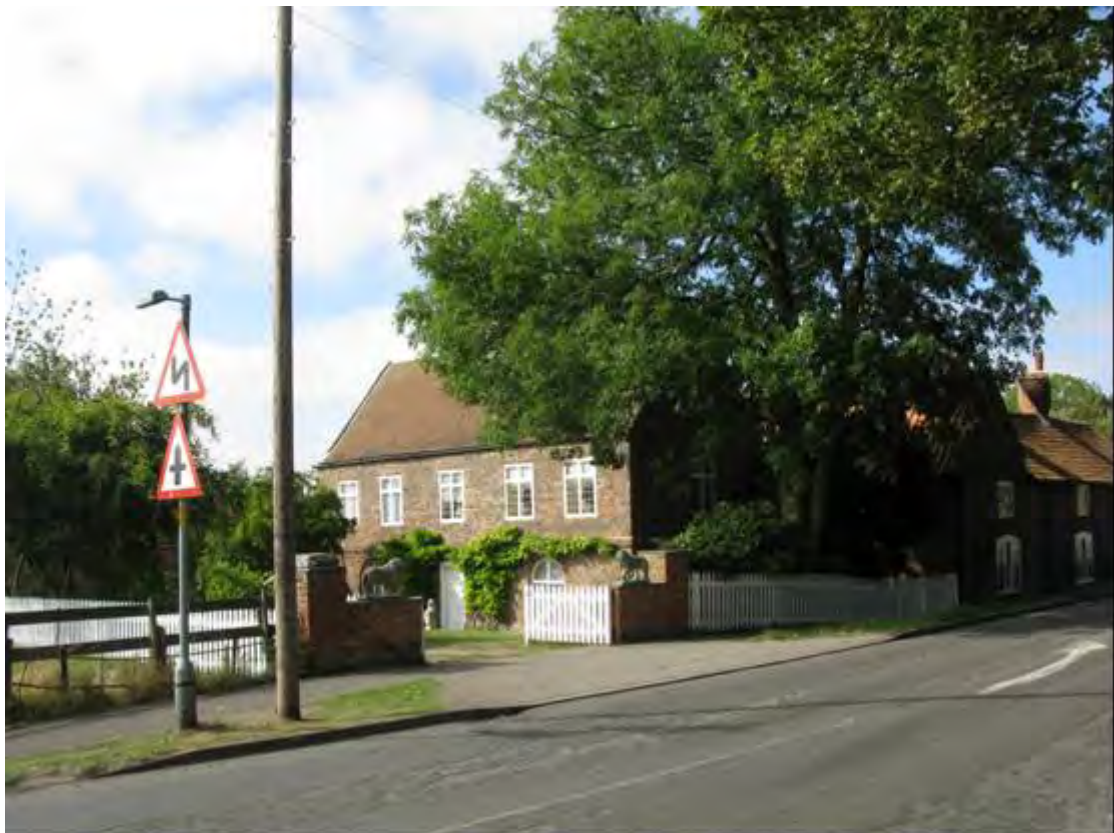
Plate 48 Manor House (SH18), Skidbrooke with Saltfleet Haven
