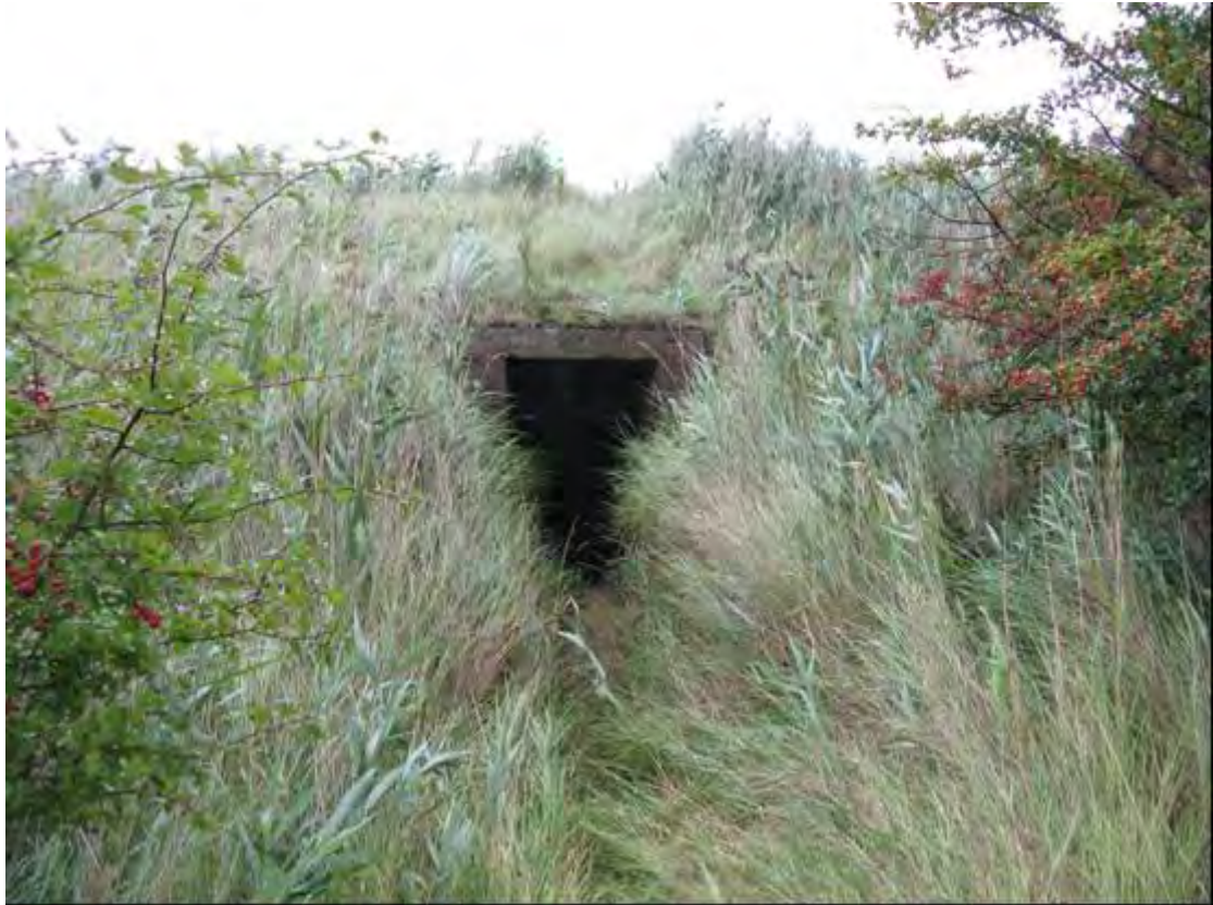
Plate 5 Entrance tunnel to WW2 observation post NS15, North Somercotes
