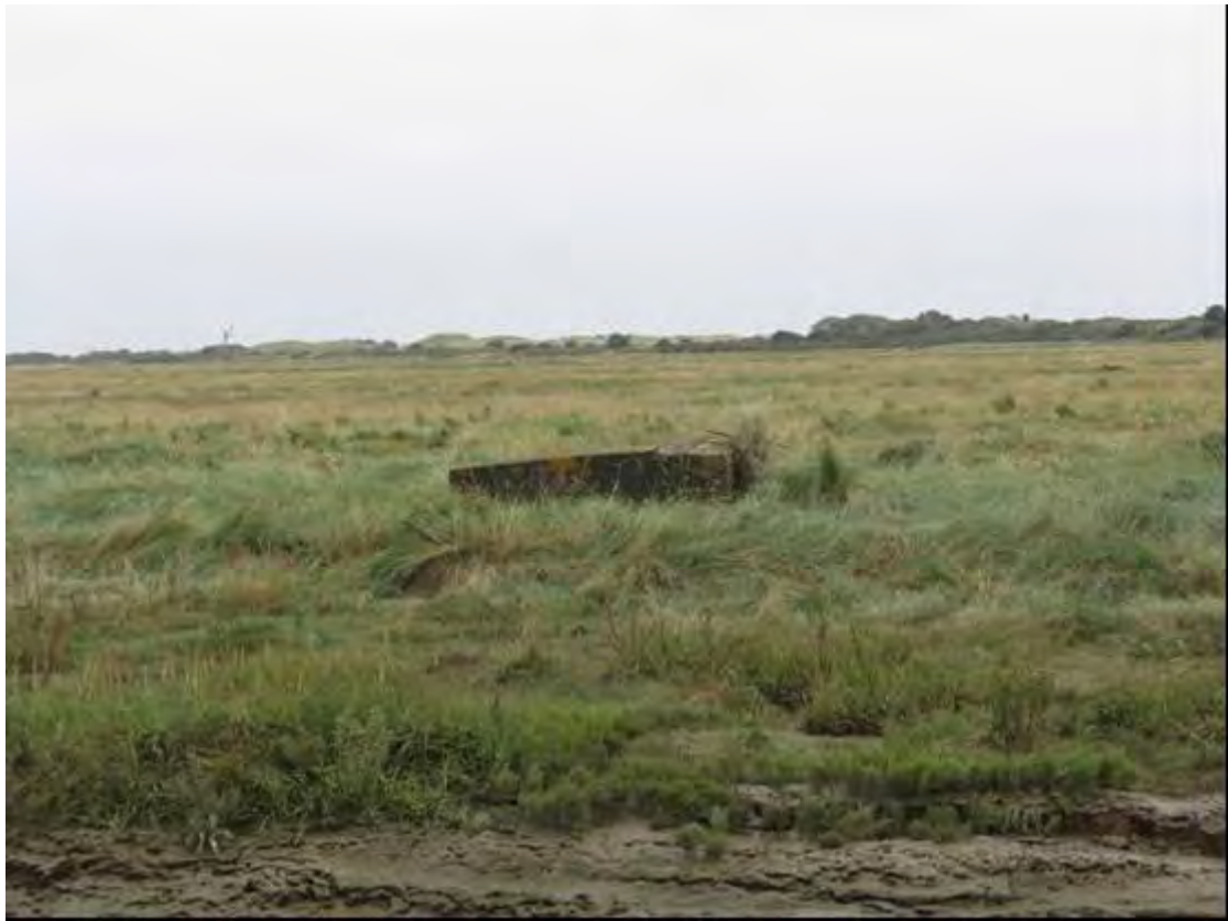
Plate 59 WW2 concrete structure SA1, Saltfleetby
