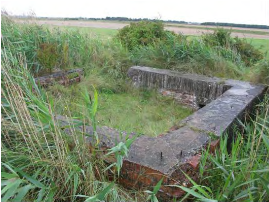
Plate 8 Base for upper floor of WW2 observation post NS15, North Somercotes
