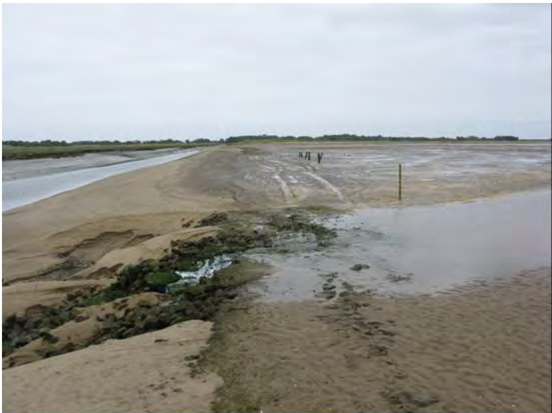
Plate 52 Exposed causeway SH22, Saltfleet Haven
