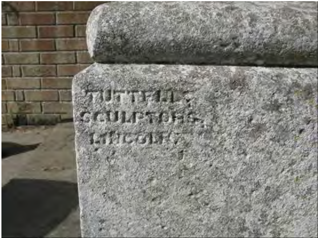
Plate 45 Mason's details, Saltfleet pump (SH14), Skidbrooke with Saltfleet Haven
