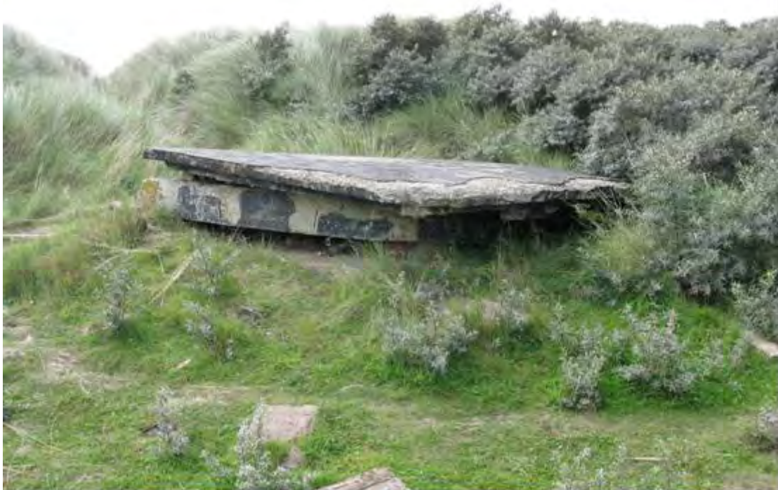
Plate 9 Collapsed WW2 pillbox or observation post NS62, North Somercotes
