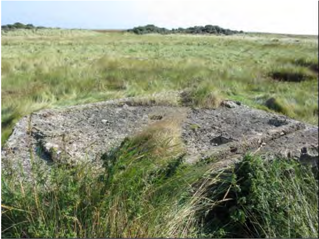
Plate 39 Roof mountings, gun emplacement SH4, Skidbrooke with Saltfleet Haven
