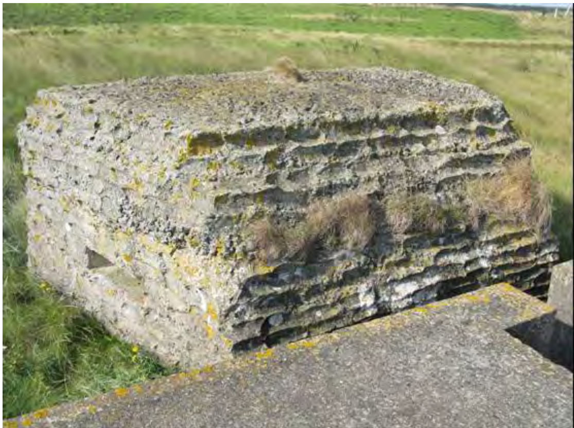
Plate 34 Rusticated square pillbox, SH1 pair, Skidbrooke with Saltfleet Haven
