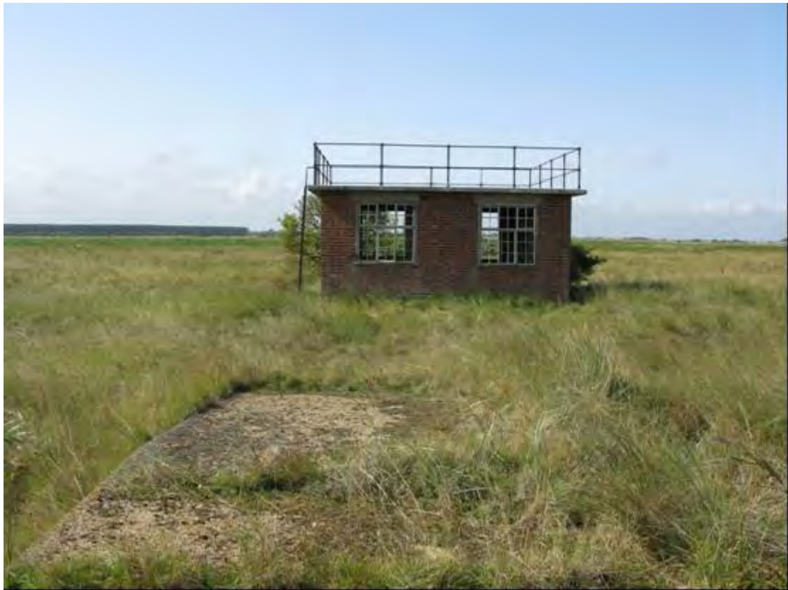
Plate 21 Brick building NS69 and ramp NS68 (foreground), North Somercotes
