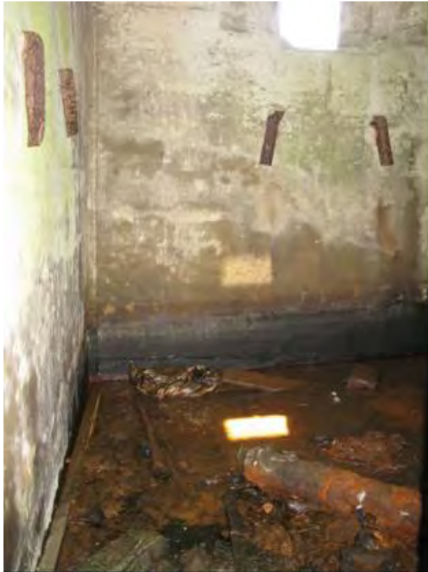
Plate 25 Interior of pillbox NS72, North Somercotes
