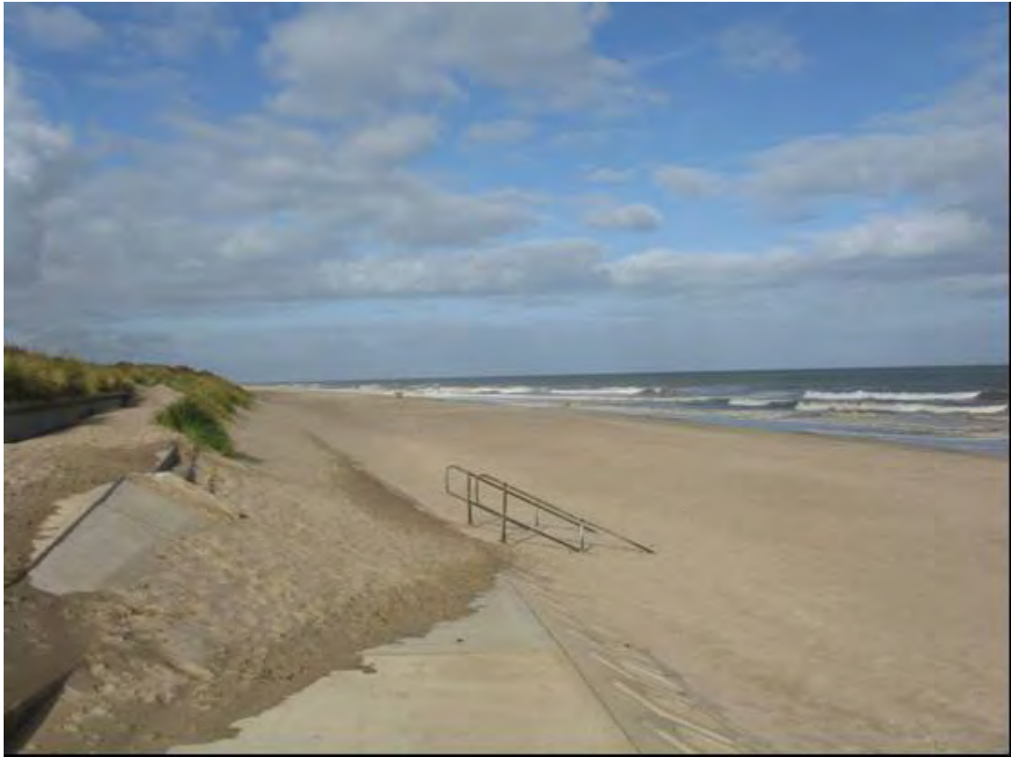
Plate 121 General view of beach and sea defences, Huttoft
