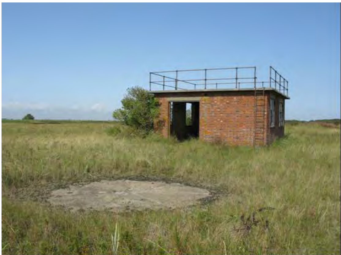
Plate 22 Building NS69 and segmented platform NS70, North Somercotes
