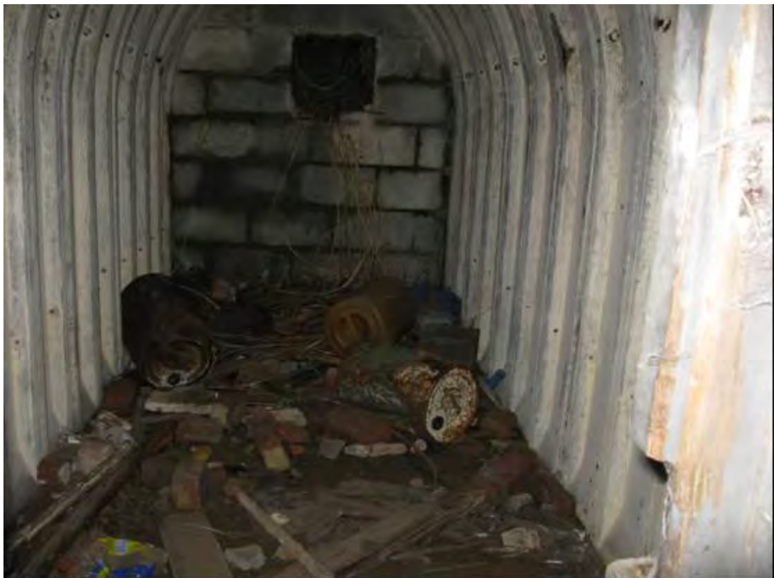
Plate 6 Side chamber, WW2 observation post NS15, North Somercotes
