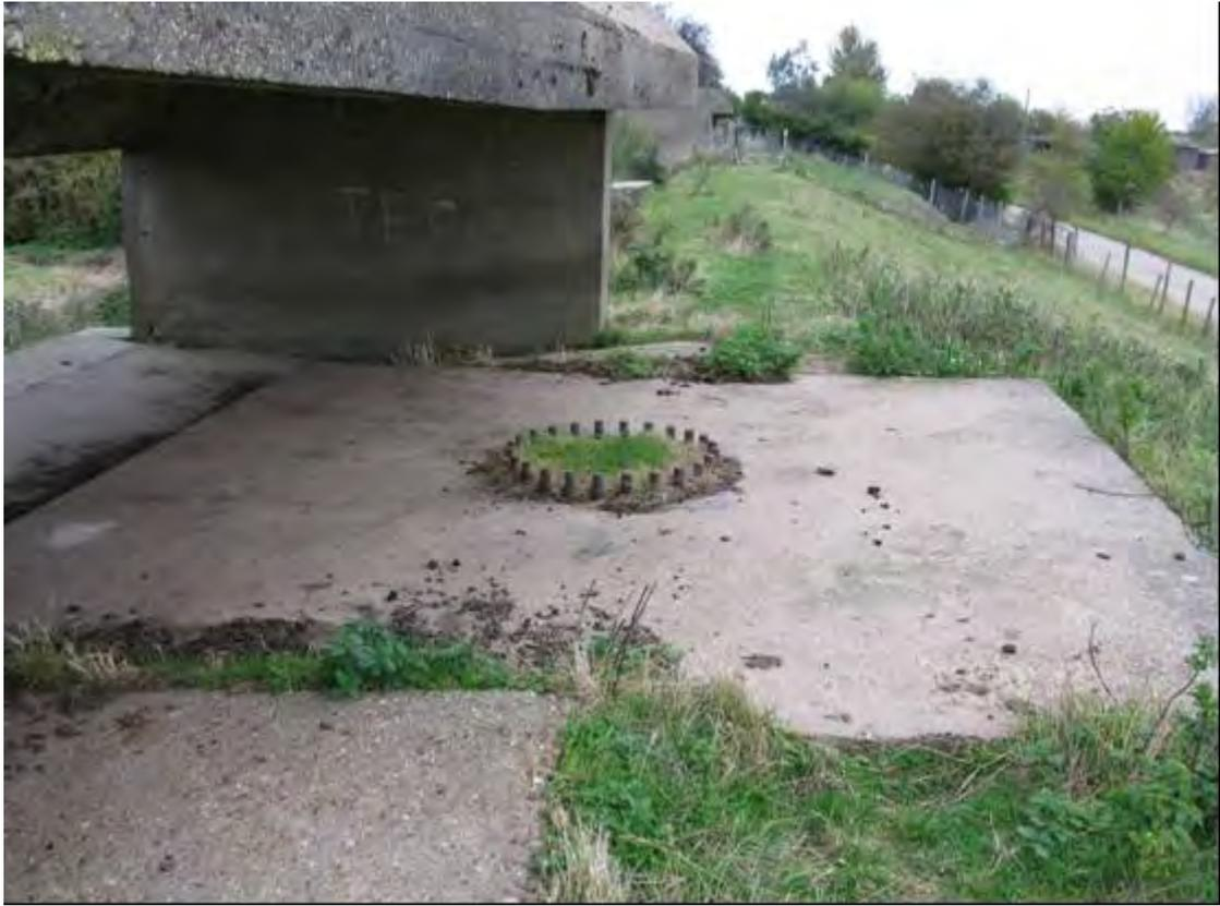
*Plate 63 Holdfast, gun emplacement (FR16), WW2 Freiston Shore Battery*
