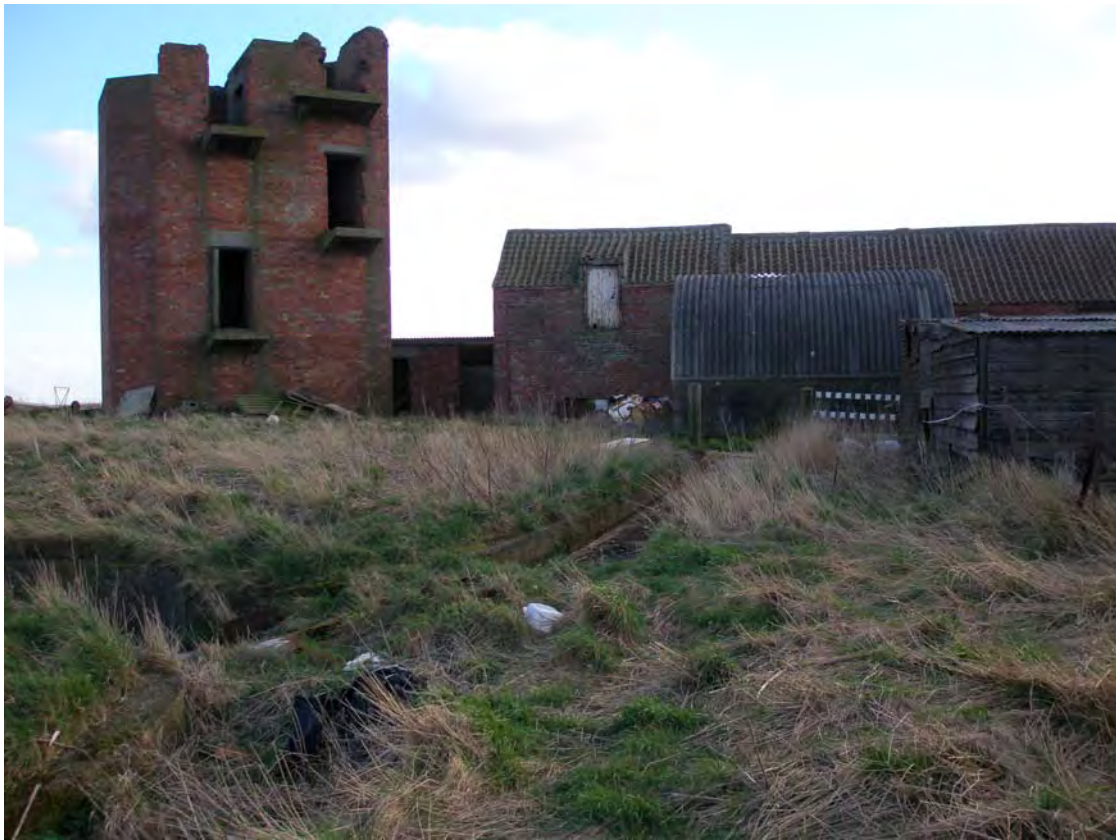
Plate 19 Battery observation post at Ringbrough Farm, Ringbrough Battery (AL52) Aldbrough
