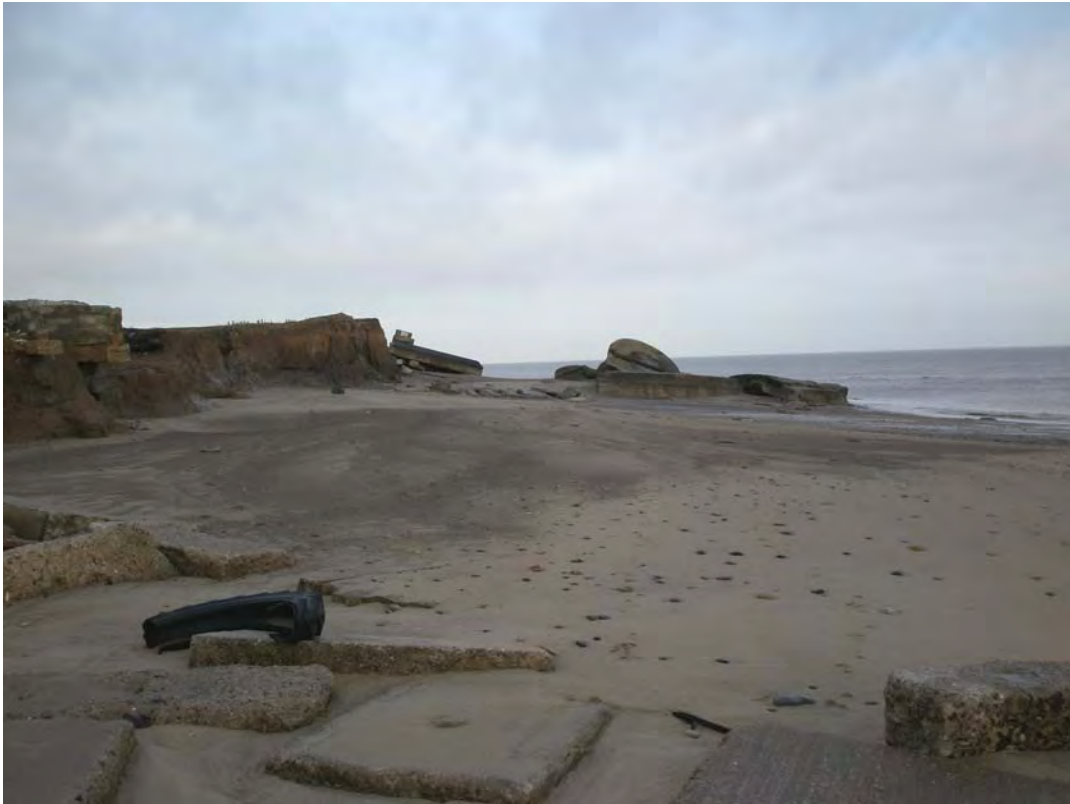
Plate 27 Second 9.2in gun platform and magazine, with remains of sea defence wall, Godwin Battery, Easington (EA182), looking north
