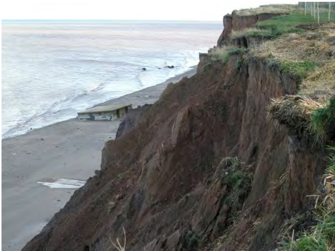
Plate 20 Eroding cliff edge, Aldbrough
