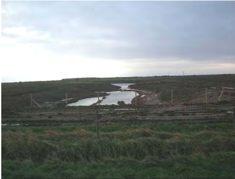
Plate 29 Work underway on borrow pits for new sea defences, Kilnsea, looking south (EA206). The field beyond the pit contains Romano-British features
