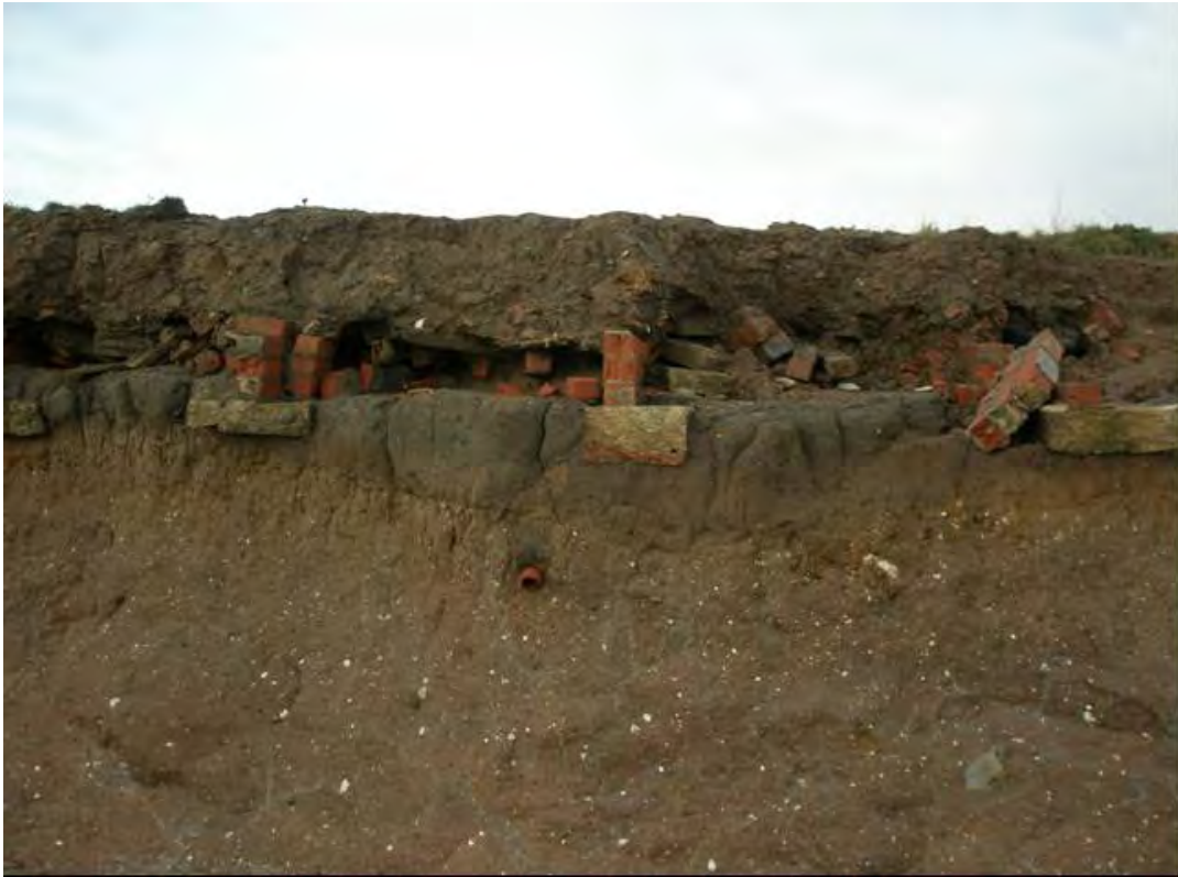
Plate 28 Demolished remains of Officers' Quarters beneath new land surface and overlying earlier soil horizon, Godwin Battery, Easington (EA182)
