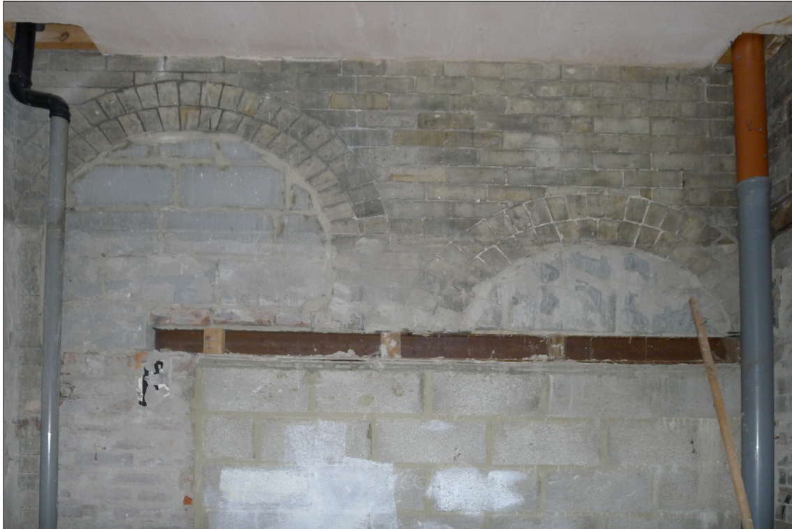
Fig 16: The former central light well, now ceiled and accessed from the billiard room. It provided light for windows on all four sides, and is executed, like the other light wells, in gault brick.. © Historic England / Lucy Jessop.
