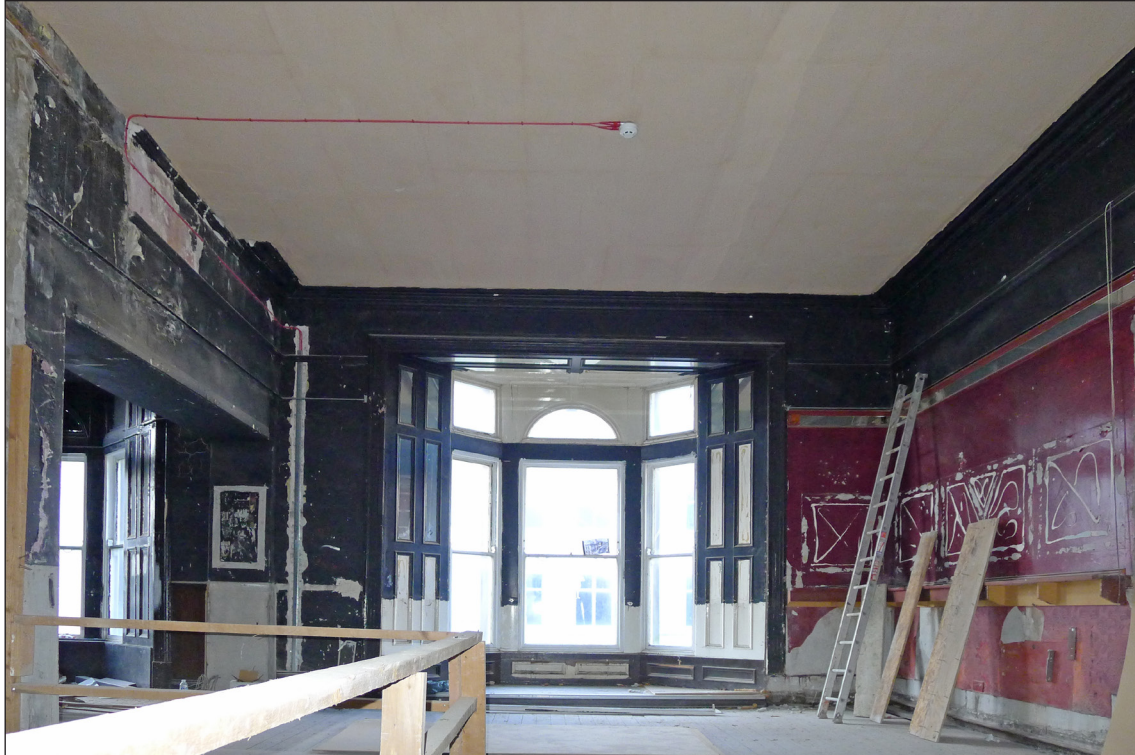
Fig 16: The former central light well, now ceiled and accessed from the billiard room. It provided light for windows on all four sides, and is executed, like the other light wells, in gault brick.. © Historic England / Lucy Jessop.
