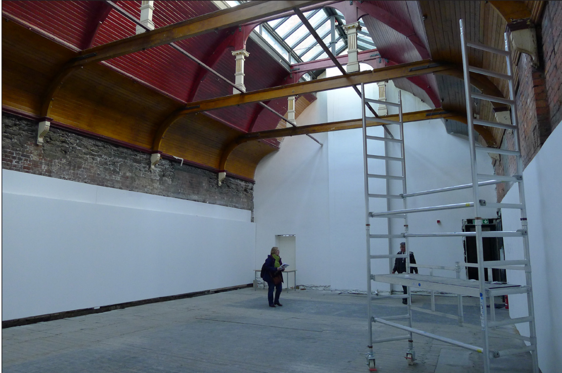
Fig 15: The 1900 billiard room, with its timber trusses with metal strapping, slender reinforcement bars, Ionic queen posts, fluted consoles and the boarded, double coved ceiling. © Historic England / Tristan Wilson.
