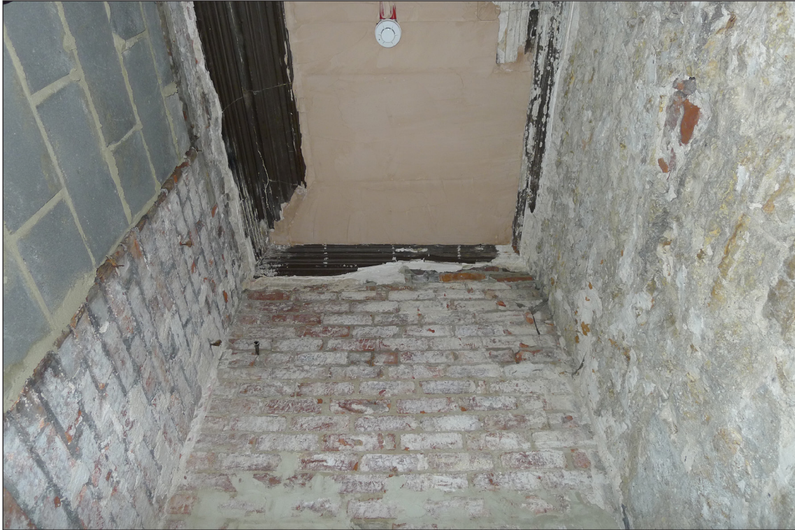
Fig 14: The end of the 1900 corridor on the first floor, looking up above the doorway to the billiard room. To the right is the surviving 1840s rubble internal wall; to the left is a tall blocked window which would have looked onto the middle light well. © Historic England / Lucy Jessop.
