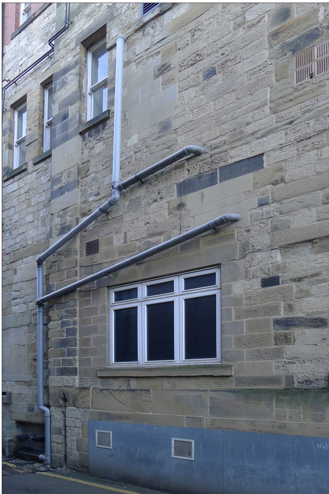
Fig 7: Detail of the eastern elevation facing the rear alleyway, Athenaeum Buildings. The open-textured limestone and sandstone ashlar of the 1840s building, with its projecting corners, can be clearly seen, with later blocked and refenestrated openings. © Historic England / Lucy Jessop.
