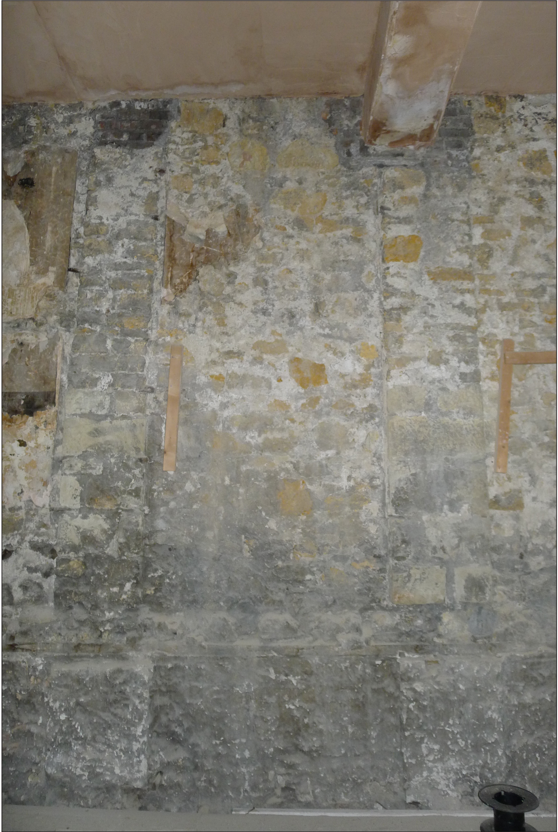
Fig 13: The rubble and ashlar party wall on the ground floor of the Athenaeum, part of the remaining 1840s fabric.. © Historic England / Lucy Jessop.
