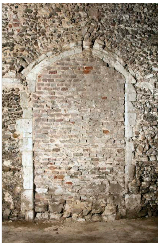
Figure 49 (Left): The rere-arch of the doorway between the north transept and the room north of the nave. © Historic England, Patricia Payne, DP217023
