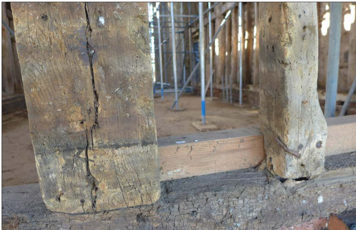
Figure 60: Intermediate Post, with VII carpenters' mark representing its position as the seventh upright timber in the gable wall. Evidence for trestle-sawn post to east gable wall of east barn. © Historic England, Elizabeth Chamberlin
