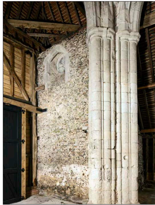
Figure 41: The blocked sexfoiled clerestory window in the north stub wall of the nave viewed from inside the crossing. © Historic England, Patricia Payne, DP217019
