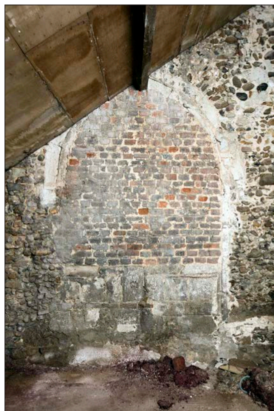
Figure 49 (Left): The rere-arch of the doorway between the north transept and the room north of the nave. © Historic England, Patricia Payne, DP217023
