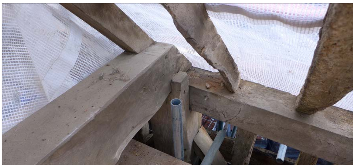
Figure 57: Tiebeam II (north side of barn). Top of post is jowled & extends beyond top of wall plate. Tiebeam is seated into the top of the jowled post. © Historic England, Elizabeth Chamberlin
