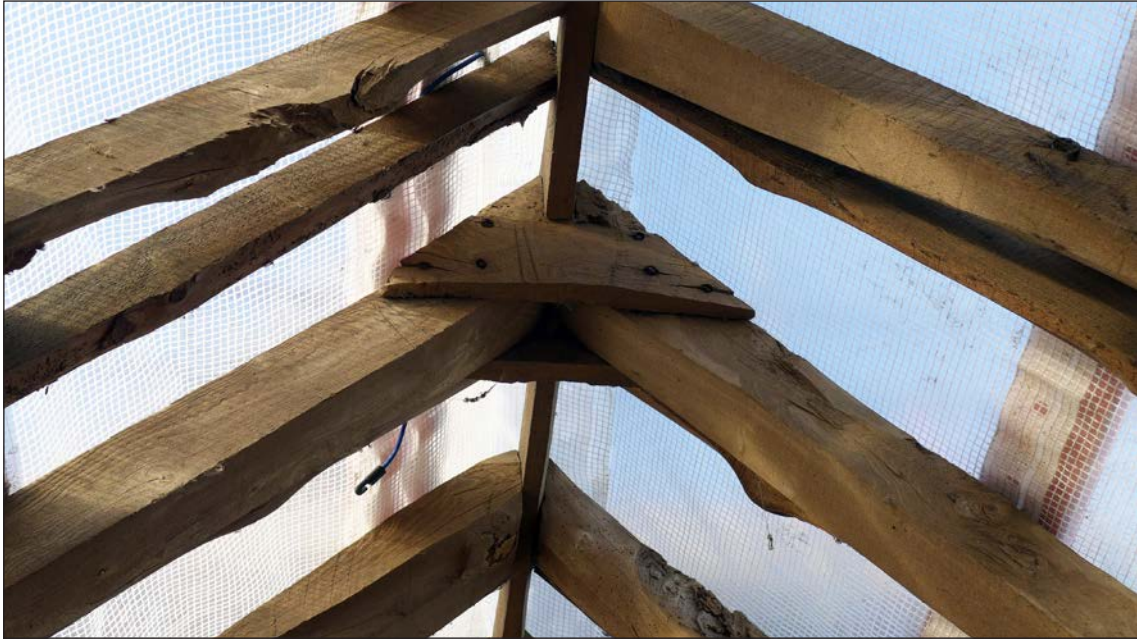
Figure 66: Apex of South Barn roof, with ridge plank and nailed saddles. There appears to be a scribed carpenter's mark on the saddle. © Historic England, Elizabeth Chamberlin
