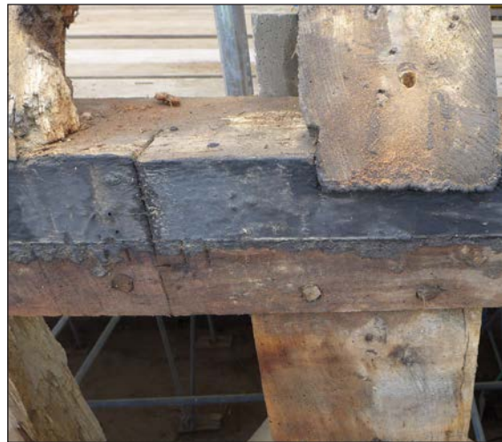
Figure 61 (Left): Roman numeral to the scarf joint of the sill beam immediately adjacent to the post appears to read PII (the horizontal stroke between the two II marks appears to be a natural mark in the timber). To the left of the image is another carpenters' mark, which appears to show a III . © Historic England, Elizabeth Chamberlin
