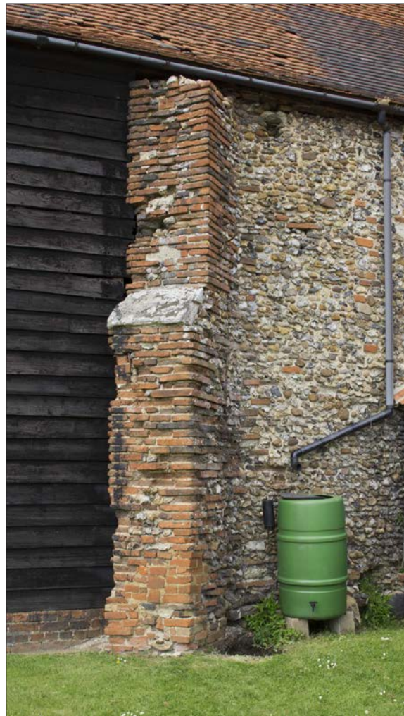
Figure 54: The brick buttress at the south-east corner of the south transept. Although heavily altered and repaired, it is possible that it is comprised largely of bricks dating from the late-12th century and manufactured at Waltham Abbey. © Historic England, Patricia Payne, DP173631
