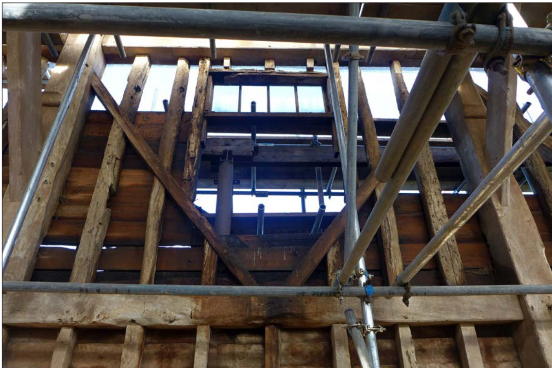
Figure 58: Inserted window in N wall of East Barn. Three chocks inserted above head of window to support the position of the frame. The mortice holes for the tenons of the original studs are just visible to chocks 1 and 3. © Historic England, Elizabeth Chamberlin
