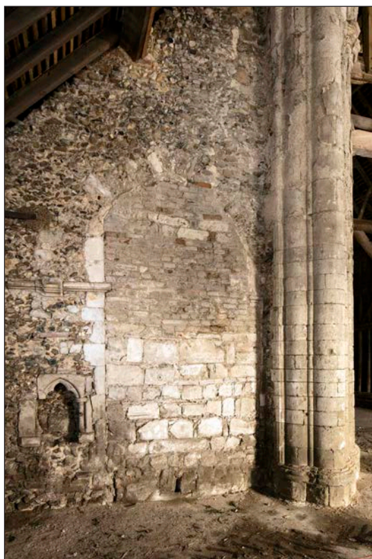
Figure 45 (Left): Heavily altered and remade arch in the east wall of the north transept. It likely accessed a north chapel. © Historic England, Patricia Payne, DP217025
