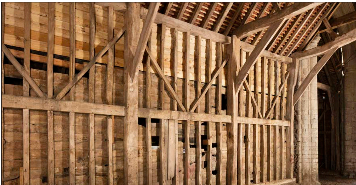
Figure 59: Close studding and tension bracing above the mid-rail. Internal view of south wall of east barn. © Historic England, Patricia Payne, DP217030
