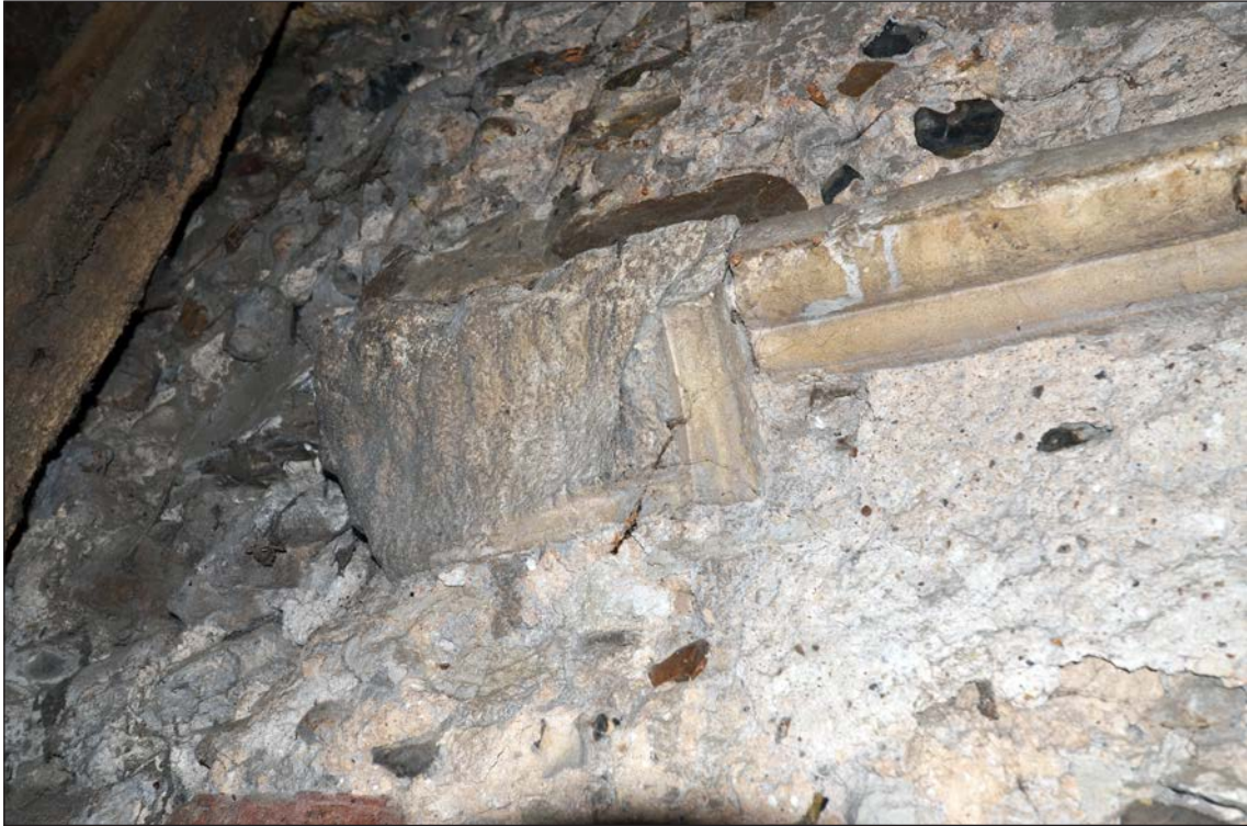
Figure 47: Ex situ worked stone used to remake an internal stringcourse. One piece may contain the fragment of a rib. © Historic England, Matthew Bristow
