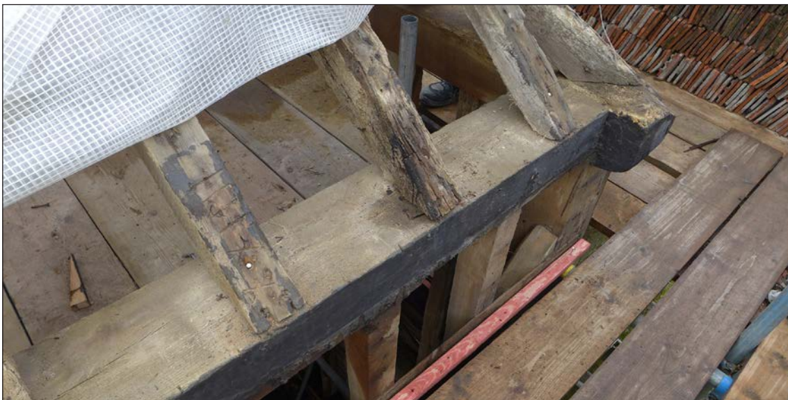
Figure 55: The transverse (east gable) wall plate is shown on the left with the longitudinal wall plate on the right (which extends beyond the end gabled wall). © Historic England, Elizabeth Chamberlin
