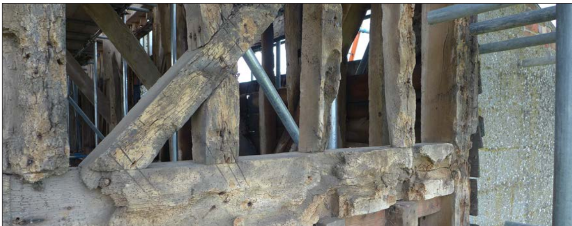
Figure 64 (Above): East elevation of East gable wall of barn, upper level, south side. The numbering of the studs and struts is consecutive, strut 4 is numbered 'CCCC', the raking strut immediately adjacent to it is numbered CCCCC and the next stud CCCCCC. © Historic England, Elizabeth Chamberlin
