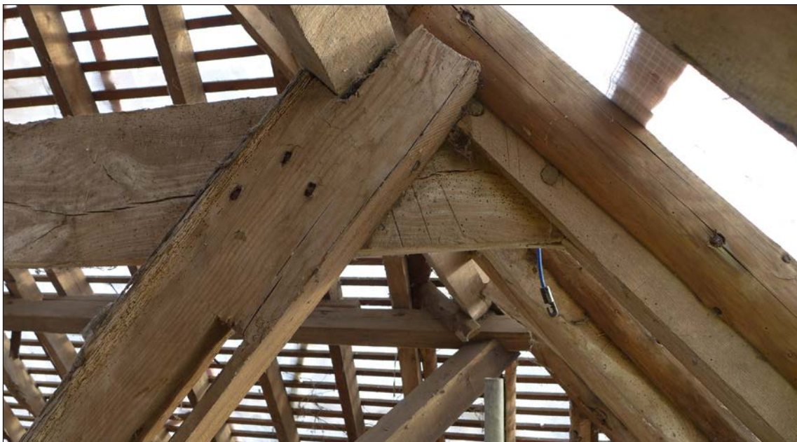
Figure 67: South Barn, raking strut inserted to provide additional support to purlin. The strut and the additional piece added to strengthen the rafter overlie the scribed carpenter's marks beneath. Note the original pegged construction of the rafter and collar and the use of nails for timbers added at a later date. © Historic England, Elizabeth Chamberlin
