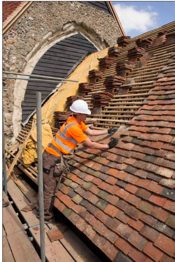
Figure 2: Work to replace the peg-tile roof of the east barn during May 2016. The exposed and heavily weathered crossing arch can be seen behind. © Historic England, Patricia Payne, DP182391
