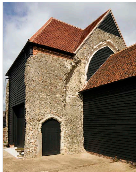
Figure 42: The deep scar west of the south transept crossing arch indicating the former location of a stair turret. © Historic England, Patricia Payne, DP217007
