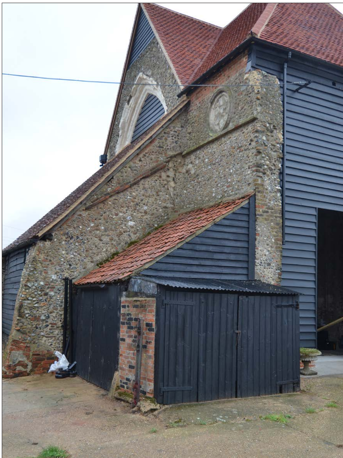
Figure 51: The blocked sexfoiled clerestory window, stringcourse and scar of roofline. ©Historic England, Matthew Bristow
