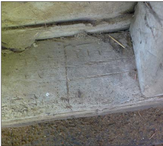
Figure 61 (Left): Roman numeral to the scarf joint of the sill beam immediately adjacent to the post appears to read PII (the horizontal stroke between the two II marks appears to be a natural mark in the timber). To the left of the image is another carpenters' mark, which appears to show a III . © Historic England, Elizabeth Chamberlin
