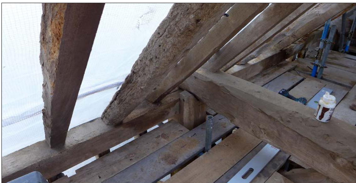
Figure 56: Tiebeam II (south side of barn). The top of the jowled post has been roughly shaped to receive the tiebeam –this is probably due to the position of scarf joints in the wall plate at this precise location. © Historic England, Elizabeth Chamberlin
