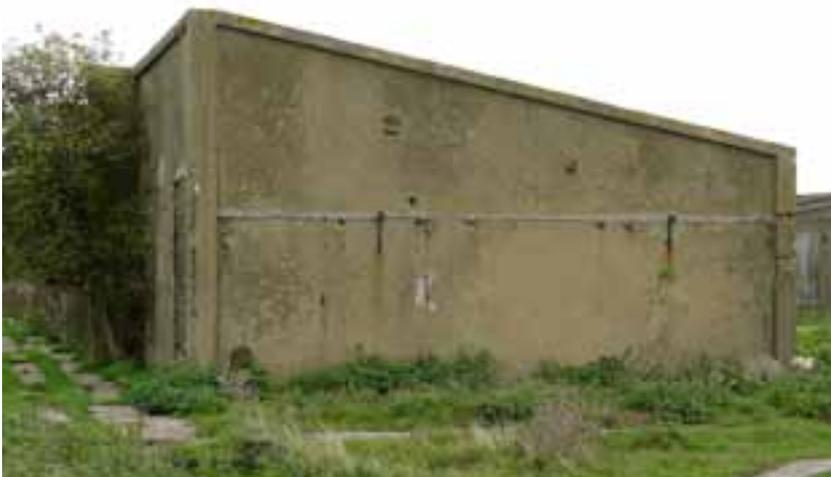
Figure 146: Cordite Press House **246**, showing iron brackets and witness marks for a lean-to structure at the west end. Photograph: Wayne Cocroft, 2010 © English Heritage.
