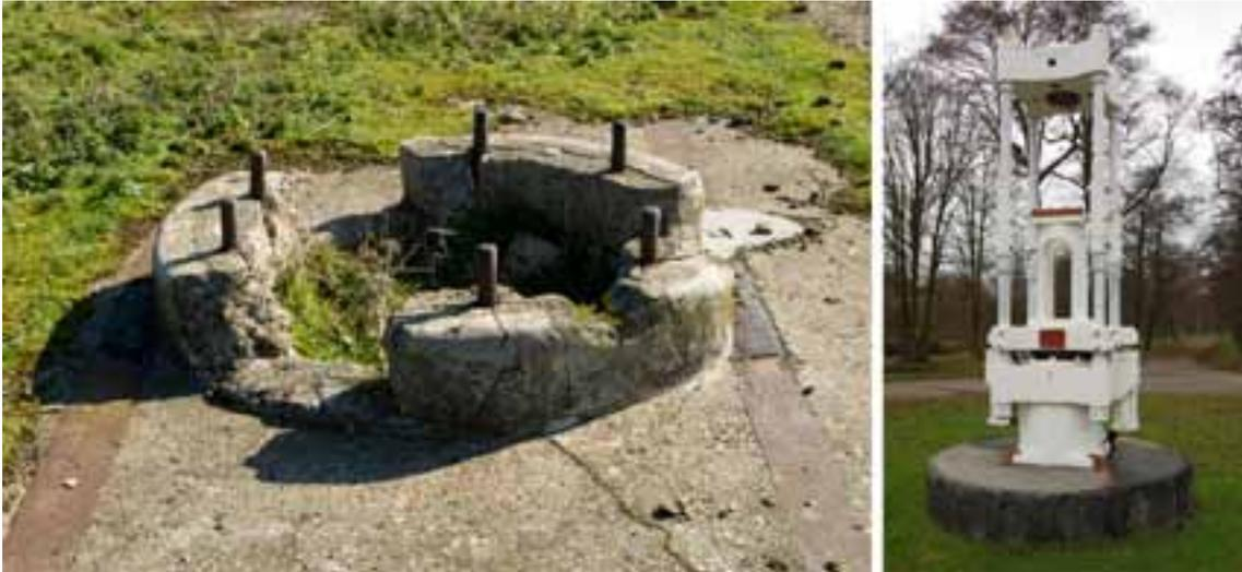
Figure 91: (above left) Detail of a hydraulic press base in structure **108**. NMR DPI41541 07-Mar-2011, Steve Cole © English Heritage.
