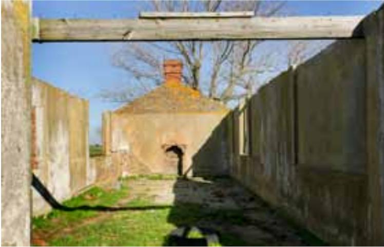
Figure 81: (above left) Inside structure **67**, looking north, showing the small fireplace and the rendered recesses of the blocked windows. NMR DPI41518 07-Mar-2011, Steve Cole © English Heritage.
