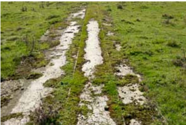
*Figure 90: Iron tram rails and cambered cement tram-bed between structures **107** and **108**, looking south-west. NMR DPI41543 07-Mar-2011, Steve Cole © English Heritage.*
