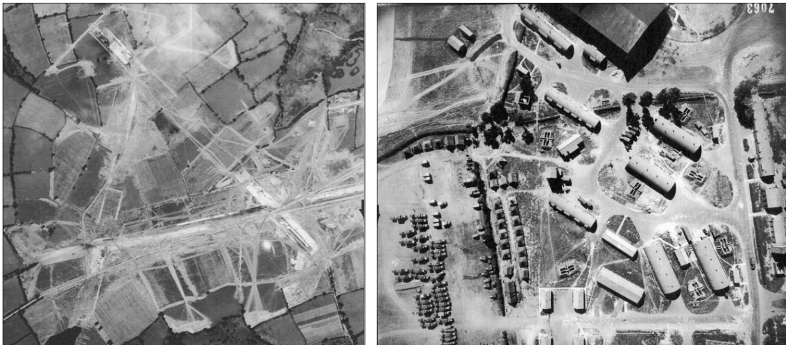
Fig 54: RAF Upottery (MDV47202) and Merryfield (SOM55403) were constructed in preparation for the invasion of Europe. RAF Upottery under construction in 1943 (left) and signs of military troop build-up in August 1944 at Merryfield, with bell tents and trucks to the left of the Nissen huts and embanked shelters (right). US/7PH/GP/LOC14 6028 09-AUG-1943 Historic England (USAAF Photography); US/7GR/LOC390 FV 7063 13-AUG-1944 Historic England (USAAF Photography).
