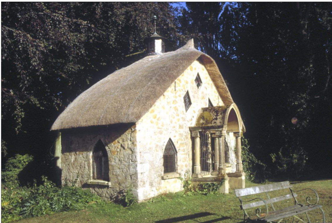
Fig 34: Grotto at Jordans House. Somerset HER image 6554. © Somerset County Council.
