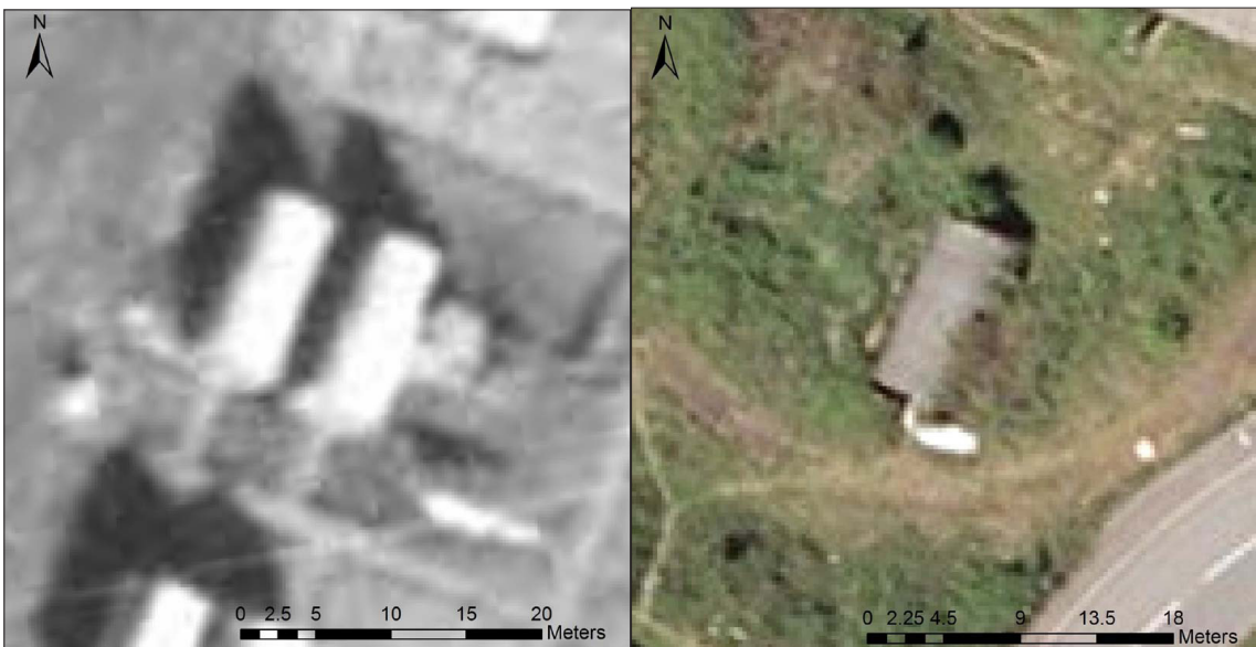
Fig 59: The sole surviving military structure at Millwey Rise in 2010 (right) and with its pair in 1948 (left); this too has now been demolished (MDV49431). RAF/CPE/UK/2431 RP 3201 22-JAN-1948 Historic England (RAF Photography). Next Perspectives APGB Imagery SY3099 23-MAY-2010. RGB Aerial Photography © Bluesky International/Getmapping PLC.
