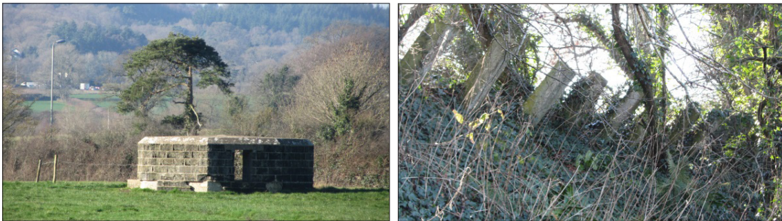
Fig 45: Anti-tank gun emplacement and concrete post forming an anti-tank obstacle on a railway embankment of Second World War date, part of the Taunton Stop Line, just beyond the survey area south of Bow Bridge, Axminster (MDV50876 and MDV50885, circa SY 290 980). Photographs: S. Knight 2017.
