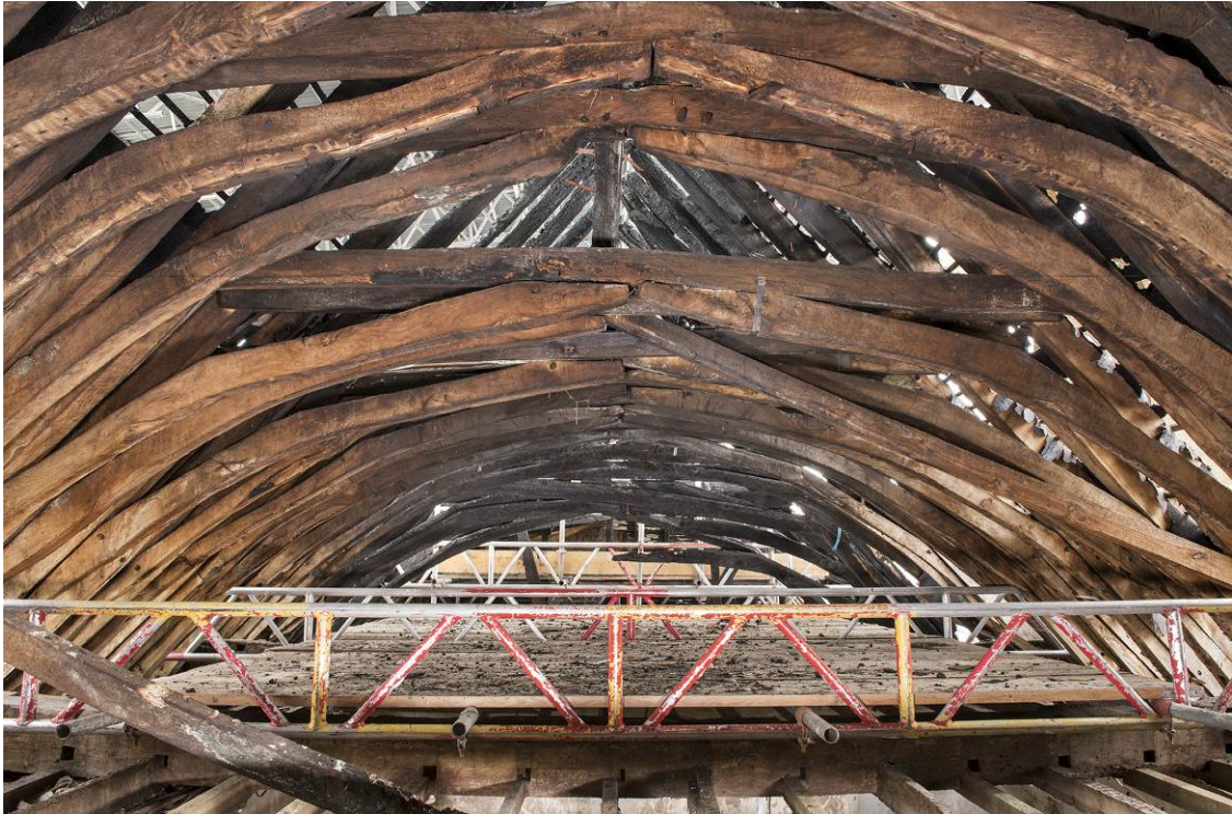
Fig 17 Looking east along the interior of the roof. The post in the upper-centre of the frame is a later addition. HEA DP196761.
