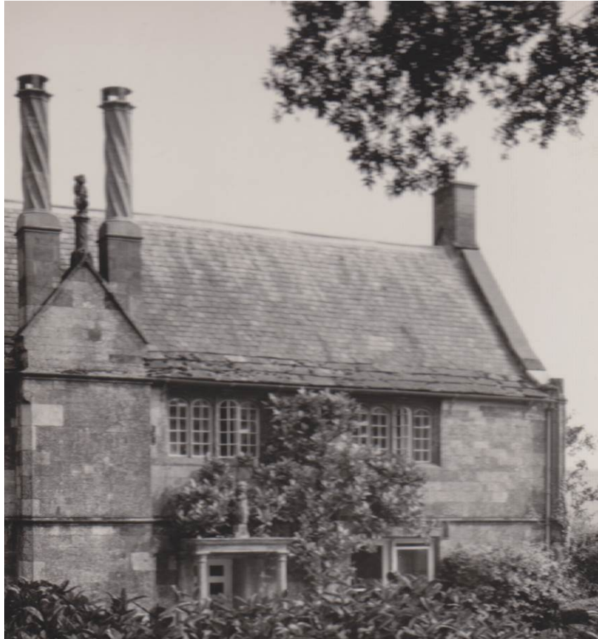
Fig 7 The eastern part of the south elevation of the house. The photograph was probably taken in 1947 by RCHME investigators. HEA IN00484 DM 1525.
