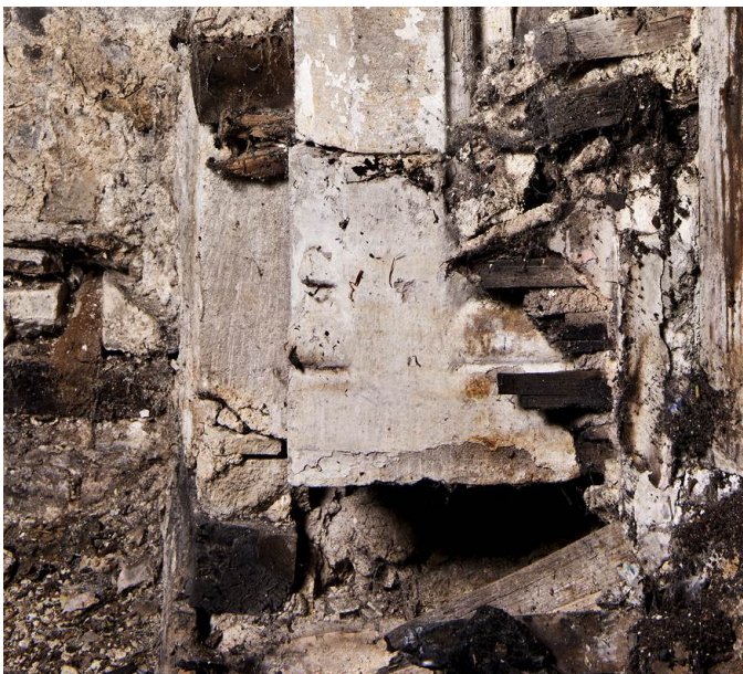
Fig 16 Detail of the lower part of the left hand side of the fireplace showing the vase stop. HEA DP196752.
