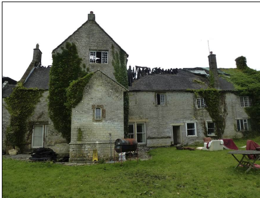
Fig 8 The north (rear) elevation shortly after the fire.
