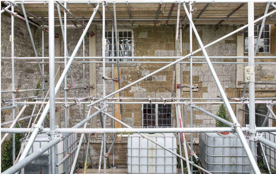
Fig 23 The straight joint between the two phases of the main range is behind the scaffolding plank below the left hand first-floor window. HEA DP196820.
