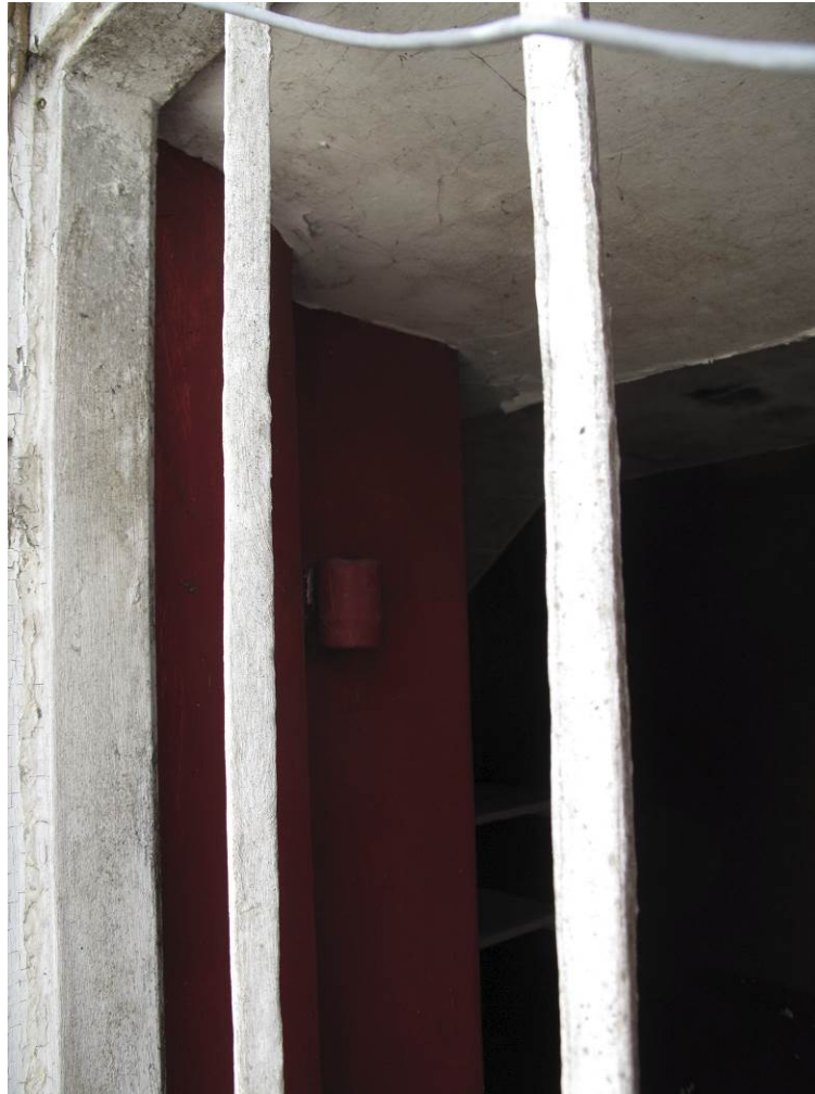
Fig 34 The metal hinge behind the window on the ground floor at the west end of the main range. It is possible this was once a doorway. Photo: Rebecca Lane.
