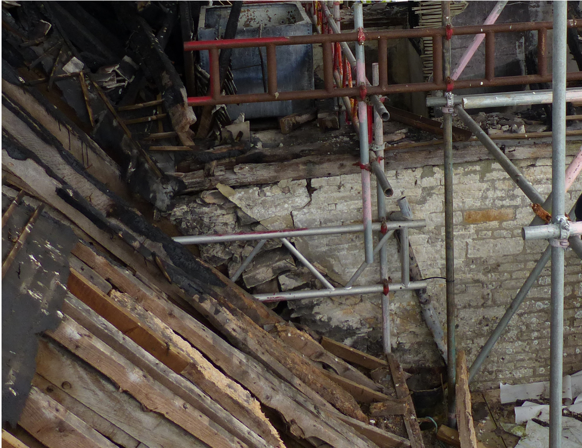
Fig 28 View looking west showing the east wall of the north range resting on the roof of the main range. Photo: Helen Winton.
