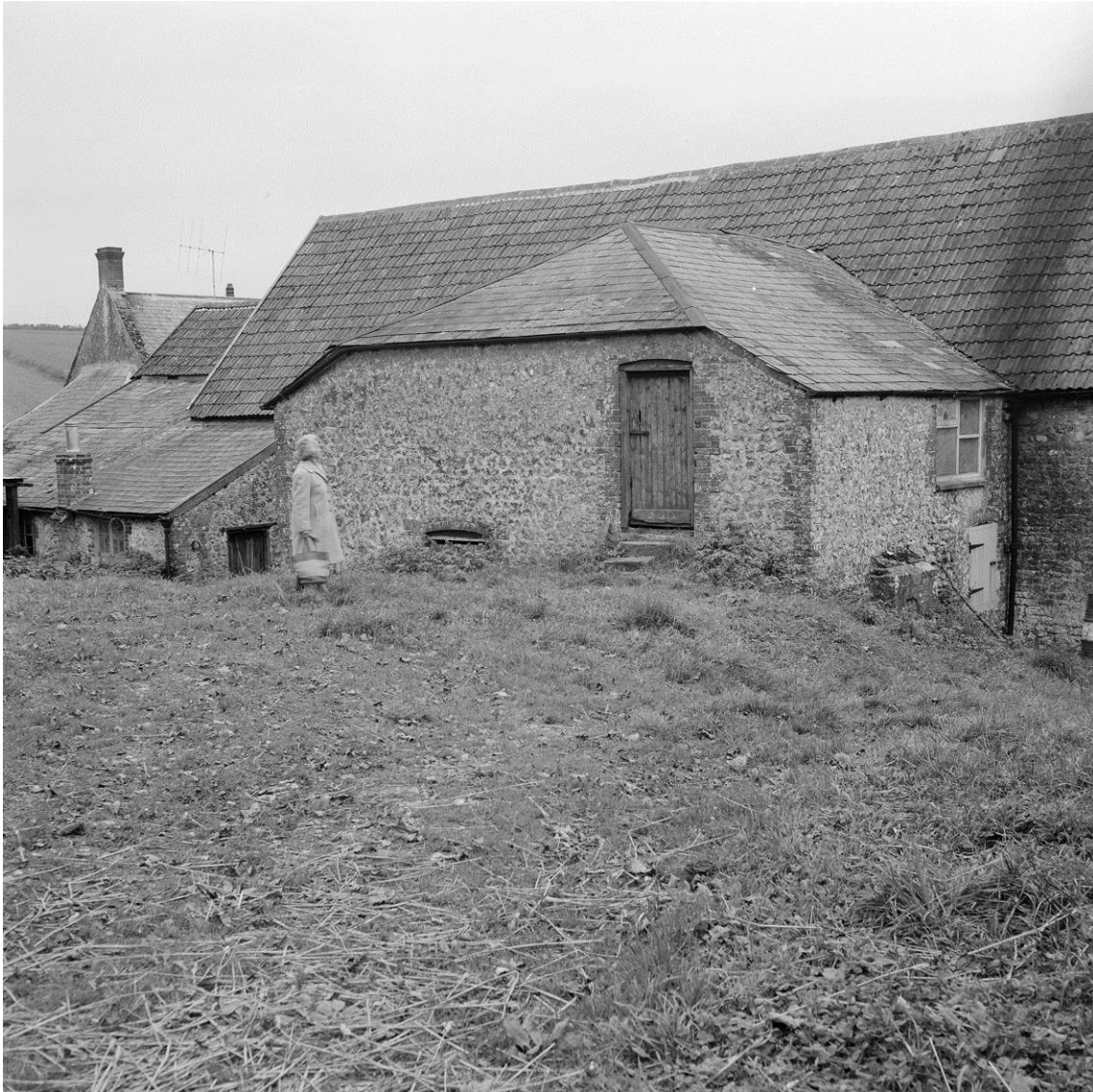
Fig 36 Looking north east towards the back of the barn c1960. The house, with the single storey extension against the west gable, is far left of the frame. HEA AA043154.
