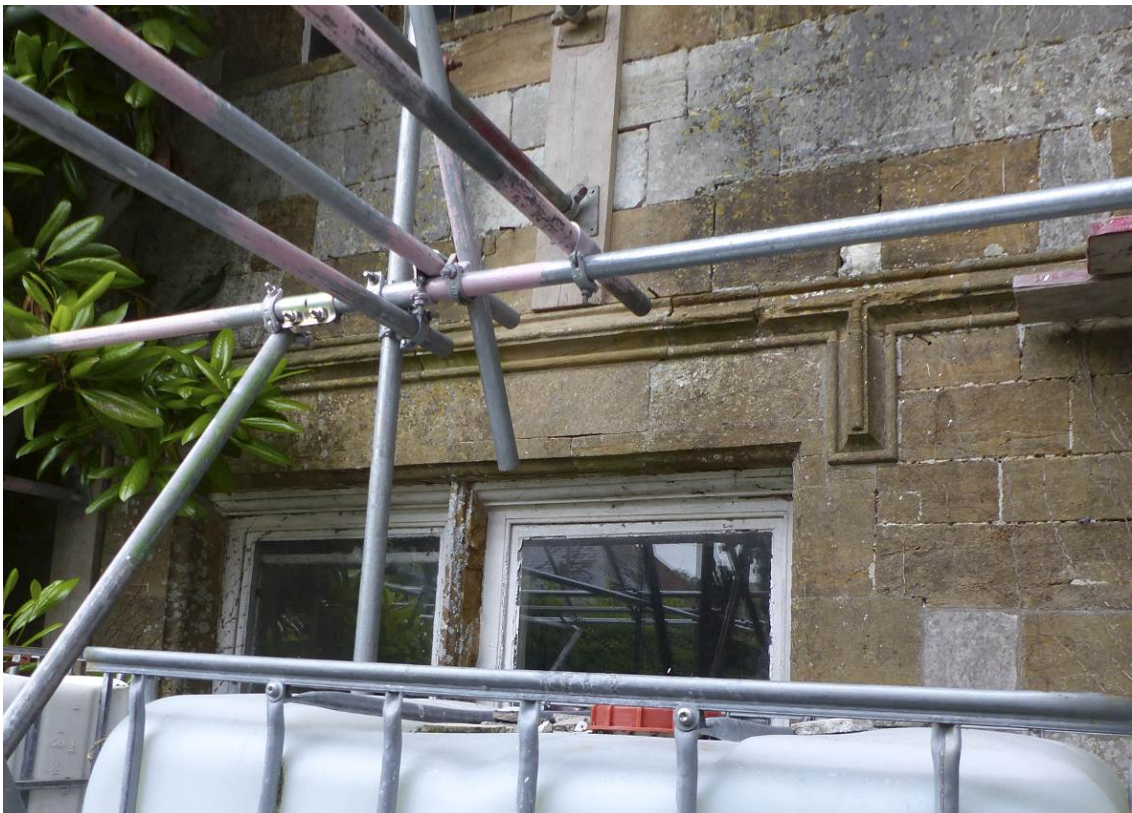
Fig 12 The south elevation showing the string course extending across the top of the ground floor window to the east of the front door. Photo: Helen Winton.
