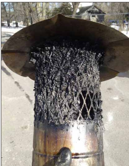
Figure 35. Tarred up chimney bird guard.
