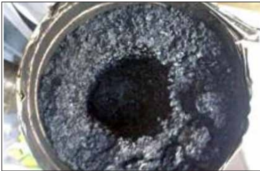
Figure 30. Tarred up chimney liner.
