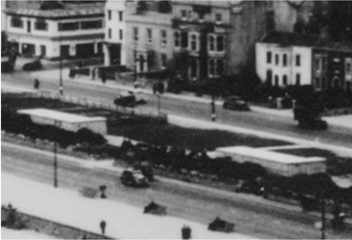
Figure 62 Public surface shelters on Beach Lawn in 1941. Detail of RAF/1416/S512184/PO-060 19-SEP-1941 Historic England (RAF Photography)
