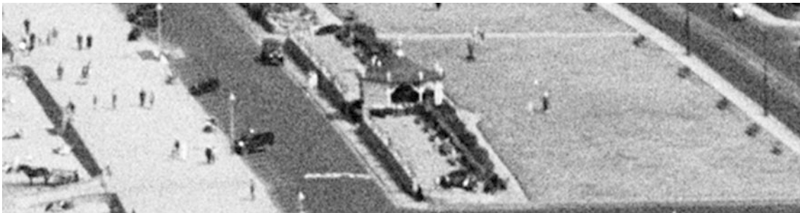
Figure 22 Repositioned bandstand on Beach Lawn seen in 1932. Detail of AFL 60818/EPW039935 Aug-1932 © Historic England (Aerofilms Collection)
