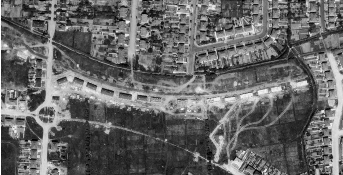
Figure 54 Cornish Units on Summerlands Road under construction. RAF/58/496 V 5132 09-JUN-1950 Historic England Archive (RAF Photography)
