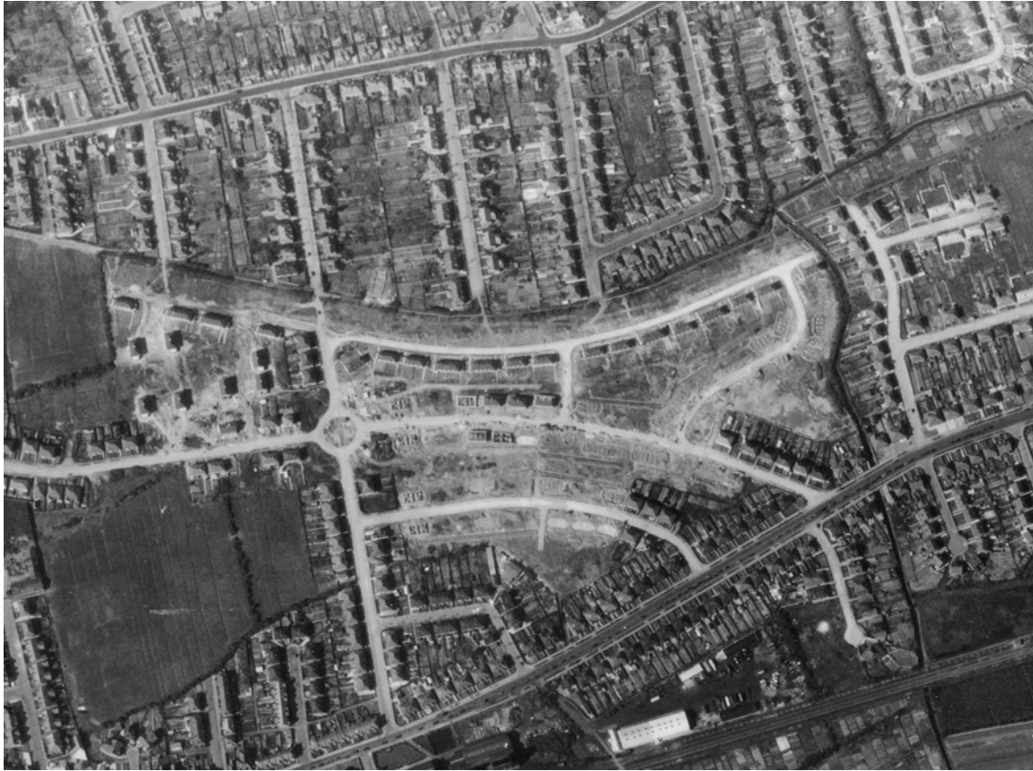
Figure 55 The Ashcombe estate under construction April 1951. RAF/540/479 RP 3022 22-APR-1951 Historic England Archive (RAF Photography)
