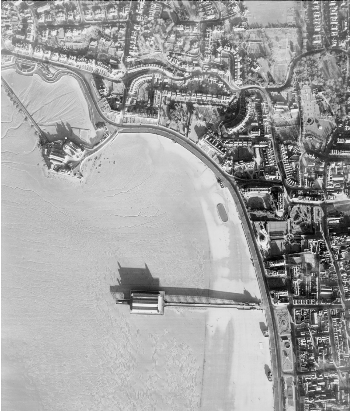
Figure 100 This RAF photograph was taken in 1946 at a scale of 1:5,000. Compare detail with Fig 2. Historic England Archive RAF Photography
