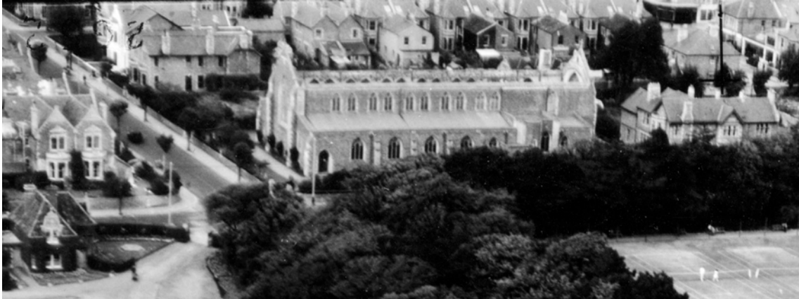
Figure 72 The shell of St Paul's Church, Clarence Road North in 1948. Detail of RAF/541/99/PSFO-0055 16-JUL-1948 Historic England Archive (RAF Photography)
