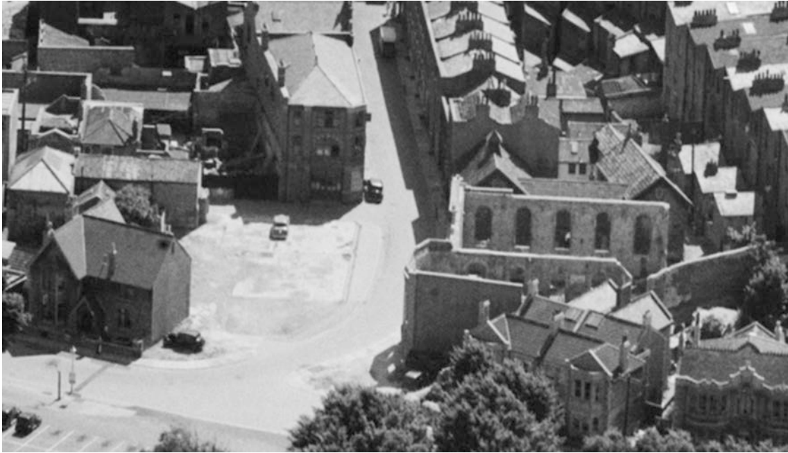
Figure 70 Bomb damage on Wadham Street 1949. The shell of the Baptist Chapel is on the right, opposite is a cleared bomb site. AFL 61877/EAW025151 25-Jul-1949 © Historic England (Aerofilms Collection)
