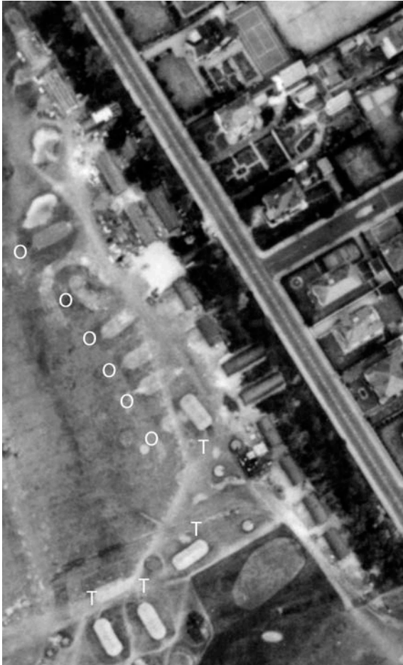
Figure 76 Uphill HAA in 1941. Tents are marked T, the outline of recently moved tents marked O. Accommodation huts can be seen alongside the road running diagonally across the image. Those at the top are still under construction. Detail of RAF/GHQ/105 V 14-MAY-1941 Historic England Archive (RAF Photography)
