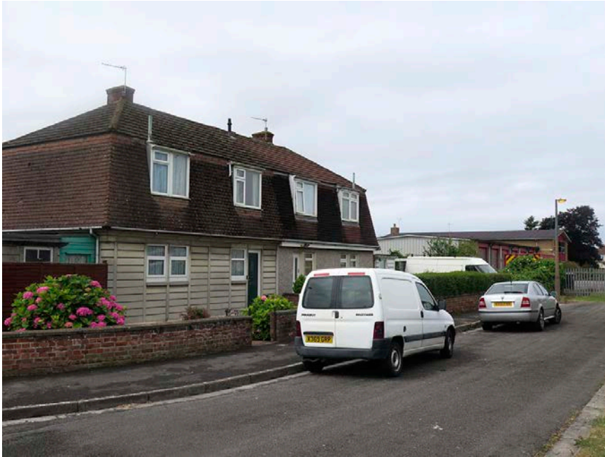
Figure 37 Cornish Unit in Summerlands Road with original concrete wall panels on the left. © Historic England
