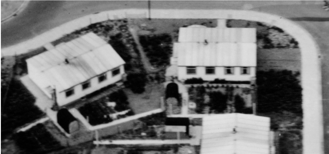
Figure 35 Prefabs on Selworthy Road, Bournville in 1948. Detail of RAF/541/99/PSFO-0059 16-JUL-1947 Historic England Archive (RAF Photography)
