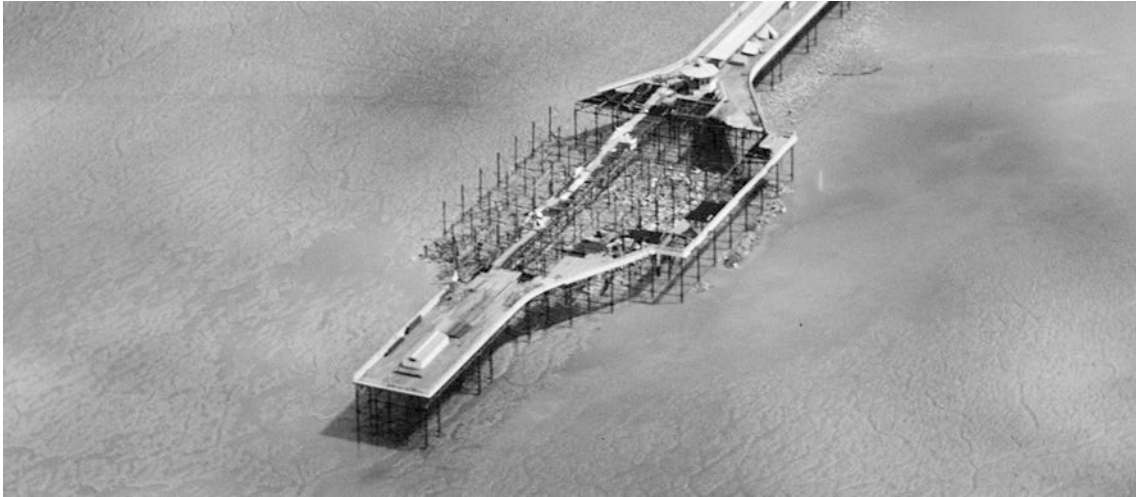
Figure 15 The fire damaged pier in 1930.
