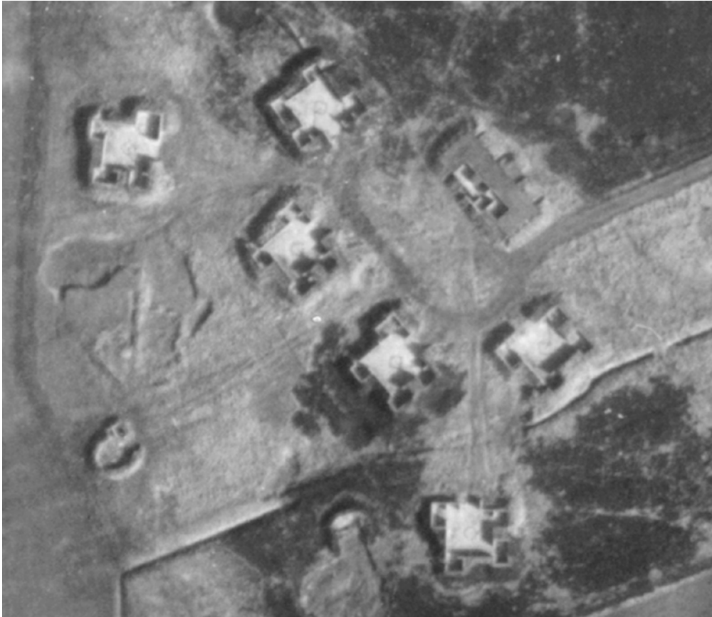
Figure 79 Uphill HAA emplacements and command post seen in 1948. RAF/CPE/UK/2489 V5053 11-MAR-1948 Historic England Archive (RAF Photography)
