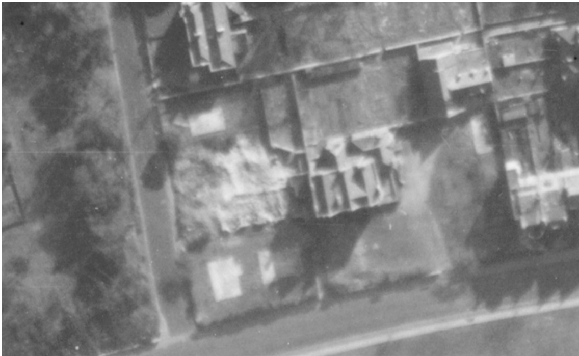
Figure 73 The rubble remains of Rossholme School on the seafront at the corner of Beach Road and Ellenborough Park South, demolished after bomb damage. Detail of RAF/CPE/UK/2489 V5049 11-MAR-1948 Historic England Archive (RAF Photography)
