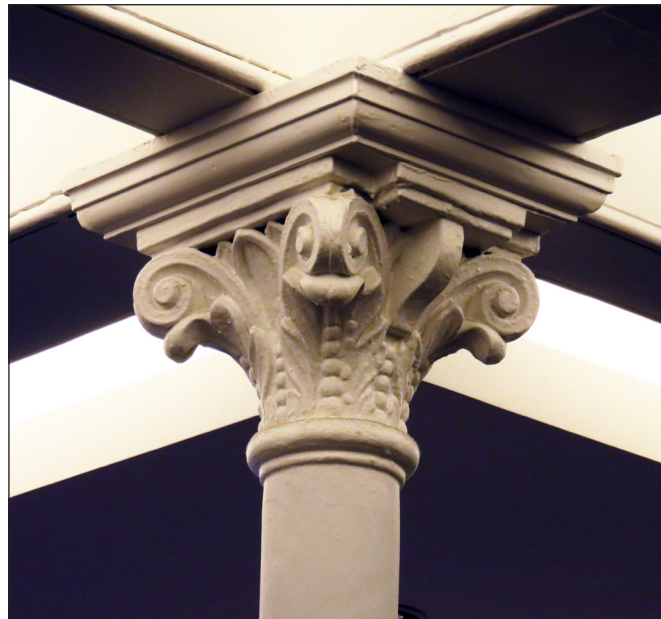
Fig 4. A cast-iron capital surviving from the first-floor gallery of Boots' 1892 shop. The ground-floor capitals (shown in figs 3 and 19) are of slightly different design. (© Historic England, K. Morrison)
