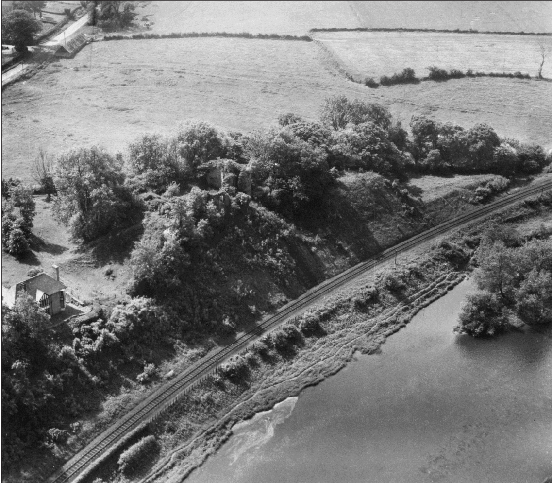
Figure 6 Clifford Castle with the Hereford Hay and Brecon Railway running beneath it along the bank of the Wye June 1947 (AFL/61506 EAW007987 30-JUN-1947)
