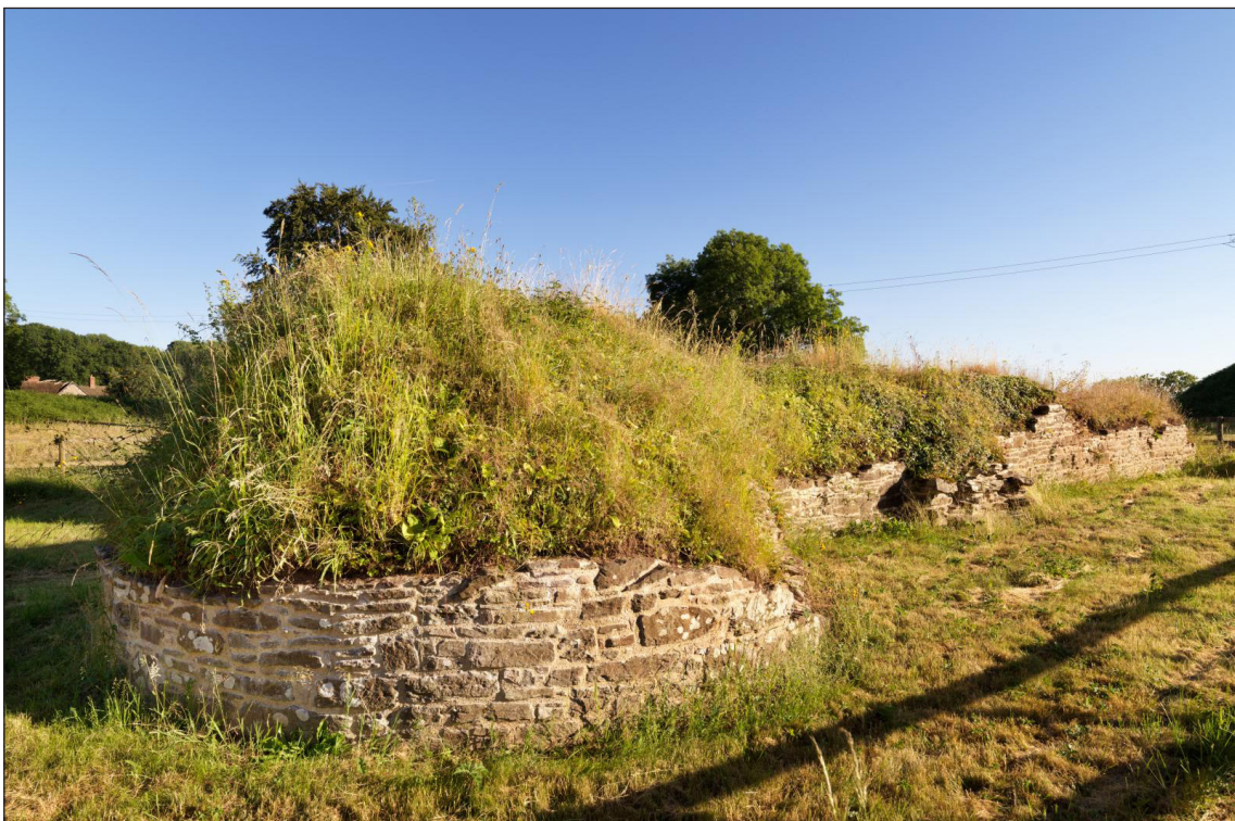
Figure 18 The gatehouse from the northeast, showing the solid drum tower to the east and the long passageway beyond (DP220709)
