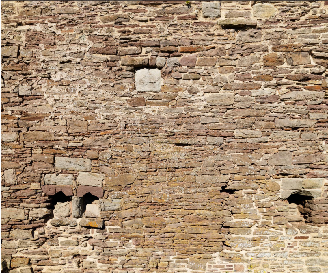
Figure 16 West curtain wall today showing traces of render (DP220701)
