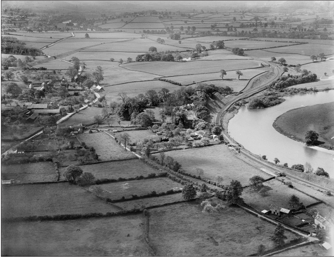
Figure 44 Clifford Castle and village with the Golden Valley railway line at top left and the Hereford, Hay and Brecon Railway on the right. May 1932 (AFL/60803 EAW038176)
