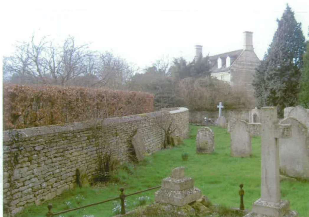
Plate 4: The curving wall on the south side of the church follows the line of the east-north-east section of the Town Street and an earlier, possibly Saxon, enclosure.
