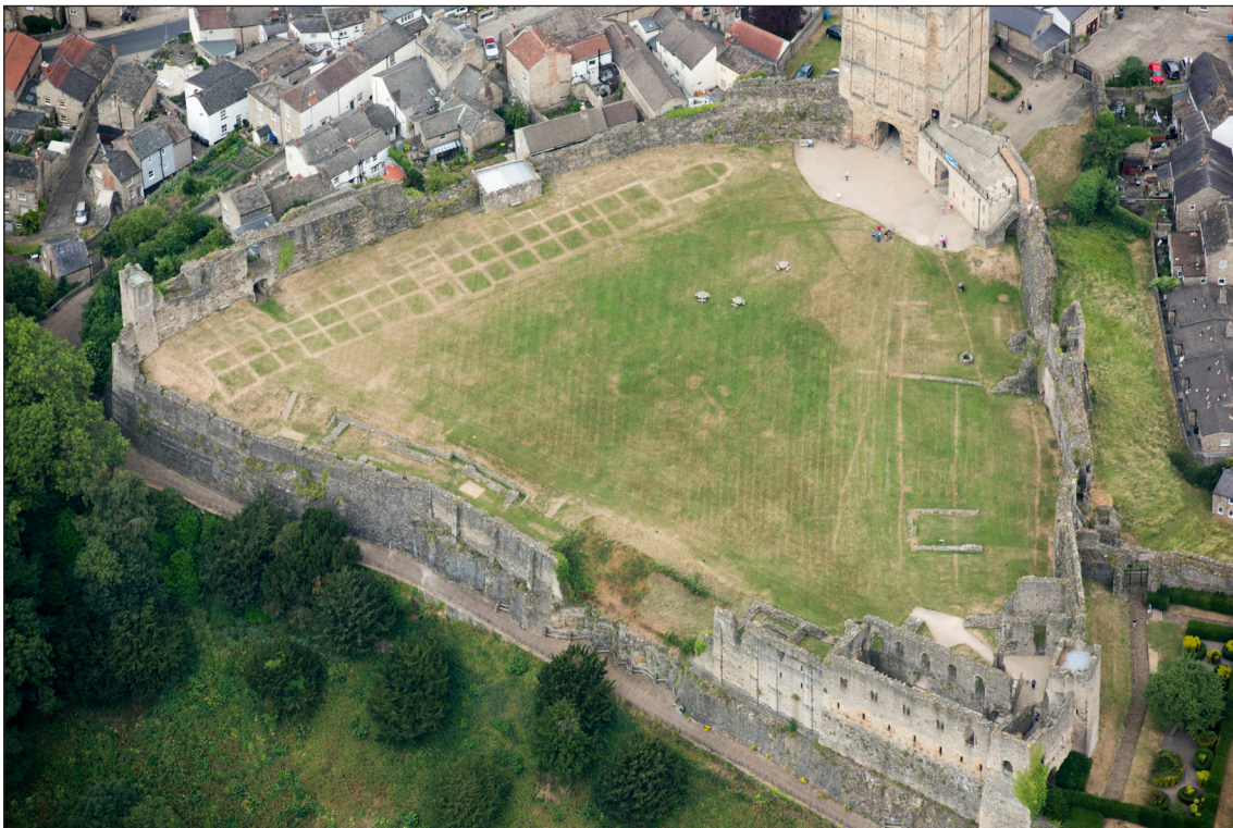
Fig 16: Parchmarks revealed within the castle courtyard during the drought of 2018. Features revealed include the buried remains of the Victorian barrack block. 34050_027 19-JUL-2018 © Historic England Archive.
