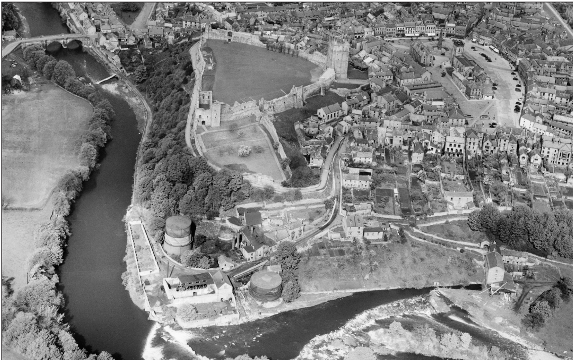
Fig 15: The town gasworks seen in 1947. Church Corn Mill can be seen in the bottom right hand corner of the image. © Historic England Archive. Aerofilms Collection EAW005578 17-MAY-1947 (detail).
