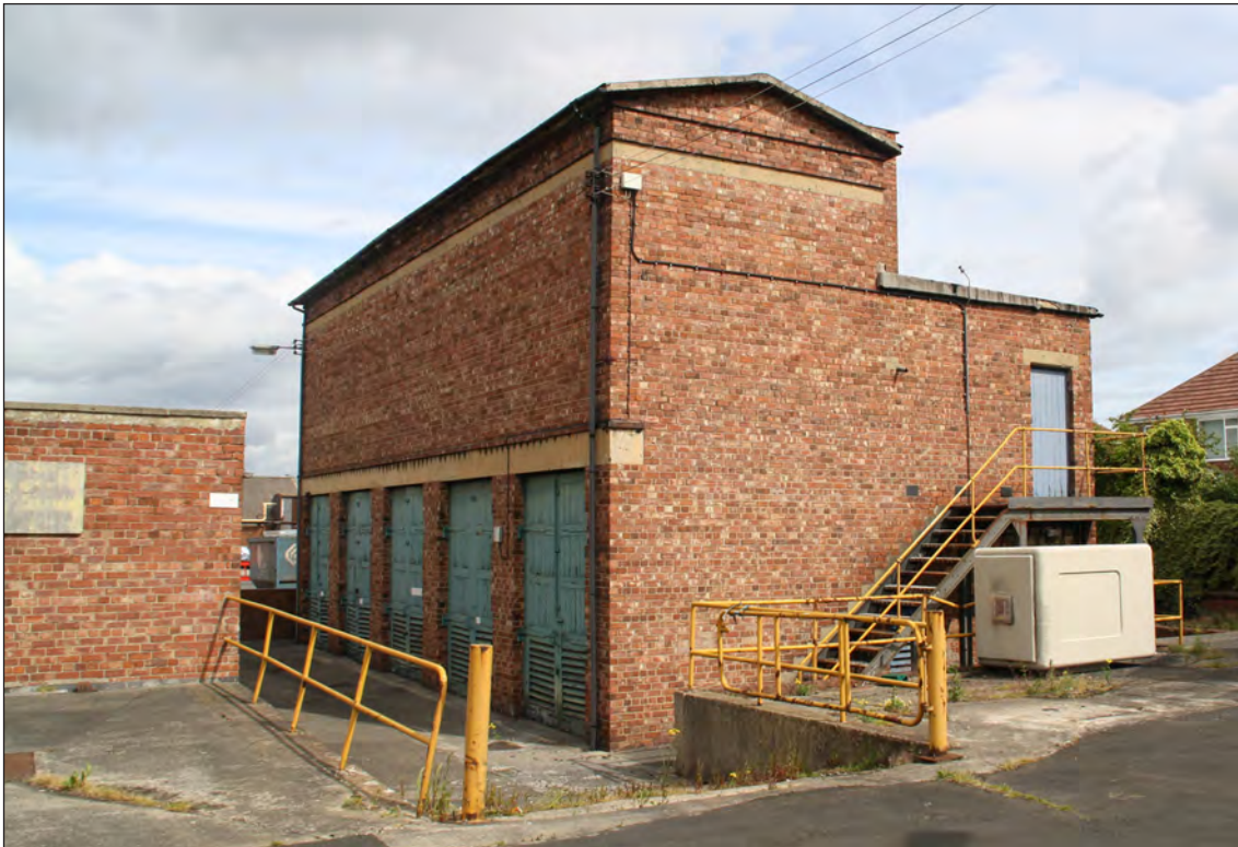
Fig 3.7. NPF Birtley, surviving electricity sub-station (W Cocroft).
