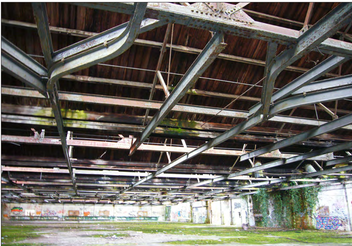
Fig 3.2. NFF Hereford, shell store with a north light roof and a complex pattern of runner beams for overhead cranes (M Bellamy).
