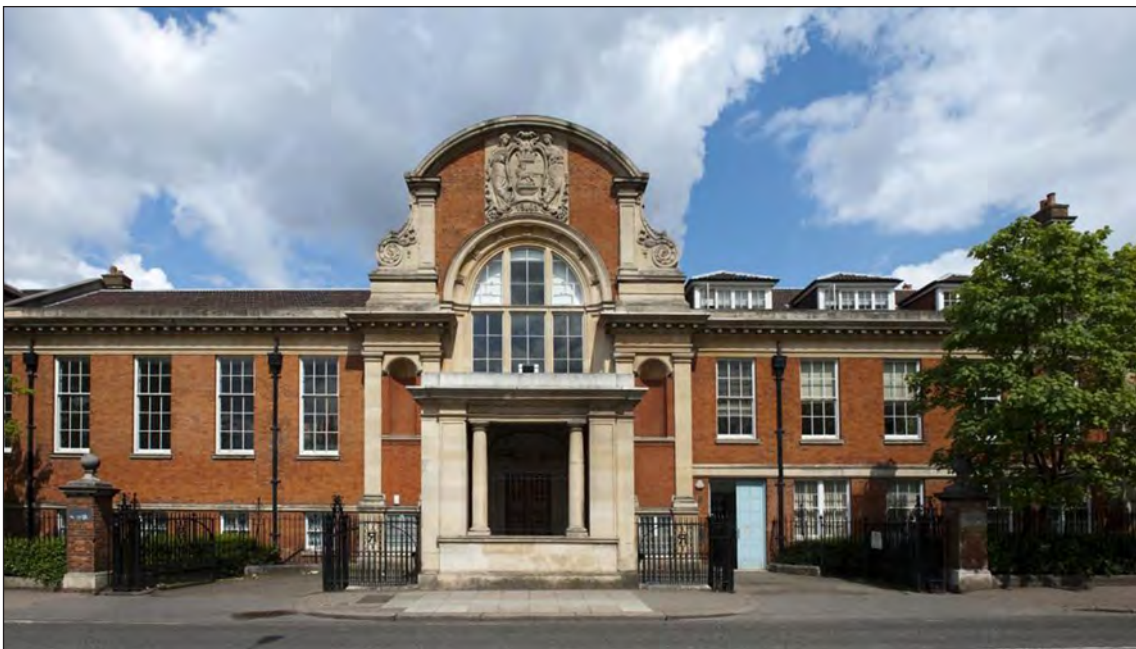
Fig. 4.39. National Aero-Engine Factory Ladbroke Grove (© Historic England DP 096484).
