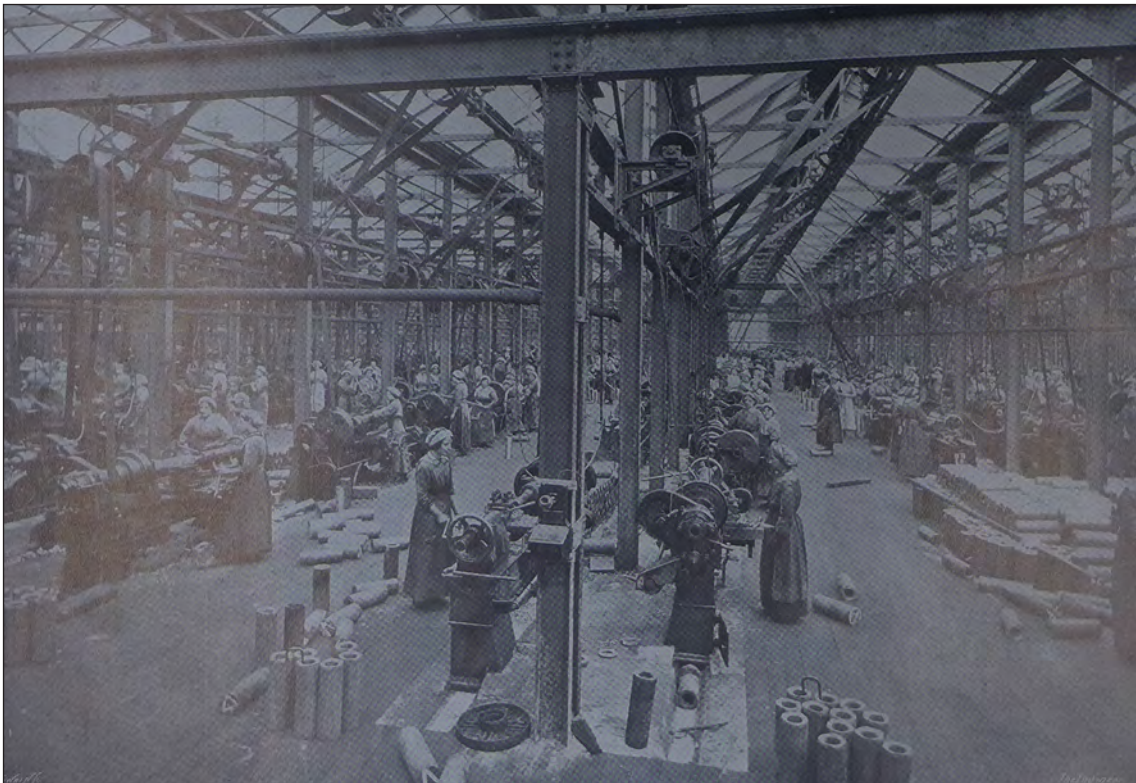
Fig. 4.16. NPF Sheffield (Templeborough), interior showing shell-turning bays in operation, 1916 (TNA MUN5/157).
