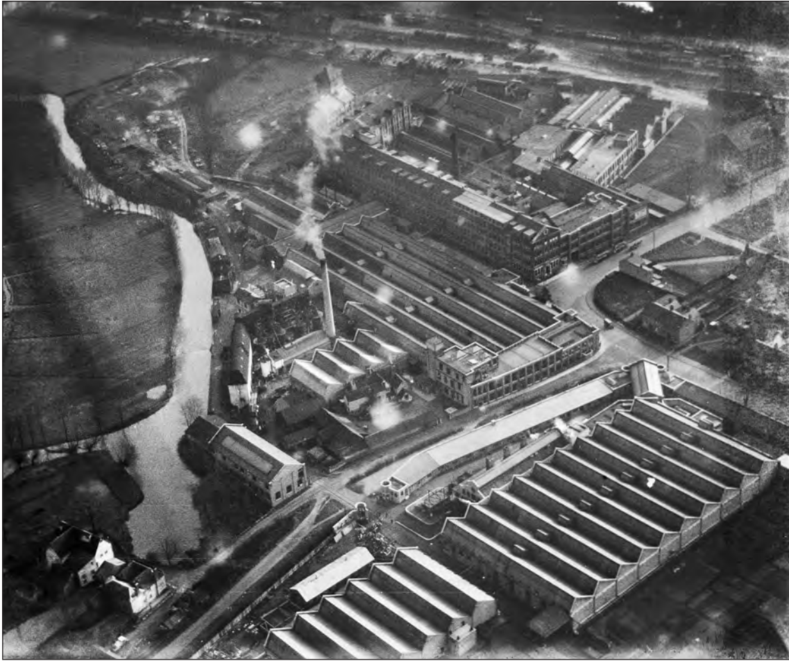
Fig. 4.43. National Ball-Bearing Factory Chelmsford, formerly Hoffman's, air photograph 1923 (© Historic England EPW009600).
