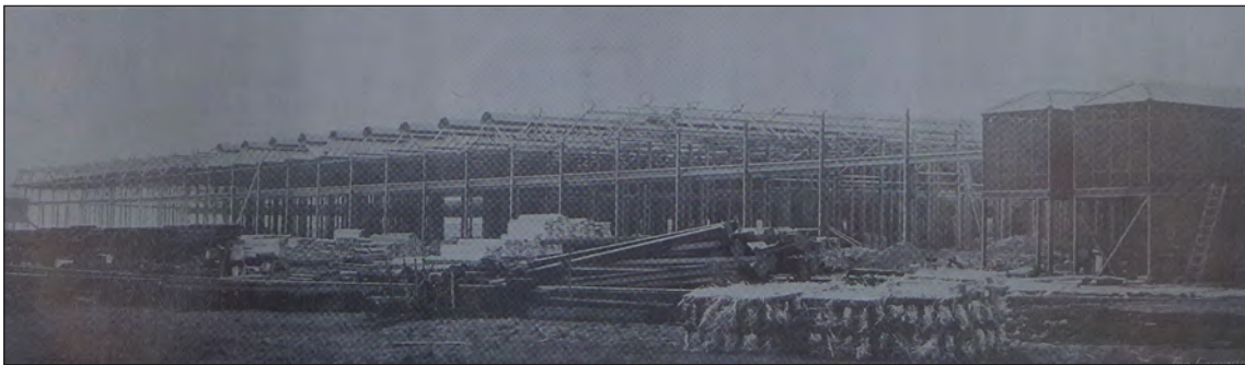
Fig. 3.1. NPF Sheffield (Templeborough) machining shop under construction, 24 November 1915 (TNA MUN5/157).
