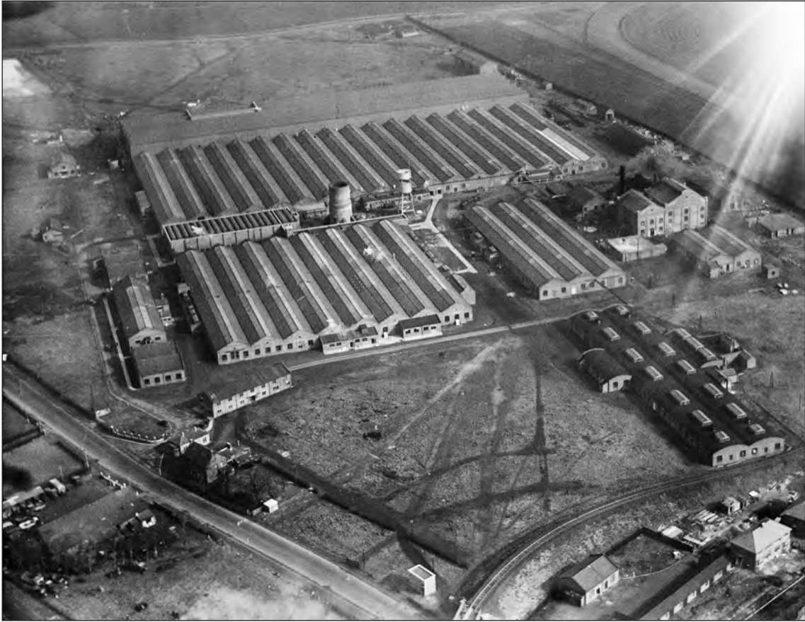
Fig. 4.37. NAF No.3 Aintree, air photograph, 1928 (© Historic England EPW020354).
