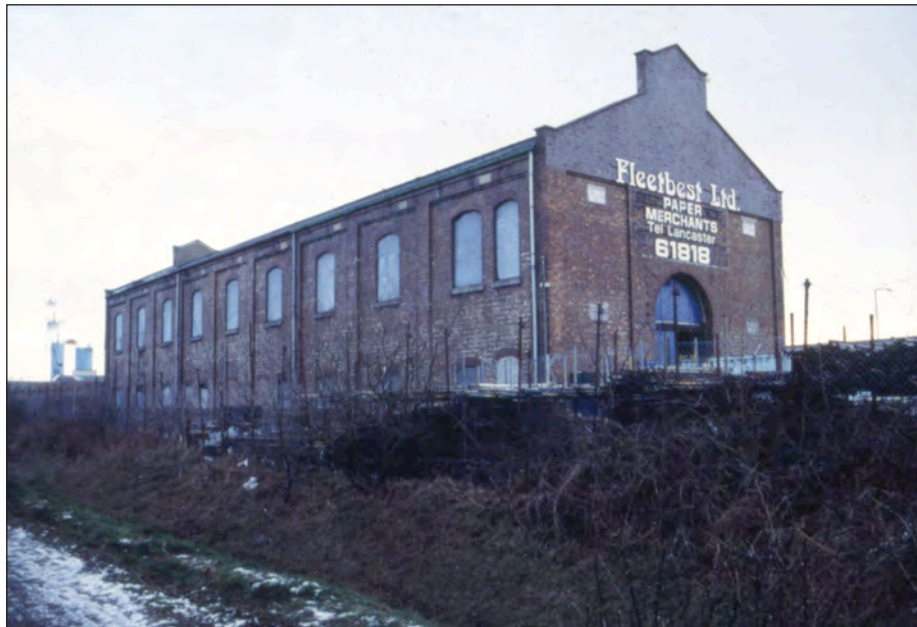
The power house in the 1990s (W Cocroft)
