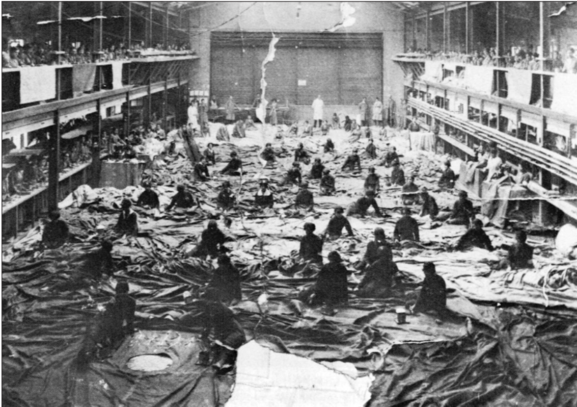
Fig. 4.40. National Balloon Factory Finchley, the interior of the Bohemia Picture Palace in use for balloon manufacture, date unknown (Friern Barnet & District Local History Society).
