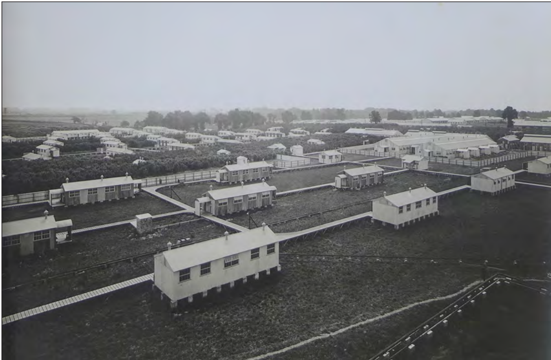
Fig. 4.28. NFF No. 7 Hayes, January 1916, showing layout of huts and clean-ways (TNA MUN5/154).
