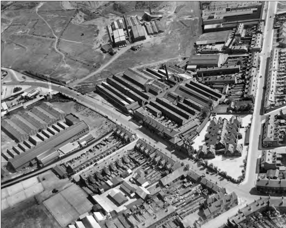
Fig. 4.41. National Radiator Factory Greet, the Motor Radiator Manufacturing Co. works at Greet, Birmingham (later Serck Radiator Co.), air photograph, 1935 (© Historic England EPW048061).
