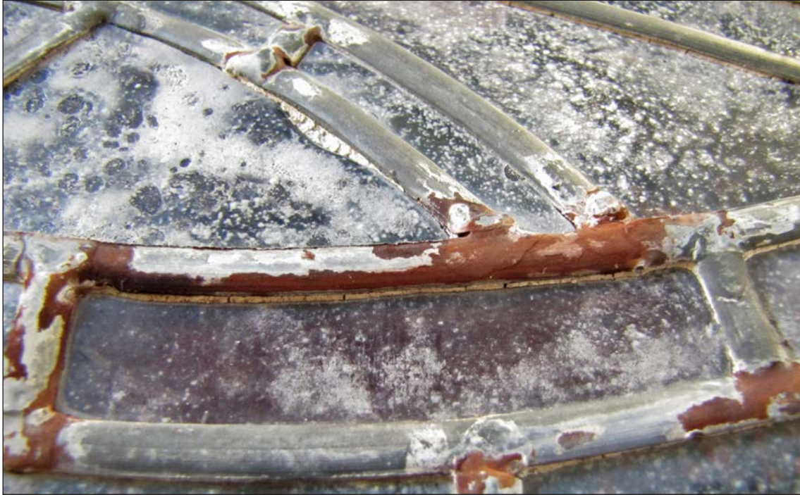
Figure 23. Superficial corrosion and discolouration of the lead came. ©Léonie Seliger
