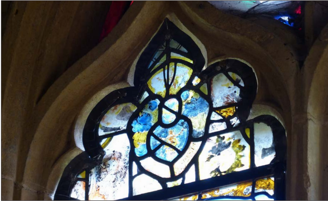
Figure 27. Internal ventilation openings at the top of the east window of St Andrew's Church, Trent, in Dorset.
