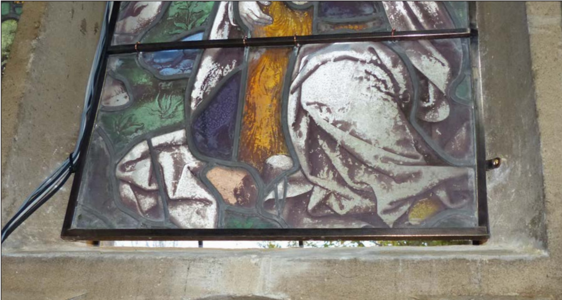
Figures 7, 8. Ventilation openings at the top and bottom of a recently installed internally vented system at the Vyne, Berkshire.
