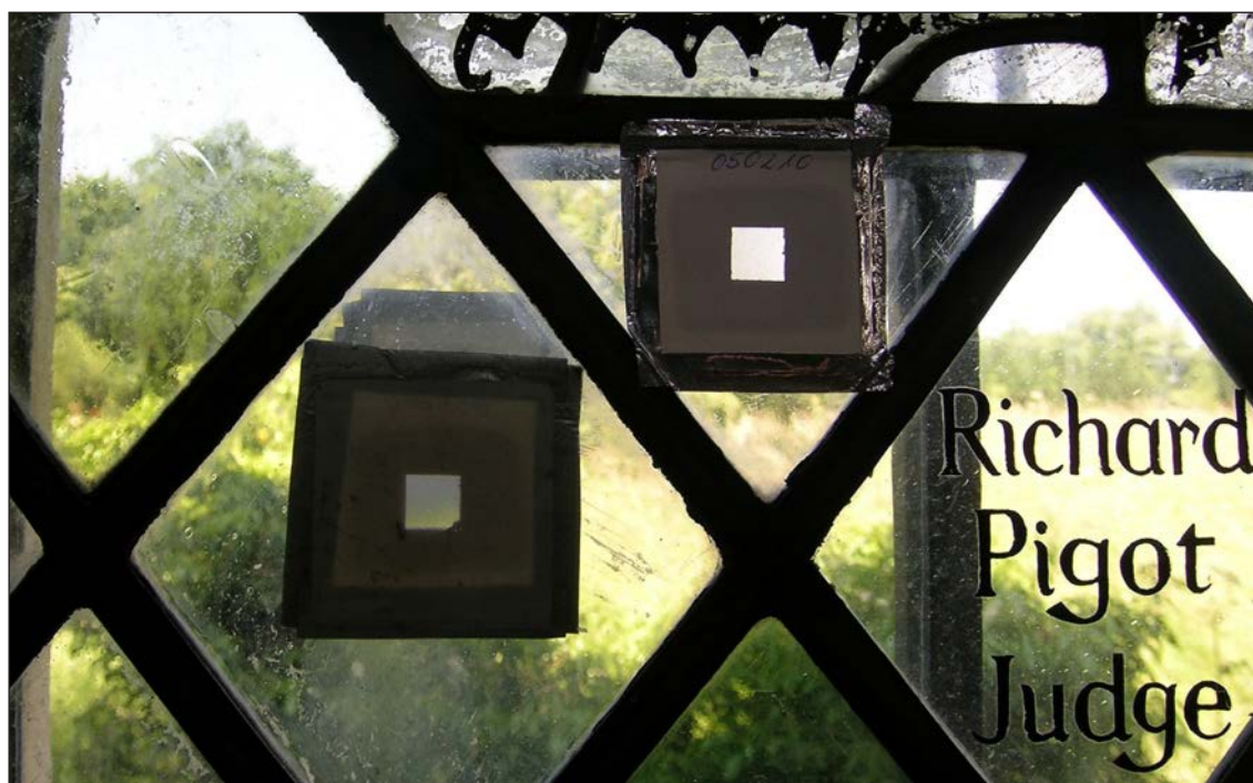
Figure 38. Glass sensors in place on the internal and external faces of the glazing at Holy Trinity Church, Long Melford.
