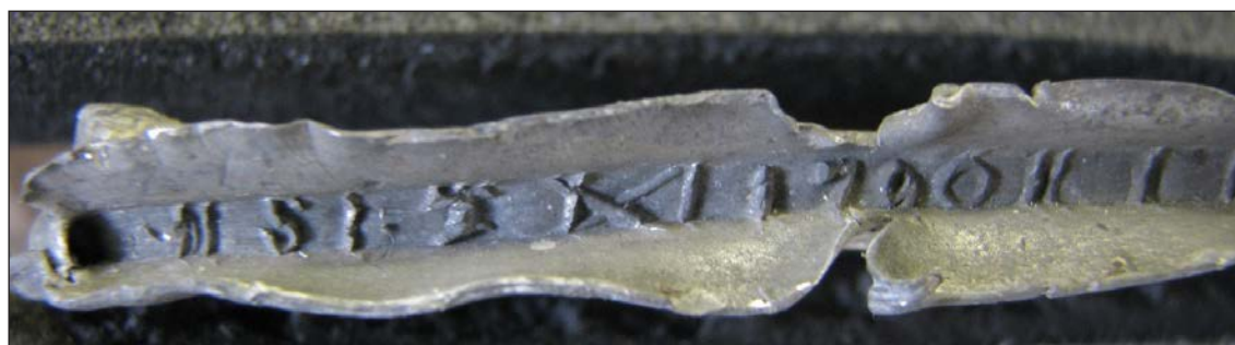
Figures 19, 20. Details of historic lead comes showing milling and makers marks.
