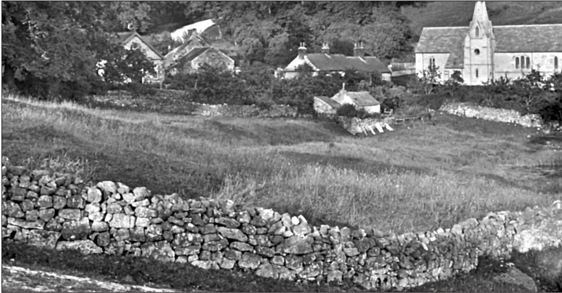
Fig 31. Photograph from the turn of the 20th century showing terraces and enclosures on the west edge of the village below the road to Bow Bridge; source author's collection.
