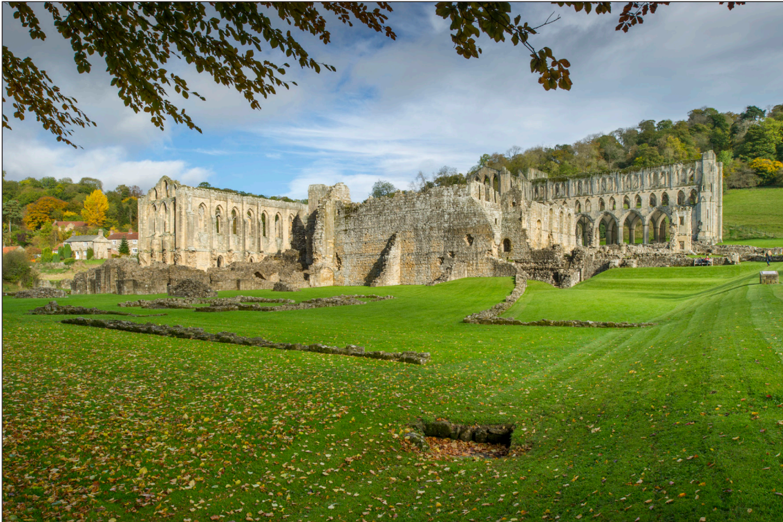
Fig 26. View looking north toward the abbey ruins showing the possible length of the monastic leat (foreground) with foundations of the fulling mill behind. Alun Bull, May 2015. © Historic England Archive, DP169422.
