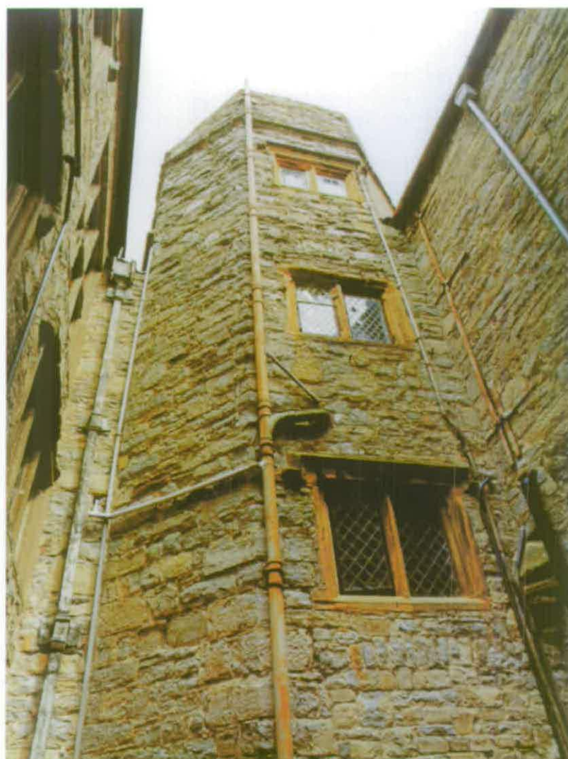
Figure 16. The winder stair tower.
