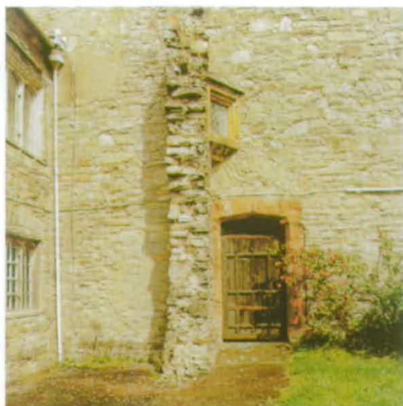
Figure 15. Detail showing corbelled stair light, with Ham Stone surround.
