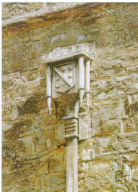
Figure 32. Rainwater spout on the north-east wing, dated 1628.
