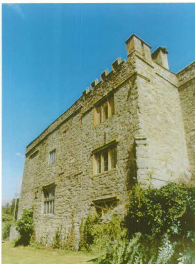
Figure 11. South elevation showing medieval porch tower with crenellated parapet.
