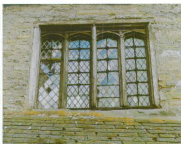
Figure 13. Detail showing wooden-framed window, with four-centred arched heads and king mullion, on the first floor of the north wall.
