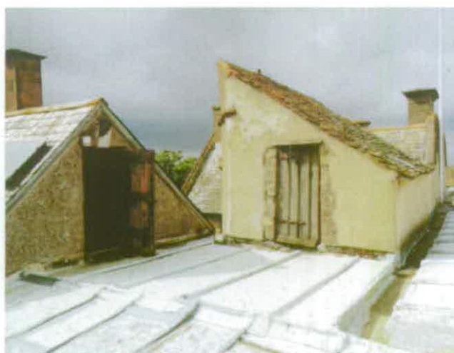
Figure 17. Mono-pitched roof of the winder stair tower.
