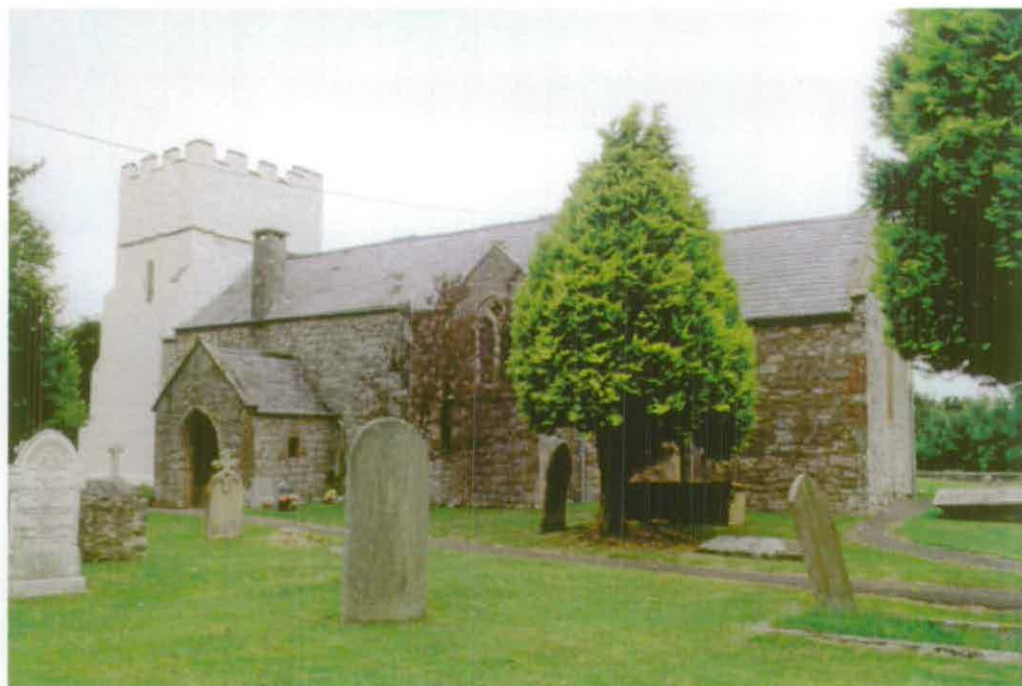
Fig. 11. St. Mary's parish church.
