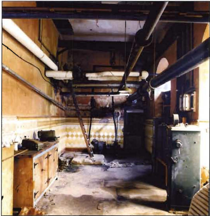
Figure 51. The Finishing Works Engine House. [AA96/00653]
