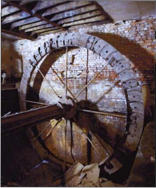
Figure 37. The surviving north shroud of the water wheel. [AA96/00680]
