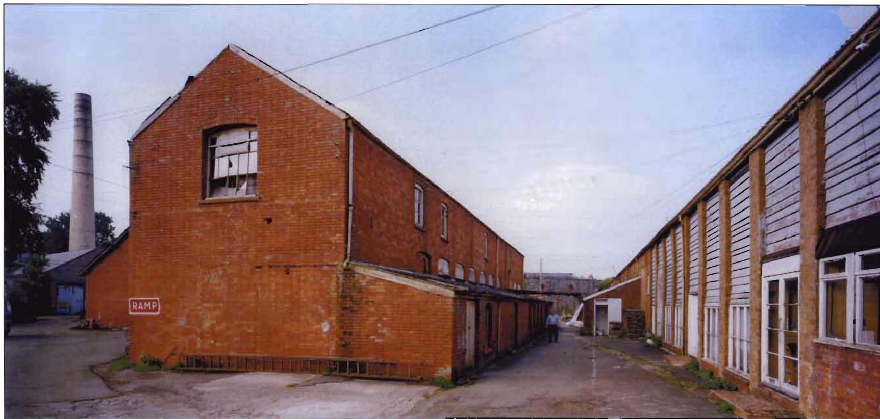
Figure 27. The pier-and-panel extension of the South Dry House (right), and the White Goods building (left). [BB96/01710]
