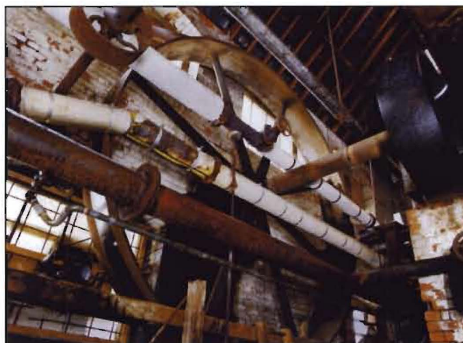
Figure 53. The belt pulley driving the primary line shaft in the Motor Room. [AA96/00677]
