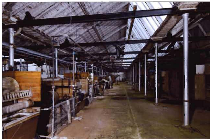
Figure 17. General view from the east end of the Finishing Shed; compare with Figure 12. [DP043932]
