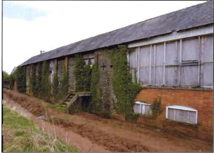
Figure 28. The North Dry House, with in situ ventilation louvers to the left of the rubble wall. [DP046034]
