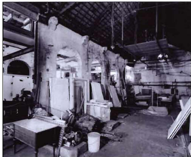
Figure 48. Interior of the 1884-5 Boiler House in 1995. [BB96/01707]
