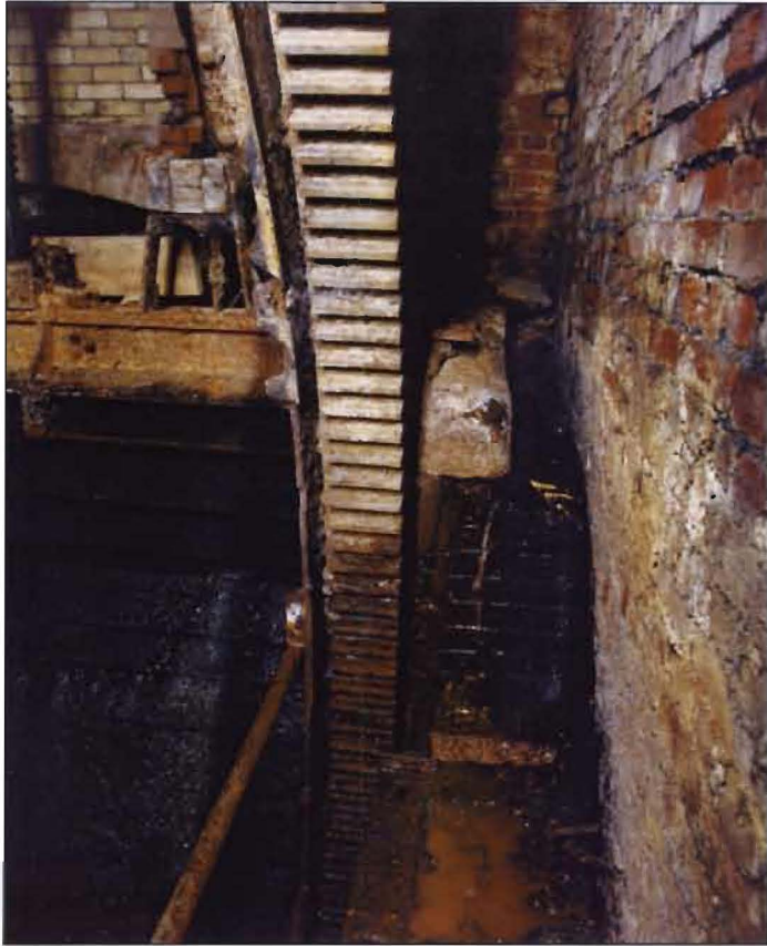
Figure 39. The ring gear added to the north shroud. The base plate of a former pinion shaft bearing remains in situ on the edge of the wheel pit. [AA96/00683]
