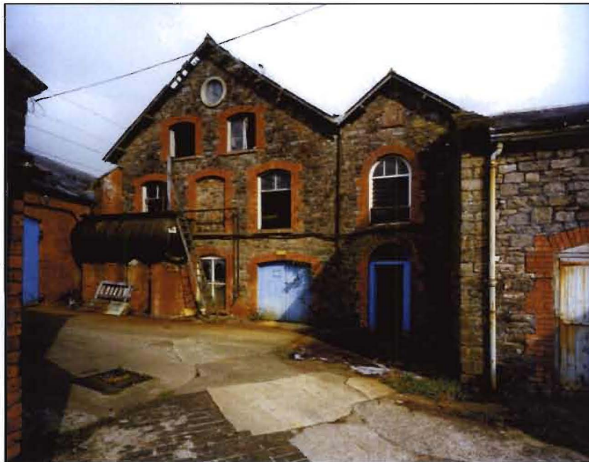
Figure 43. The front elevation of the Dye Works was rebuilt in the late 19th century, but incorporated a re-set 18th-century date stone. [BB96/01702]
