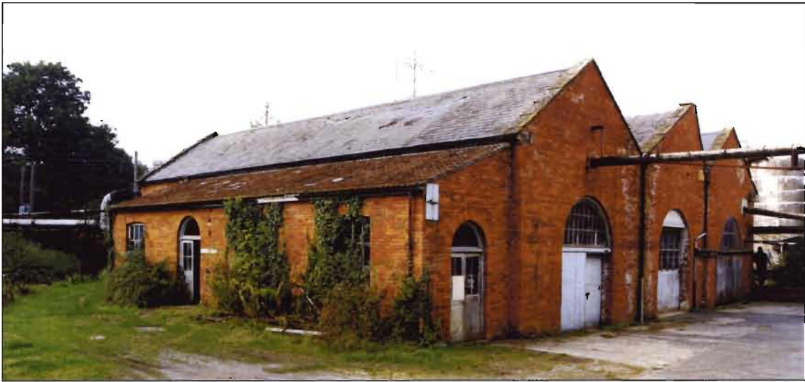
Figure 47. The 1884-5 Boiler House. [AA96/00730]
