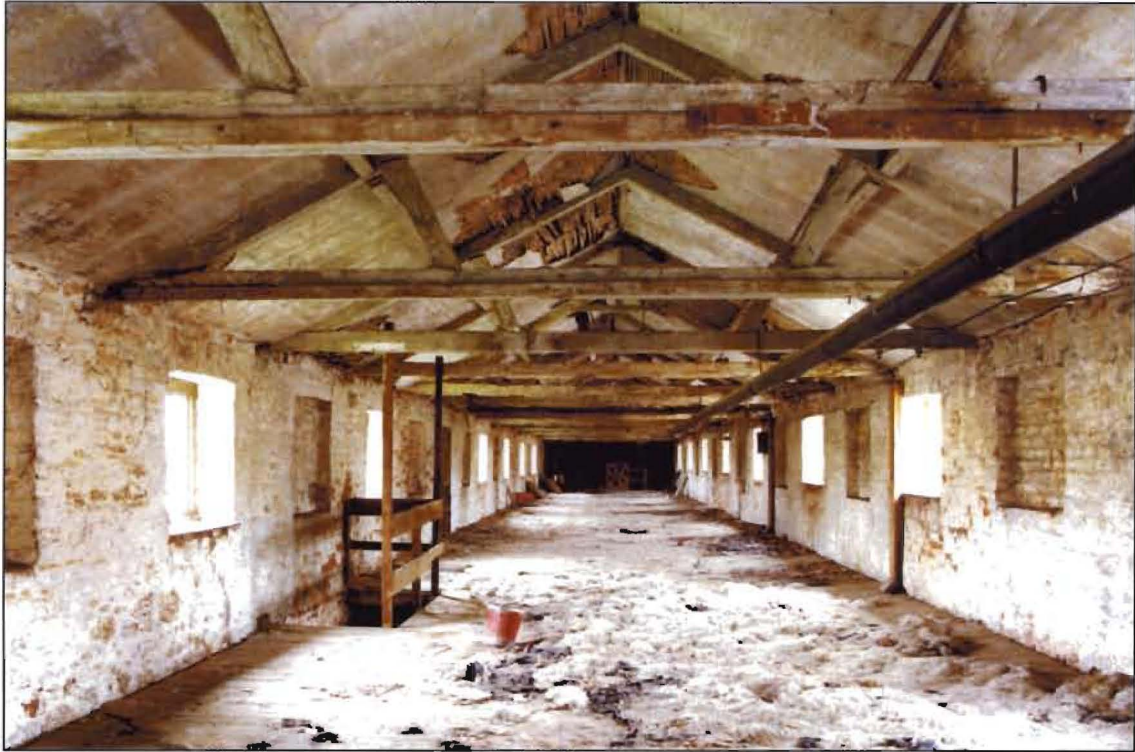
Figure 26. Attic of the South Dry House. [AA96/00720]
