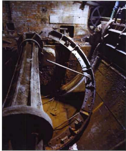
Figure 38. The partially-dismantled middle ring in the wheel pit. [AA96/00684]
