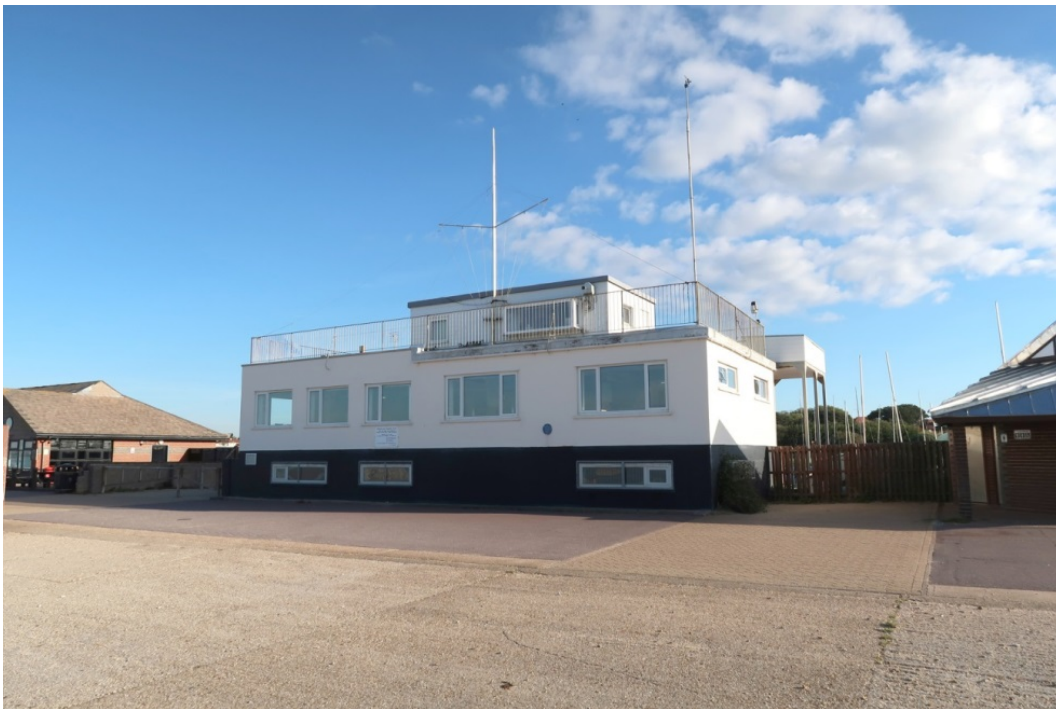
Figure 52. The southern and eastern elevations of the D Day control centre (now Stokes Bay Sailing Club). The western third of this building (to the left of the step in the roof line) is a post war addition (© Historic England).
