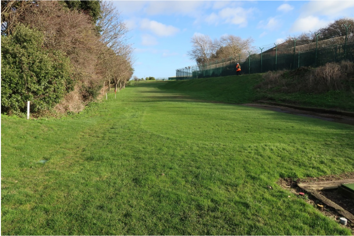
Figure 88. Looking east along Fort Monckton moat (© Historic England).
