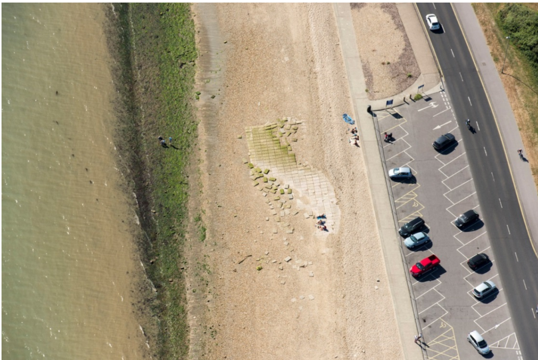
Figure 50. Looking west across the concrete apron (under car park) and concrete matting (exposed on the beach) at Embarkation hard G2 (33562_026 26/06/2018 ©Historic England Archive).
