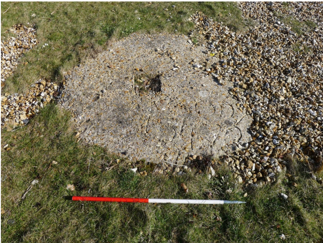
Figure 77. Circular concrete slab with square post hole to west of Fort Gilkicker, scale 1m (© Historic England, photograph Wayne Cocroft).
