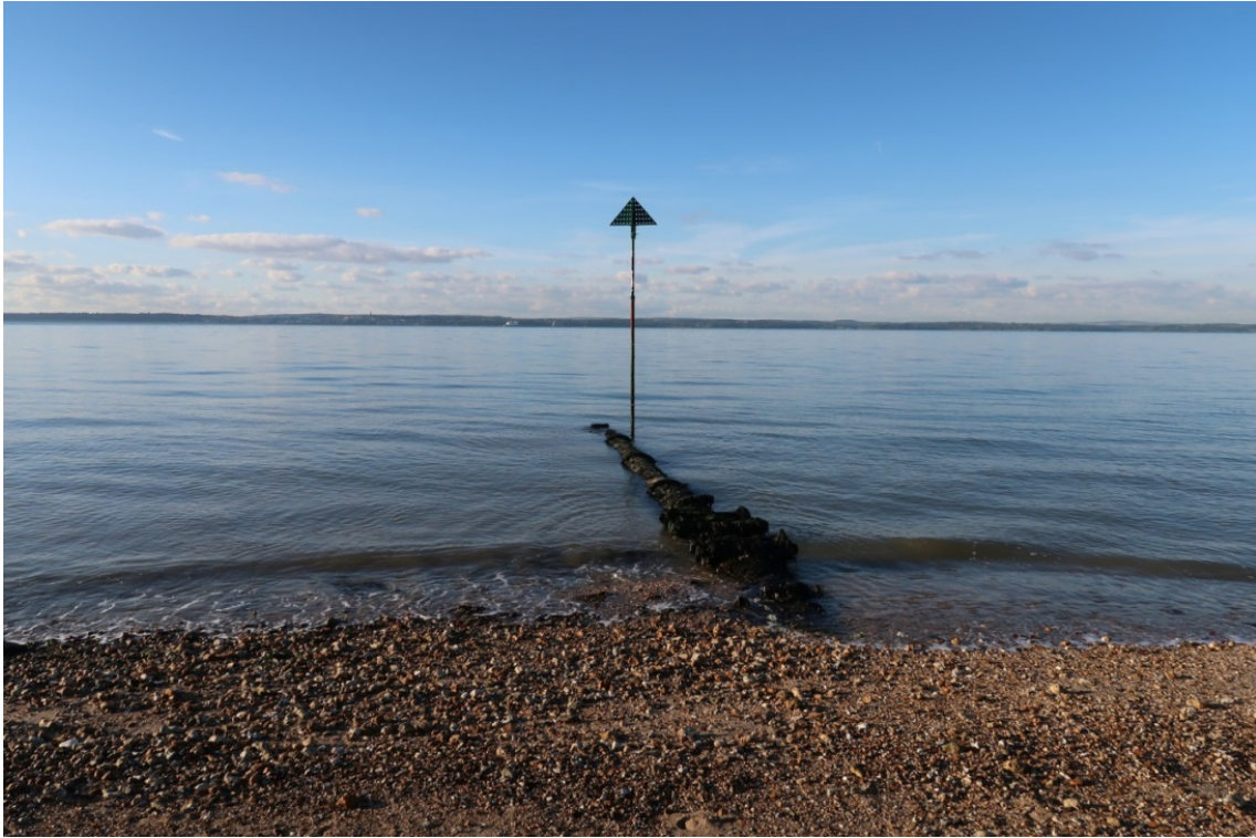
Figure 24. Outfall from the Stokes Bay Lines (© Historic England).
