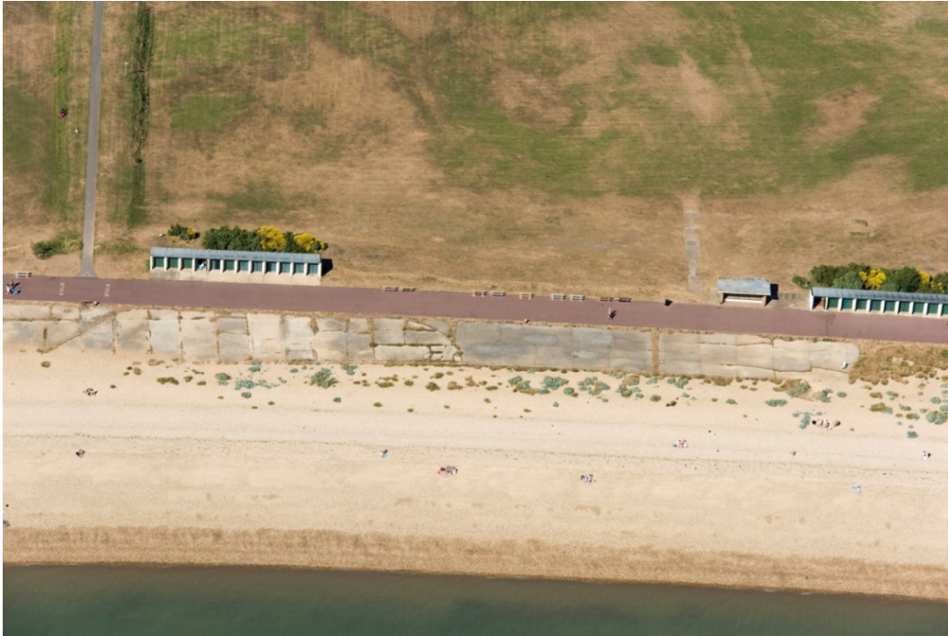
Figure 53. Looking north across embarkation hard G4. The two larger areas of concrete with sweeping landward corners in the centre and right of the image comprise the apron for the hard. The smaller slabs of concrete in the centre and left of the image comprise the south eastern corner of Phoenix caisson construction site 1 (33562_046 26/06/2018 ©Historic England Archive).
