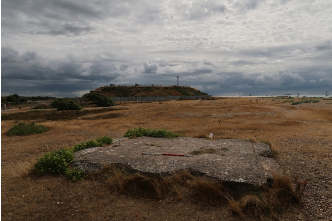
Figure 76. Looking south east towards the concrete base for search light 4 with Fort Gilkicker in the background, scale 1m (© Historic England).
