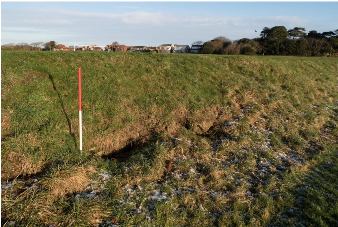
Figure 59. 1950s causeway made from reinforced concrete fragments derived from clearing Phoenix caisson construction sites. Concrete is visible in the face of the embankment, scale 1m (© Historic England).
