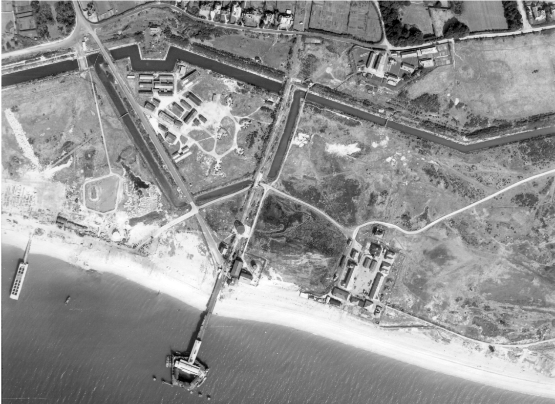
Figure 63. Gilkicker Heavy Anti-Aircraft Battery and its associated hutted encampment in March 1946, framed by the southern protrusion of the Stokes Bay Lines and Batteries 4 and 5. A mooring dolphin associated with embarkation hard G4 and Stokes Bay Pier are visible on the foreshore. Barrage balloon site 2.28 is a circular feature in the top right of the image and the bathing pool is visible on the left of the image and the School of Electrical Lighting and associated tramway is on the right of the image. RAF/106G/UK/1322 V 5037 28-MAR-46, Historic England Archive (RAF Photography).
