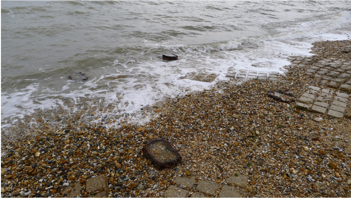
Figure 47. Detail of iron posts associated with embarkation hard G1 (© Historic England, photograph Wayne Cocroft).
