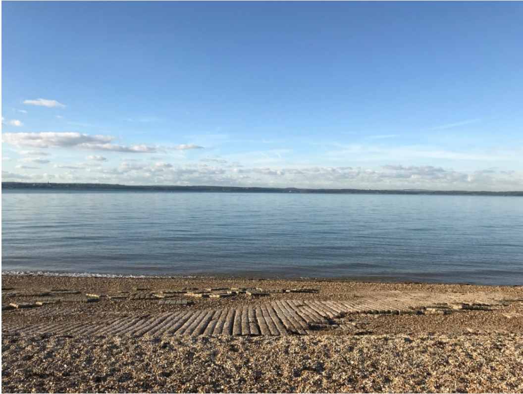
Figure 49. Looking south across 'chocolate block' concrete matting on the foreshore at embarkation hard G2 (© Historic England).
