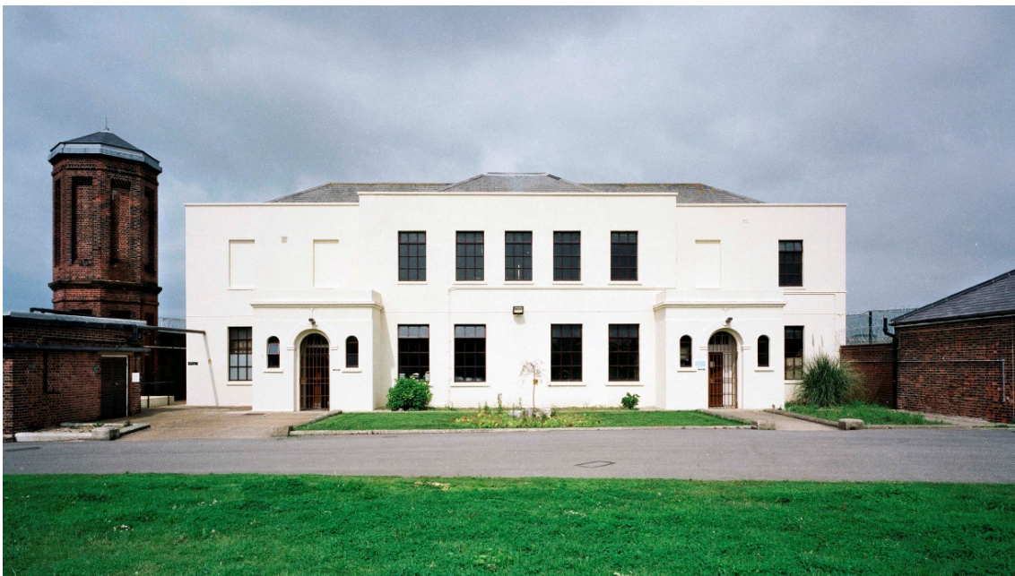
Figure 44. Headquarters building at Haslar Barracks, later the Haslar Immigration Removal Centre. Early to mid 19th century building with later porches, used as Infectious Wards at the end of the 19th century, photographed in 1998. (© Historic England photograph AA98_08858).
