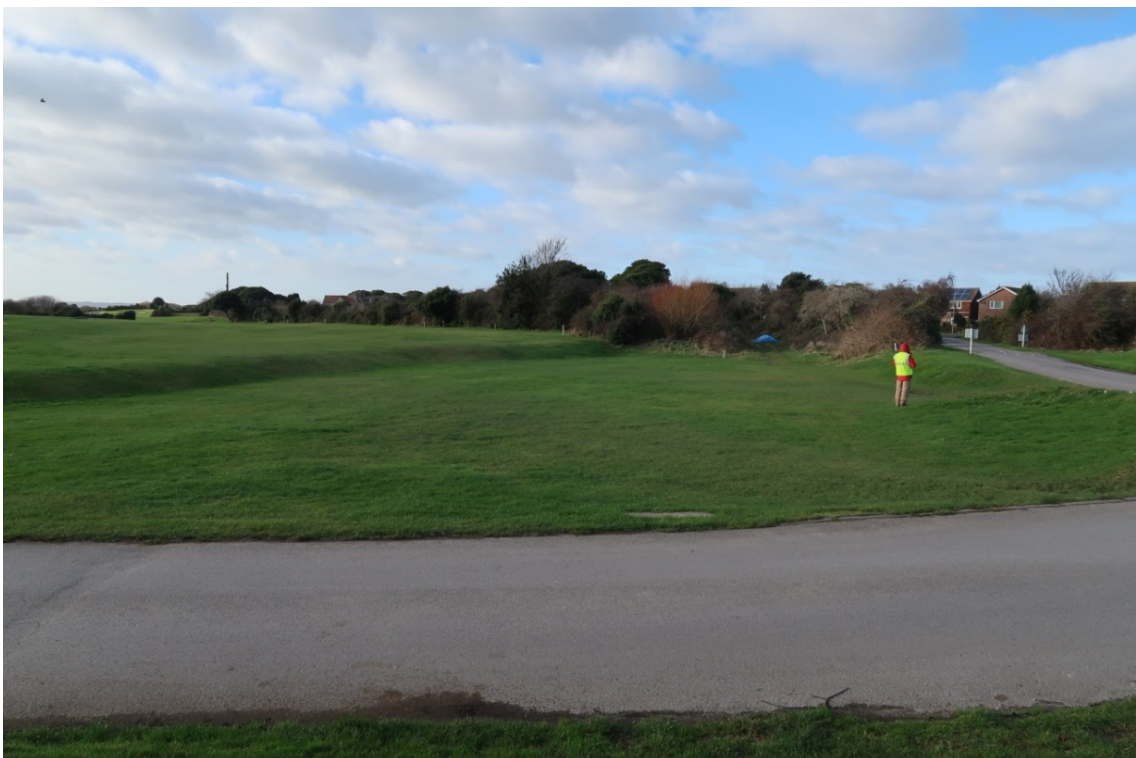
Figure 87. Looking west along the partly infilled line of Fort Monckton moat (© Historic England).
