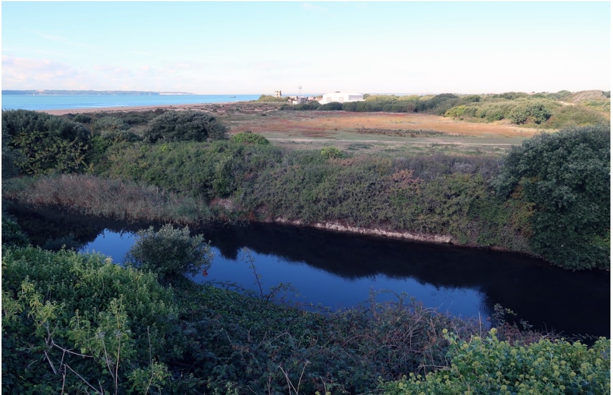
Figure 18. The water-filled and concrete-lined Stokes Bay Lines immediately west of Battery 2 (© Historic England).
