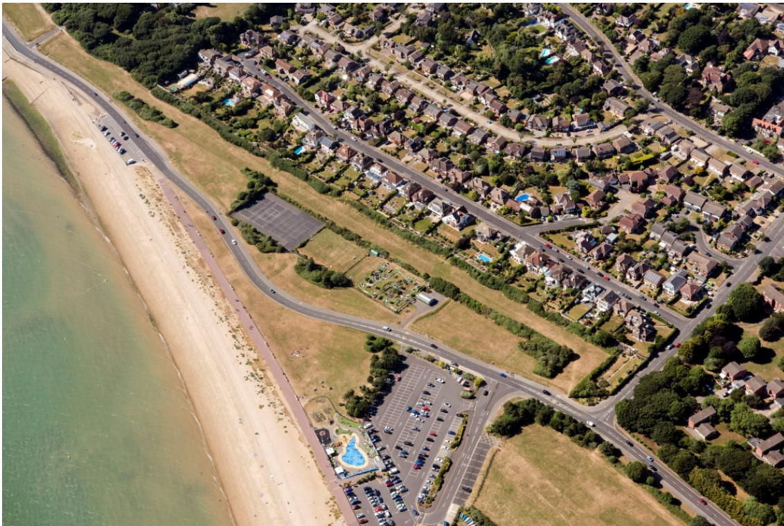
Figure 5. The angled design of the Stokes Bay Lines had a marked influence on later development (33560_027 26/06/2018 © Historic England).
