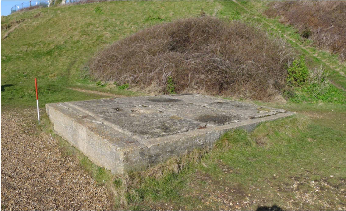
Figure 74. Concrete base for search light position 2, looking west towards Fort Gikicker, scale 1m (© Historic England, photograph Wayne Cocroft).
