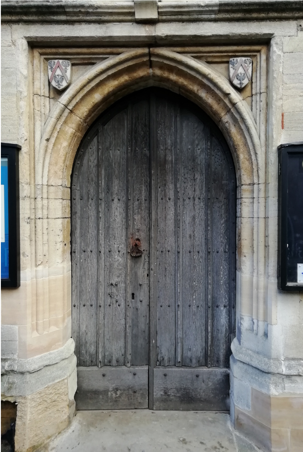
Figure 5: View of the front of the entrance doors, showing the heraldic features in the stonework and general style of the porch, attributed to c AD1485 (photograph Martin Bridge)
