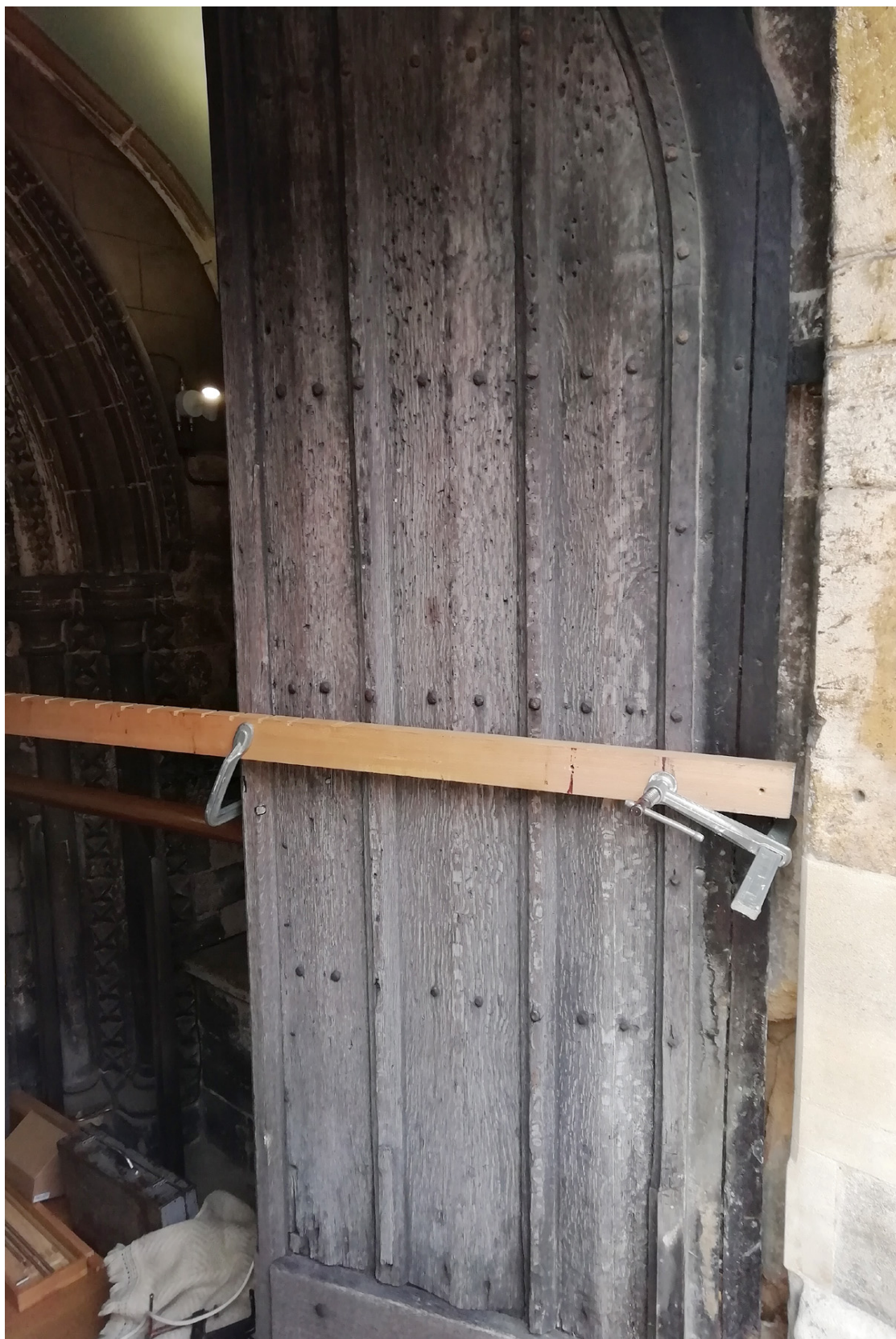
Figure 8: Jig in position on the south-door leaf, prior to coring (photograph Martin Bridge)
