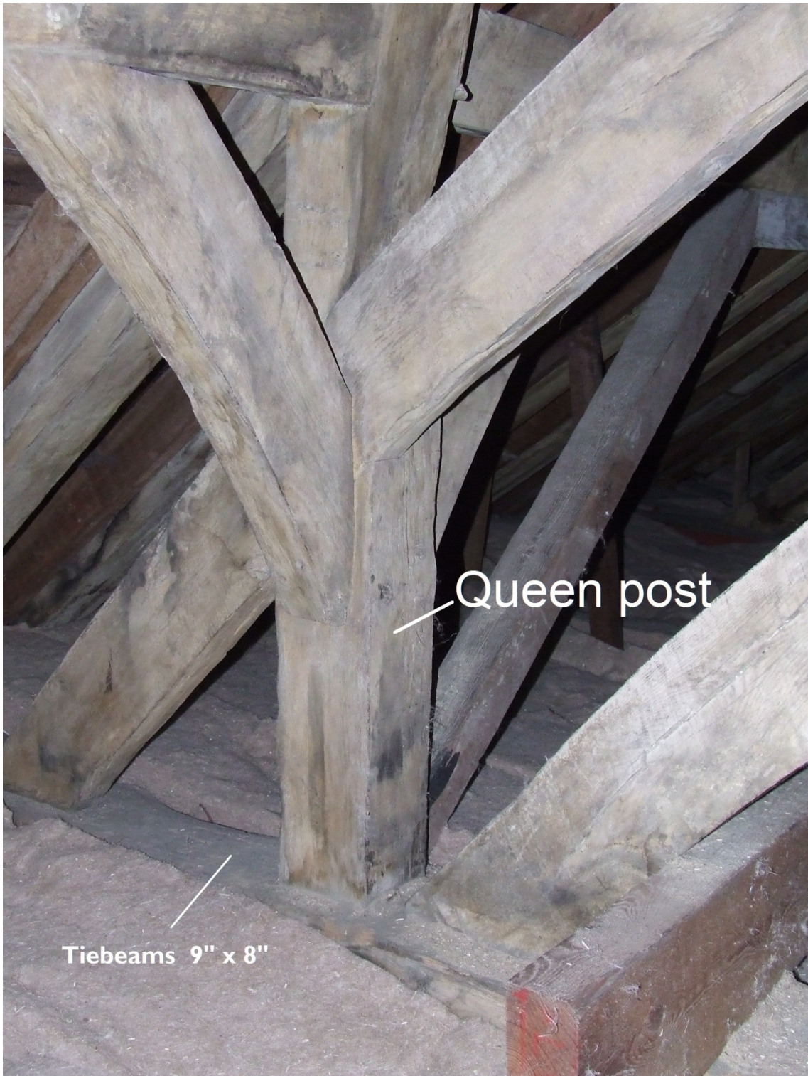
Figure 4: View of a queen post and other truss elements showing the yellow ochre decoration (photograph Martin Bridge)
