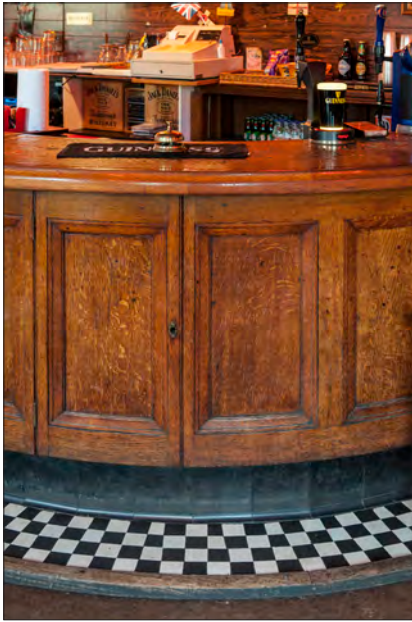
5.48 The counter in the saloon bar of the Palm Tree, Mile End, London (c. 1929), with its chequered tiled border. Such borders helped to protect floors and counters from damage by ash and discarded cigarette ends, and also from floor cleaning. (© Historic England, Derek Kendall, DPI52214)
