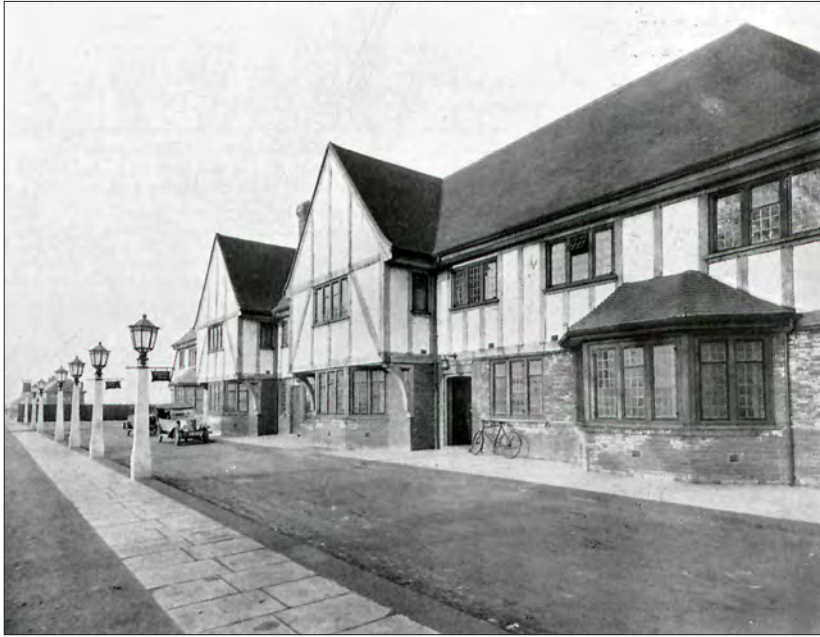
4.7 An image from The House of Whitbread showing the Robin Hood, an improved pub built by Whitbread's on the LCC estate of Becontree, London, in 1926-29, to designs by T. F. Ingram. The building and its gardens (see Fig. 6.12) included a range of facilities, and were consciously designed to attract the whole family. The Robin Hood was demolished in c. 2005; its site is now occupied by a Lidl supermarket.
