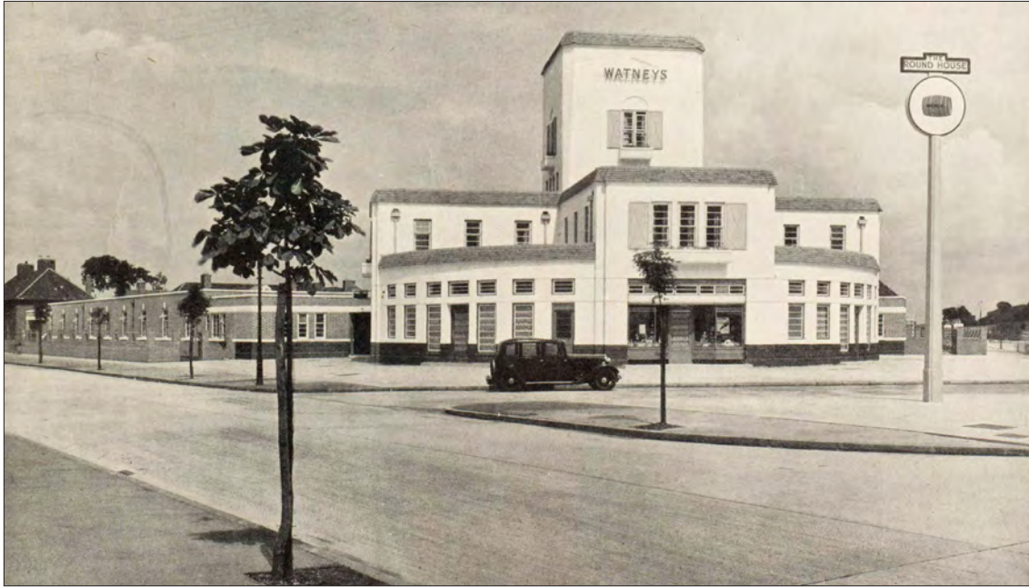
5.16 Another pub of the Moderne style is the Round House, Becontree, London, designed by A. W. Blomfield; it is shown here soon after completion in 1936, in an image published in The Builder . The wing on the left of the main pub building contained a bowling hall, while that on the right contained a children's room. The off licence at the pub's centre has now been removed. The free-standing pub sign does not survive.
