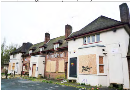
1.2 The Thimblemill pub, Smethwick, Birmingham, built in 1928 to designs by T. Spencer Wood of Wood, Kendrick and Edwin F. Reynolds. The pub was closed and demolished in 2014, to be replaced with a care home. (© Historic England, Emily Cole)
