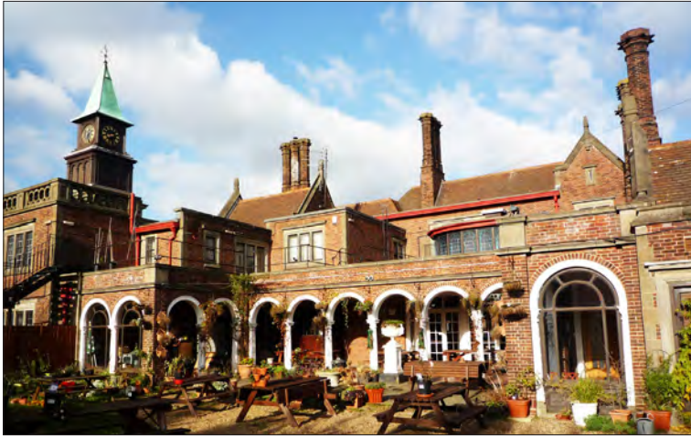
10.5 Some listed pubs are notable in terms of their quality of architecture and design, an example being the Suffolk Punch, Ipswich, Suffolk (1936-37, by Cautley & Barefoot for the Tollemache Brewery; listed grade II). This photograph shows the pub's rear elevation and garden. (© Historic England, Emily Cole)
