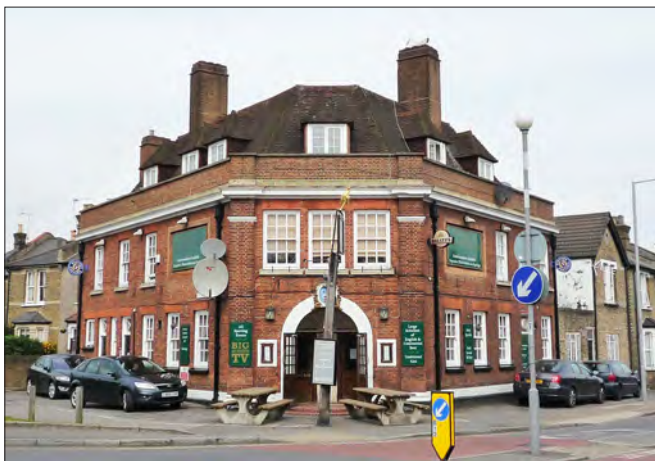
7.1 The Duke of Buckingham, Kingston-upon-Thames, London. The pub was built by Hodgson's Kingston Brewery in 1932 to designs by Joseph Hill. Hill was a noted and active pub architect in the inter-war years, though many of his buildings have subsequently been much altered. (© Historic England, Luke Jacob)
