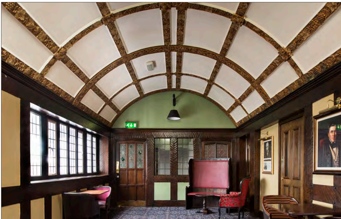
5.35 The first-floor anteroom at the Black Horse, Northfield, Birmingham (1929, by Francis Goldsbrough), adjacent to the assembly room, looking towards the stair head. Such spaces helped to ease the quick and safe dispersal of crowds. (© Historic England, James O. Davies, DPI66432)
