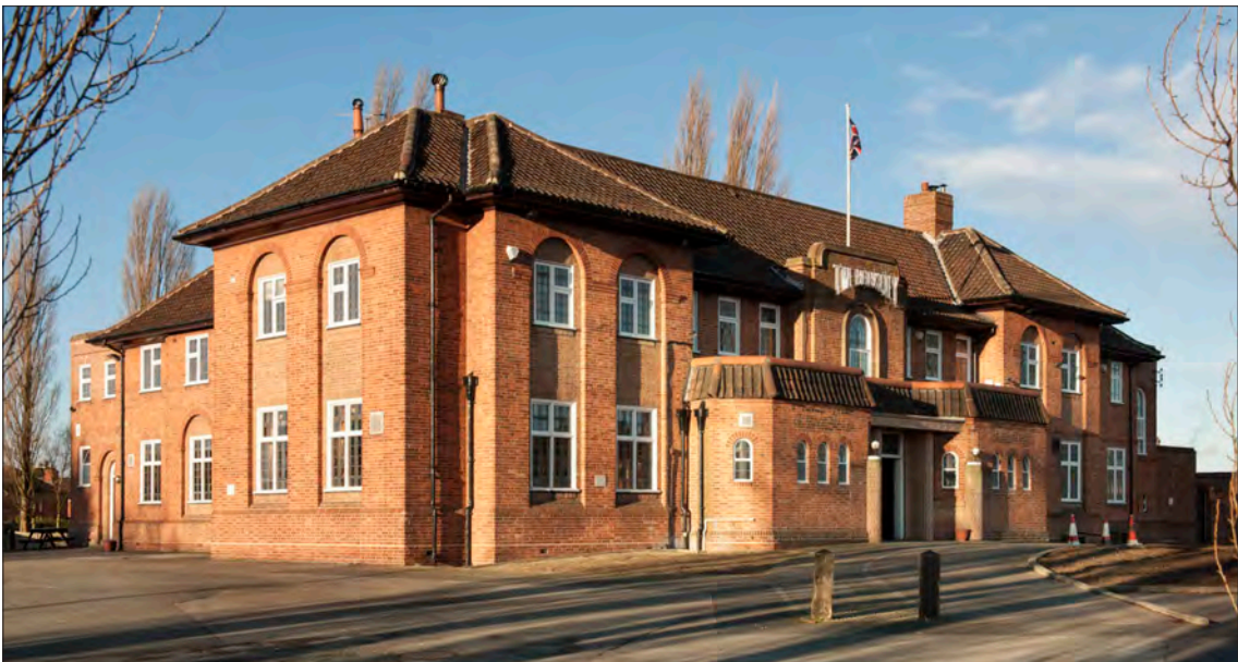
6.3 The car park at the Berkeley Hotel, Scunthorpe, Lincolnshire (1938-40, by Scott and Clark), extends around the front and south-west sides of the building. This enabled customers to park adjacent to the areas of the pub they wished to use. The doorways on the left elevation, for instance, led to the public bar and the off sales compartment. (© Historic England, Derek Kendall, DPI52414)
