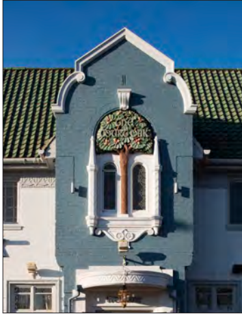
5.18 A detail of the main façade of the Court Oak, Quinton, Birmingham (1932), showing the carved pub sign and the original green pantiles. The sign is probably the work of William Bloye or one of the sculptors in his circle. (© Historic England, James O. Davies, DPI66395)
