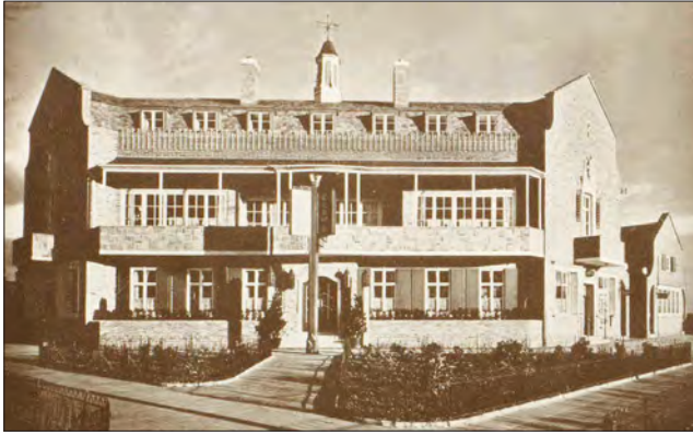
7.5 A photograph published in Architecture Illustrated in 1933 showing the Crown Hotel, Walton, Liverpool, built in c. 1932 to designs by the acclaimed firm Harold E. Davies & Son. The pub, more recently known as Dickie Lewis's, closed in c. 2006, and was demolished after a period of dereliction and following damage by fire.
