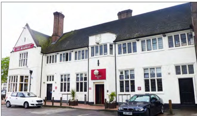
1.5 The Wernley pub, Sandwell, Birmingham, was listed grade II in 2014 as a result of an English Heritage survey of inter-war pubs in the area. It was built in the Jacobean style in 1933-34 to designs by Edwin F. Reynolds. (© Historic England, Luke Jacob)
