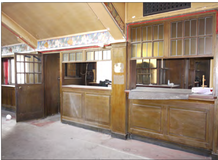
5.25 Counters in pubs built under the state management scheme in the Carlisle district were often of limited size and divided from the bar area by glazed screening. This was the case, for instance, with the first-floor rooms of the Apple Tree in central Carlisle (1927, by Harry Redfern; listed grade II). Shown here is the counter of the first-floor room reserved for 'men 1st class'. (© Historic England, Clare Howard)
