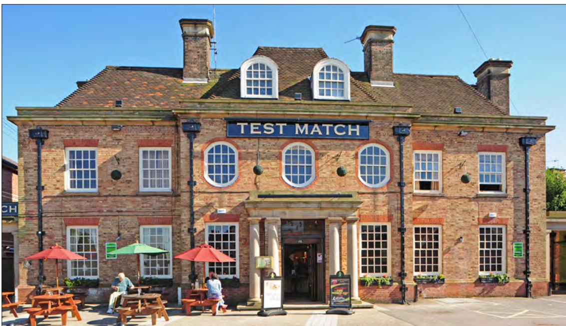
10.6-10.8 A particularly high level of preservation is reflected in the grade II*-listing of three inter-war pubs: the Margaret Catchpole, Ipswich, Suffolk (1936); the Eastbrook, Dagenham, London (1937-38; shown here is the vestibule to the music room); and the Test Match, West Bridgford, Nottinghamshire (1938). (all images © Michael Slaughter LRPS)
