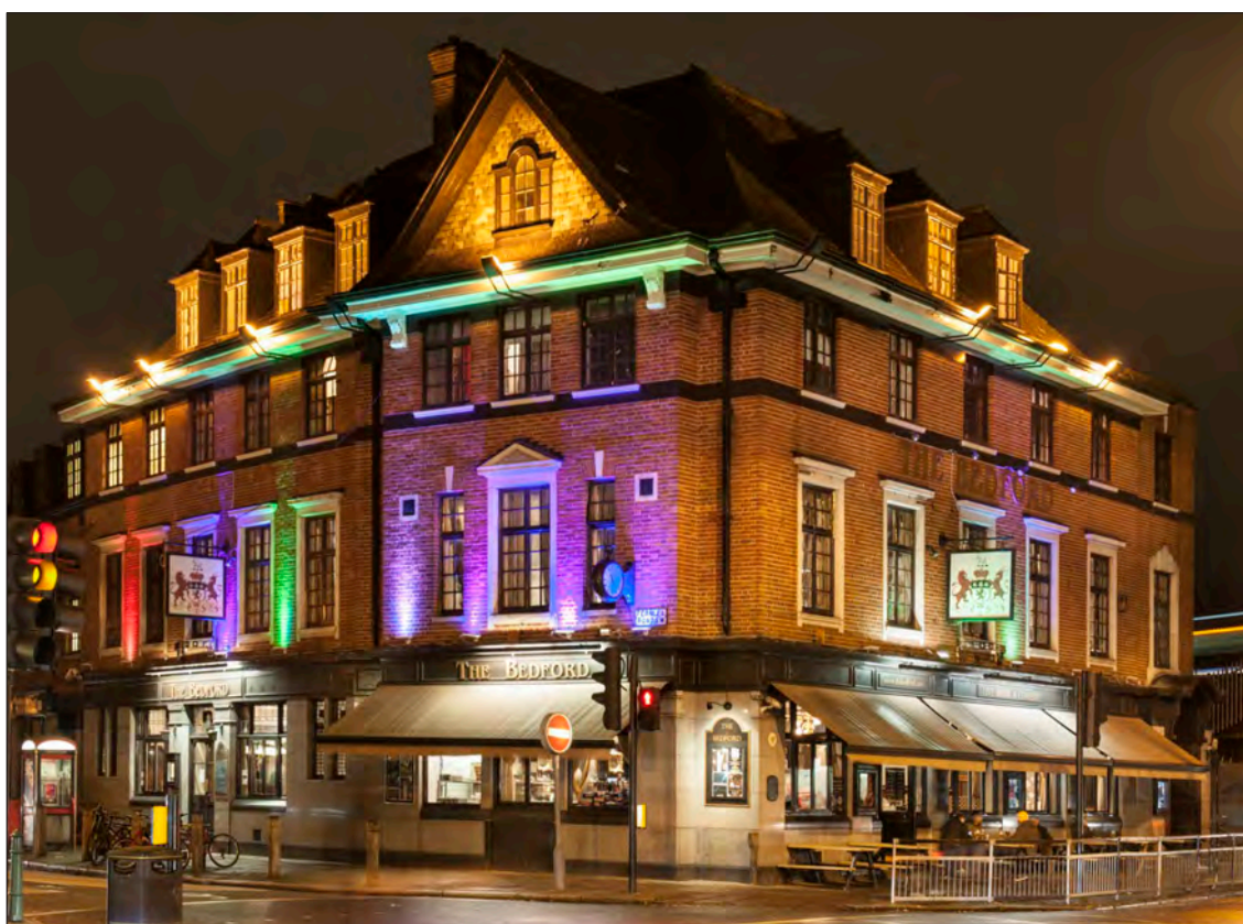
7.8 The most active brewery in terms of building projects undertaken during the inter-war period was Watney, Combe & Reid of London. Their works included the Bedford Hotel, Balham (c. 1931, by A. W. Blomfield), shown here at night-time. The building tender for the pub totalled £30,000. (© Historic England, Derek Kendall, DPI52236)
