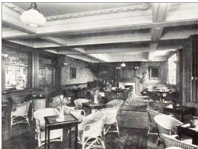
4.4 The interior of the saloon lounge at the rebuilt Green Man, Southend village, Catford, London, as featured in Building. The image shows the scale and sophistication of the new pub of 1927. Lounges were an innovation of inter-war pub planning, provided with the aim of attracting a respectable and more mixed class of clientele.
