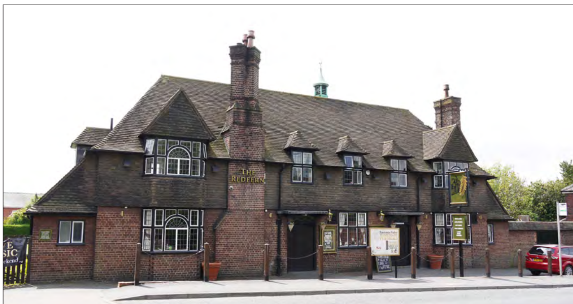
3.9 The Redfern Inn, Etterby (1939-40; listed grade II), is the only new 'model' pub built in the Carlisle area during the inter-war years that was not designed by Harry Redfern. It was the work of Redfern's assistant, Joseph Seddon. (© Historic England, Clare Howard)
