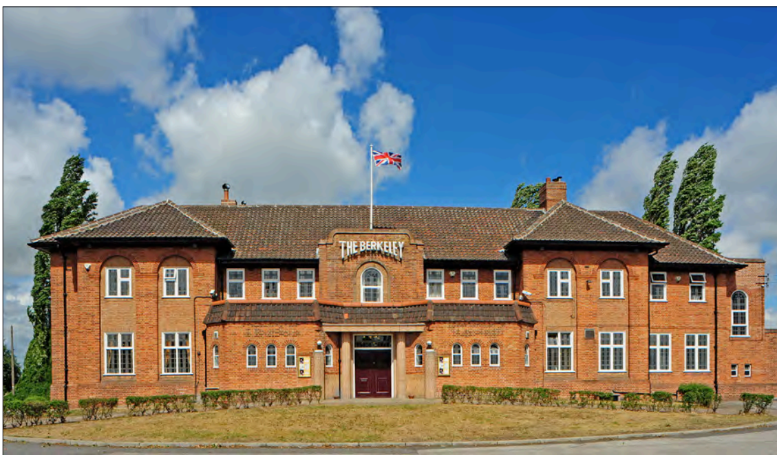
5.4 The Berkeley Hotel, Scunthorpe, Lincolnshire (1938-40, by Scott and Clark), is a classic example of the large, restrained pubs that were built in the inter-war period, especially in the 1930s. In style, it is broadly Neo-Georgian. (© Michael Slaughter LRPS)
