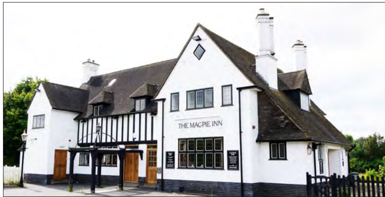
3.6 Another Carlisle pub built to Harry Redfern's designs was the Magpie Inn, Botcherby, of 1933 (listed grade II). The pub was closed in 2014 but is in good repair. (© Historic England, Clare Howard)
