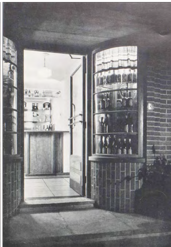
5.43 The display windows at the Nag's Head, Bishops Stortford, Hertfordshire (1936, by E. B. Musman; listed grade II), in a photograph published in the Architectural Review in 1936. The doorway led into the off sales compartment. It is now the main entrance to the pub, which has been altered in its planning.
