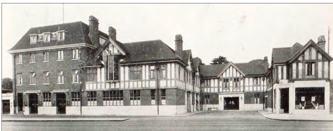
4.3 The Green Man, Southend village, Catford, London, following rebuilding, as illustrated in Building. The new pub, completed in 1927 for Watney's, was of a substantial size; it was designed by Grace & Grace & Farmer, with M. T. Saunders. The four-storey block on the left contained public and private bars on the ground floor, kitchen on the first floor, and staff accommodation on the two upper floors. The saloon bar, saloon lounge, assembly hall and other higher-class rooms were in the pub's timbered section, while a block on the right contained an off licence.
