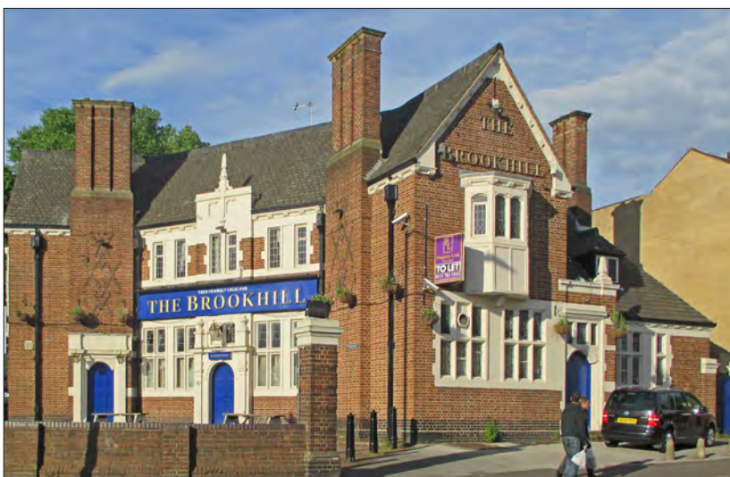
2.8 The Brookhill Tavern, Alum Rock, Birmingham, a Mitchells & Butlers pub of 1927-28 which has been studied in detail as part of this project. The pub has considerable historical and architectural significance, though it has suffered a recent period of neglect after closing in early 2014. (© Robert Jones)
