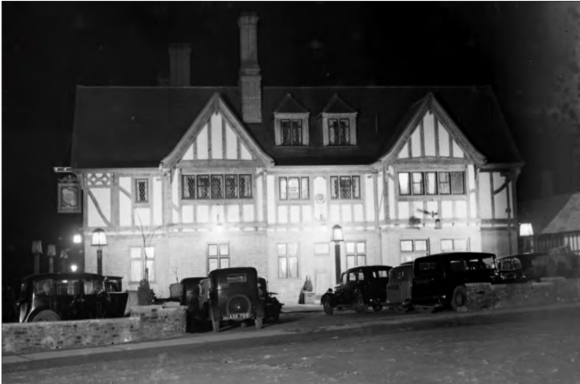
6.2 The north elevation of the Daylight Inn, Petts Wood, London (1935, by Sidney C. Clark), in a photograph of 1936. The car park – placed by the entrance to the pub’s ballroom and enclosed by low boundary walls – is here shown filled with cars. (© TopFoto)
