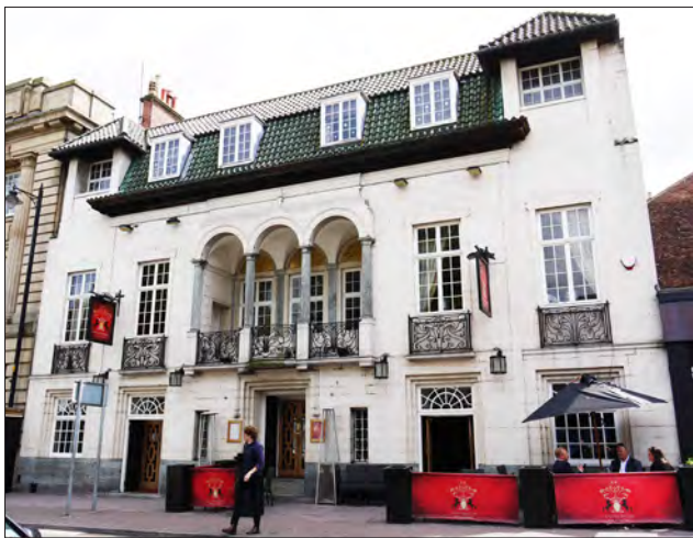
10.10 Currently, seven of the pubs newly built in the inter-war period under the state management scheme in the Carlisle area are included on the statutory list, all at grade II. These include the Spanish-style Crescent Inn, built in 1932 to designs by Harry Redfern. The building now functions as a restaurant. (© Historic England, Emily Cole)
