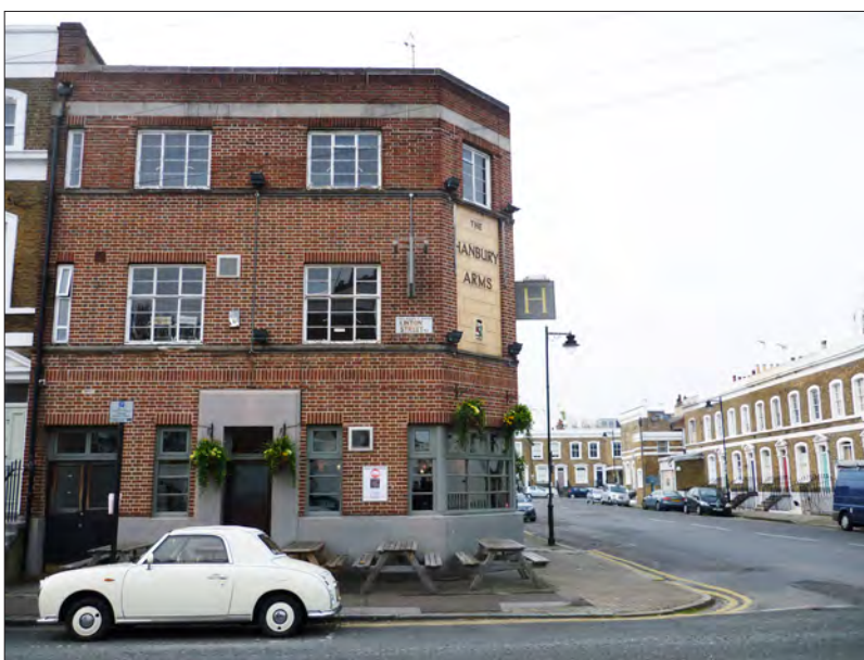
11.13 The inter-war period saw a greater variety in the scale of new pubs than at any other time. This pub is on the smaller side of the spectrum; it is the Hanbury Arms, Islington, London (1936-37). (© Historic England, Luke Jacob)
