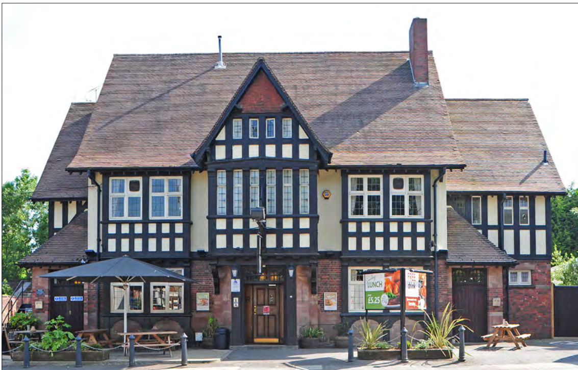
12.6.1 The main (north) elevation of the Biggin Hall Hotel. (© Michael Slaughter LRPS)
