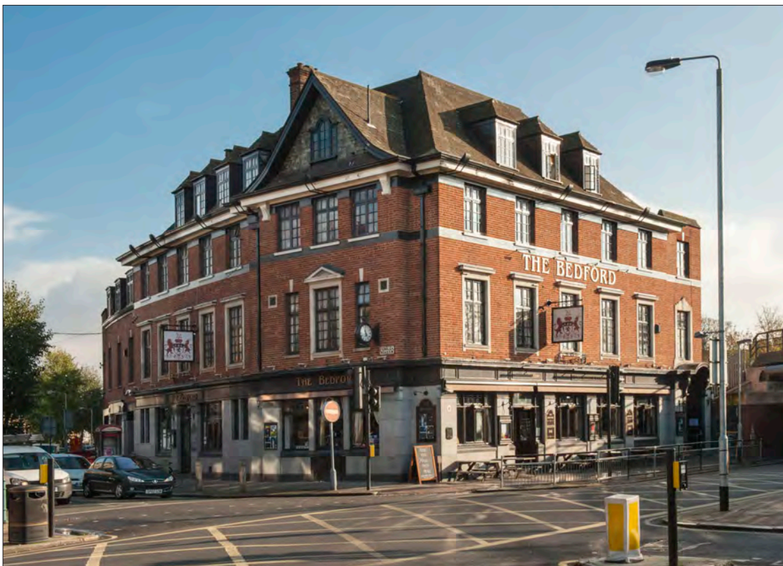
12.3.1 The Bedford Hotel, seen from the north-west. (© Historic England, Derek Kendall, DPI52226)
