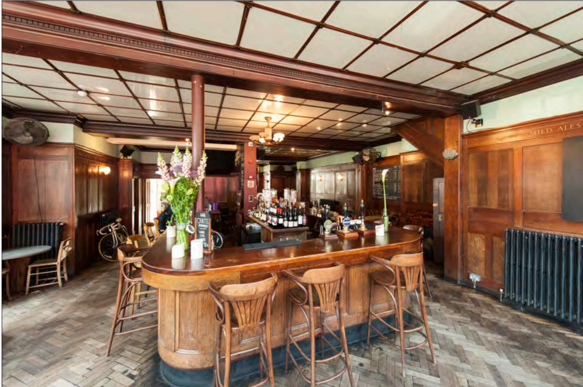
12.32.4 The interior of the Royal Oak, now unified, looking north-west. Original features include the Vitrolite ceiling, the island servery and the panelling. The saloon bar was originally on the left and the public bar on the right, the two areas divided by an off sales compartment. (© Historic England, Derek Kendall, DPI70451)
