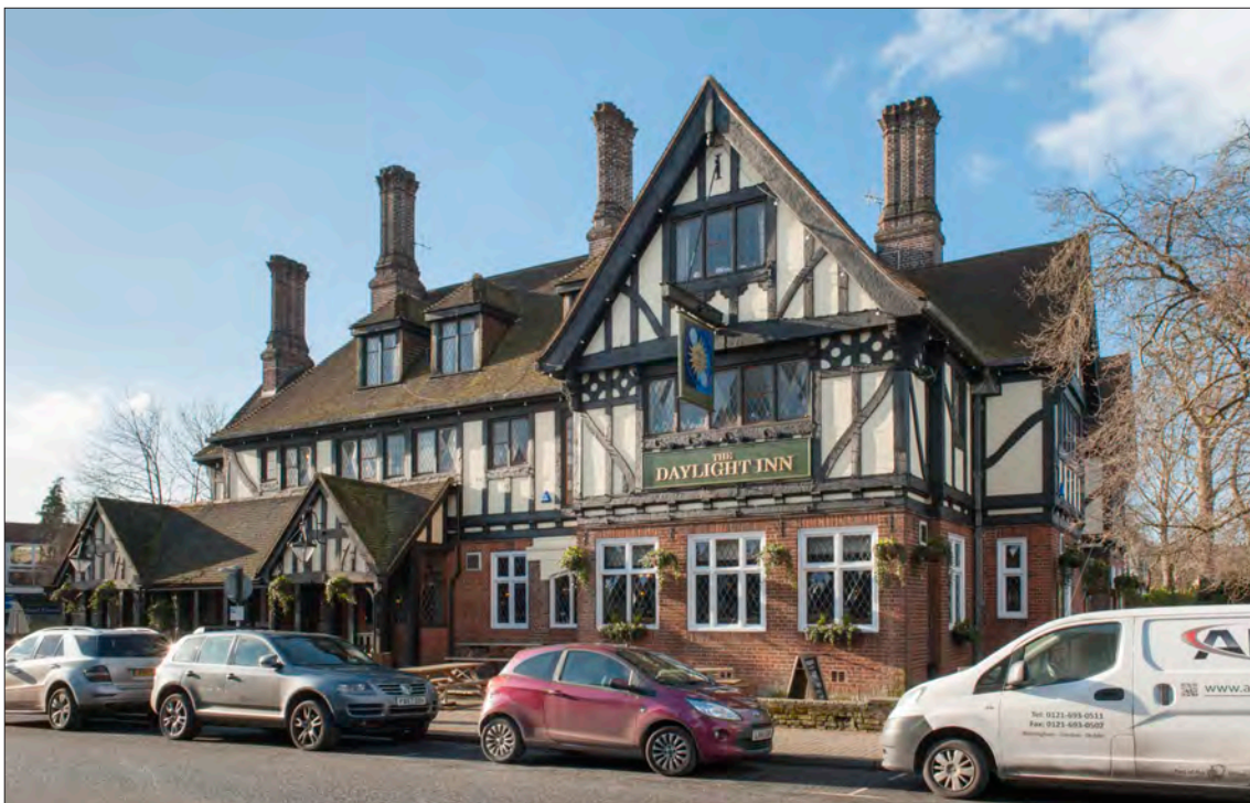
12.14.1 The Daylight Inn seen from the north-east. The single-storey gabled extension on the left of the picture was added in 1996, in sympathetic style. (© Historic England, Derek Kendall, DPI70023)
