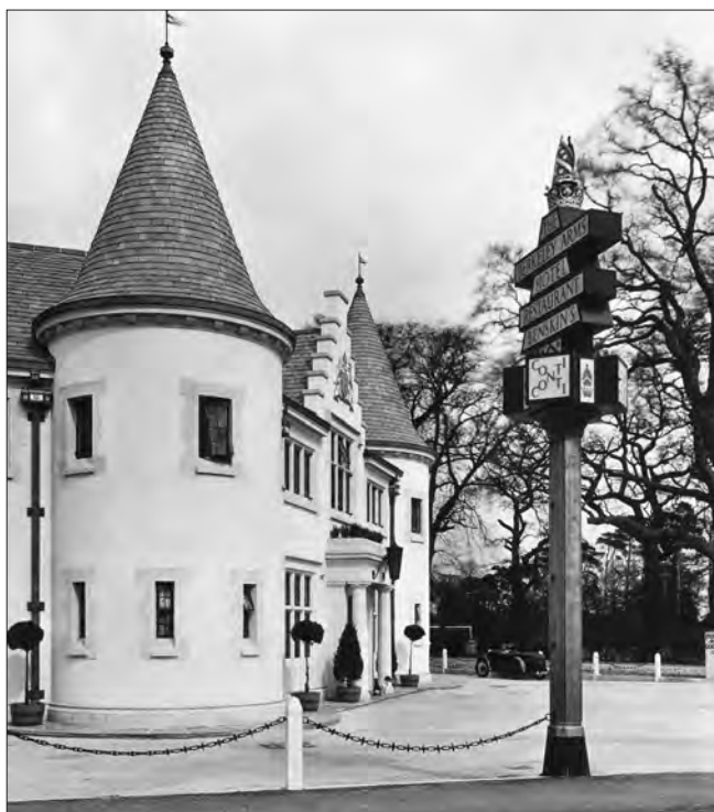
12.4.3 The central elevation, 'draw in' for cars and free-standing sign of the Berkeley Arms Hotel in a photograph of 1932, taken shortly after the building's initial completion. (© Architectural Press Archive/RIBA Library Photographs Collection)
