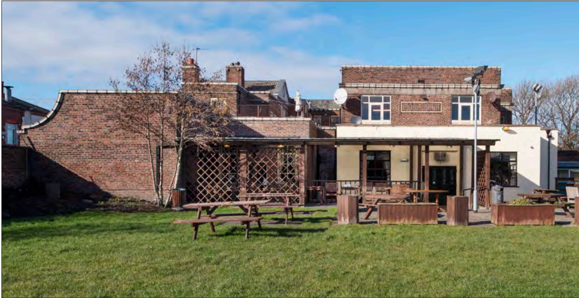
12.19.2 The rear elevation of the Farmers' Arms. Much inter-war work remains, though there have been modern additions, including the rendered block which stands on the site of the former stone loggia. The lawned area was originally a secondary bowling green, the main one being out of view to the right. (© Historic England, James O. Davies, DPI66551)
