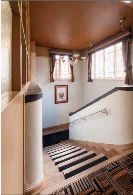
12.5.8 The guest staircase at the centre of the pub's plan, seen from the first-floor landing. The glazed screening on the left is an insertion of the 1970s, added for fire safety reasons. (© Historic England, Derek Kendall, DPI52482)
