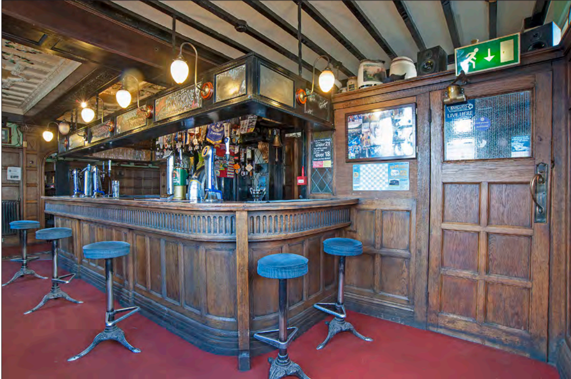
12.27.4 The interior of the public bar. The change in ceiling design marks the division between the old (Victorian) work and the new, simpler beamed work of the inter-war years. The vertical strut on the bar marks the position of a former partition; this seems to have divided the public bar (on the left) and the off sales compartment (on the right). (© Michael Slaughter LRPS)
