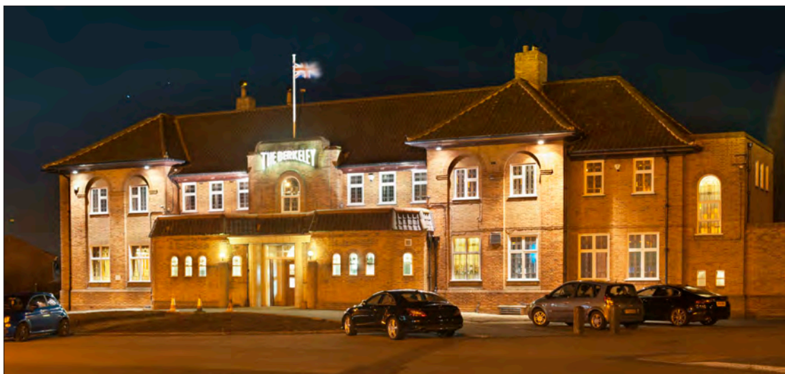
12.5.1 A night-time view of the main elevation of the Berkeley Hotel. (© Historic England, Derek Kendall, DPI52409)
