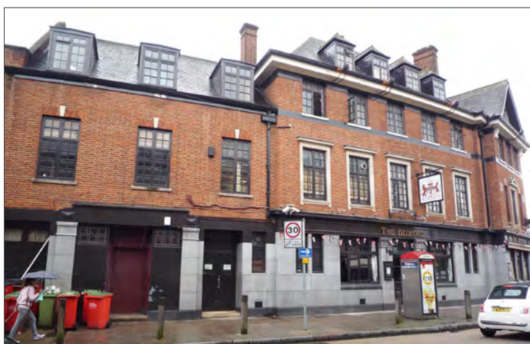
12.3.2 The side (north/Fernlea Road) elevation of the Bedford Hotel, with the former off licence on the left of the image. (© Historic England, Emily Cole)
