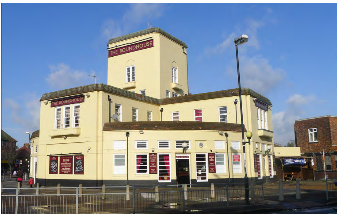
12.31.1 The striking exterior of the Round House, seen from Porters Avenue. The ground floor of the two-storey block on the left of the image originally contained an off licence with showcase windows (see Fig. 5.16), but this area has since been infilled. (© Historic England, Luke Jacob)
