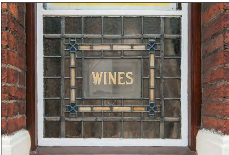
12.2.3 A detail of the coloured glass on the pub's Matthias Road elevation. Originally, this window seems to have lit the off sales compartment. (© Historic England, Derek Kendall, DPI70115)
