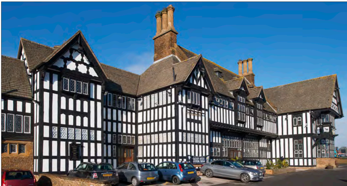
12.7.1 The main elevation of the Black Horse, fronting onto Bristol Road South. The pub was built on an especially lavish scale, of high-quality materials. It is one of the country's most important examples of the Brewers' Tudor style. (© Historic England, James O. Davies, DPI66423)
