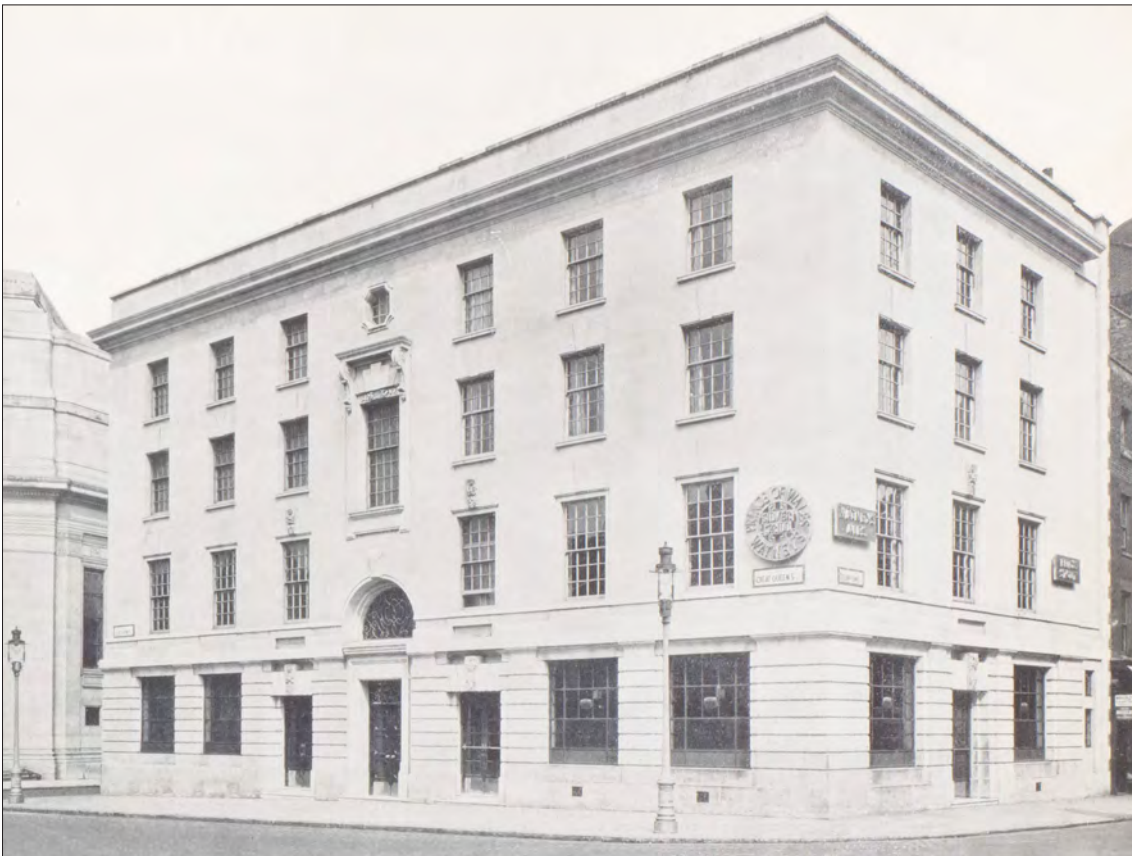
12.28.2 The Prince of Wales in an image published in Architectural Design and Construction in 1934. The project was unusual in that the pub only occupied part of the building (the right half). The remainder was designed by the same architect – A. W. Blomfield of Watney's – but was intended for use by Lambert & Butler's, whose tobacco factory and offices were situated to the rear of the site.
