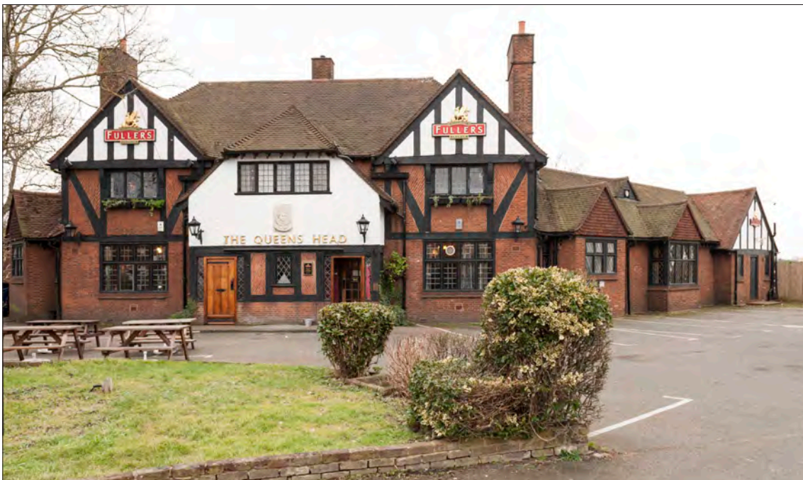
12.29.1 The Queen's Head seen from the north-west. The single-storey wing on the right contains the former saloon lounge, while the pub's 'draw in' and car park can be seen in the foreground. (© Historic England, Derek Kendall, DPI70056)
