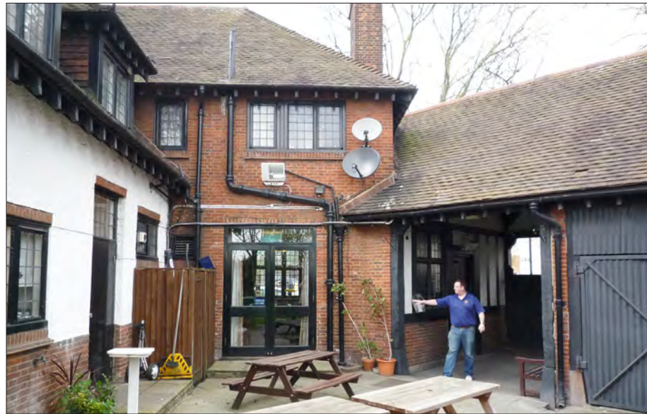
12.29.2 The rear elevation of the pub, showing the 'drive-in' in the north-east wing. The modern doors at the centre of the photograph open from the public bar. (© Historic England, Emily Cole)
