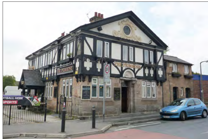
12.27.3 The pub's side elevation to Withens Lane, with its bullseye window and decorative surround at attic level. The side doorway led to the off sales area, and also to the parlour, with access to the other main rooms of the pub. (© Historic England, Emily Cole)
