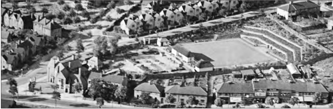
12.9.3 Aerial view of 1931 showing the extensive gardens of the Brookhill Tavern. The pub is on the left of the image; the gardens ascend gradually behind it, culminating in the bowling green with a stepped terrace beyond. (© Historic England. Aerofilms Collection.)
