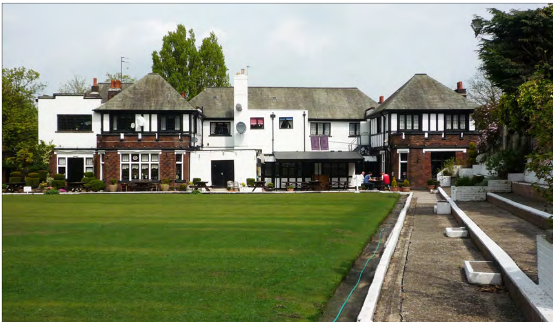
12.35.2 The Wheatsheaf's rear (south) elevation, with the bowling green in the foreground and the terraced viewing area on the right. Some of the structures at the centre of the pub's façade are modern additions, including the projecting roof canopy. (© Historic England, Emily Cole)
