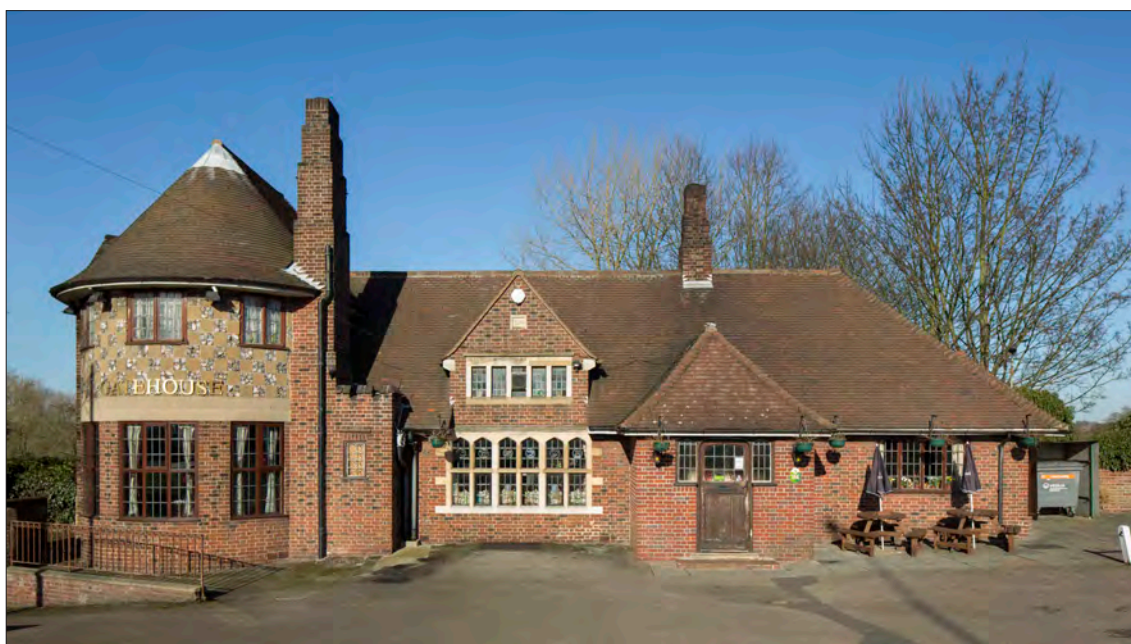
12.20.1 The main elevation of the Gate House survives largely as built. The entrance porch is an addition, but is sympathetic in style and reuses original work. The pub is notable for its distinctive design, influenced by the Arts and Crafts and local vernacular traditions. (© Historic England, Patricia Payne, DPI72331)
