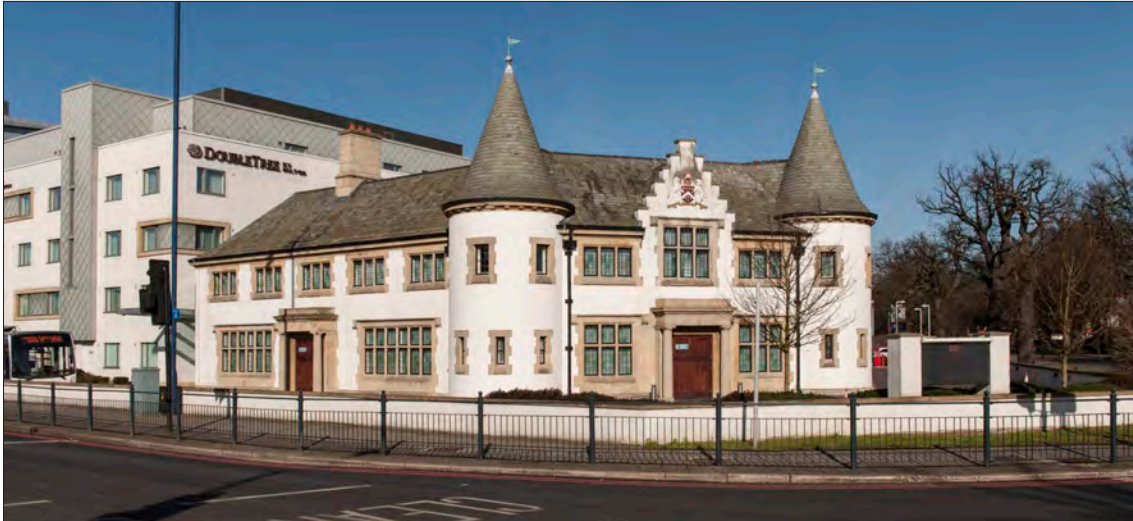
12.4.2 The former Berkeley Arms Hotel, seen from the A4 (Bath Road), with the modern hotel extension to its left. (© Historic England, Derek Kendall, DPI70177)
