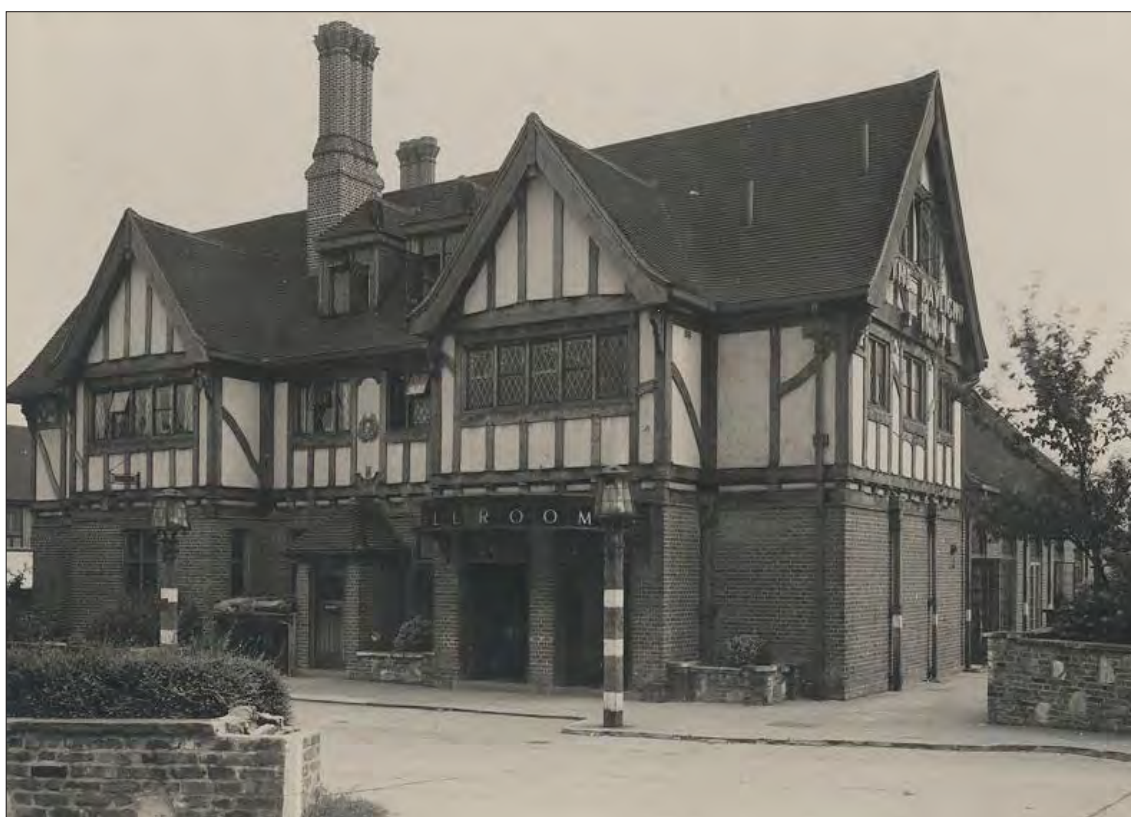
12.14.3 A photograph of 1941, taken from the pub's north-west. A curved canopy bears the name of the ballroom, which filled the block which can be seen to the rear right. (Image courtesy of the National Brewery Centre, Burton on Trent)
