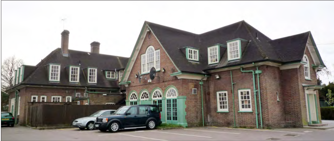
12.26.2 The Pear Tree seen from the north-east. The car park was always to the north of the pub. The doorway on the right of the image leads to the stairhall which provides access to the first-floor club room, lit by Venetian windows at each end. (© Historic England, Luke Jacob)
