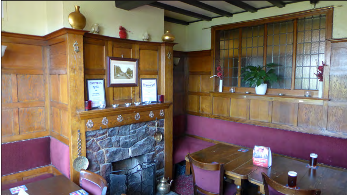
12.15.3 The snug, with original panelling, fireplace, beamed ceiling and leaded glazing. (© Historic England, Luke Jacob)
