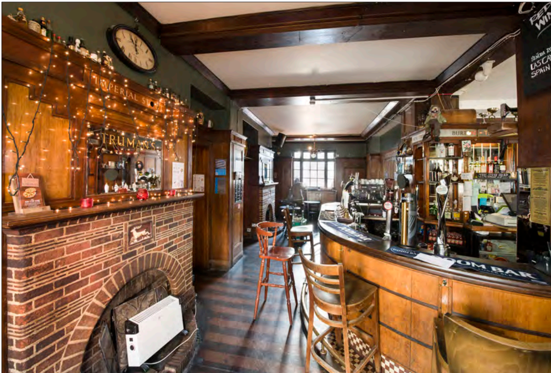
12.33.4 The east (left-hand) side of the Stag's Head, which contained the saloon bar and, to the rear, what was probably a saloon dining room, both served by brick fireplaces and a Moderne-style counter. Doorways have been inserted in the left wall to provide access to the function room block added in c. 1970. (© Historic England, Derek Kendall, DPI52388)
