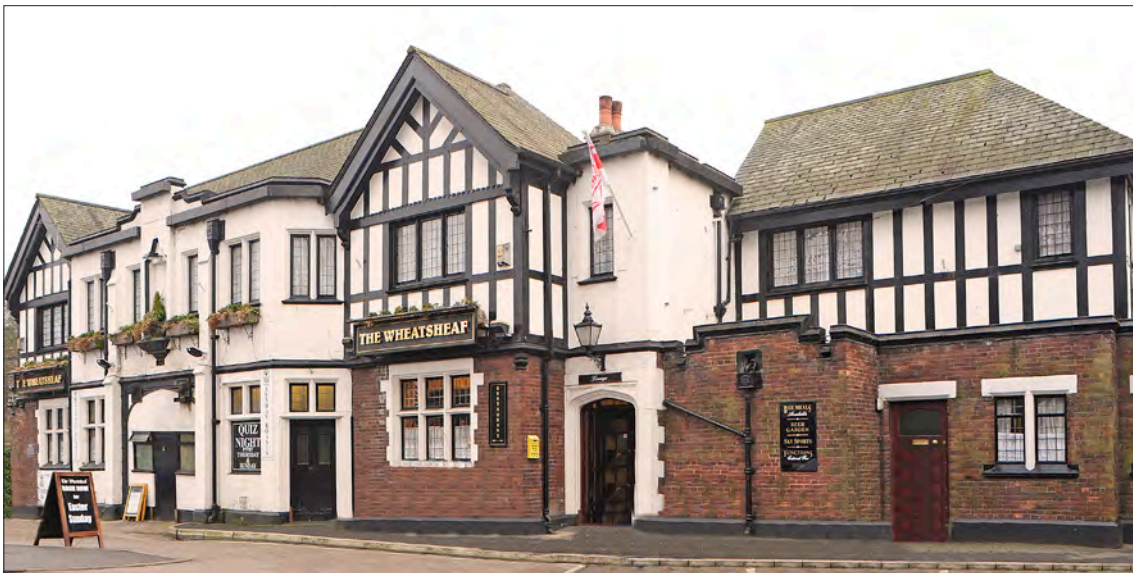
12.35.1 The principal (north) elevation of the Wheatsheaf. The only notable alteration has been the infilling of the archway at the centre of the main part of the façade. The first floor of the block on the right of the picture contains the accommodation of the pub's landlord/manager. (© Michael Slaughter LRPS)
