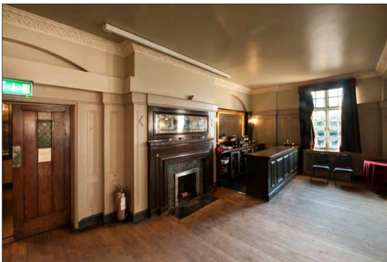
12.3.8 The fireplace at the south end of the first-floor ballroom. The servery to the right is modern; it occupies the site of what were in and out doors accessing an adjacent service room. (© Historic England, Derek Kendall, DPI52264)
