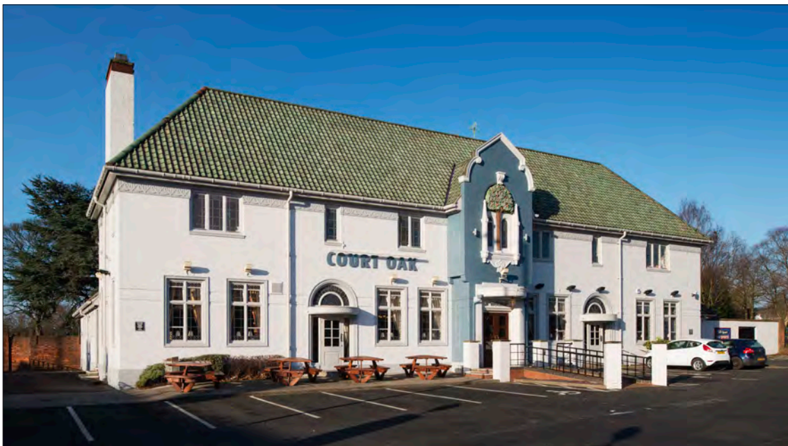
12.13.1 The main elevation of the Court Oak, designed in a style influenced by Hispano-Moorish architecture. The car park, elaborate carved sign and green tiled roof are original, though the sloping disabled access leading to the central doorway is a modern addition. (© Historic England, James O. Davies, DPI66392)
