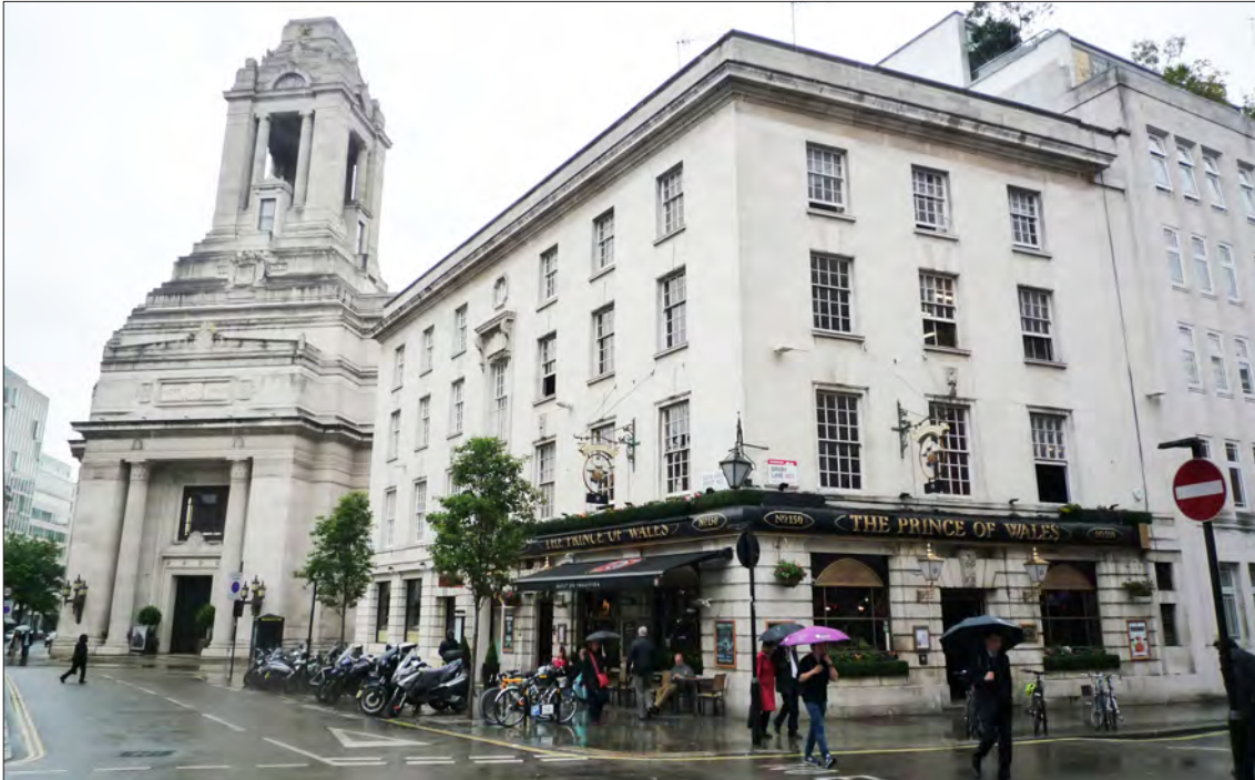
12.28.1 A modern view of the Prince of Wales, taken from Drury Lane, with the Freemasons' Hall of 1927-33 (listed grade II*) on the left of the photograph. (© Historic England, Emily Cole)
