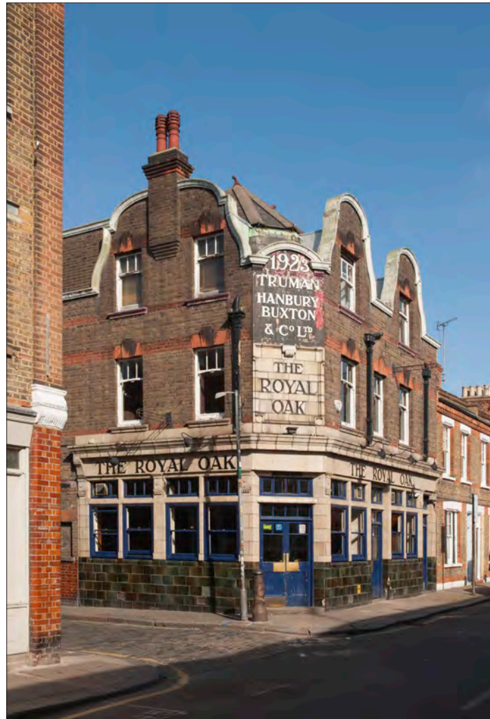
12.32.2 The pub seen from Columbia Road. The exterior has been very little altered since the building's completion in 1923. (© Historic England, Derek Kendall, DPI70190)
