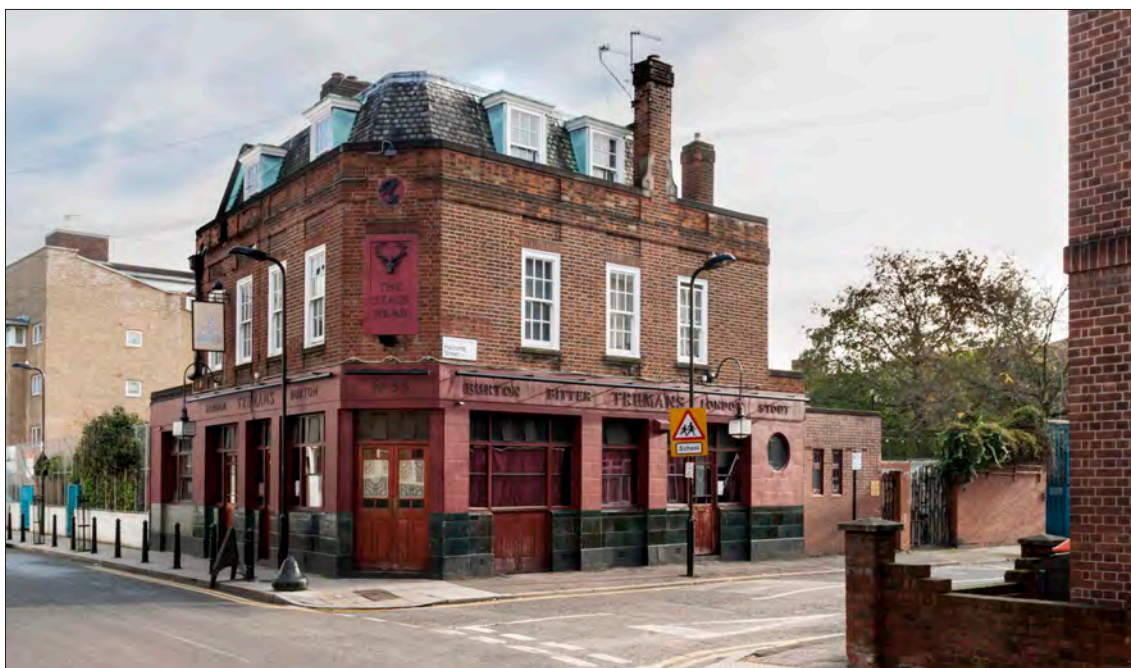
12.33.1 The exterior of the Stag's Head. The single-storey block on the left of the pub – containing a function room – was built in c. 1970 in sympathetic style and of similar materials. (© Historic England, Derek Kendall, DPI52384)
