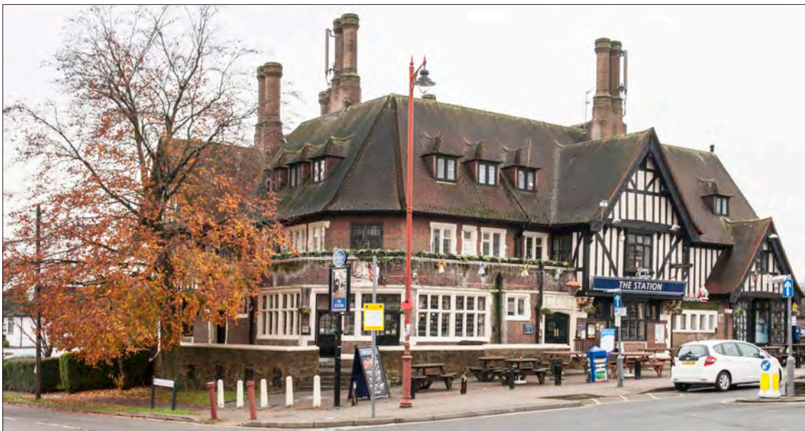
12.34.1 The Stoneleigh Hotel, seen from the Broadway. The former off licence is on the right of the image, topped by a gable. (© Historic England, Derek Kendall, DPI52333)
