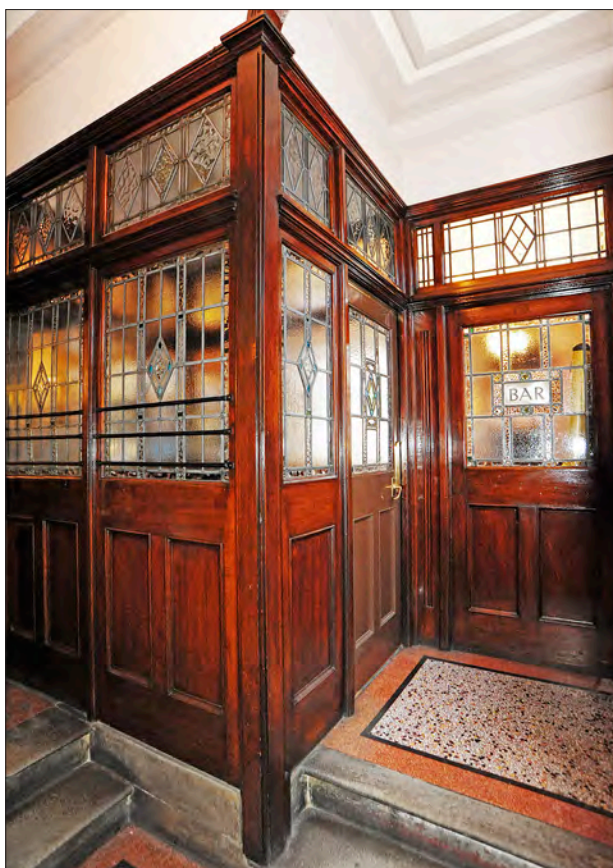
12.17.2 The entrance vestibule of the Duke William, with its leading glazing and terrazzo flooring. The steps on the right lead to the public bar (named 'bar' on the door), while the doorway on the left of this formerly led to the off sales compartment (now the main entrance to the public bar). (© Michael Slaughter LRPS)
