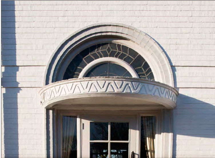
12.13.2 A detail of the Court Oak's main elevation, showing the canopied entrance to one of the side bars. (© Historic England, James O. Davies, DPI66396)
