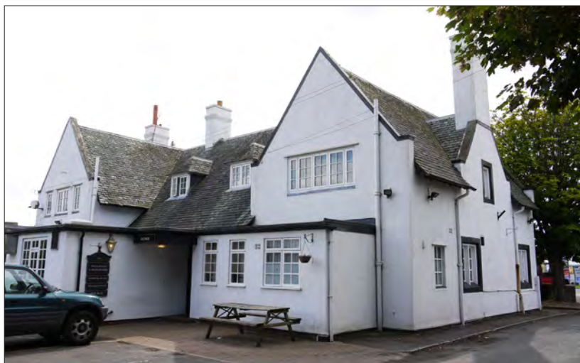
12.11.2 A photograph from the north-east, showing the pub's rear and side (north) elevations. (© Historic England, Clare Howard)
