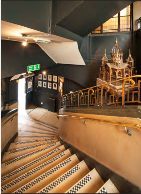
12.3.6 The curved marble and terrazzo staircase at the pub's south-west, looking down towards the lobby and entrance hall. The stair provides access to the pub's first-floor 'entertainment suite'. (© Historic England, Derek Kendall, DPI52251)
