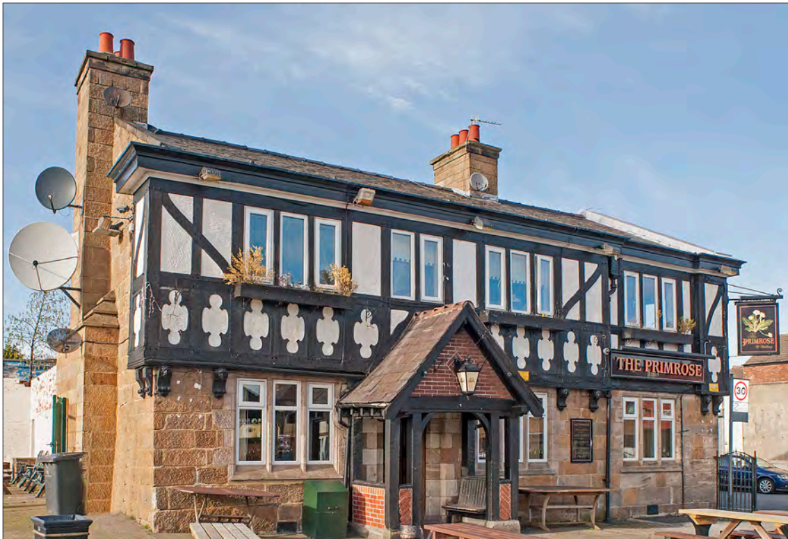
12.27.1 The main (south-east) elevation of the Primrose. Aside from the replacement windows, the pub appears to survive largely as rebuilt in 1922-23. (© Michael Slaughter LRPS)
