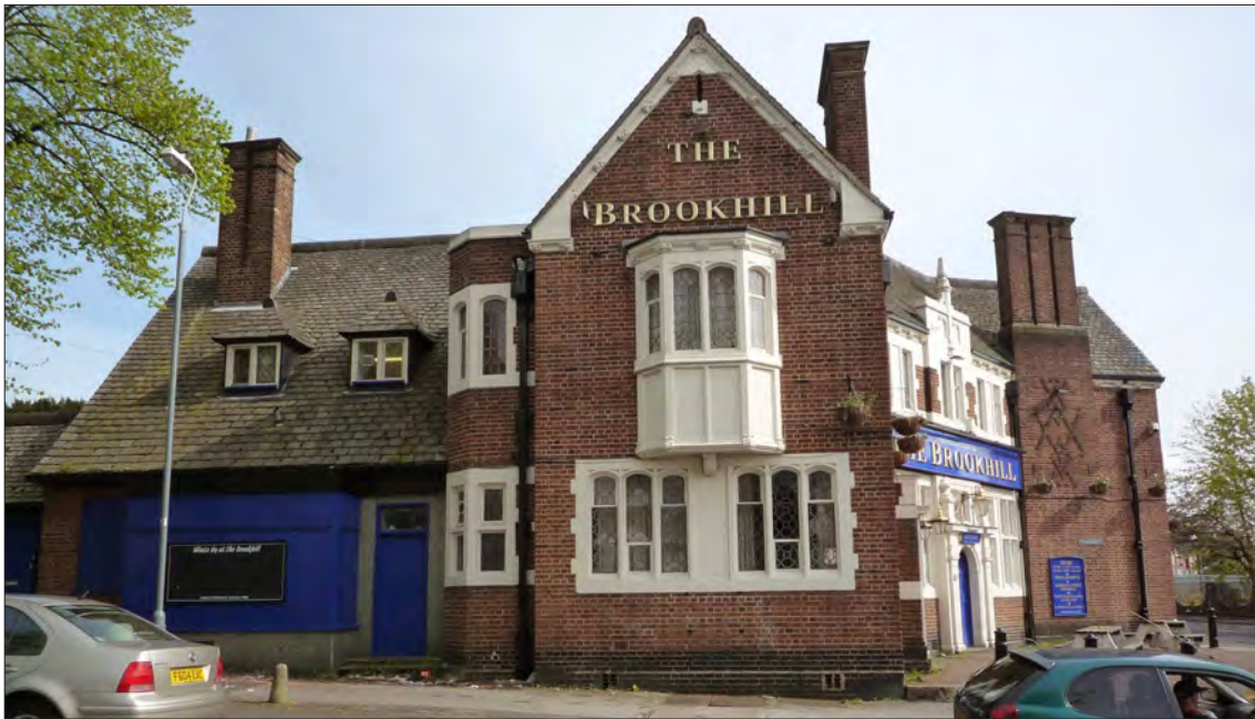
12.9.2 The Brookhill Tavern in April 2014, seen from Brook Hill Road. The shopfront on the left of the image seems to have been inserted around the late 1950s, and probably served as an off licence. It occupies the site of the pub's original off sales compartment. (© Historic England, Emily Cole)
