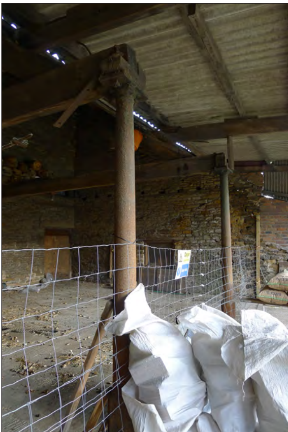
Fig 121. Alderthwaite's northern farm building: (a) the spine-wall viewed from the north (note the remaining trusses on iron columns at the far end) and (b) iron columns supporting the better preserved south side, D Went, November 2017. © Historic England.
