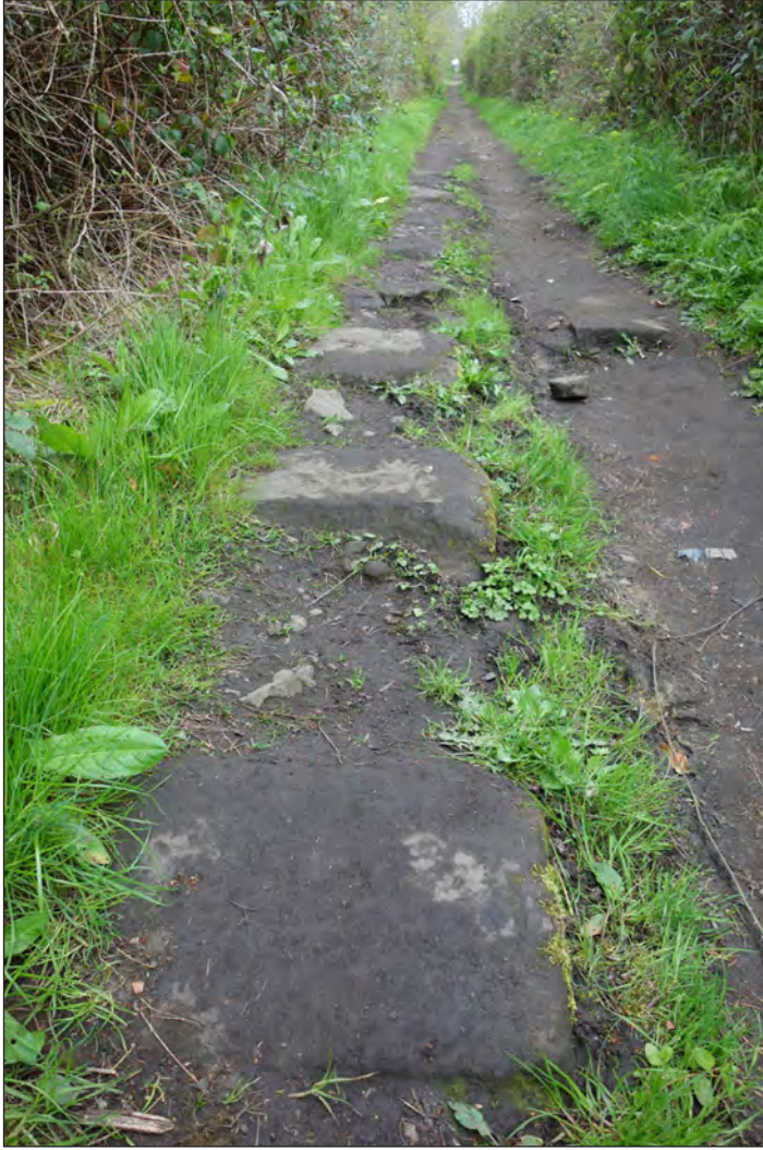
Fig 185. Stone sleepers visible on the line of the Elsecar-Milton incline west of Fitzwilliam Street, viewed from the east D Went, April 2019. © Historic England.
