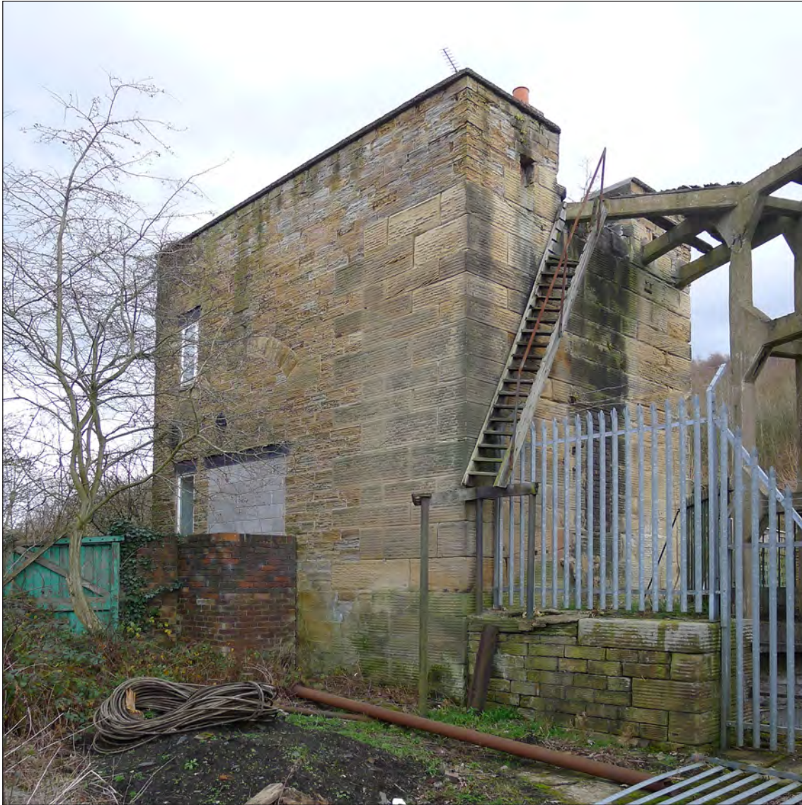
Fig 100. Pump House at Hemingfield Colliery, L Jessop, December 2017. © Historic England.
