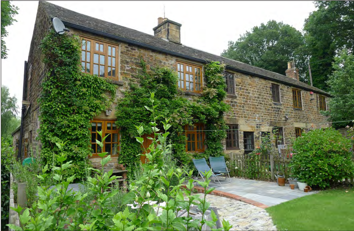
Fig 87. Nos. 4-8 Distillery Side from the front, L Jessop, June 2017. © Historic England.
