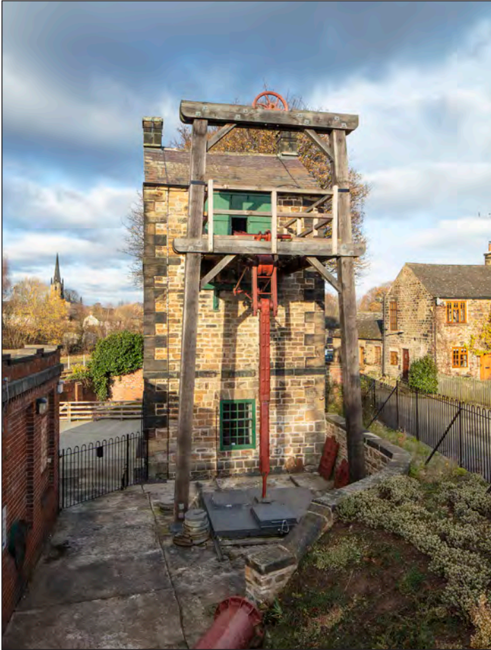
Fig 36. (a) The Newcomen engine with 20th-century brick pump- and fan house in the foreground, Alun Bull, October 2017, and (b) looking north-west showing the current boiler and the base of the former chimney behind, L Jessop, June 2017. © Historic England.
