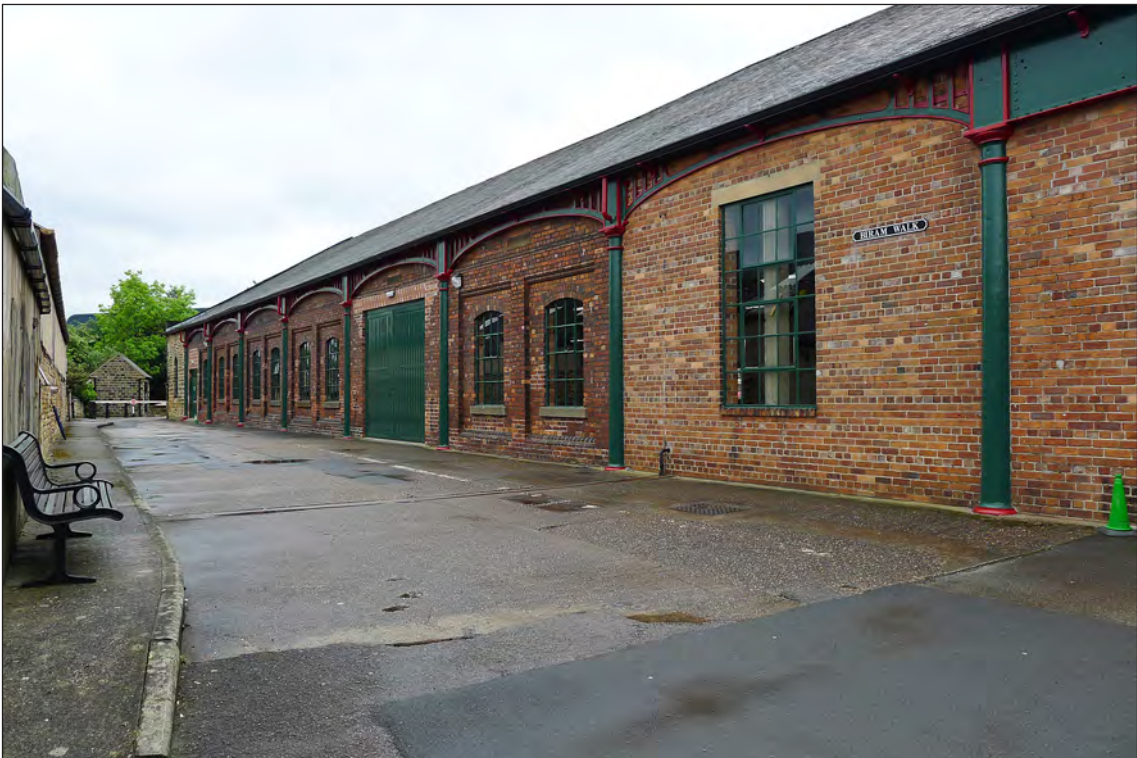
Fig 64. (a) above: Building 21, east elevation and (b) below: west elevation. L Jessop, June 2017. © Historic England.
