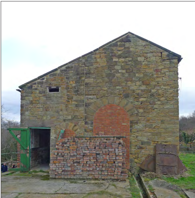
Fig 98. Engine House at Hemingfield Colliery, L Jessop, December 2017. © Historic England.
