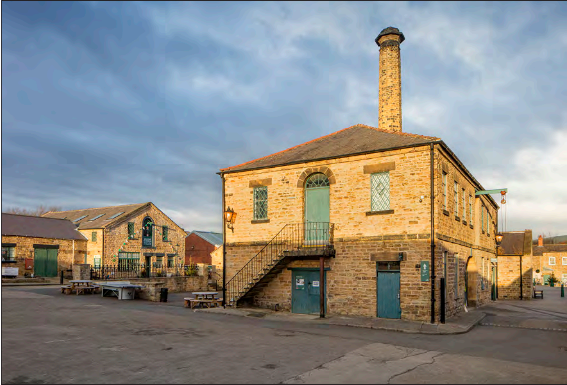
Fig 78. Building 22 looking north-west, Alun Bull © Historic England.
