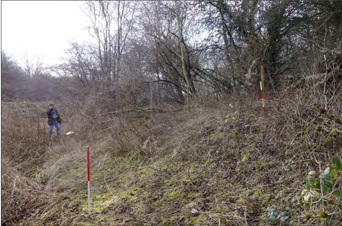
Fig 47. The deep cutting for the inclined plane. February 2018 © Historic England.
