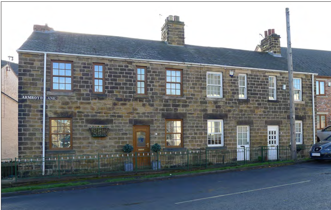
Fig 177. Nos. 2, 6 & 8 Armroyd Lane, D Went, November 2017. © Historic England.
