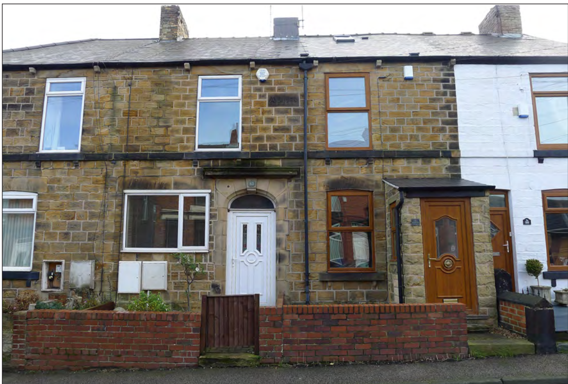
Fig 169 (a) top left: nos. 16-18 Hill Street (b) top right: 'St Helens Terrace' 66-70 St Helen's Street and (c) below: no. 63 St Helen's Street, detail of doorway, D Went, November 2017. © Historic England.
