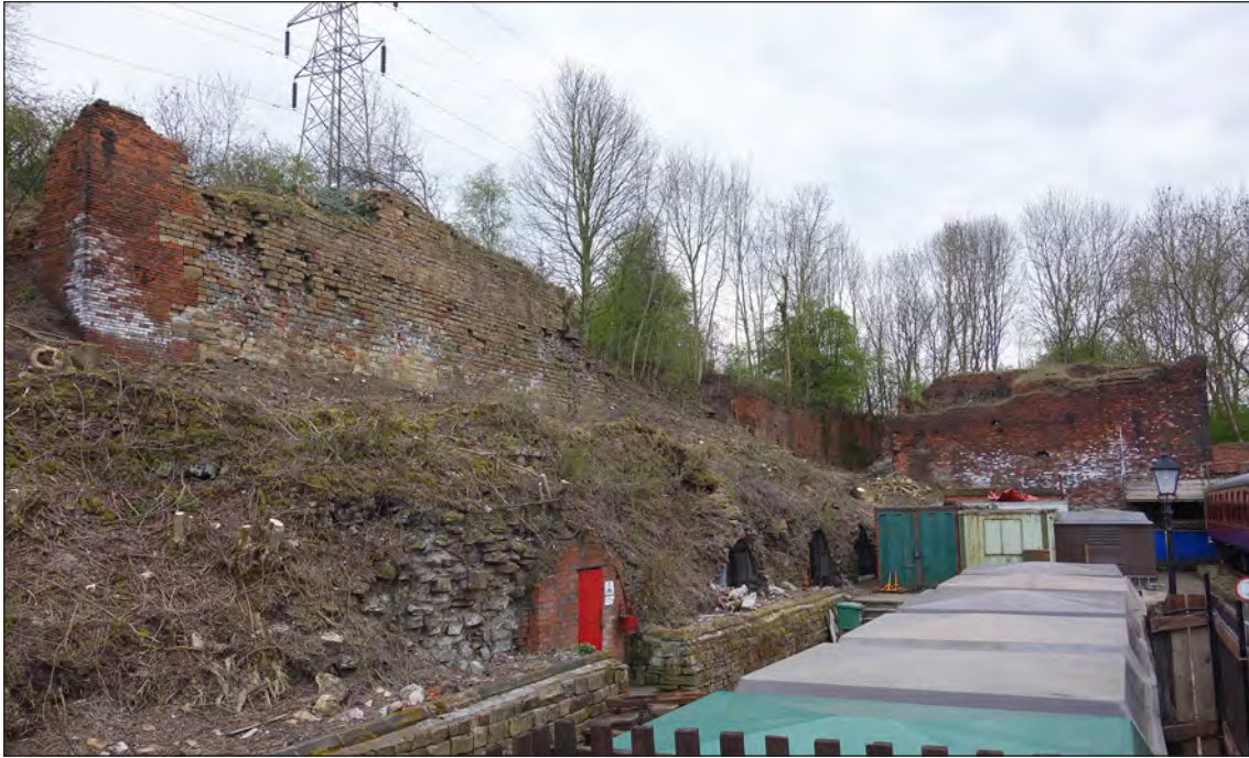
Fig 49. The area of the former blast furnaces, which stood in front the alcoves at the rear of the Heritage Railway station, following tree clearance, D Went, April 2019. Note the solid retaining wall across the slope to the left and the massive brick wall in the background which formed part of the blowing engine house and boiler yard. © Historic England.
