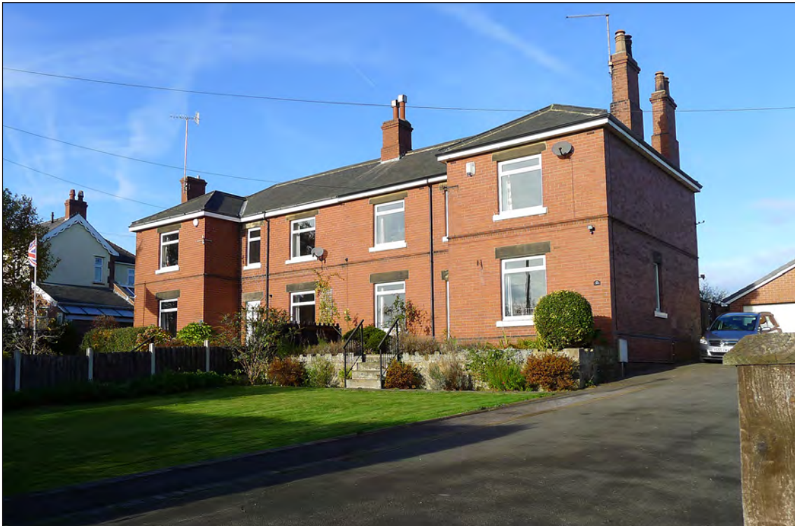
Fig 134. 31-33 Armroyd Lane, one of two semi-detached pairs built for the Fitzwilliam estate in 1924, D Went, November 2017. © Historic England.
