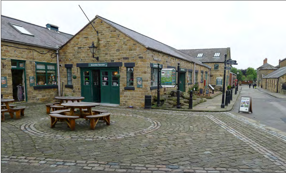
Fig 80. Wath Road range, looking north, L Jessop, June 2017. © Historic England.
