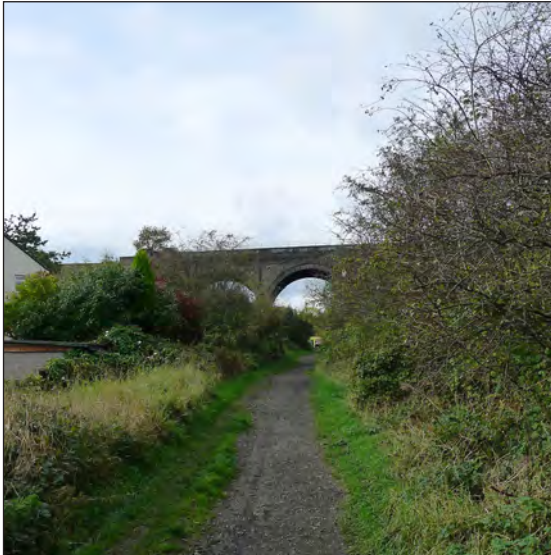
Fig 197. The line of the former Jump (Hoyland Silkstone) incline running north-west from Welland Crescent under the Midland Railway viaduct which was built to accommodate it, D Went, October 2017. © Historic England.
