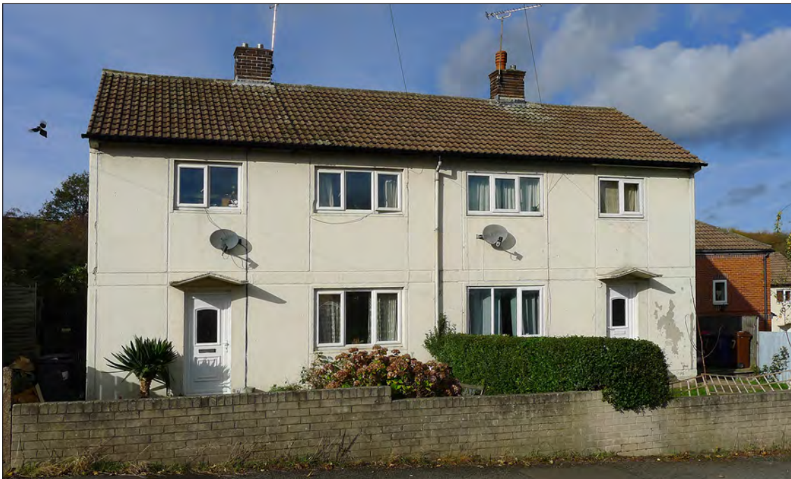
Fig 200. Wates pre-cast concrete housing, Welland Crescent, D Went, November 2017. © Historic England.
