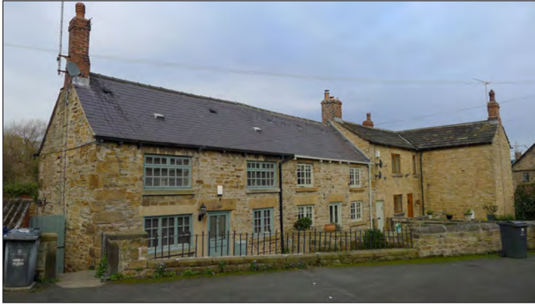
Fig 154. Nos. 9 and 10 Market Place, D Went, November 2017. © Historic England.
