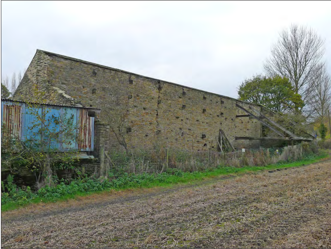
Fig 121. Alderthwaite's northern farm building: (a) the spine-wall viewed from the north (note the remaining trusses on iron columns at the far end) and (b) iron columns supporting the better preserved south side, D Went, November 2017. © Historic England.
