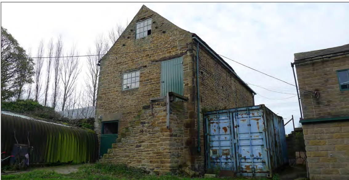
Fig 120. Alderthwaite. 18th-century cow house and hayloft viewed from the east, D Went, November 2017. © Historic England.
