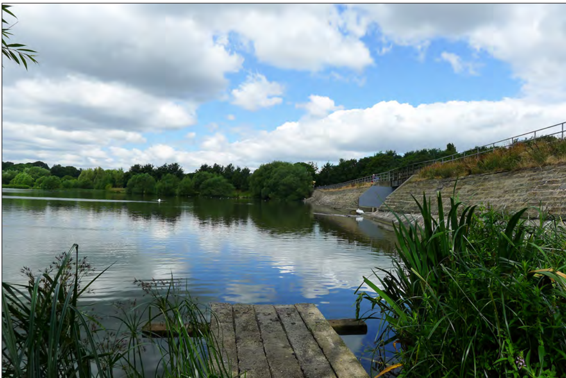
Fig 110. Elsecar Reservoir looking north-west, with the dam to the right of the frame, L Jessop, July 2017. © Historic England.
