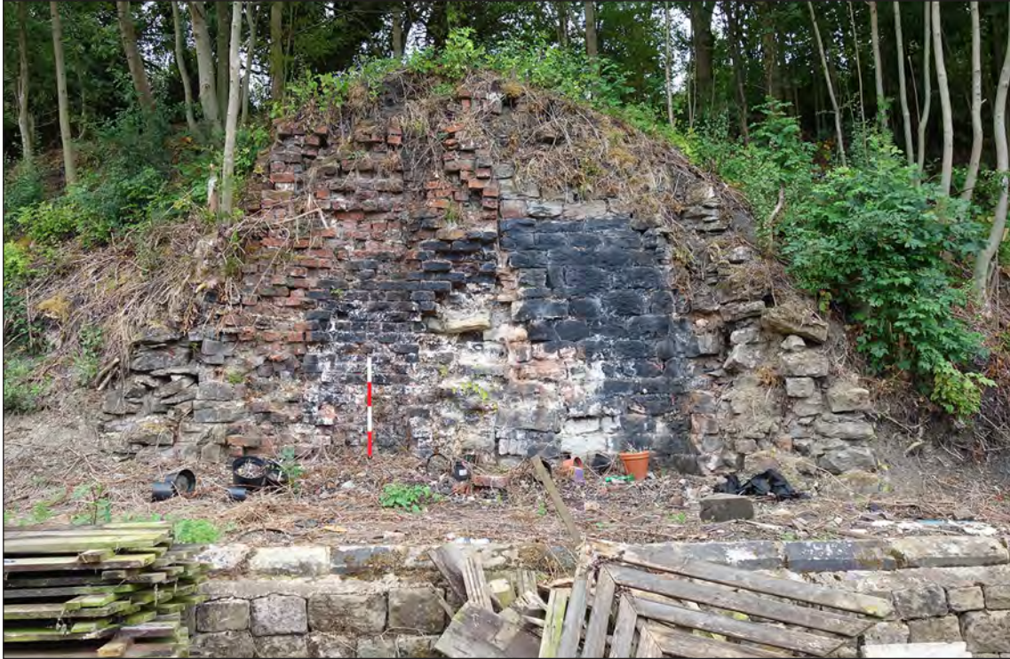
Fig 53. The blacked and scorched section of the rear yard wall, about 11m north of the paint store alcove. Note the straight joint between the brick structure to the left and the stone wall to the right, and the traces of a brick wall projecting into the yard from this junction. The lower boundary wall below is a 20th-century construction of reclaimed materials, February 2018 © Historic England.
