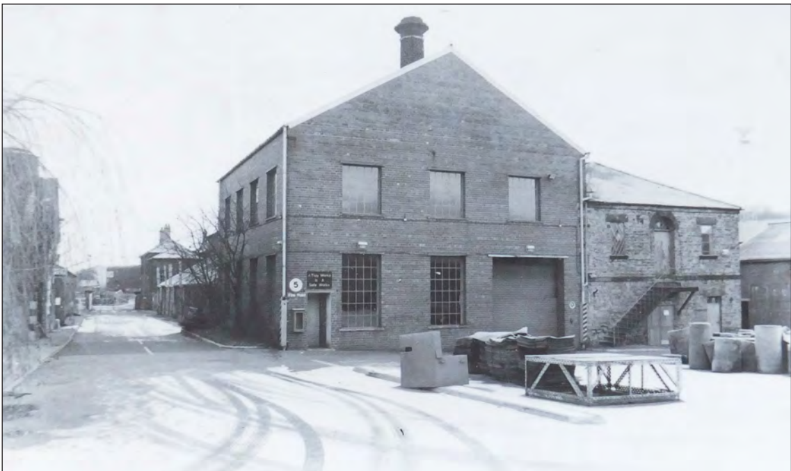
Fig 29. Photograph of the large NCB building at the southern end of Building 17. Reproduced with the kind permission of Barnsley Archives and Local Studies, Elsecar NCB workshops archive photo 11.
