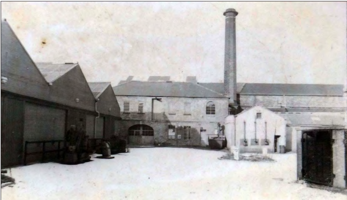
Fig 75. Building 17, (a) Looking north-east, L Jessop, June 2017, © Historic England and (b) 1980s photograph looking north-west towards the chimney and boiler house, reproduced with kind permission of Barnsley Archives and Local Studies, NCB workshops archive photo 32.
