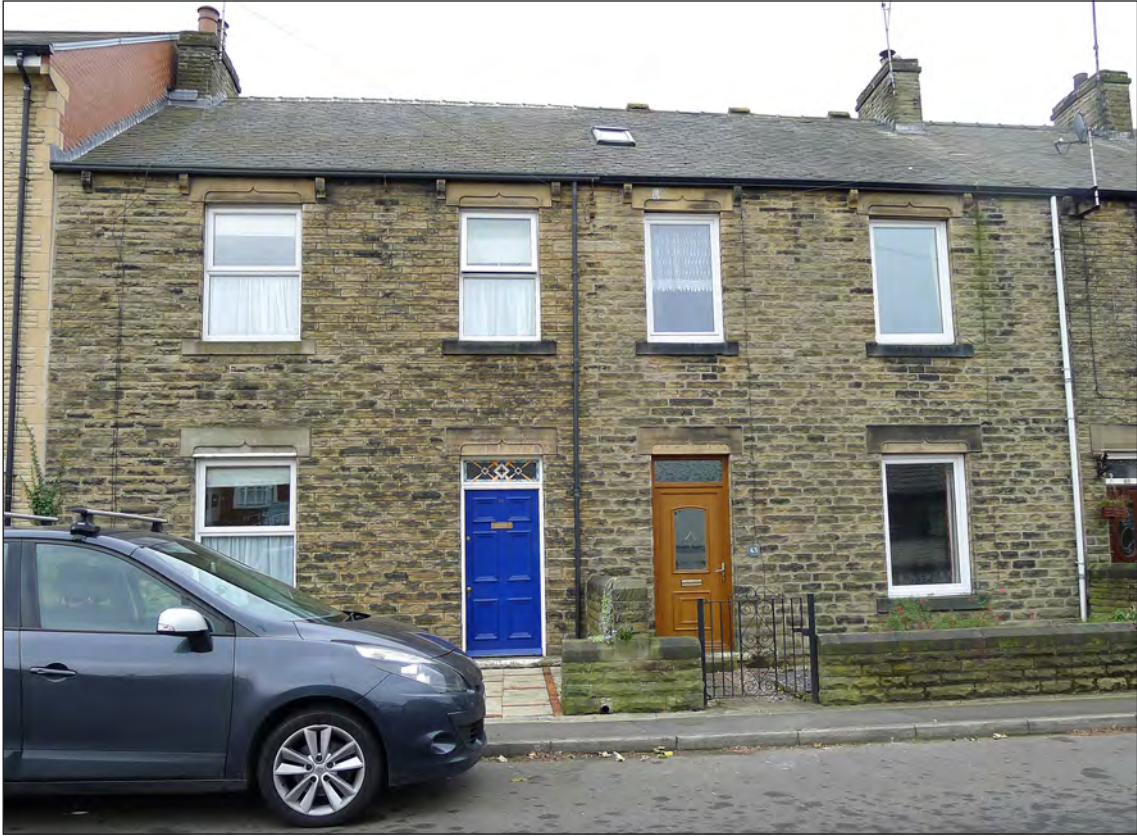
Fig 176. Nos. 55-65 Church Street, with detail of window lintels with ogee mouldings, D Went, November 2017. © Historic England.
