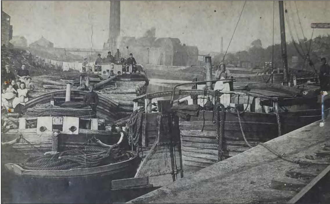
Fig 95. Elsecar's canal basin in the late 19th century. Note the unladen barge riding high, up to the level of the wharf, and the railway track (no longer present) alongside. Reproduced with the kind permission of Barnsley Archives and Local Studies A/3133/Z/1-2.
