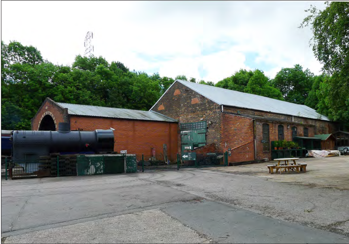
Fig 69. Building 1, former Elsecar Ironworks looking south-east, L Jessop, June 2017. © Historic England.
