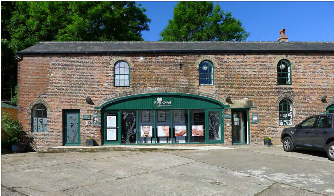
Fig 67. (a) above: Building 3, former ironworks building, from Forge Lane, Alun Bull, November 2017; and (b) below: from within the former ironworks site, L Jessop, June 2017. © Historic England.
