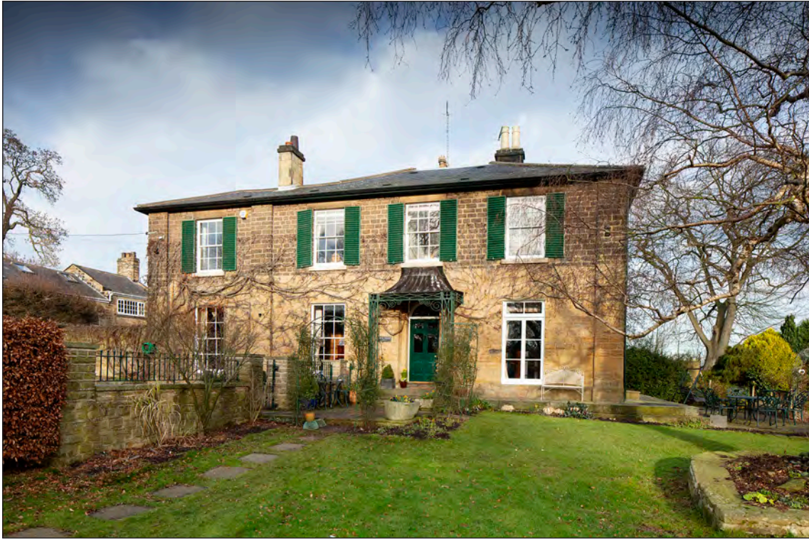
Fig 128. Skiers Spring Lodge viewed from the west. Note the remaining section of iron veranda serving as a porch, Alun Bull, January 2019. © Historic England.
