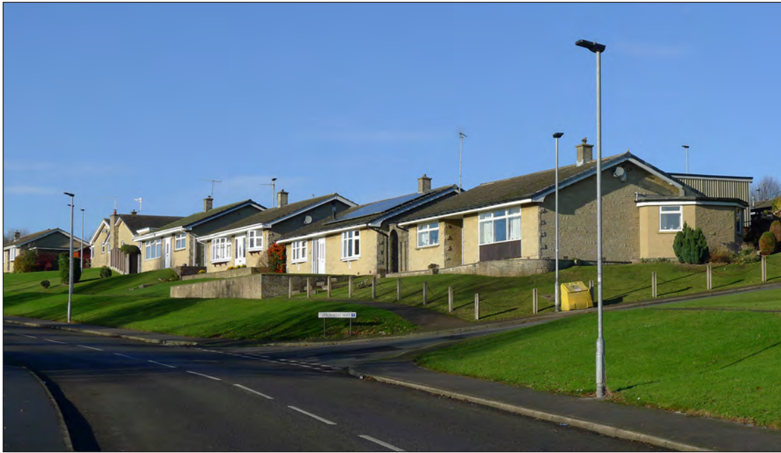
Fig 149 (a) above: Pine Close, McKay VC Memorial Cottages (b) below: bungalows to Clough Fields Road, D Went, November 2017. © Historic England.
