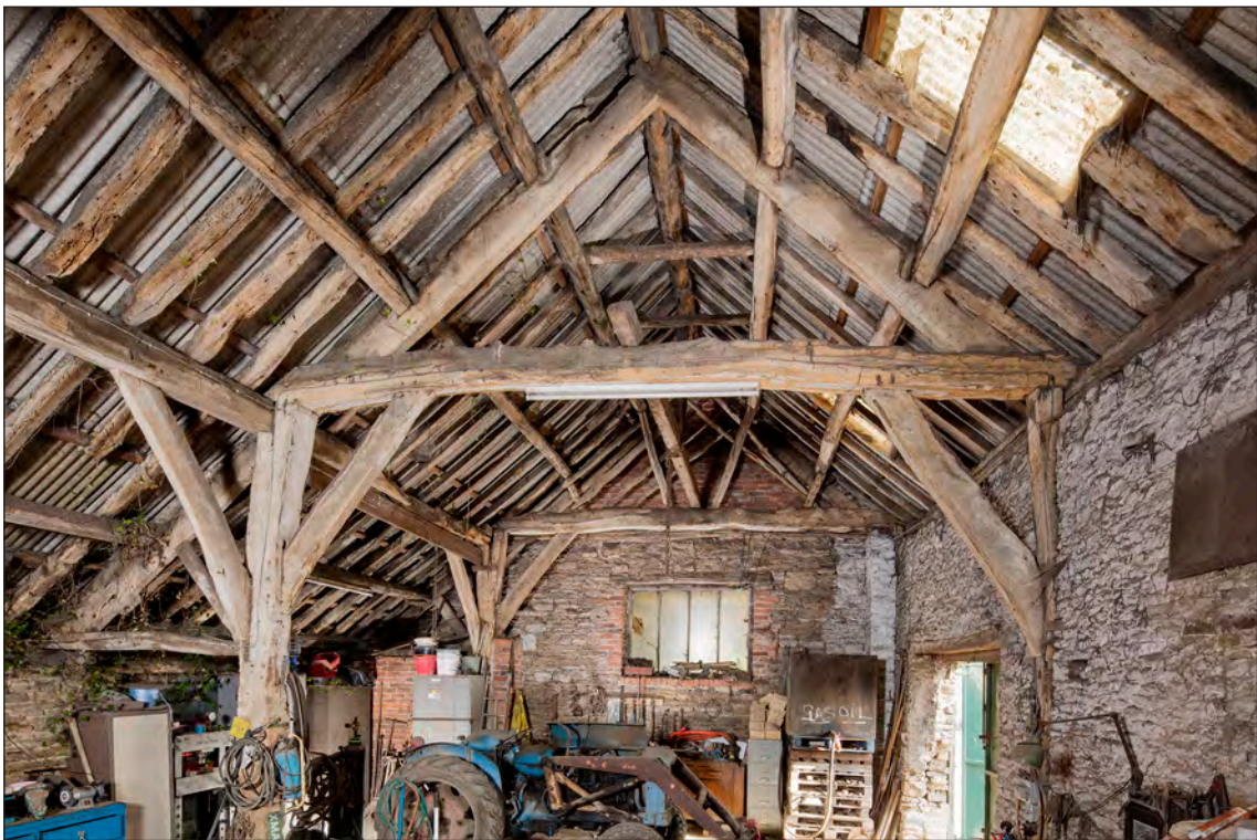
Fig 119. Alderthwaite's timber-framed barn (a) viewed from the west; (b) internal view from the north, note the central truss, Alun Bull, July 2017. © Historic England.
