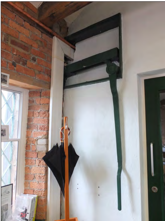
Fig 79. (a) Building 22, ground floor looking north-east, L Jessop, June 2017. © Historic England and (b) clutch mechanism embedded in the dividing wall (first floor level) between the former saddler's workshop and engine room, T Roberts, July 2019. © Barnsley Museums.
