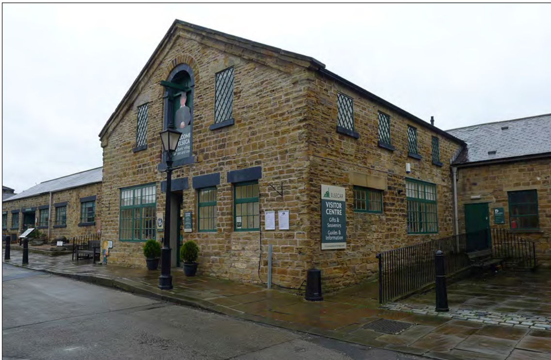
Fig 81. Building 10 looking west, L Jessop, June 2017. © Historic England.
