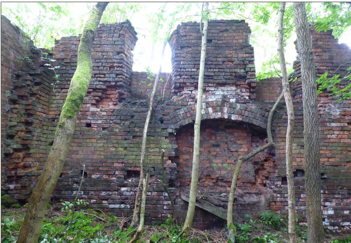
Fig 59. The interior west wall of the blowing engine house, J Rimmer, July 2017. © Historic England.
