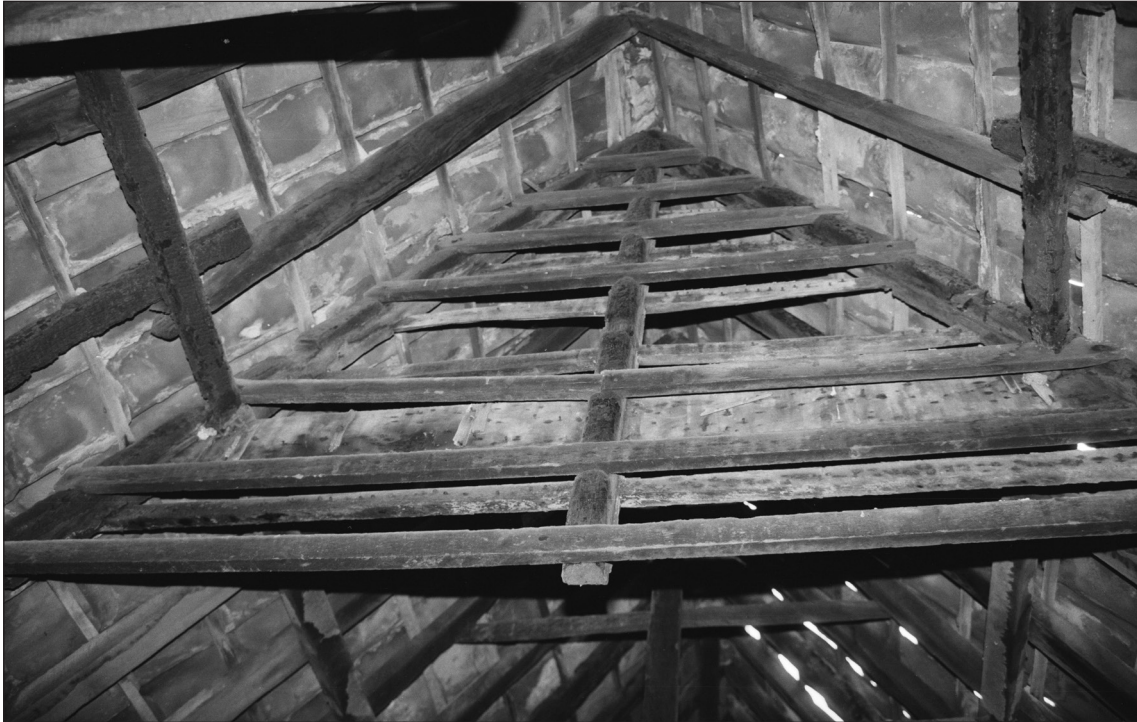
Figure 69: The attic storey or roof space of number 333 Whapload Road. Beneath the pantiles, smoke blackened loaves, survived in situ evidencing the building's former use for fish smoking. The central vertical strut had been cut down and the horizontal racking removed to allow the insertion of a first floor. © Crown Copyright. Historic England Archive, 92/E/26
