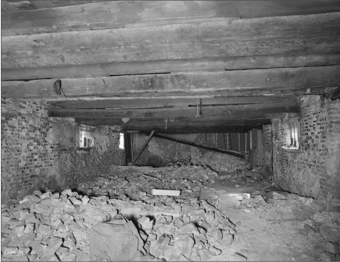
Figure 67: The ground floor of 333 Whapload Road looking east. Amongst the rubble, it is possible to discern the lower stages of brick partition walls which defined compartments lit by diamond mullioned ventilators. © Crown Copyright. Historic England Archive, BB98/00901
