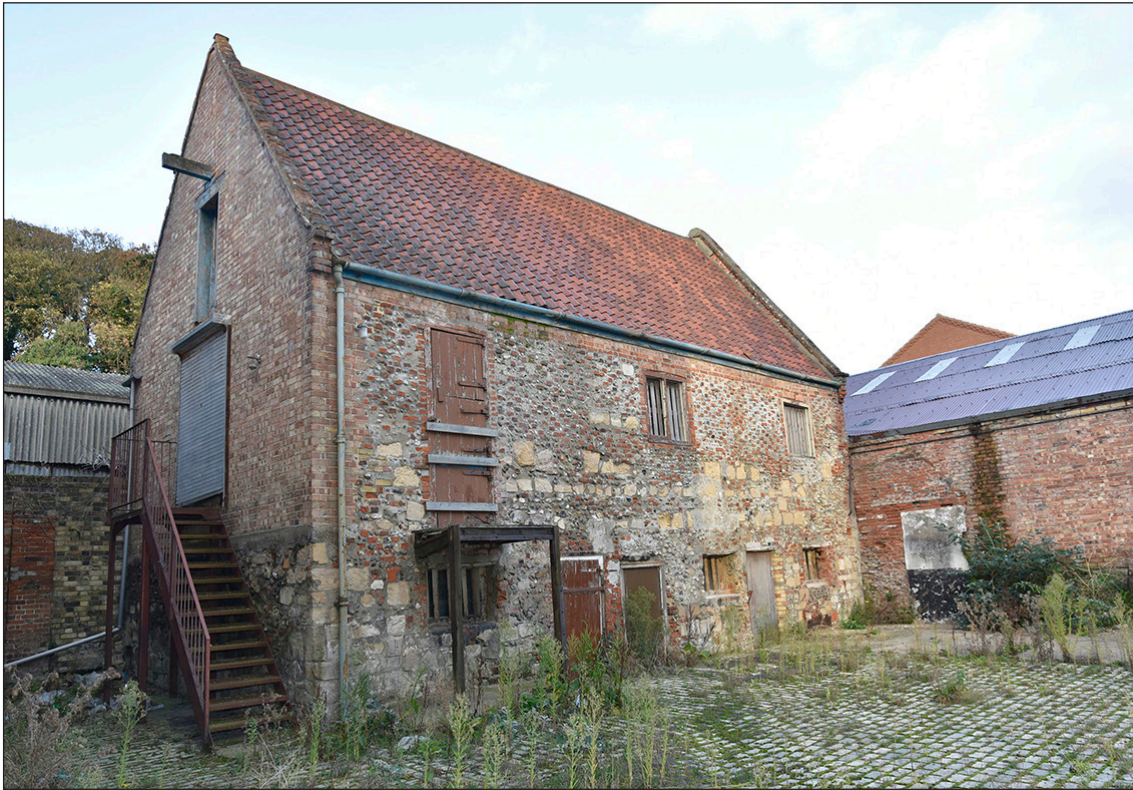
Figure 32: The southern gable end showing evidence of reconstruction following damage sustained during 1943. © Ark Property Services
