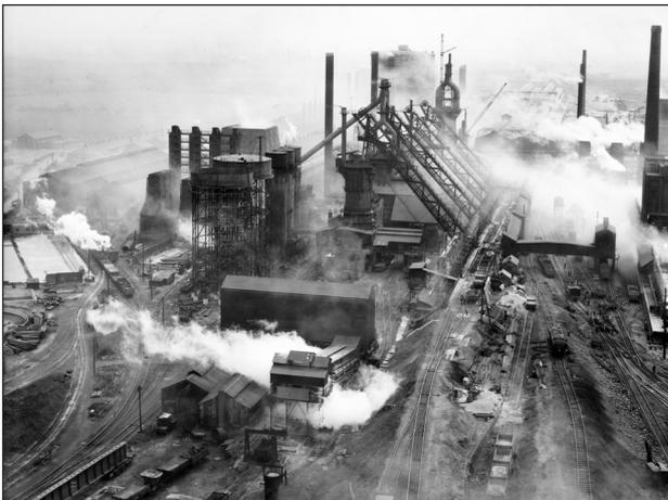
Figure 1. Blast furnaces at the former Normanby Park steelworks, Scunthorpe, 1950, illustrate the scale, complexity and environmental impact of the later integrated steelworks (EAW028583, Historic England Archive).
